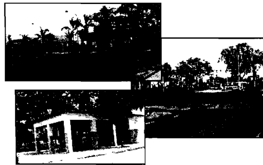
Carter Park Renovations
