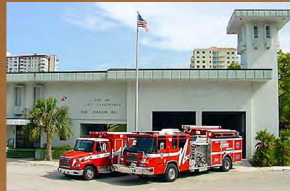
STATION 54 3200 NE 32 nd St.
