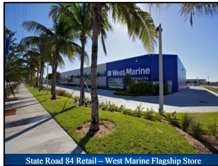
State Road 84 Retail – West Marine Flagship Store
