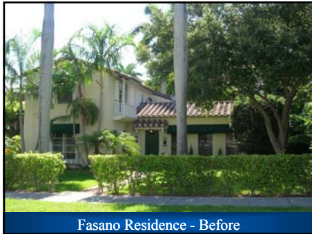
Fasano Residence - Before
