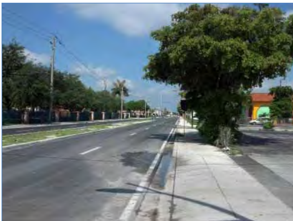
LOOKING WEST ALONG SISTRUNK BOULEVARD IN FRONT OF SUBJECT
