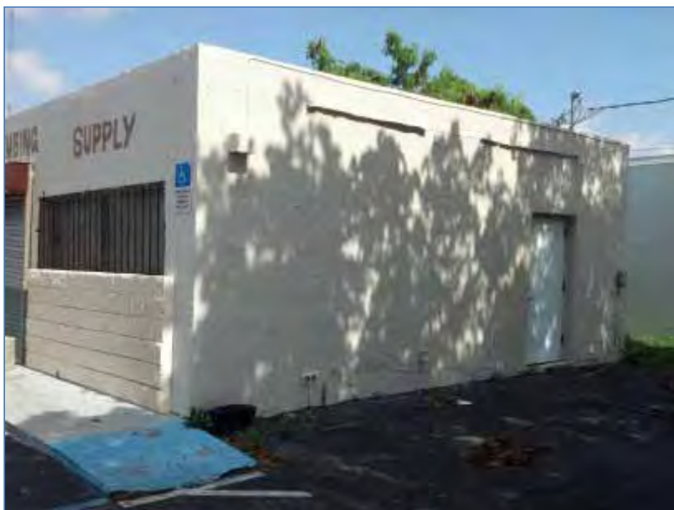
VIEW OF EAST SIDE OF BUILDING
