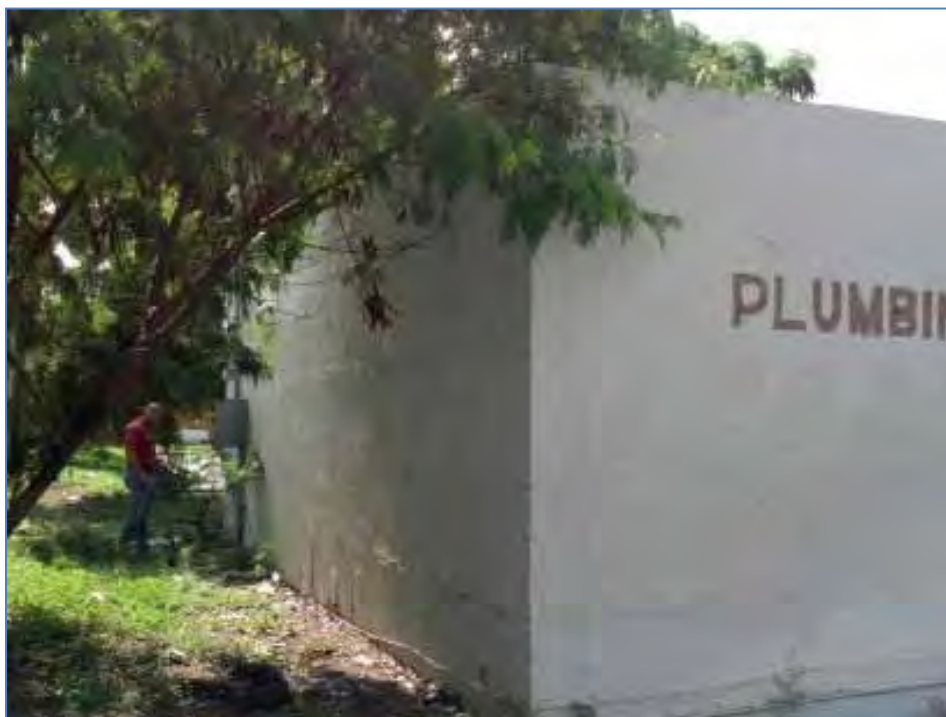
VIEW OF REAR OF BUILDING
