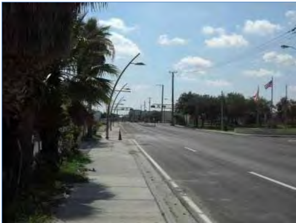
LOOKING EAST ALONG SISTRUNK BOULEVARD IN FRONT OF SUBJECT
