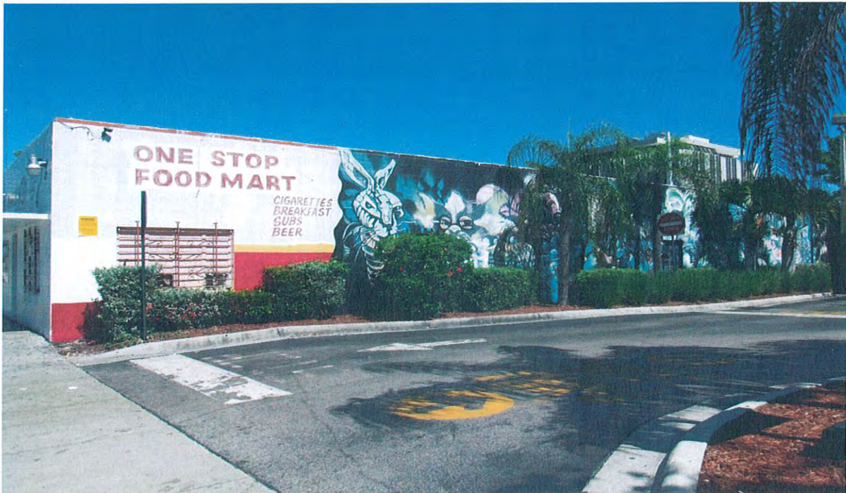
Existing West Façade of Building
