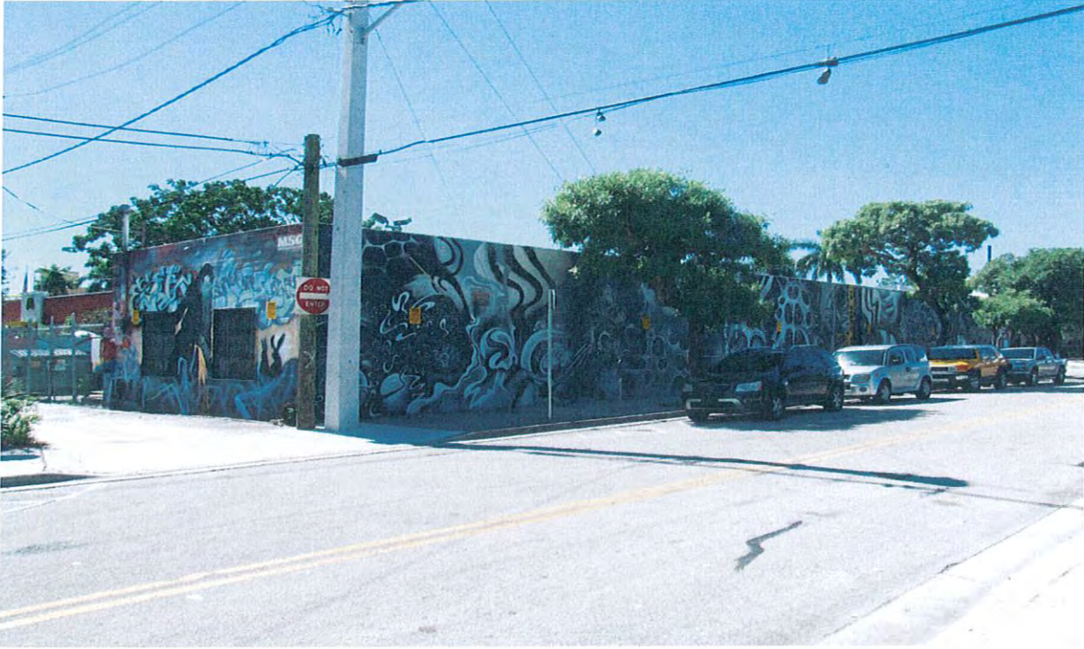
Art of Shade, LLC – 16 NW 1 Street - Existing South and East Façade of Building
