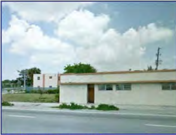
915 Sistrunk Boulevard, Before
