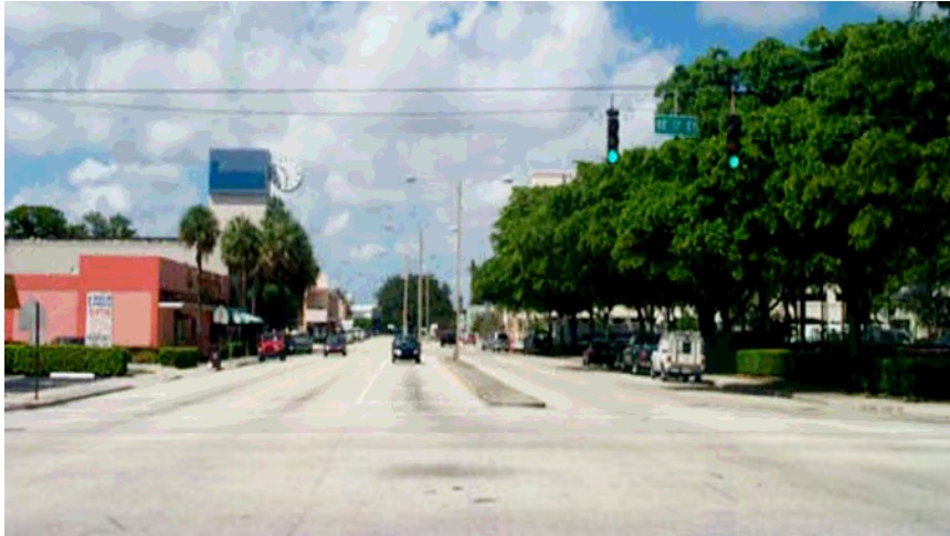
Figure 3.3, South Andrews Avenue at SE 17 th Street, Existing Condition, 2010
