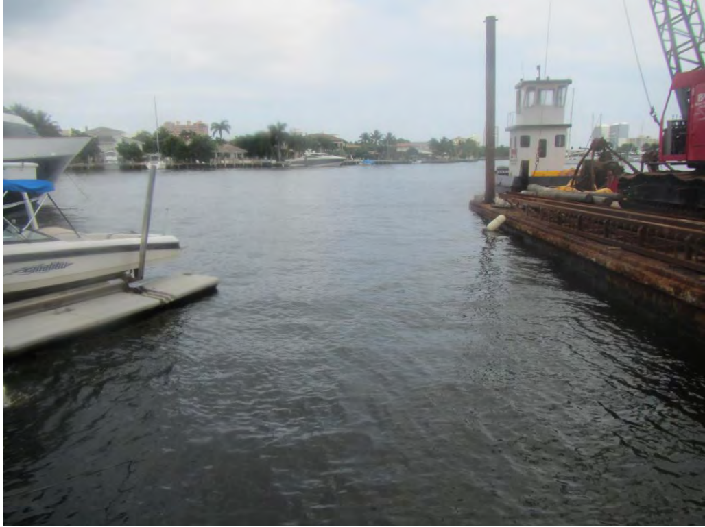
1. Northern property boundary, facing east.
