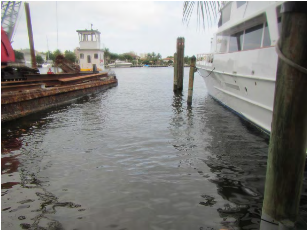
4. Southern property boundary, facing east.
