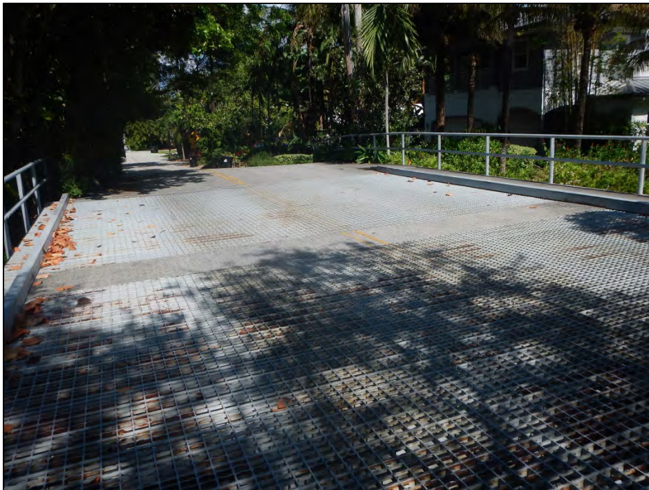
Open Steel Grid Deck
