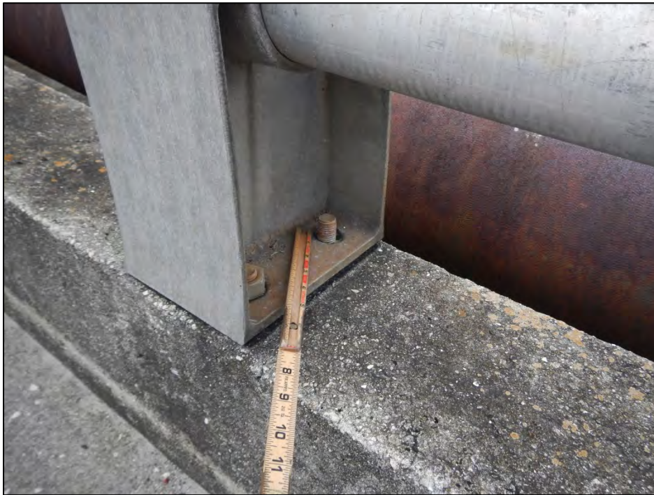
Photo 6 – West railing Post I-2L is missing 2 of 4 anchor bolt nuts.
