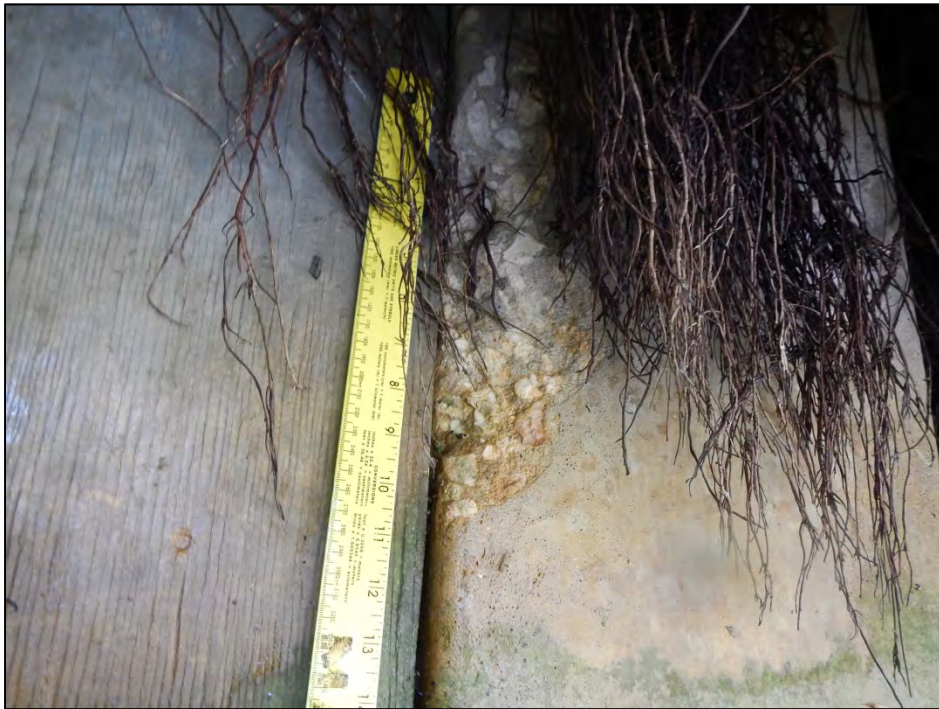
Photo 4 – Spall in Pile I-5.
