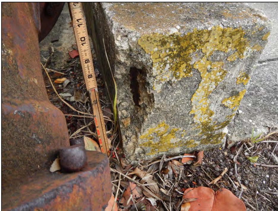
Photo 8 – West railing has a spall with exposed steel at the south end.
