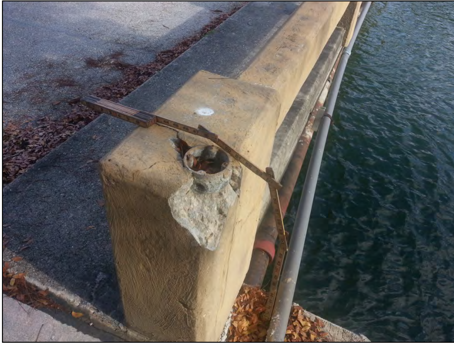
Photo 1 – Spall in Post 5-3, left.
