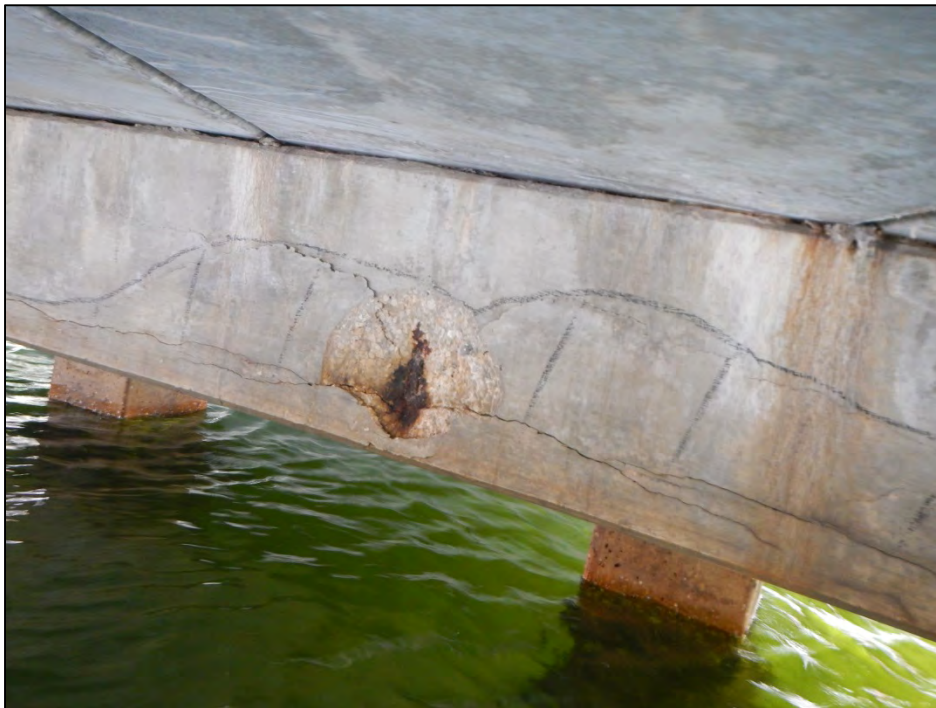
Photo 12 – Delamination/Spall with exposed rebar at Bent 2 cap.
