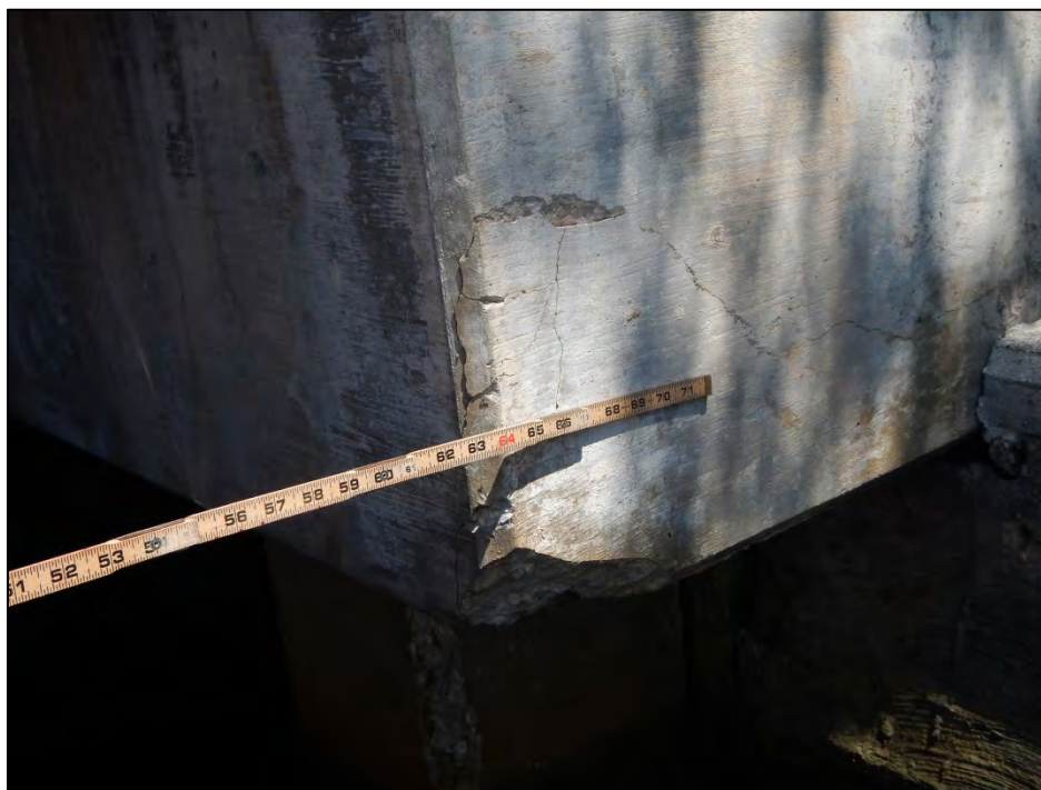
Photo 5 – Delamination in west end of Abutment I cap.
