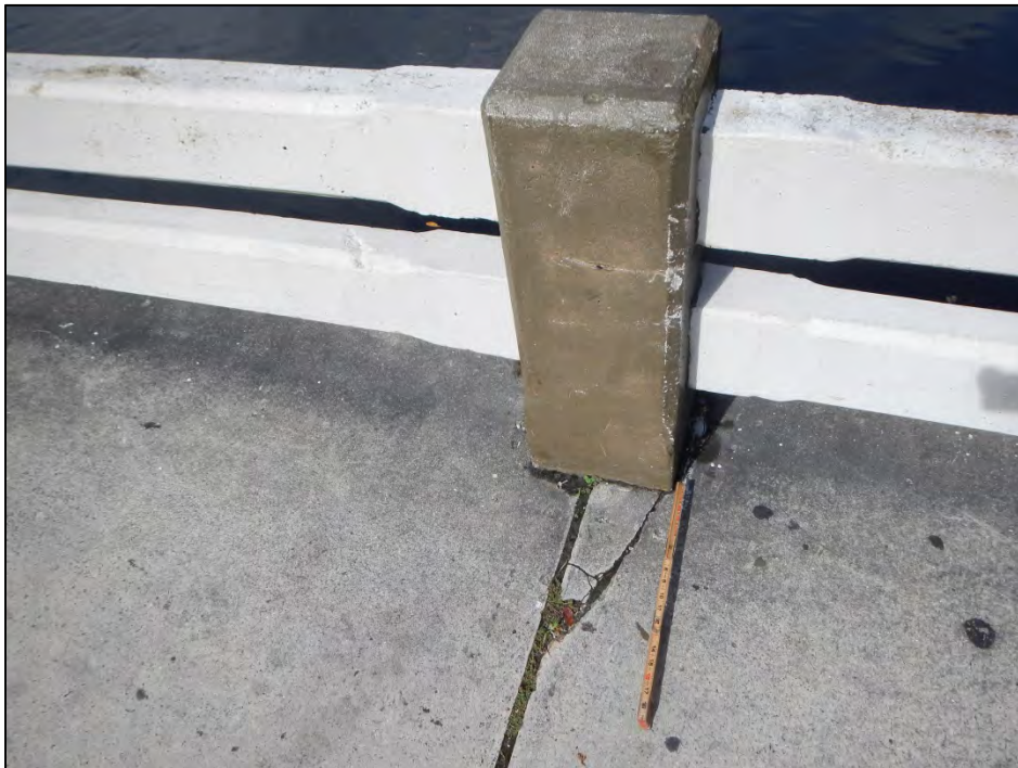
Photo 4 – West sidewalk delamination over Bent 3.
