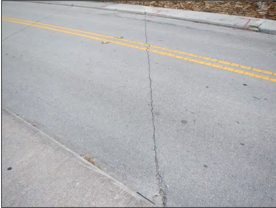
Photo 1 – End Bent 1 joint seal exhibits a transverse crack.
