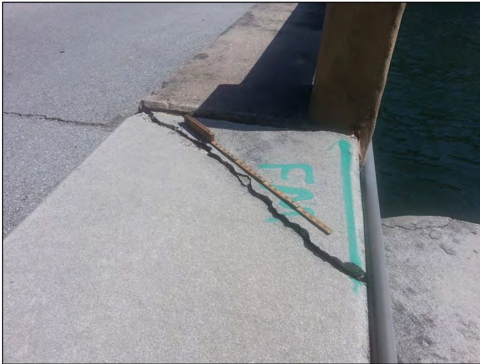
Photo 6 – Crack in the north approach sidewalk.
