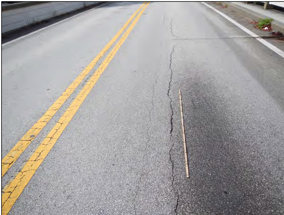
Photo 2 – Deck top longitudinal cracks.
