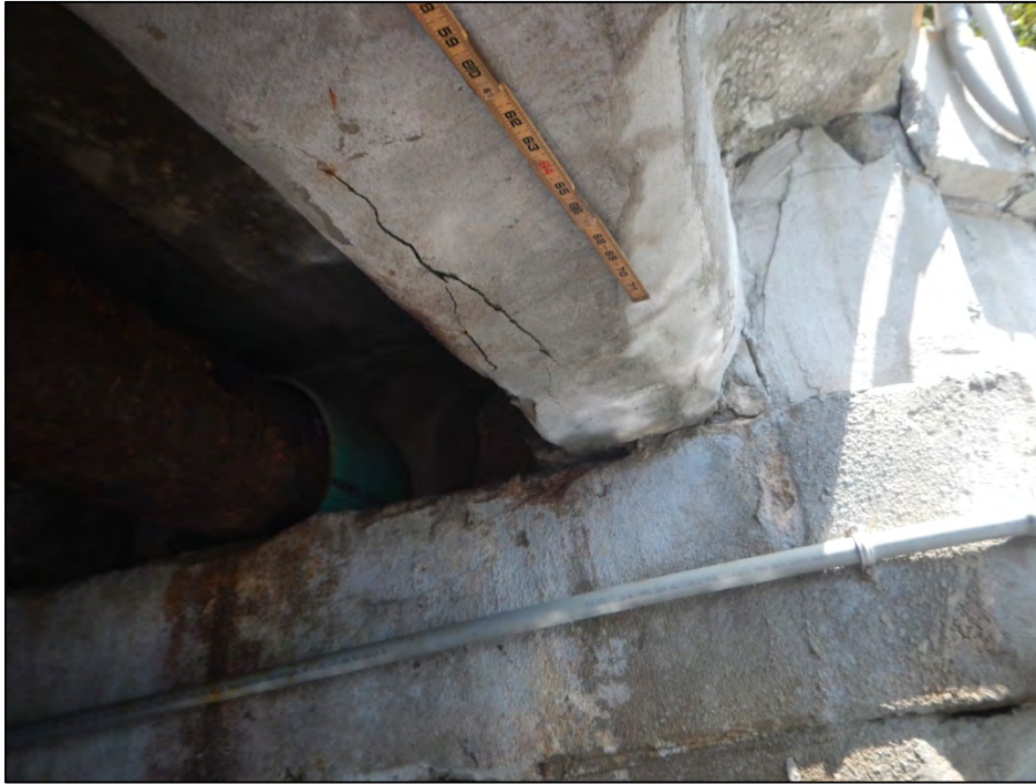
Photo 3 – Delaminated patch on Beam 6-4, right leg at Abutment 7.
