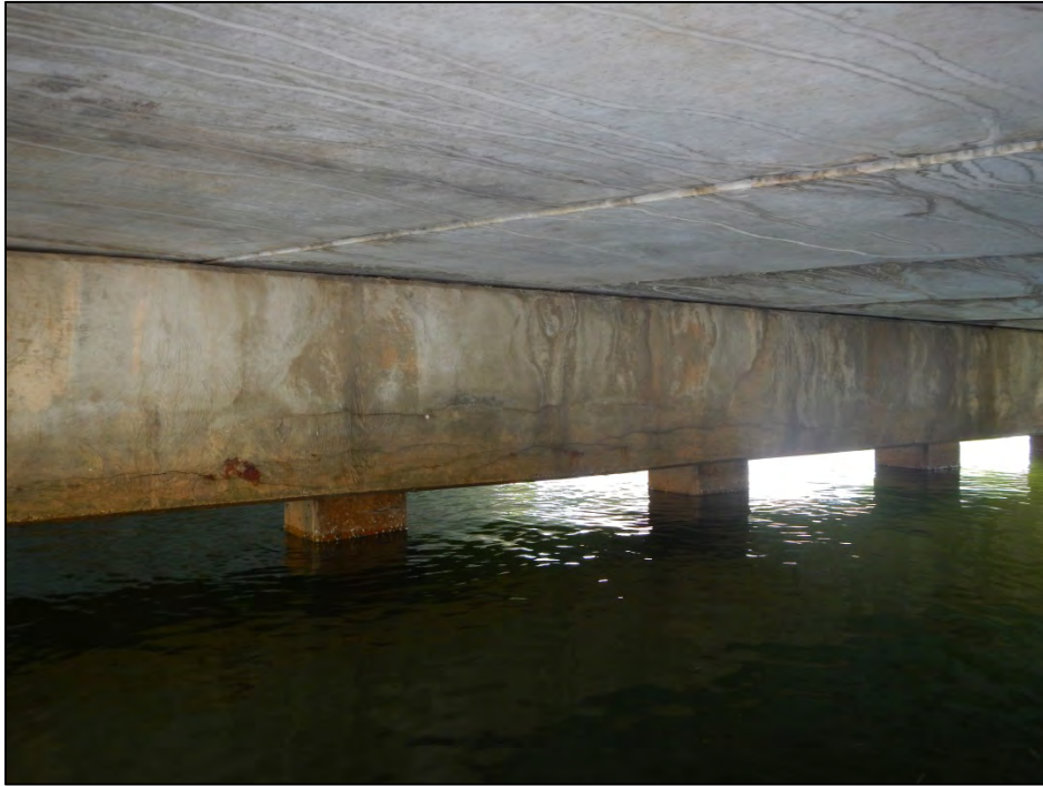
Photo 3 – Delamination in Bent 2 cap.
