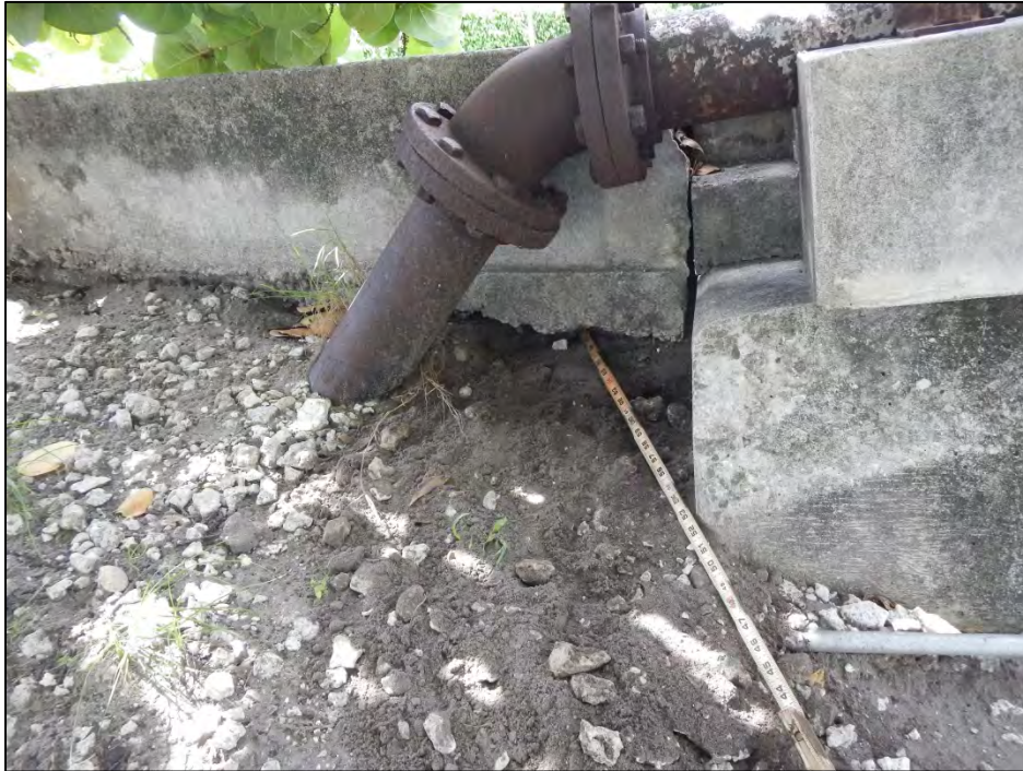
Photo 21 – Northeast corner approach slab undermining.
