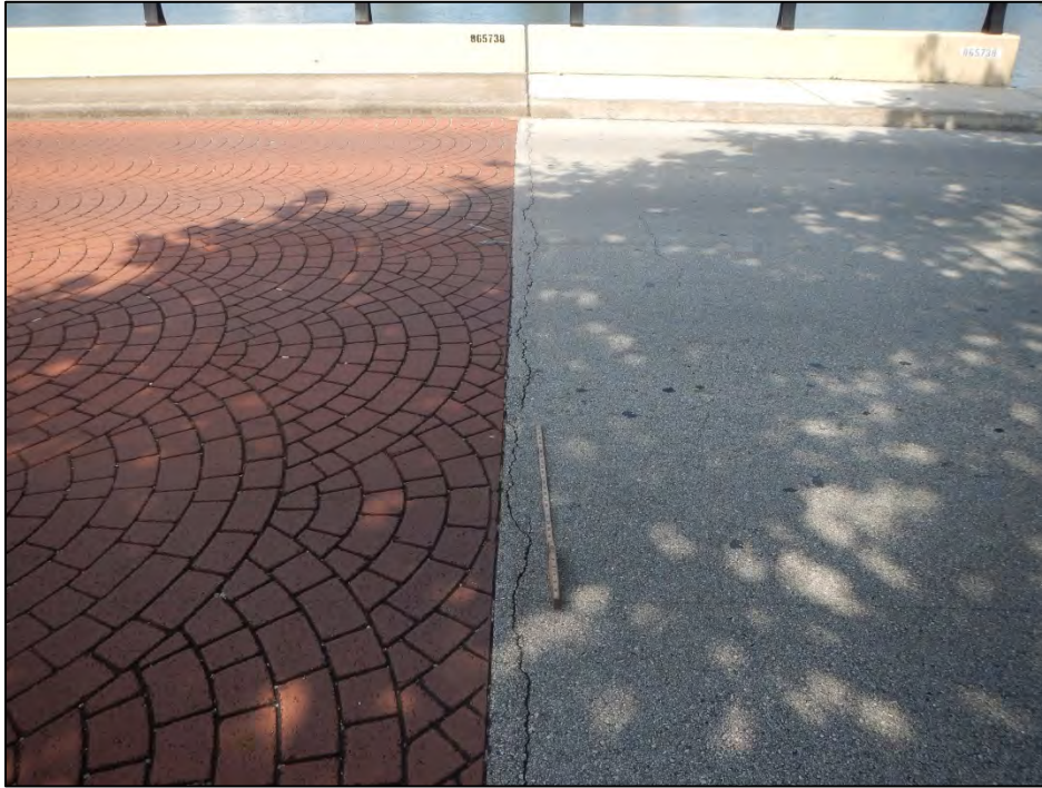
Photo 1 – Cracks in asphalt overlay at abutment. Note no striping present.
