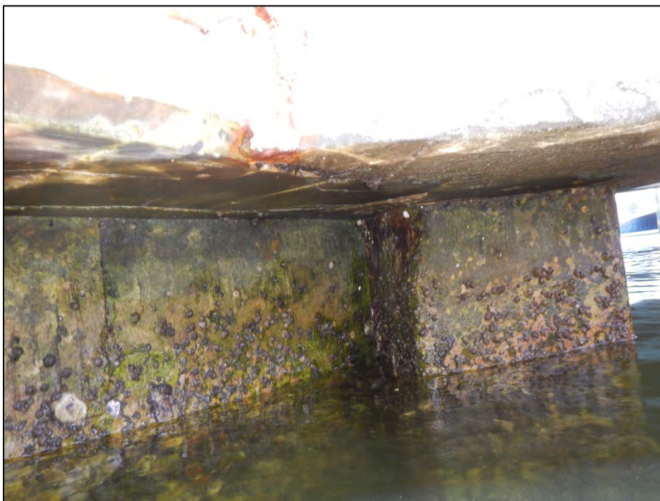
Photo 4 – Spall in Pile I-5.
