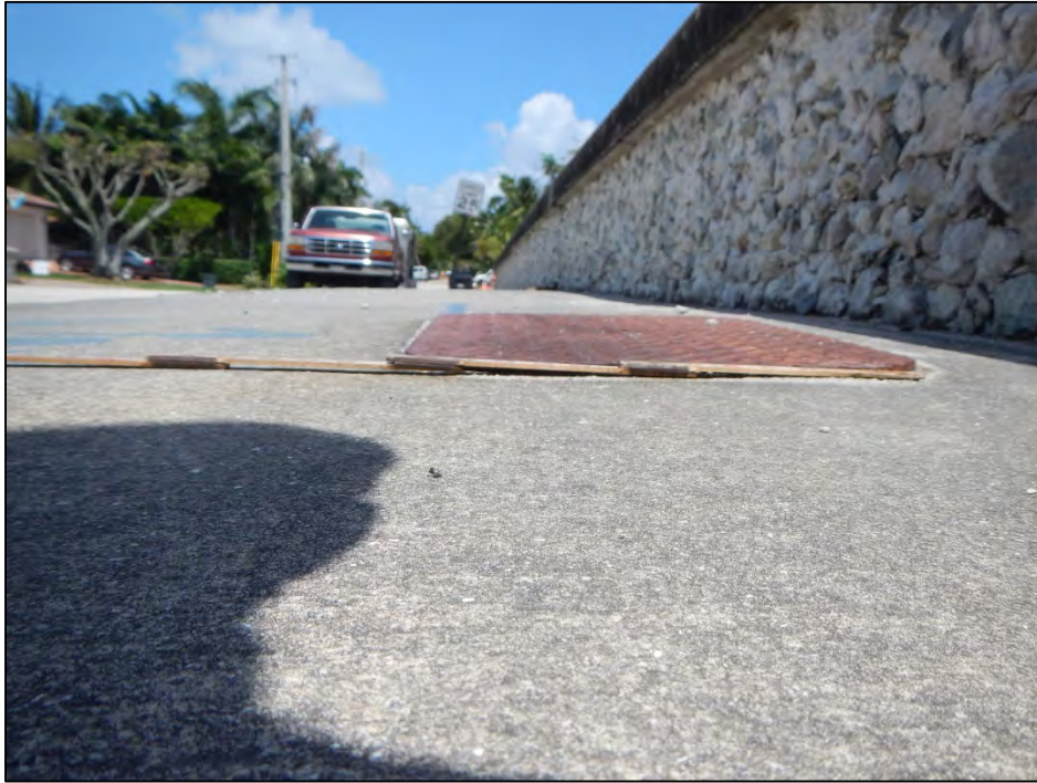
Photo 1 – Elevated water main access cover.
