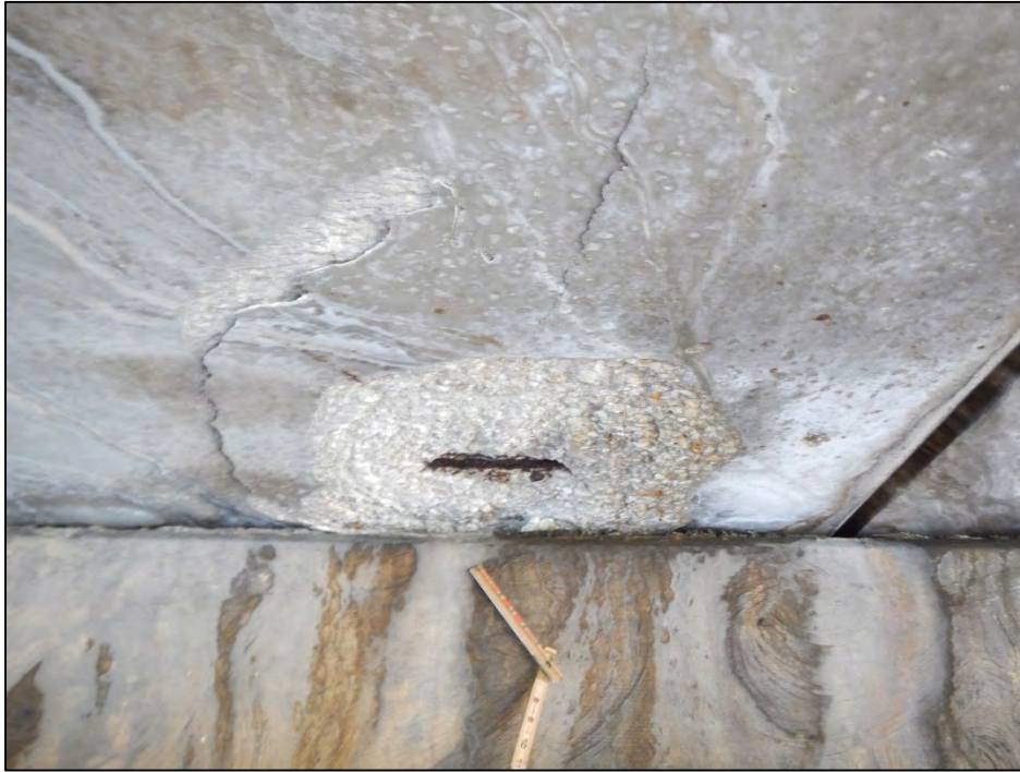
Photo 3 – Spall with exposed rebar in the underside of Slab Unit 1-2.
