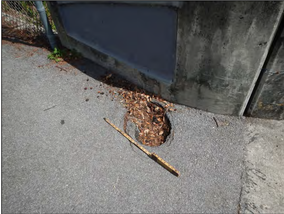
Photo 1 – The northwest approach sidewalk exhibits settlement.
