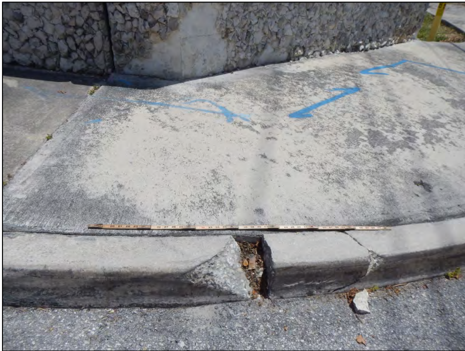
Photo 4 – Spall in the south approach sidewalk curb.
