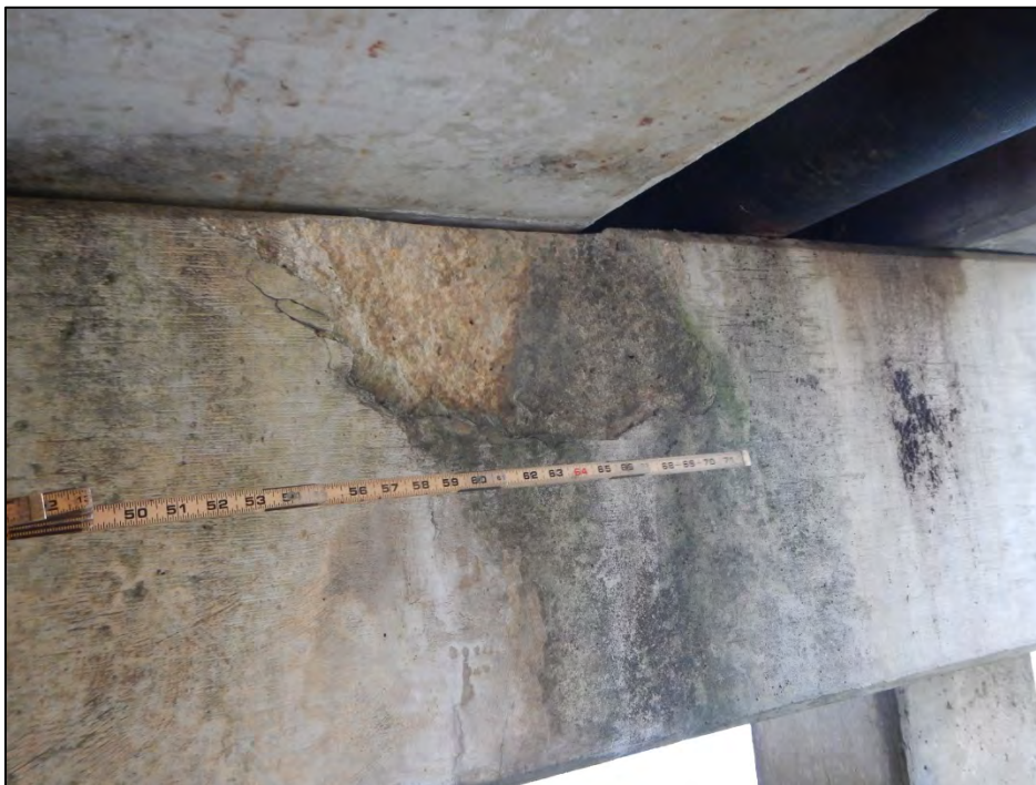
Photo 8 – Spall in south face of Bent 2 cap.
