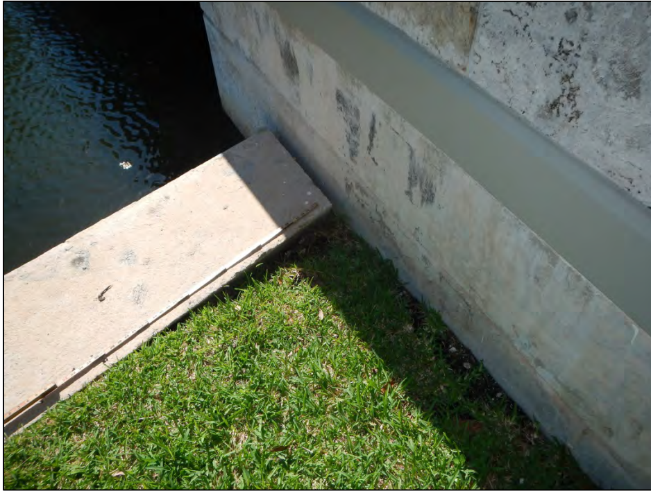
Photo 5 – Washout at southeast bulkhead.
