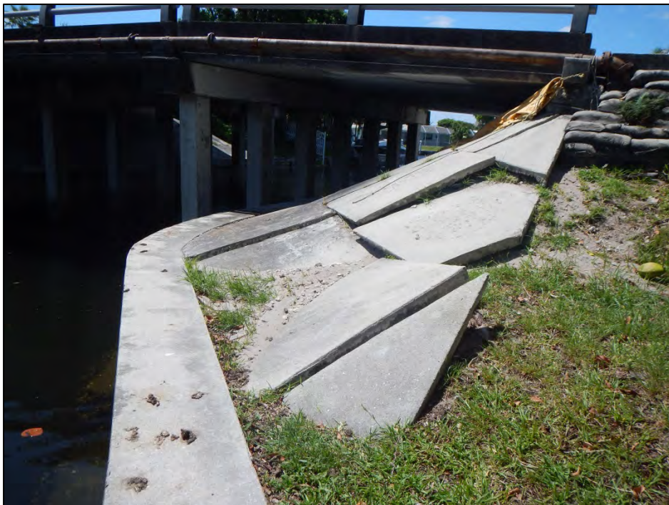
Photo 24 – Northwest slope protection displacement.
