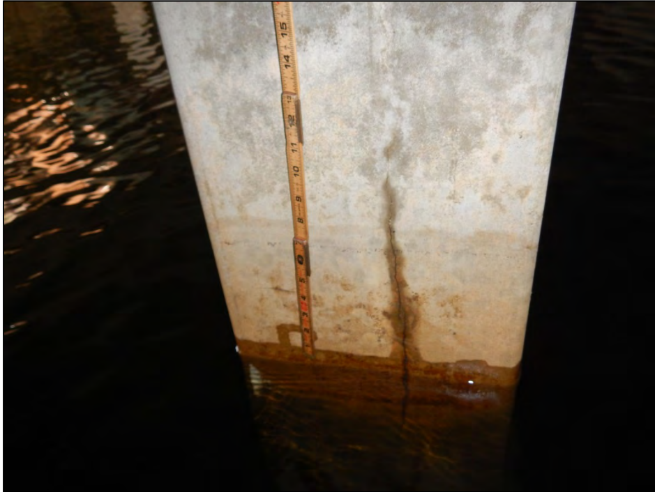
Photo 7 – The east face of Pile 2-4 exhibits a vertical crack.
