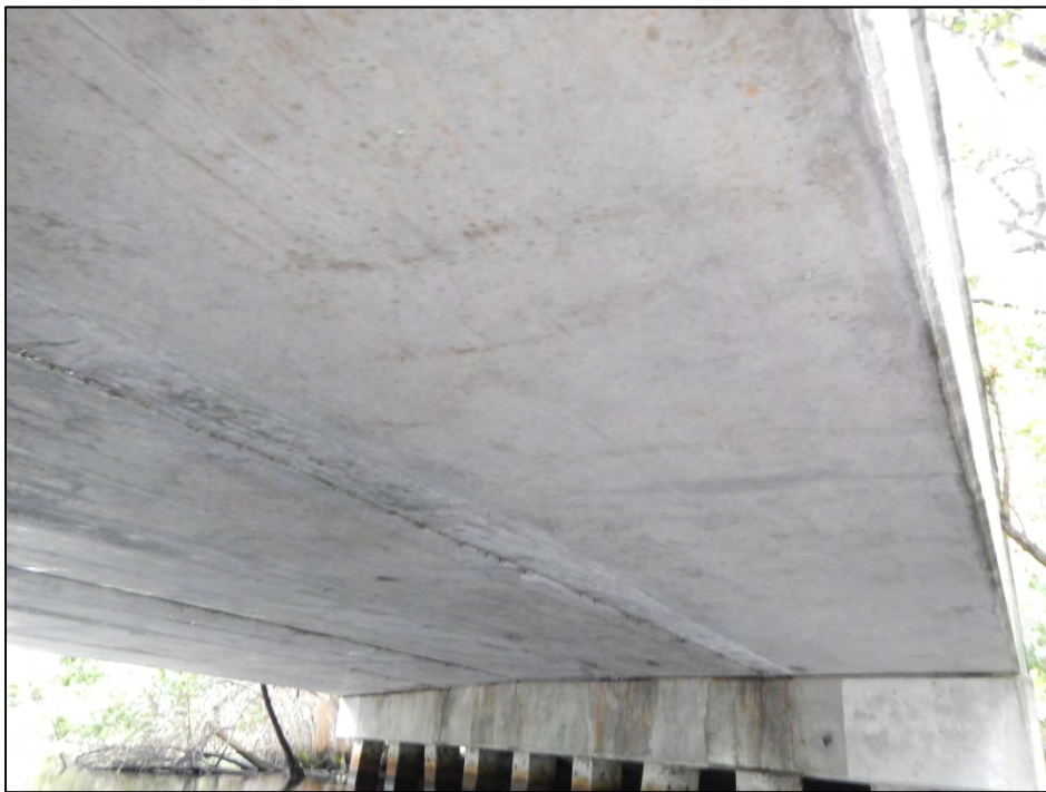
Photo 10 – Span 2 deck underside exhibits hairline cracks with efflorescence.
