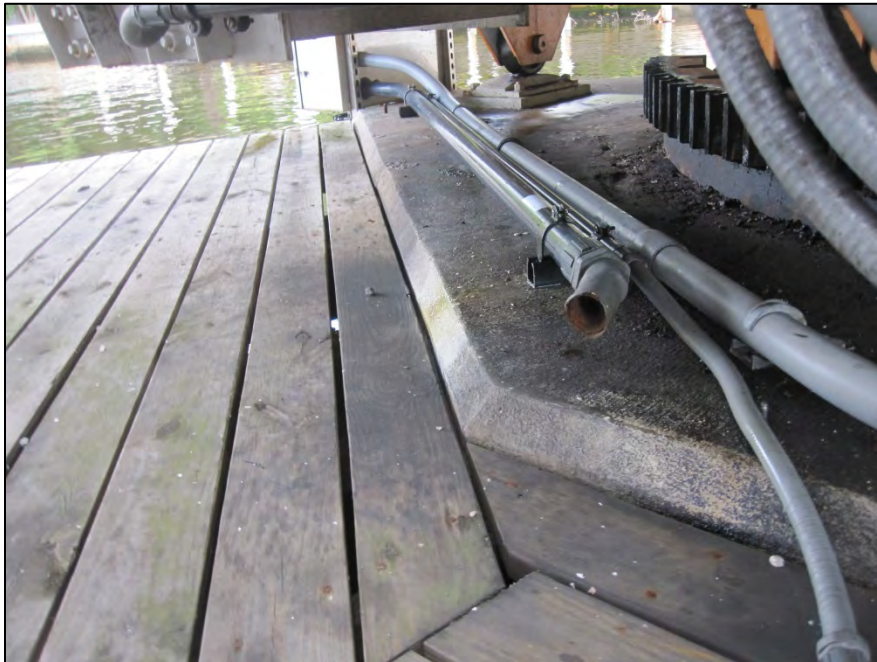
Photo 26 – Cut flexible conduit at within the machinery area.
