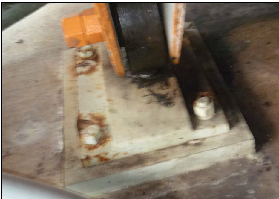
Photo 18 – West Elevator Wheel: Note surface corrosion on Strike Plate.
