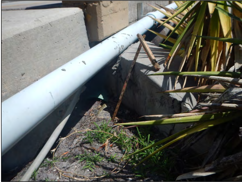
Photo 5 – Area of washout around the utilities at the northwest wingwall.
