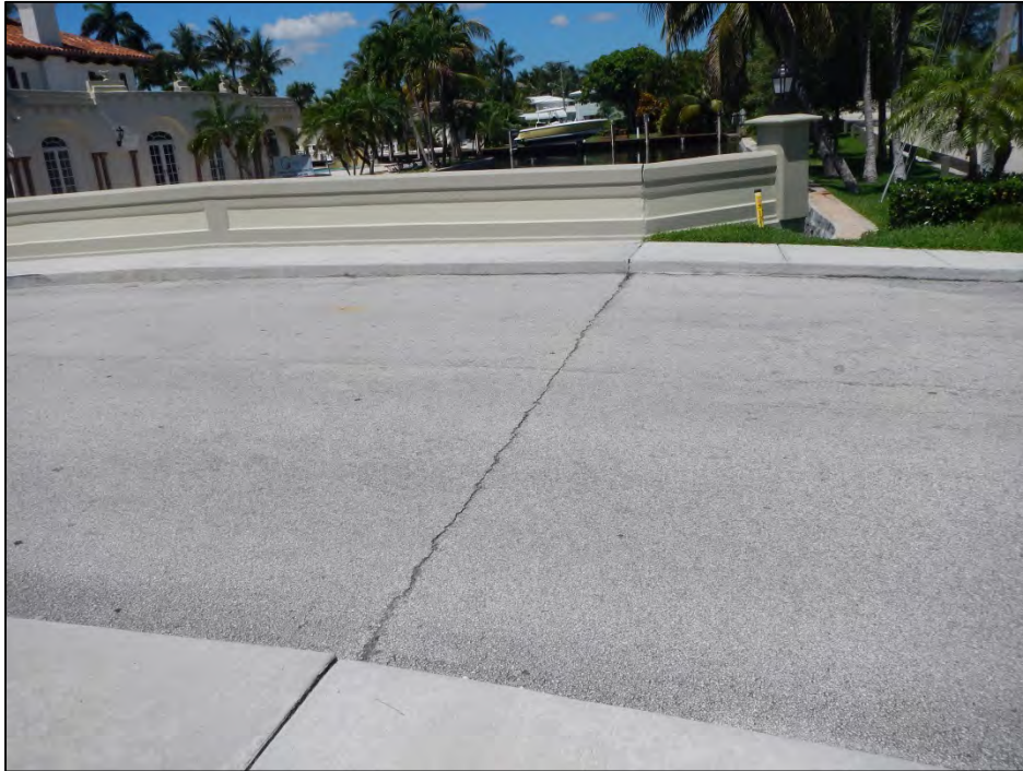
Photo 1 – Cracks in asphalt surfacing over joints.
