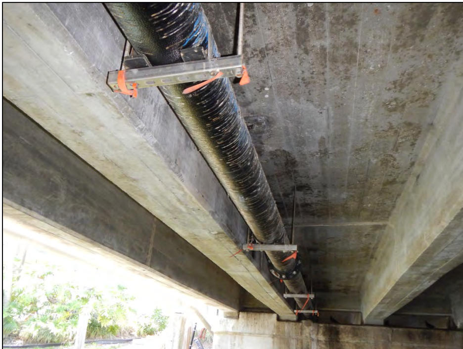
Utility Pipe Mounted under South Side of Bridge
