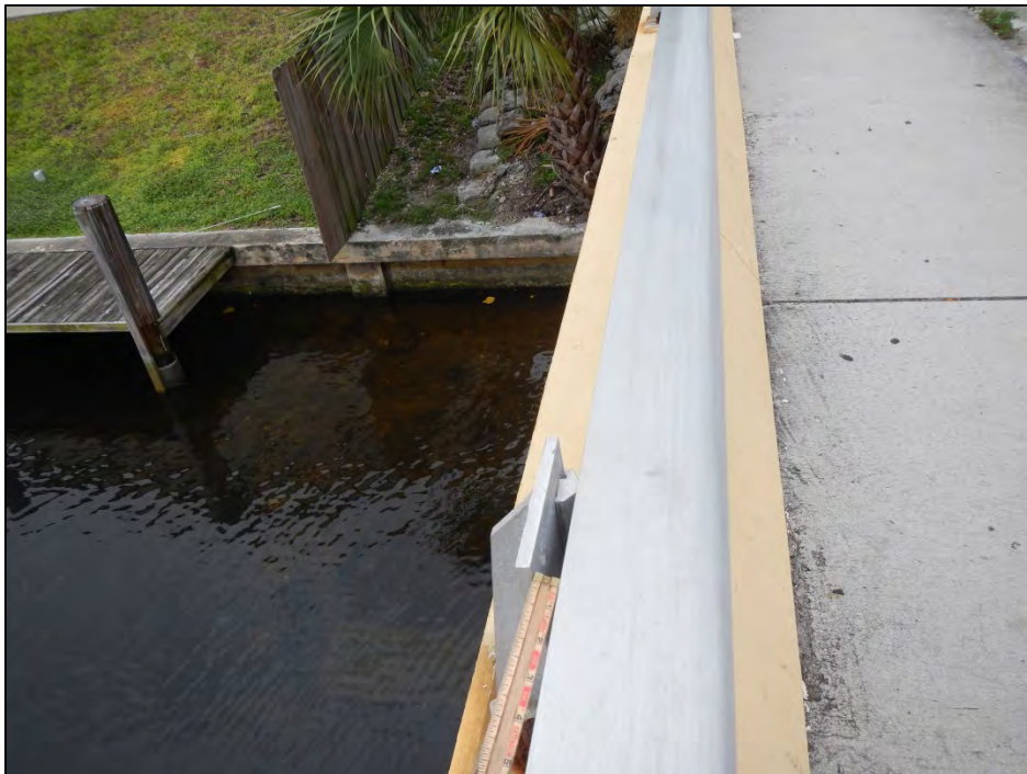
Photo 4 – Bolts are missing at Post I-3R.
