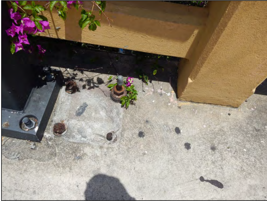
Photo 1 – The left sidewalk between Railing Posts 1-4 and 1-5 exhibits 4 protruding steel rods.
