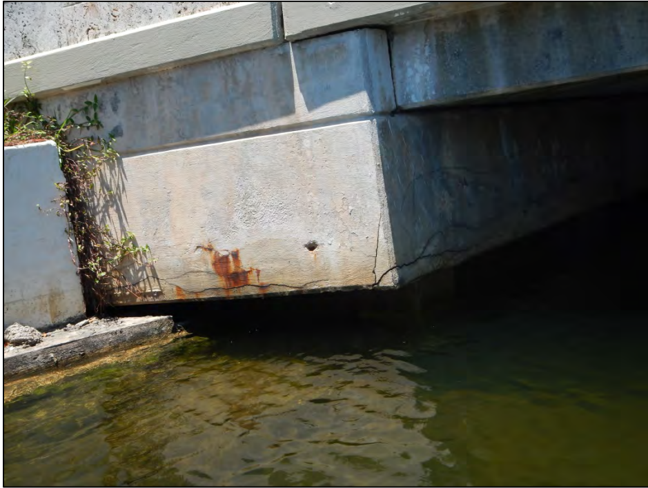
Photo 5 – Delaminated area in Abutment I cap.
