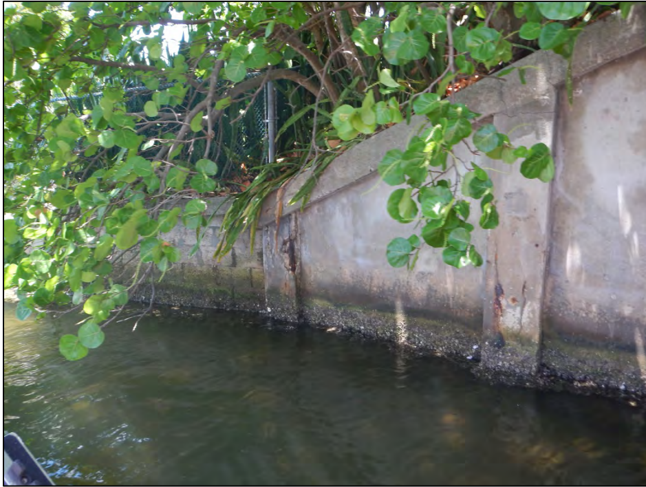
Photo 11 – Spalls in the piles at the northwest wingwall.
