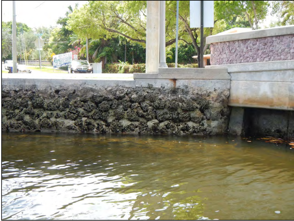
Photo 7 – Cracked and delaminated area at the transition to the southwest wingwall.
