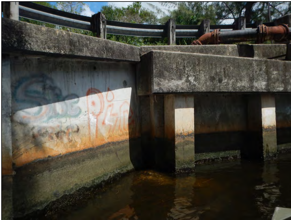
Photo 8 – The southwest backwall exhibits diagonal cracks and graffiti.
