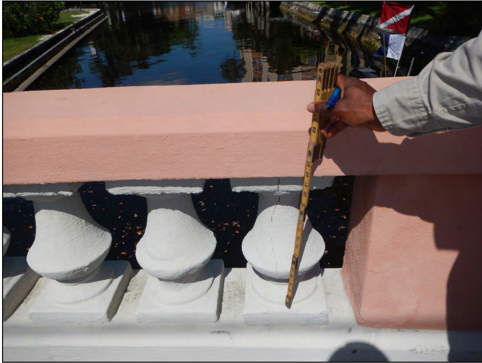
Photo 7 – Crack on 7 th spindle from south at west railing.
