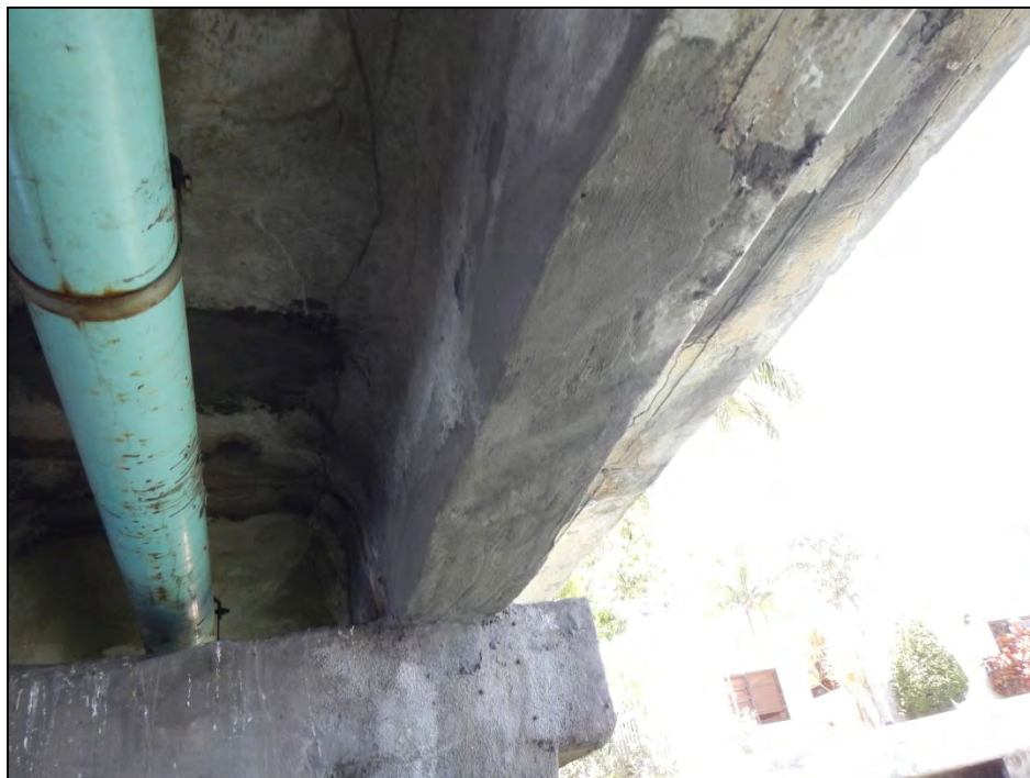
Photo 2 – Typical patching on the T-beams.
