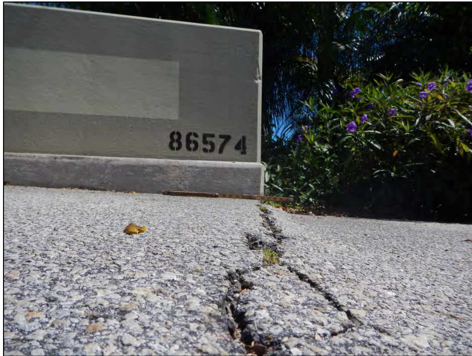
Photo 15 – Settlement of west roadway in relation to west approach slab.
