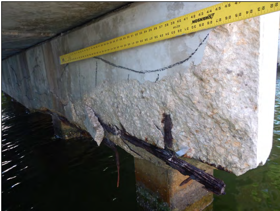
Photo 10 – Spall with exposed rebar at Bent 2 cap.
