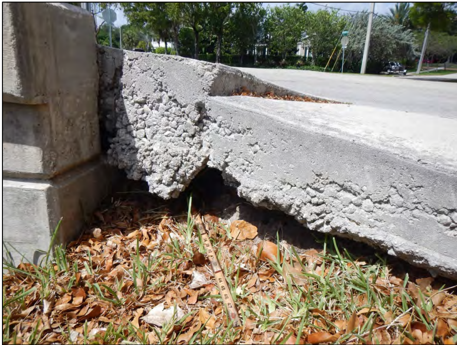
Photo 6 – Undermining at the northwest approach sidewalk.
