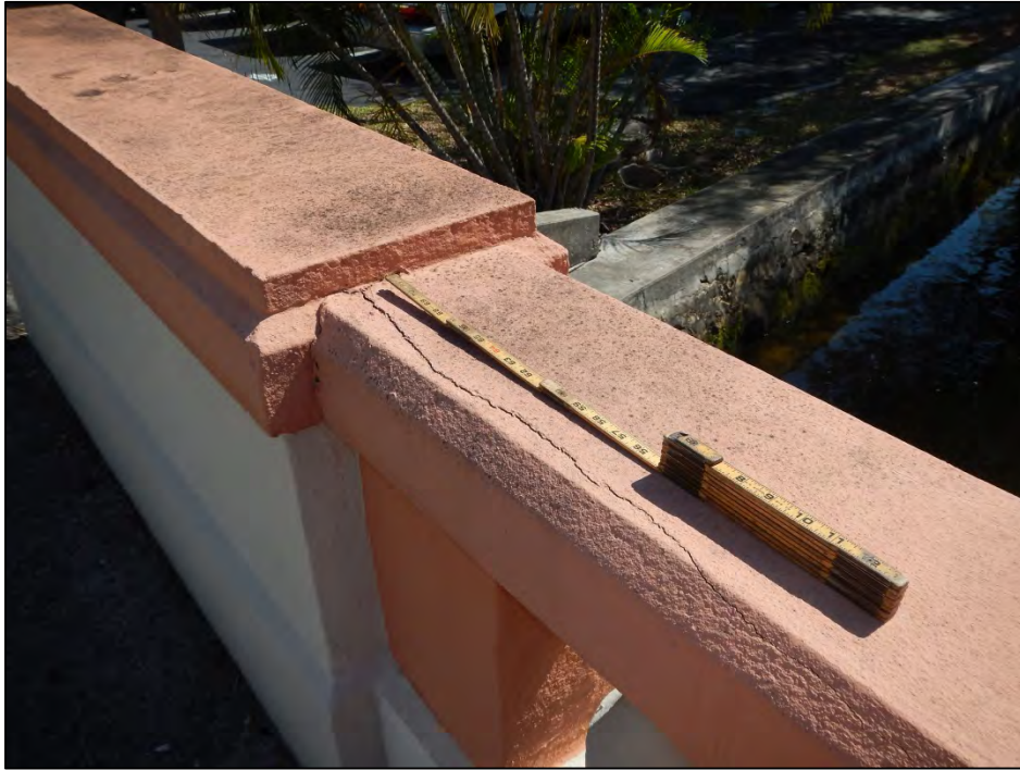
Photo 5 – Crack at north end of east railing.
