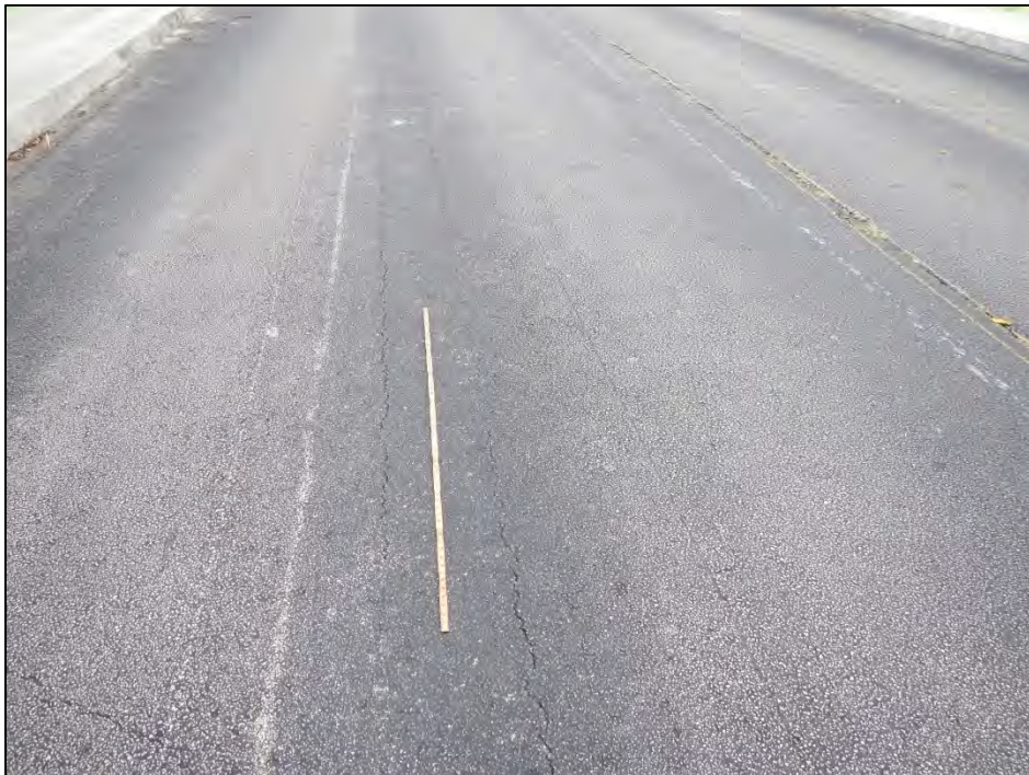
Photo 2 – Deck top longitudinal cracks at Span 4.
