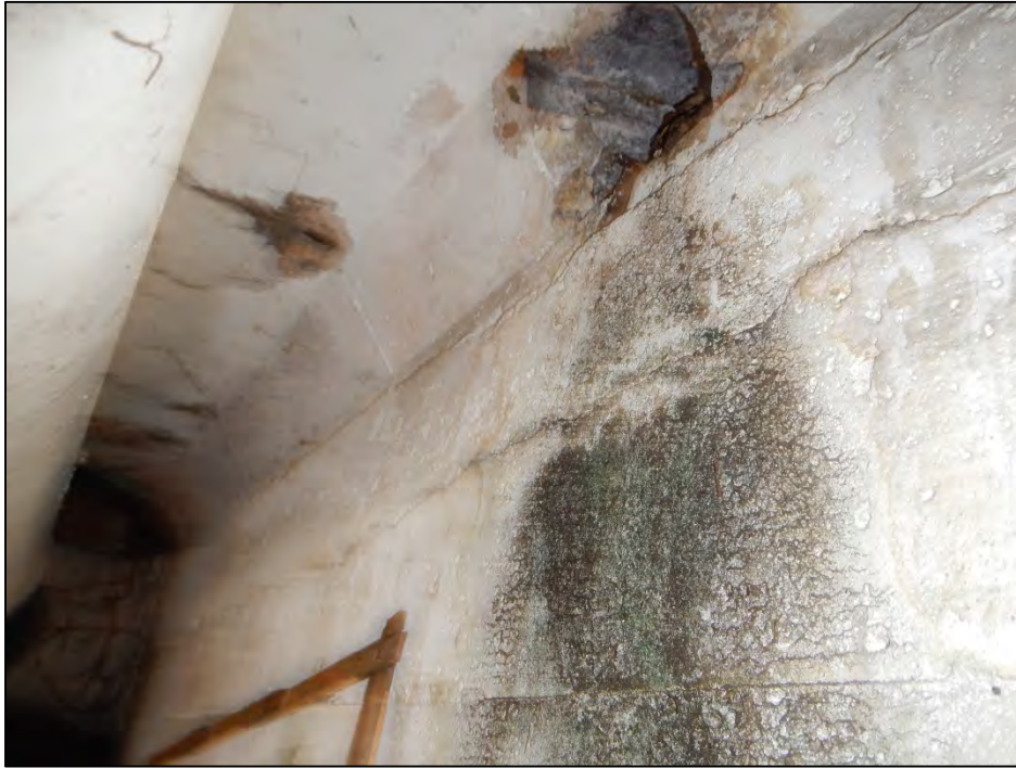
Photo 15 – Beam 1-8 over Abutment 1 exhibits a horizontal crack.
