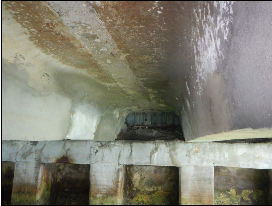
Typical Double T-Beam
