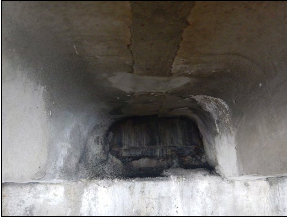
Photo 5 – Abutment 9 cap cracks with corrosion staining.
