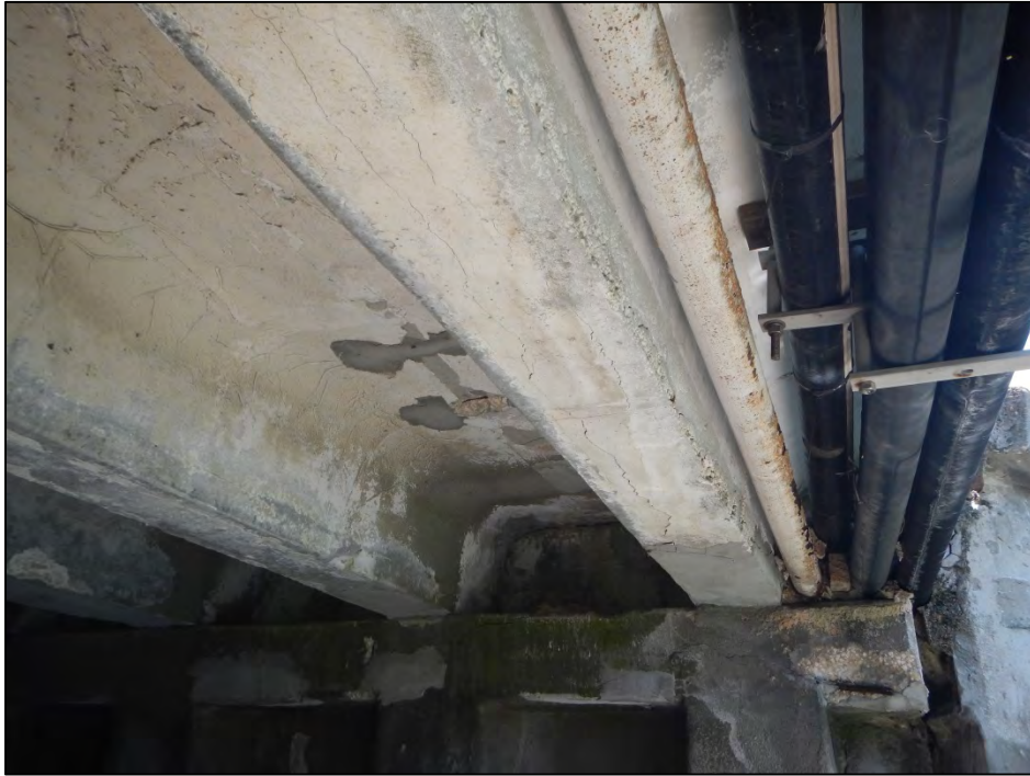
Typical Double T-Beam. Note Utilities Mounted at West Fascia
