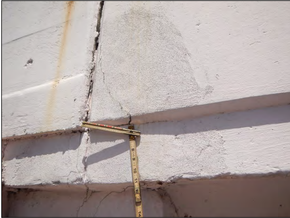
Photo 1 – The west face of the left barrier over End Bent 4 exhibits a delamination.
