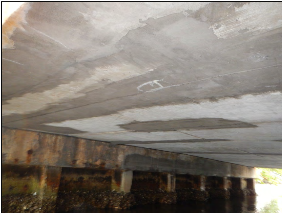
Photo 12 – Typical repaired areas at deck underside and abutment cap.
