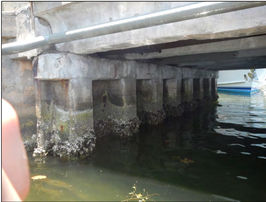
Photo 4 – Delamination with corrosion staining on the cap at Abutment 1.
