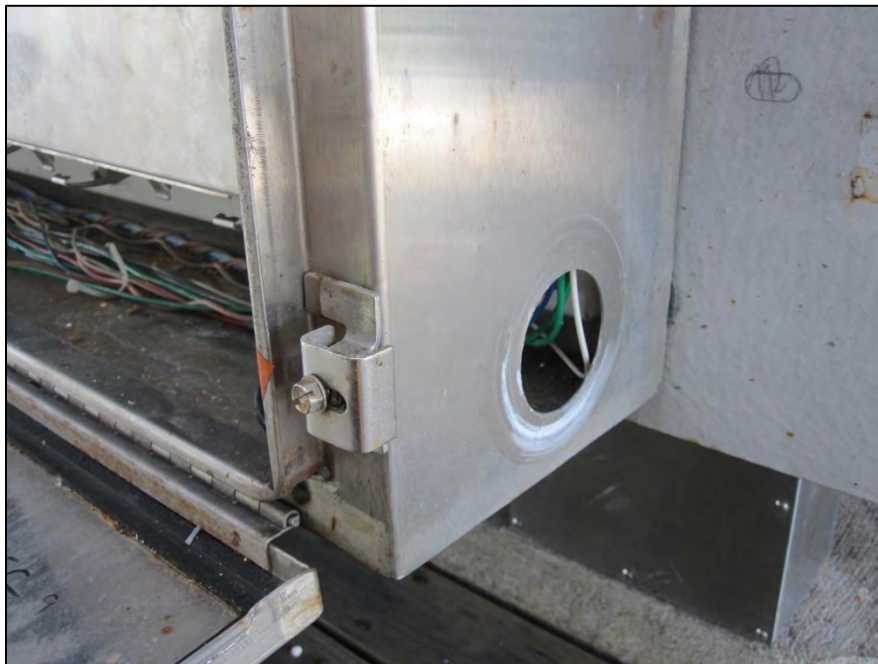
Photo 24 – Unplugged hole at the terminal box in the machinery area.
