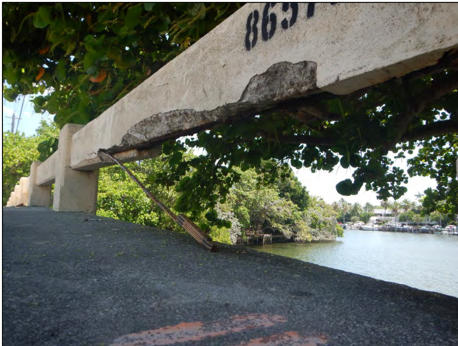
Photo 2 – Spalled concrete railing with exposed reinforcing steel.
