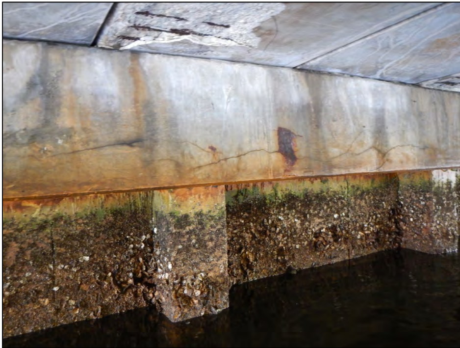
Photo 6 –Delamination at Abutment 4 cap.
