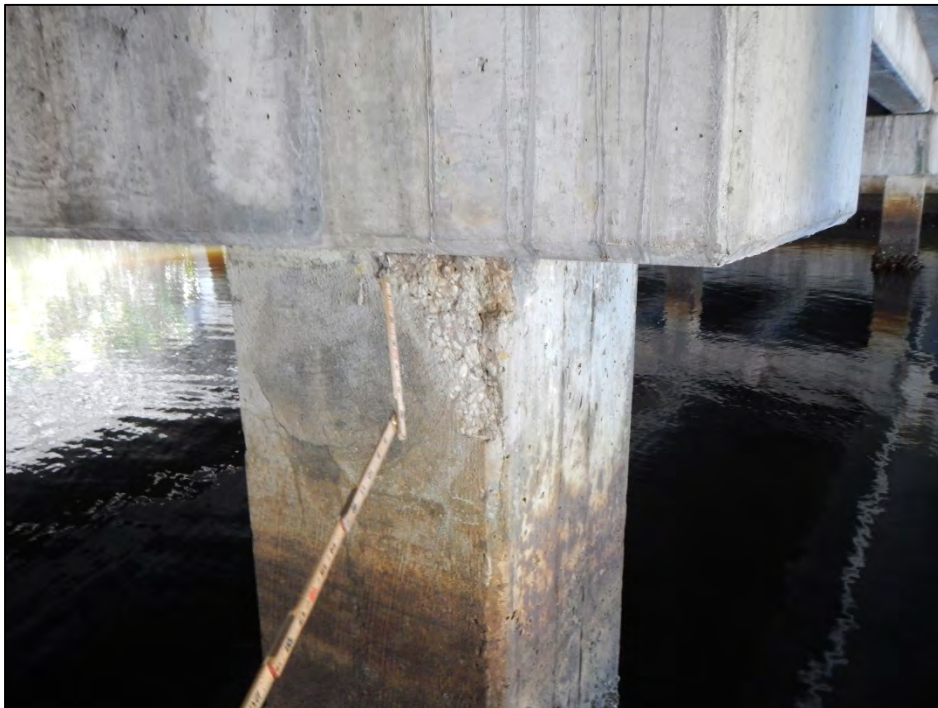
Photo 12 – The southeast corner of Pile 3-7 exhibits a delamination.
