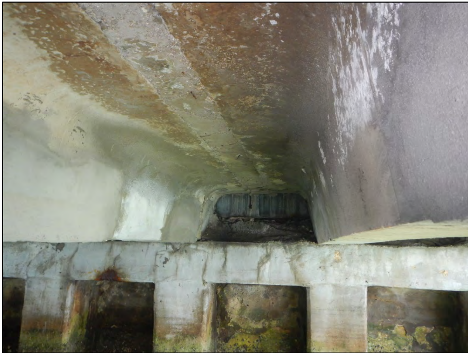
Photo 4 – Spall in Abutment I cap.
