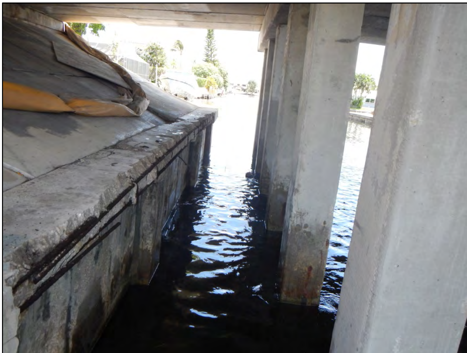
Photo 26 – West bulkhead cap at End Bent I exhibits a spall/delamination with exposed steel.
