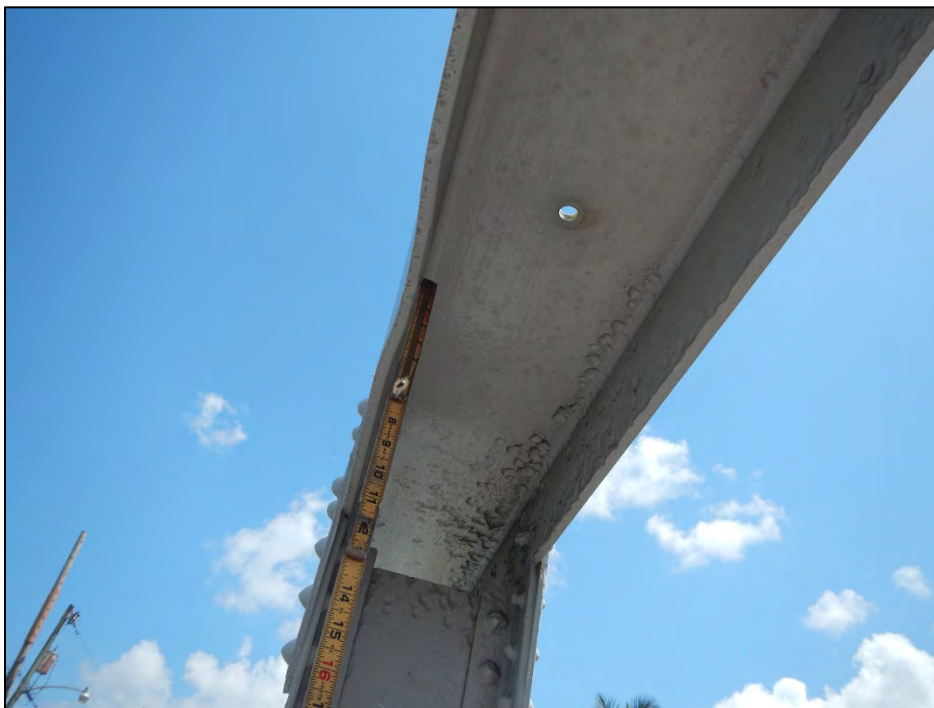
Photo 13 – Bent west top chord adjacent to U6.
