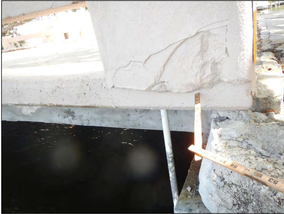
Photo 1 – Post I-I left exhibits a spall/delamination.
