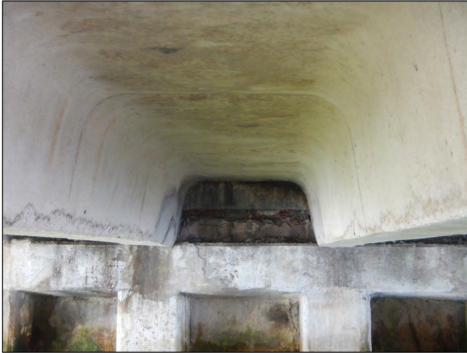
Typical Double T-Beam
