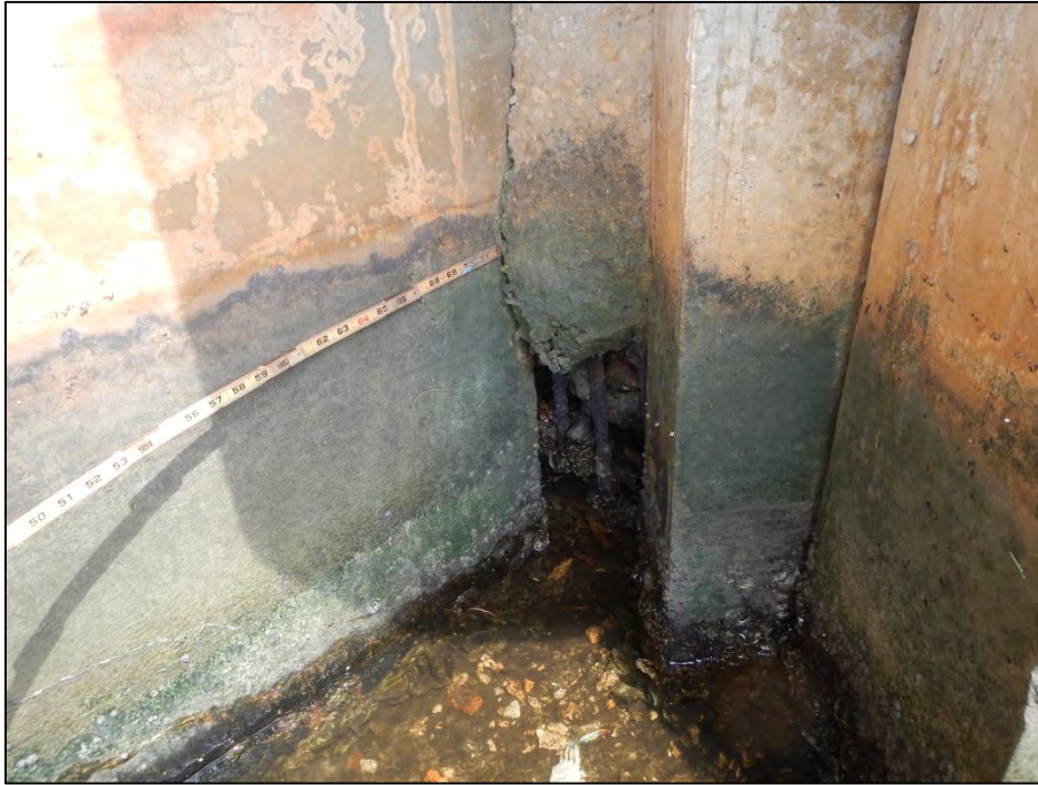
Photo 7 – The southwest retaining wall is open and exposes corroded steel.
