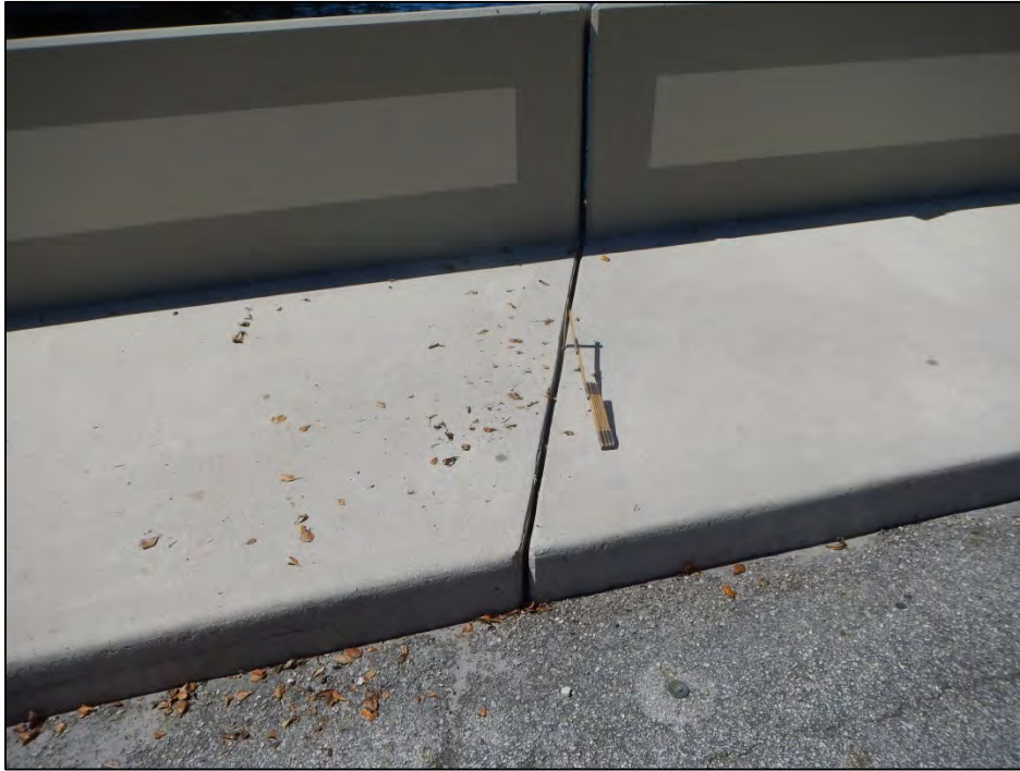
Photo 3 – Dirt and debris accumulating in failed sidewalk and curb sealant.
