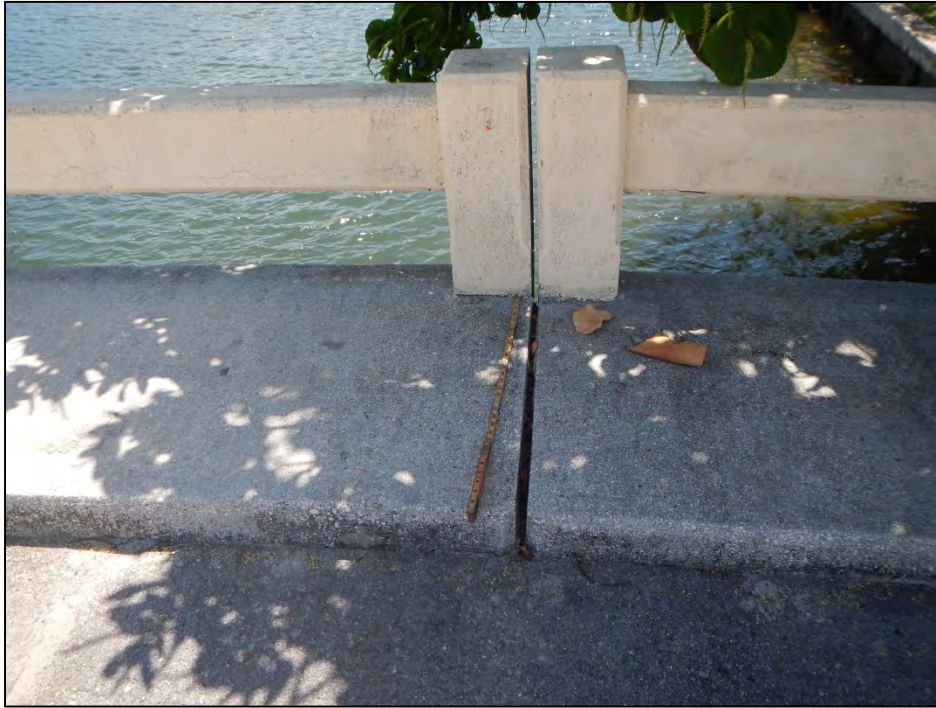
Photo 3 – Deteriorated joint over the right sidewalk.
