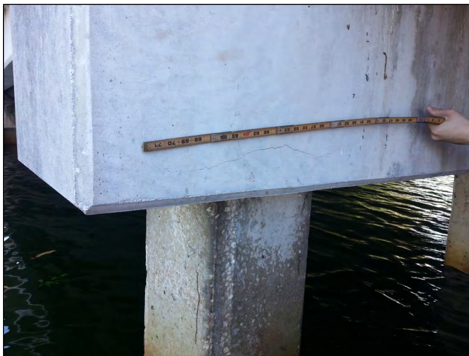
Photo 7 – Delamination in east end of north face of Bent 2 cap.
