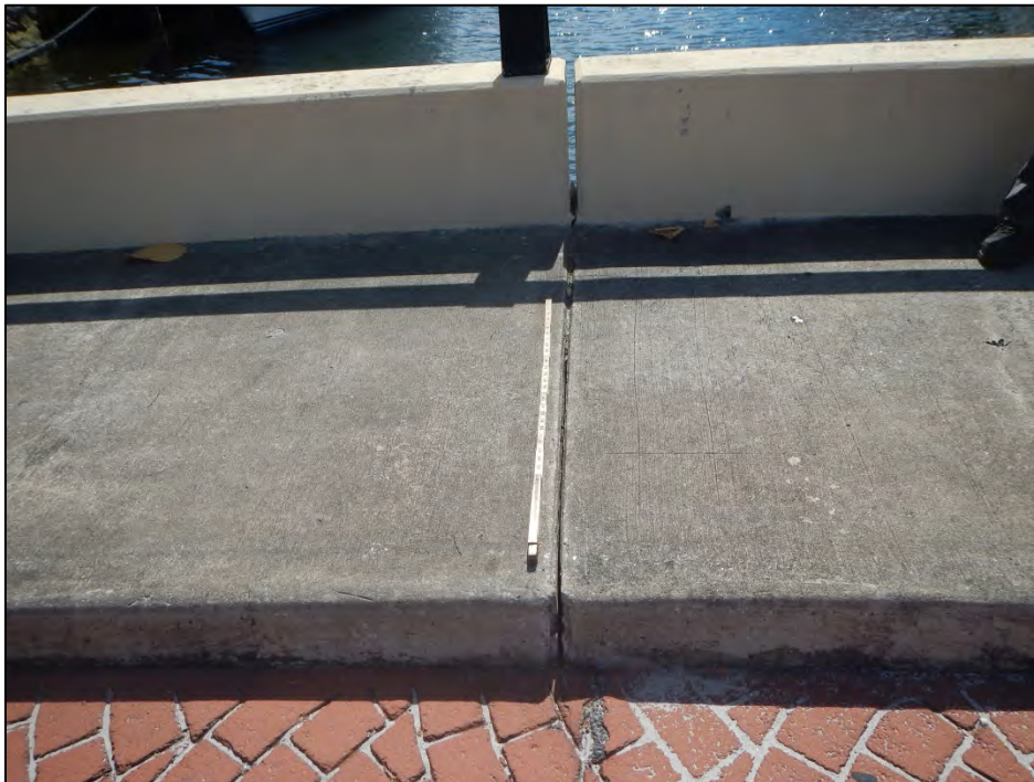
Photo 2 – Sidewalk joints not sealed; they are filled with dirt and debris.
