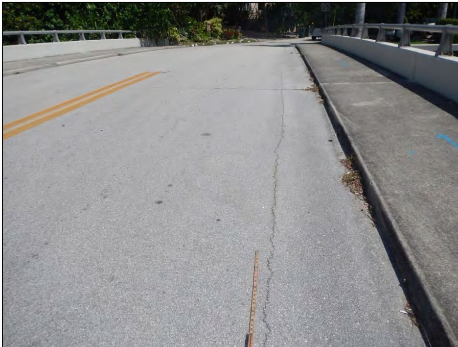
Photo 2 – Longitudinal cracks in asphalt overlay above slab unit joints. Note vegetation at the curb line.
