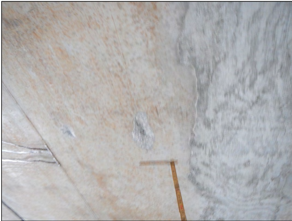
Photo 6 – Slab 3-3 spalls mid-span.
