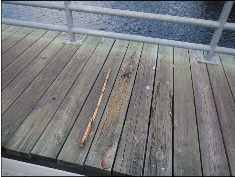
Photo 3 – Decay at the west sidewalk.
