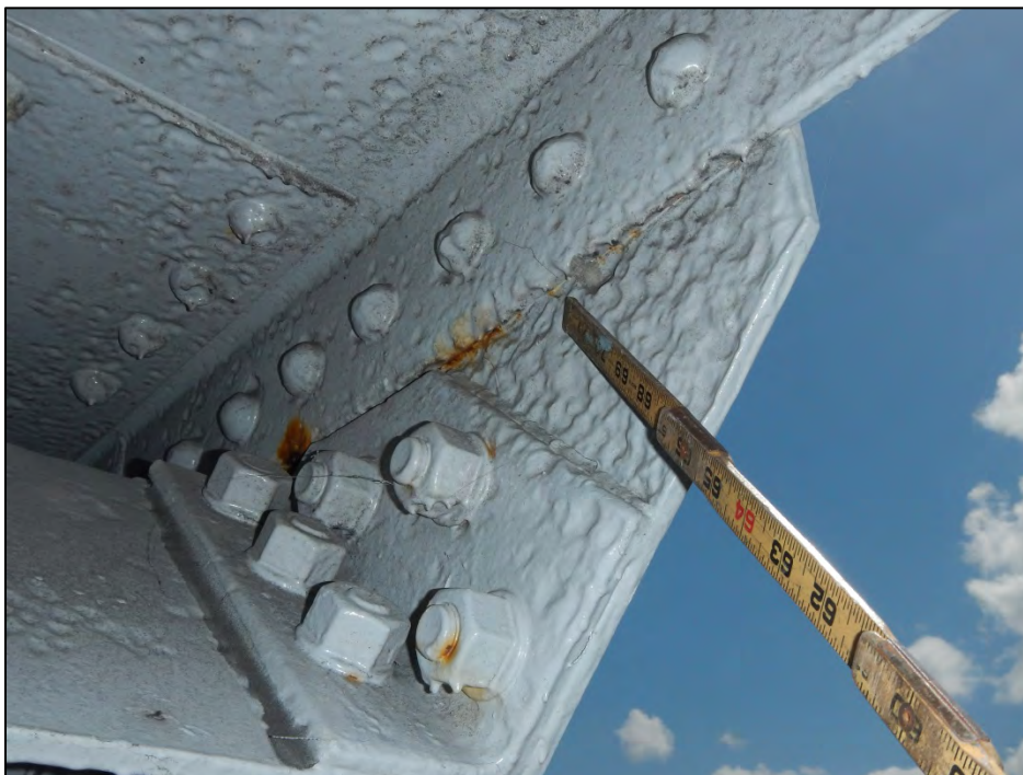
Photo 11 – Typical painted section loss on gusset plates.
