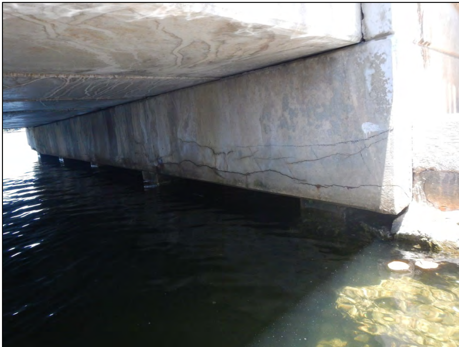
Photo 4 – Delamination in south end of east face of Abutment 1 cap.
