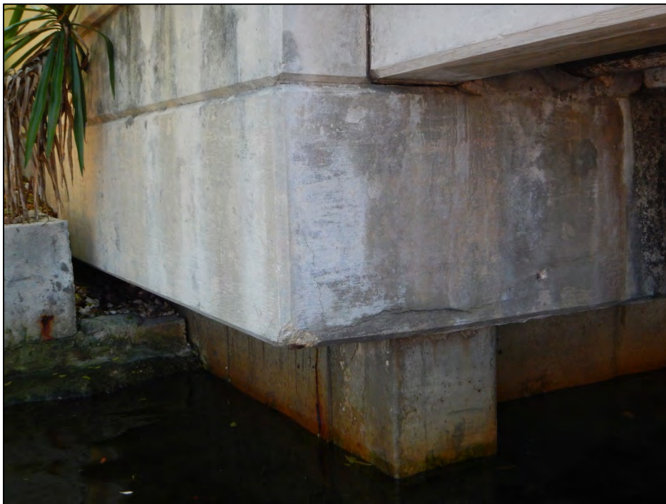
Photo 7 – Delamination/spall at east end of Abutment 1 cap.
