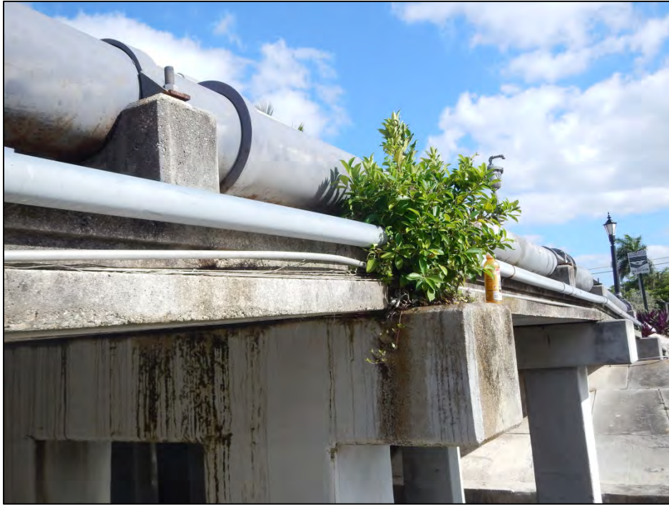
Photo 9 – There is minor vegetation growth between the caps and the Slab Units at the east end of Bent 2.
