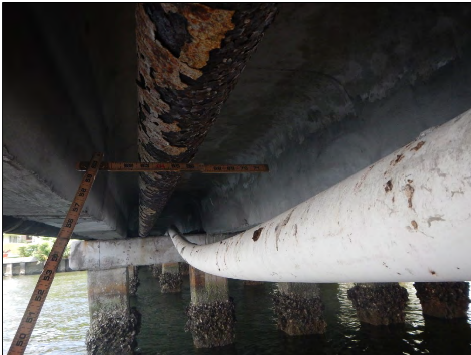
Photo 2 – Sagging utility line in Span 2.
