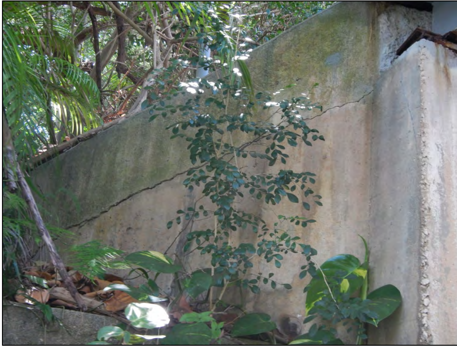
Photo 7 – Crack in NE wingwall.
