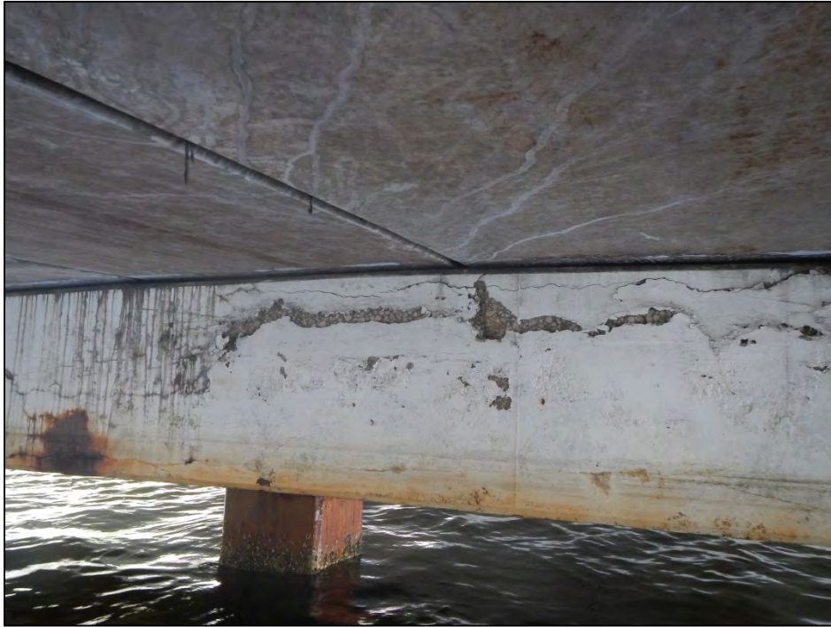
Photo 15 – Spalled/delaminated area in Bent 2 cap.
