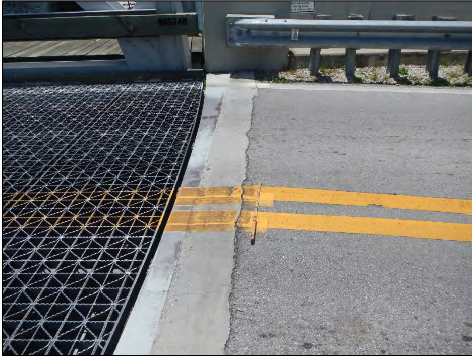
Photo 15 – Depressed north approach slab relative to abutment backwall.
