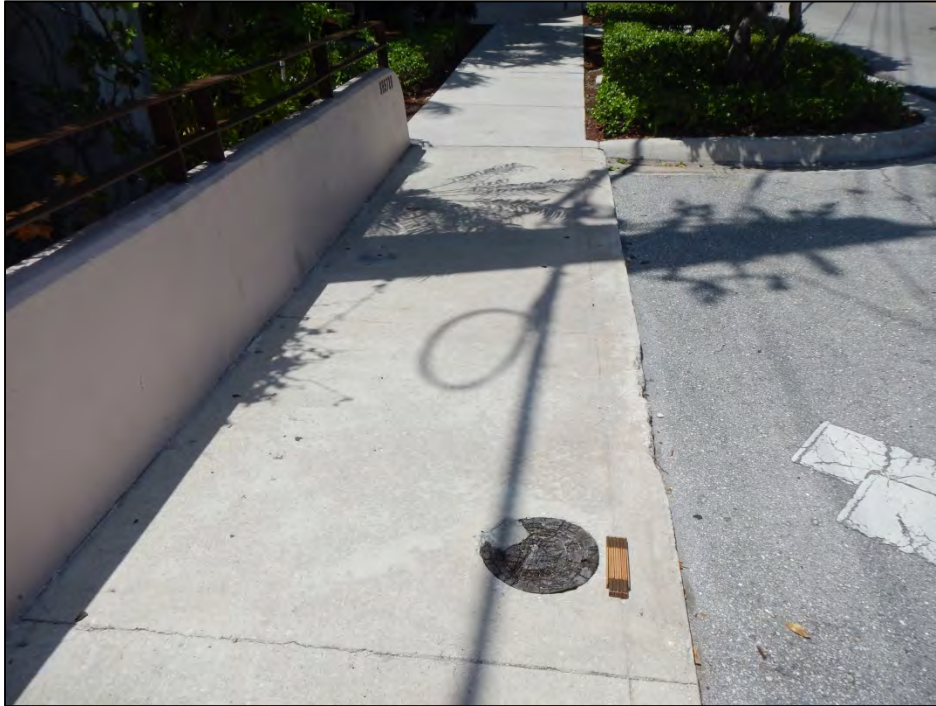
Photo 13 – The northwest approach sidewalk has a 1 ft. diameter timber column.
