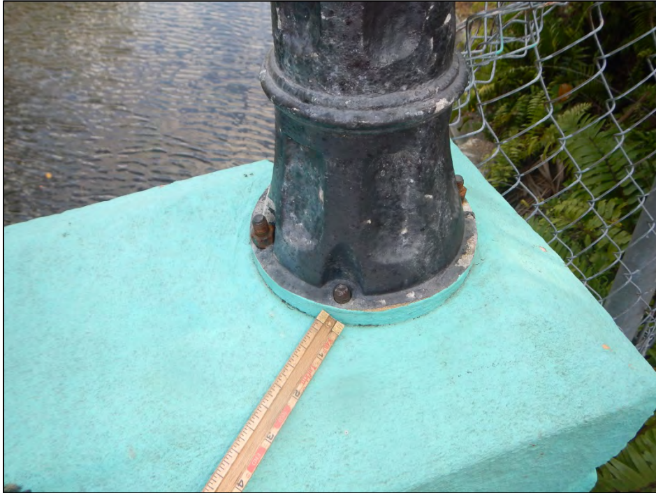
Photo 9 – The first light pole on the south barrier is missing 1 of 4 anchor bolt nuts.
