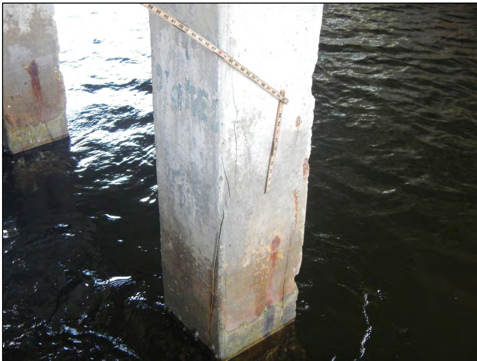
Photo 16 – The southeast and southwest corners of Pile 2-5 exhibit spalls/delaminations.
