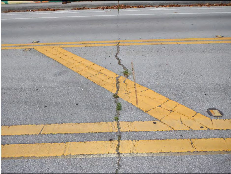
Photo 1 – Transverse crack in asphalt over joint at Abutment 2.
