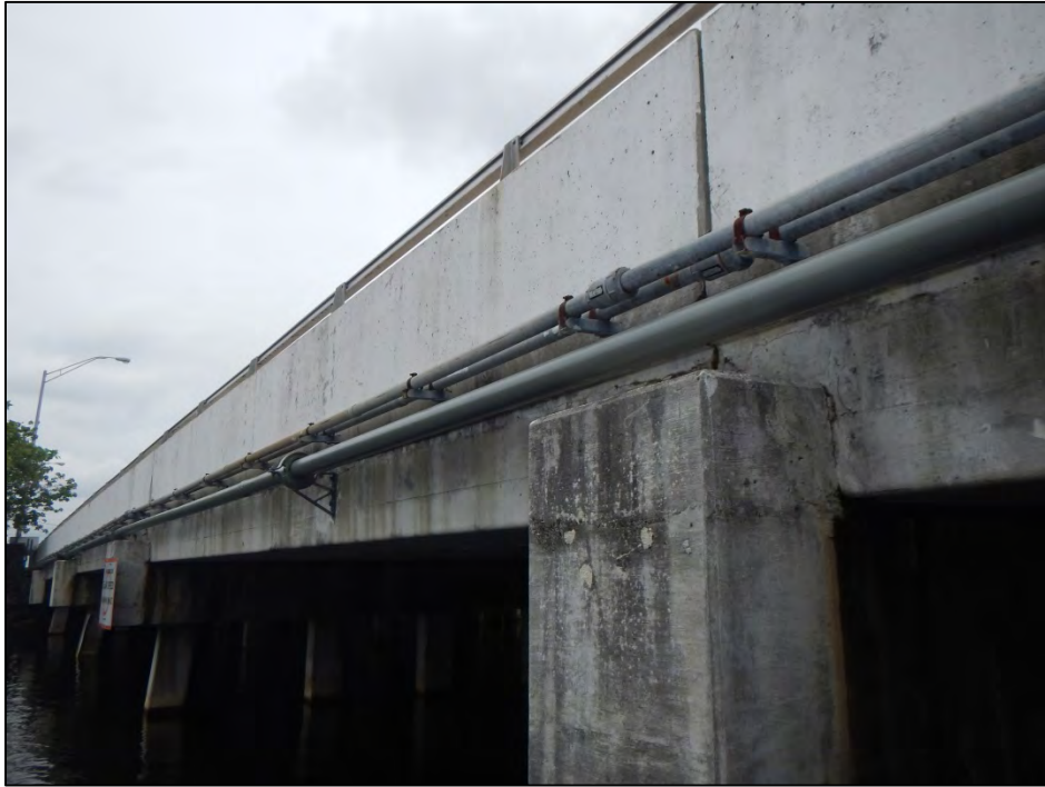
Utilities Mounted on West Side of Bridge
