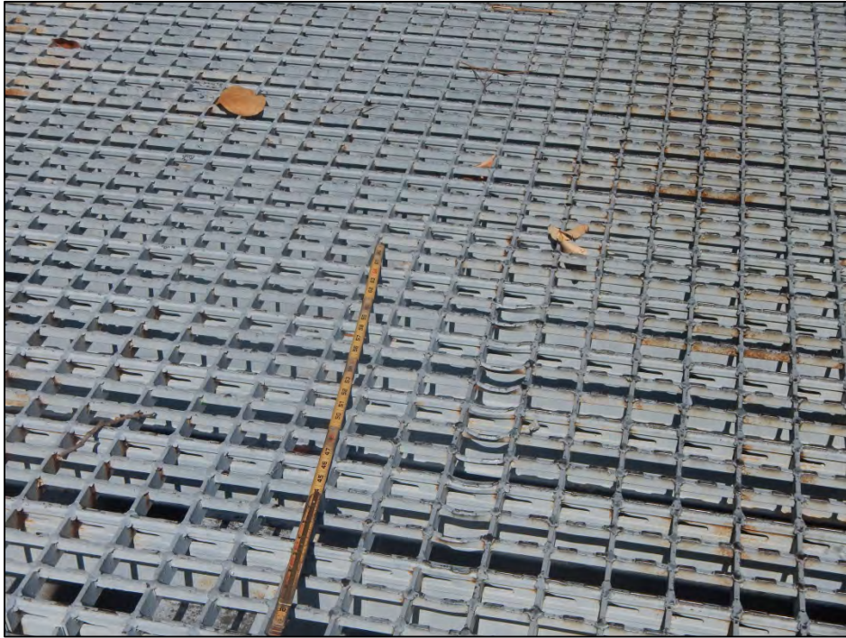
Photo 1 – Damaged and corroded open grid deck.
