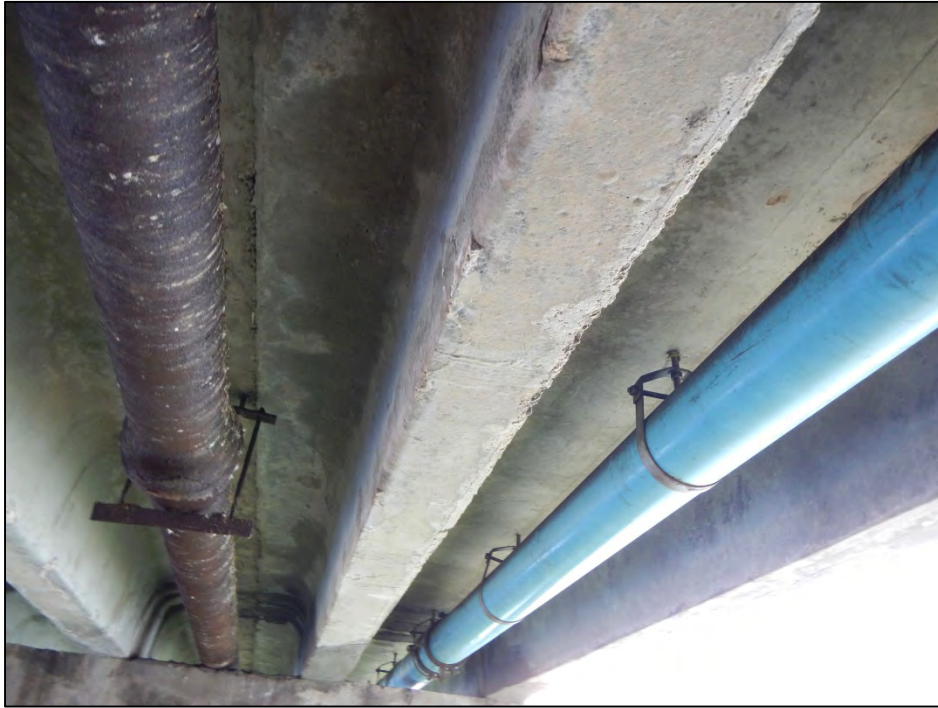
Concrete T-beam. Note Utility Pipe.
