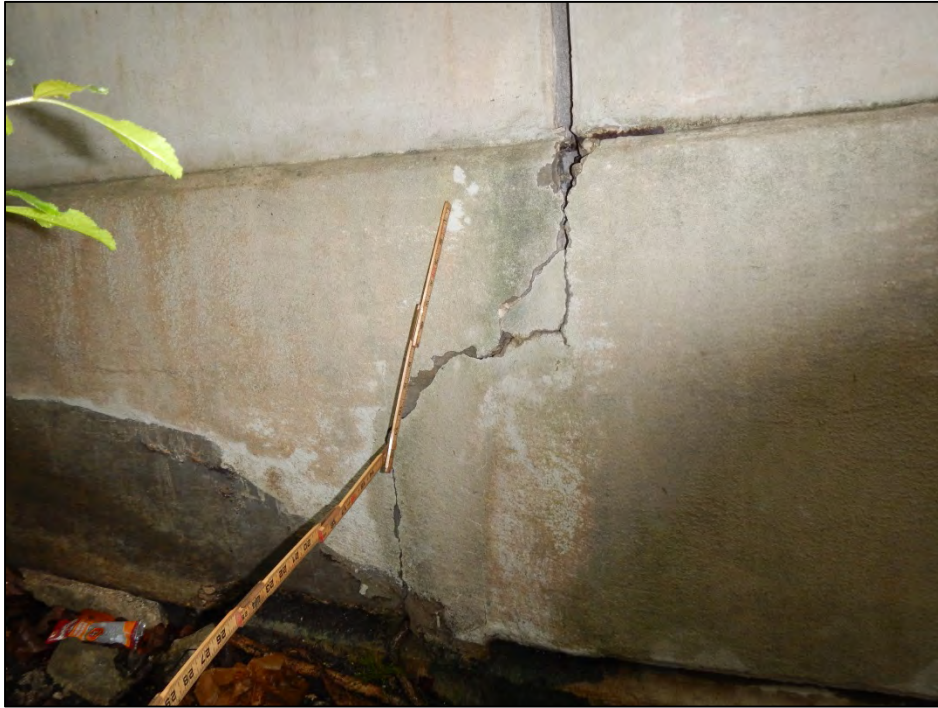
Photo 5 – Vertical crack in the south face of Slab Unit 6-1.
