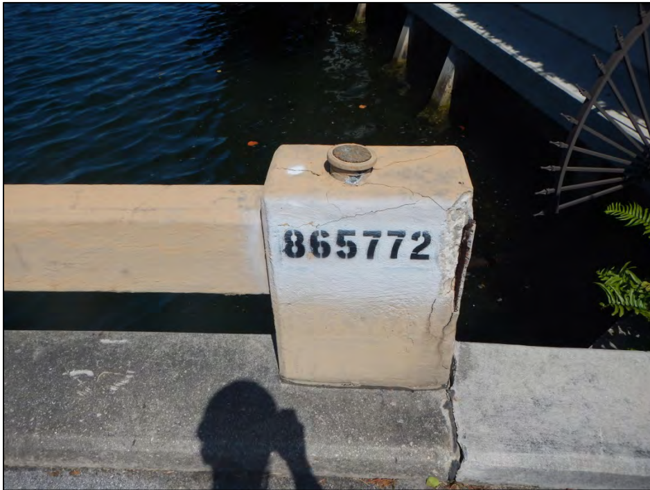
Photo 1 – Delamination and spall with exposed rebar in Post 1-1, Left.
