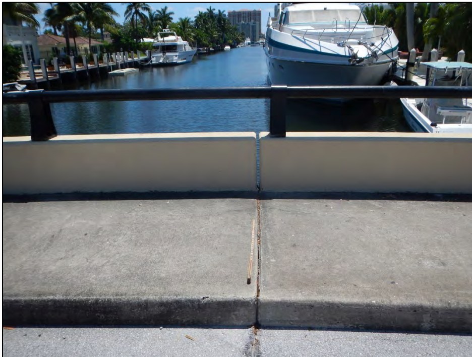
Photo 2 – Deteriorated sidewalk joint sealant filled with dirt and debris.
