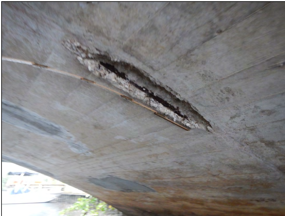
Photo 8 – Span 2 spall with exposed steel.
