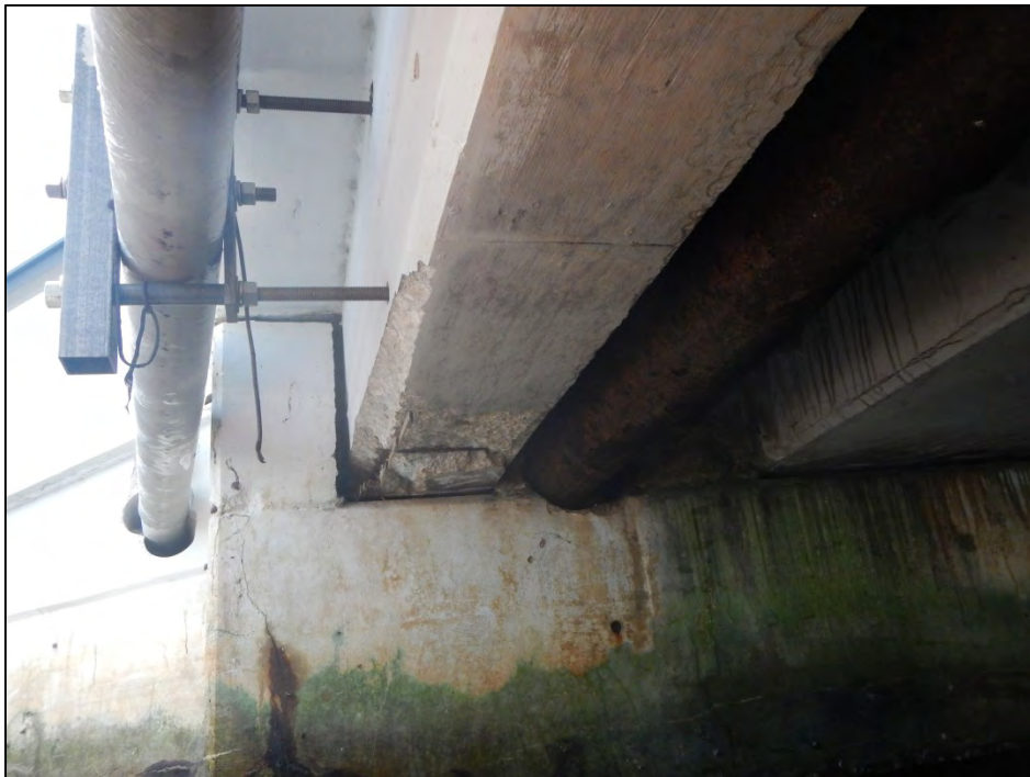
Photo 8 – Spall with exposed steel in the east fascia beam.
