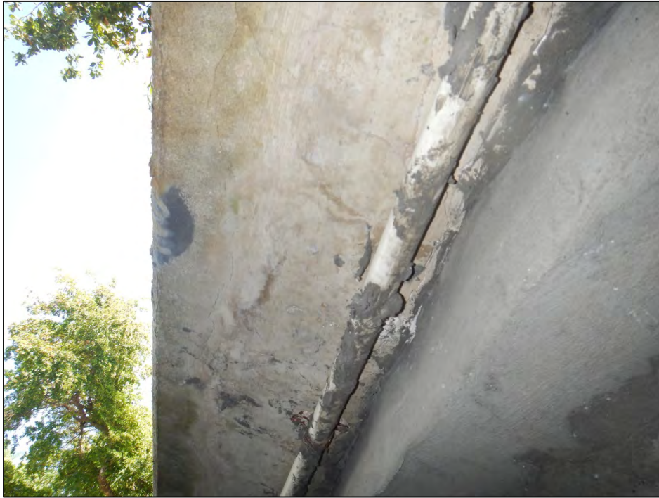
Photo 3 – Beam I-I exhibits longitudinal cracks.
