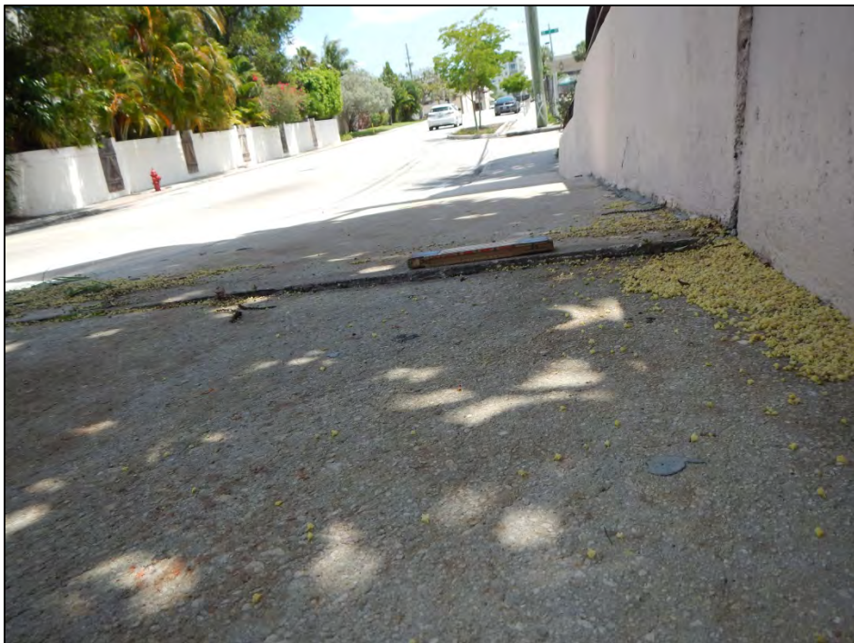
Photo 12 – The left sidewalk over Abutment 1 exhibits a difference in elevation.
