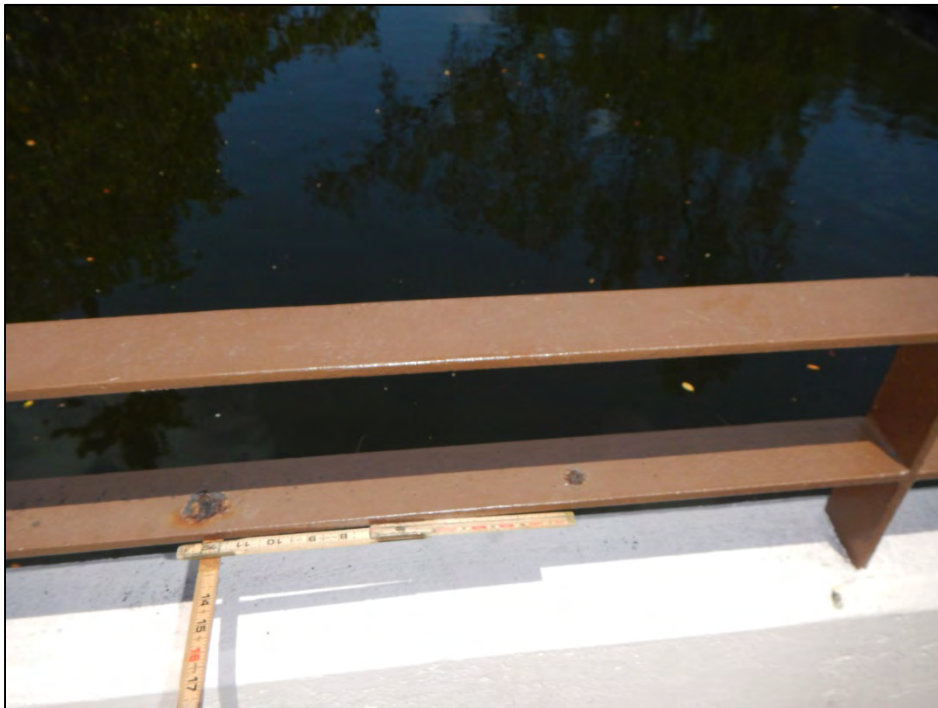
Photo 2 – The east railing at mid span over Span 2 exhibits corrosion.
