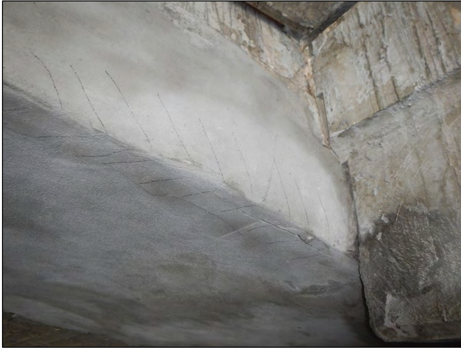
Photo 5 – The northwest end of the arch exhibits shrinkage cracks with hollow sounds.
