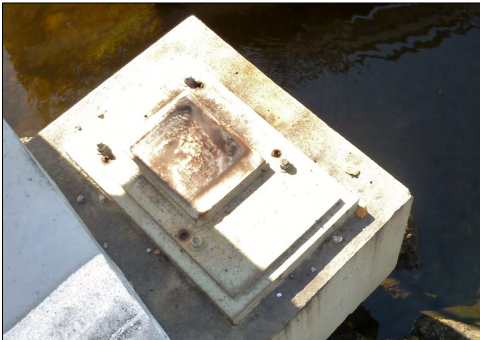
Photo 17 – Northwest Live Load Bearing: Note surface corrosion on Strike Plate.
