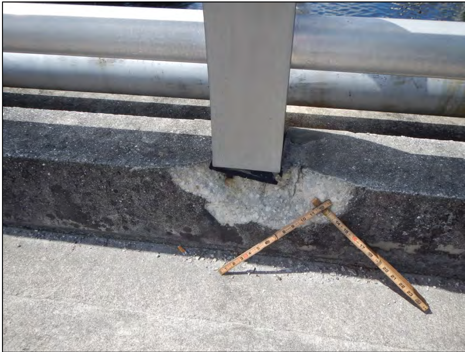
Photo 7 – Spall with exposed steel below Post 2-2 Right.
