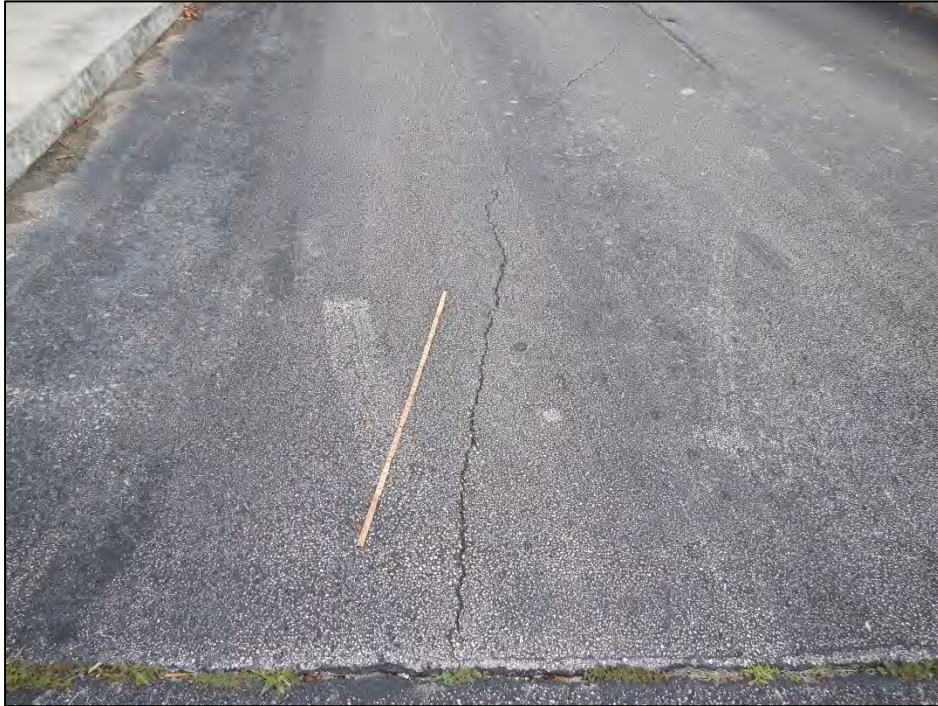
Photo 13 – East approach slab diagonal crack.
