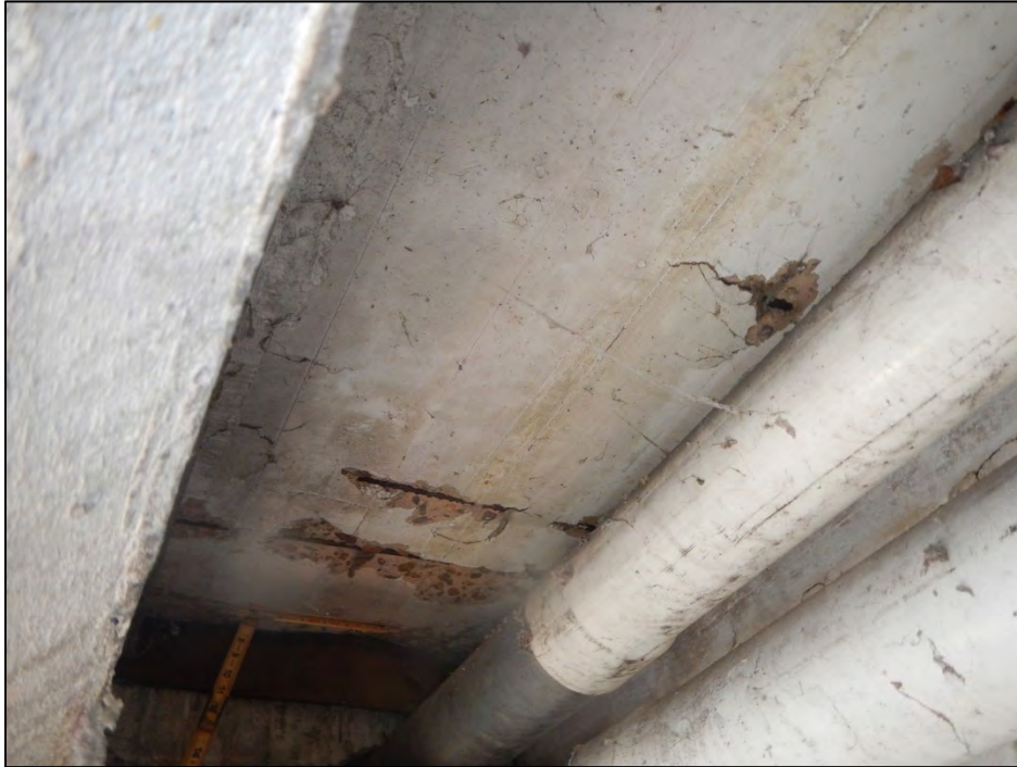
Photo 7 – Bay 8 over Abutment I exhibits a spall/delamination with exposed steel.
