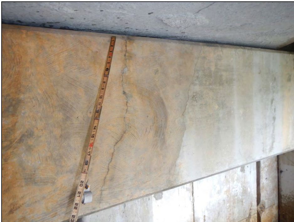
Photo 4 – Abutment I cap exhibits a vertical crack.
