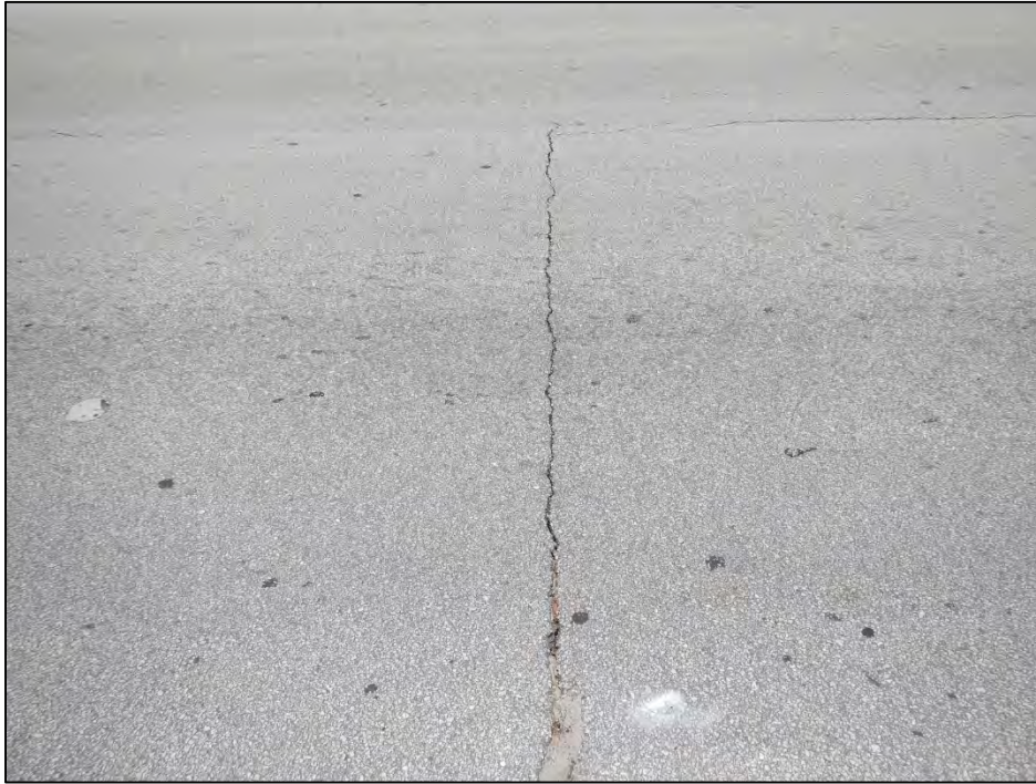
Photo 3 – The eastbound deck top joint exhibits a transverse crack over Bent 2.
