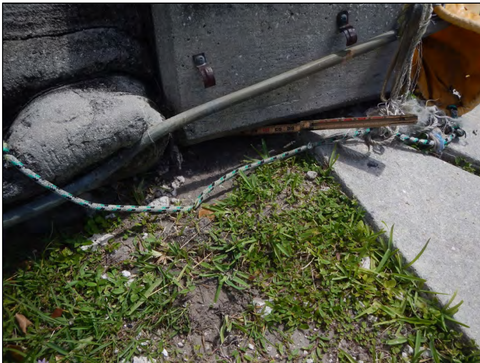
Photo 12 – The south end of End Bent 1 cap is undermining.
