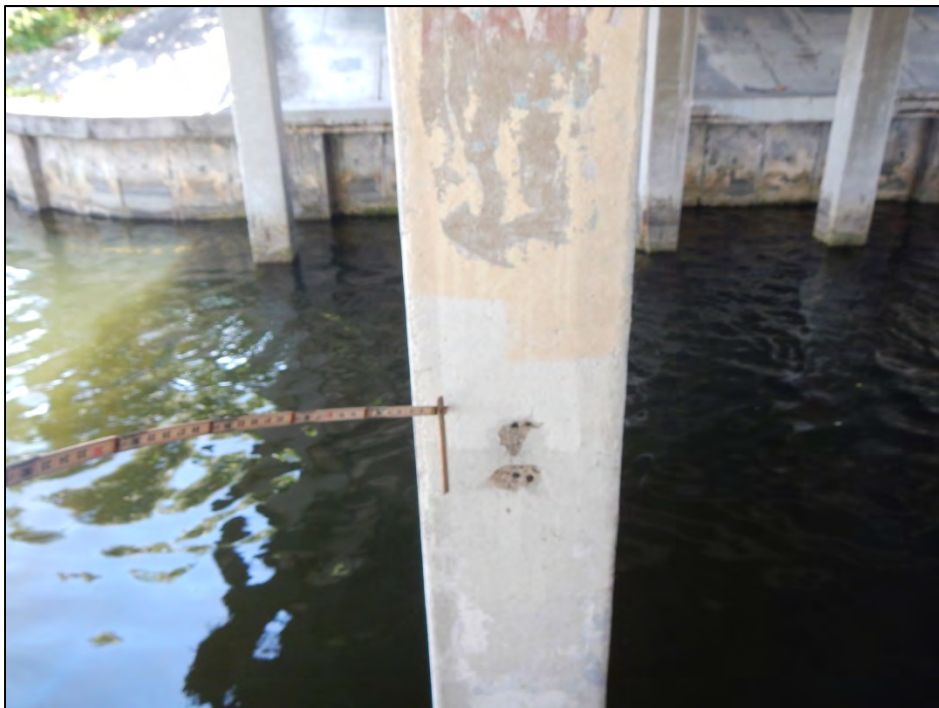
Photo 14 – The west face of Pile 2-2 exhibits a popout.
