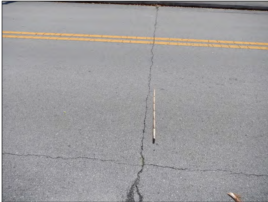
Photo 3 – Typical transverse crack in asphalt overlay at intermediate bent.
