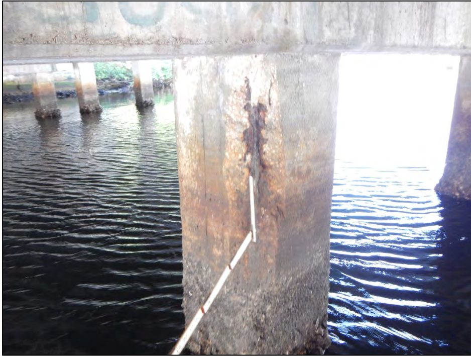
Photo 11 – Spall/delamination with exposed steel at the southwest corner of Pile 3-6.
