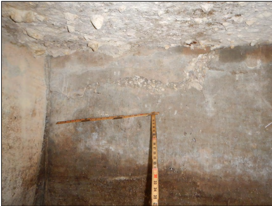
Photo 6 – End Bent I backwall spall and delamination
