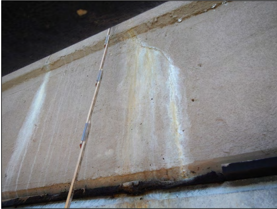
Photo 1 – Vertical cracks in the east fascia over Bent 3.
