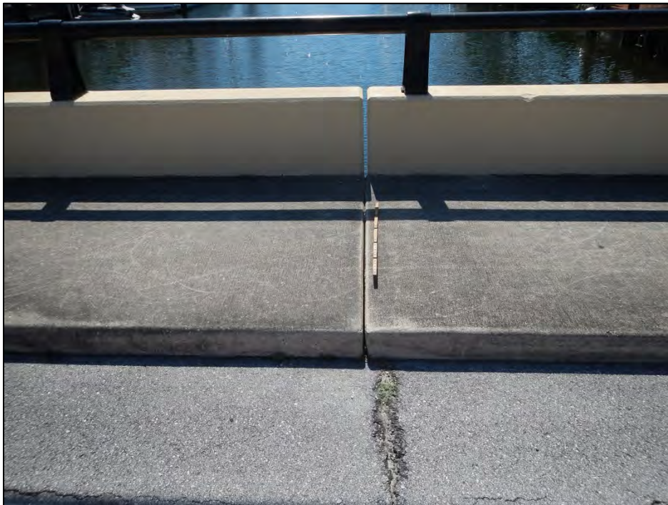
Photo 2 – Deteriorated sidewalk joint sealant.
