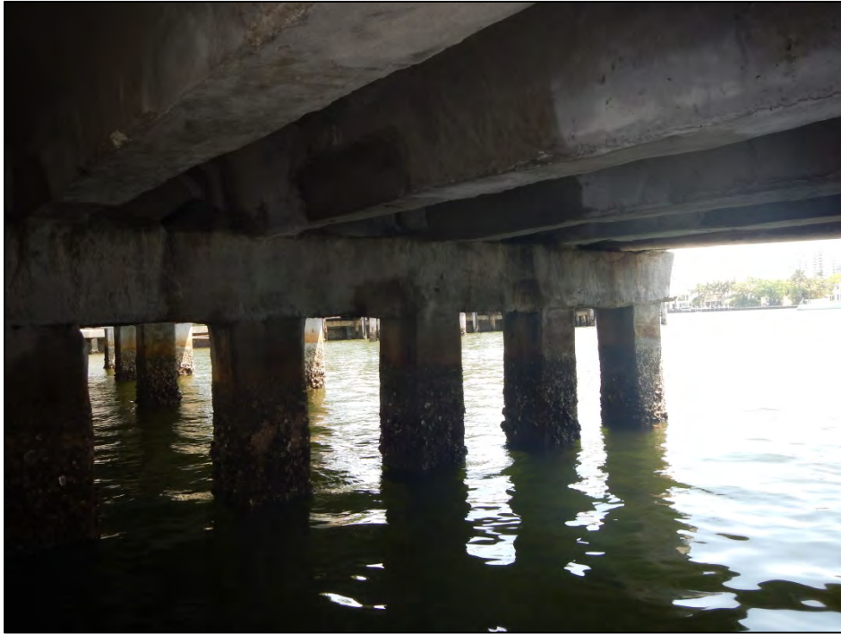
Photo 7 – Typical spalling (UW may take out).
