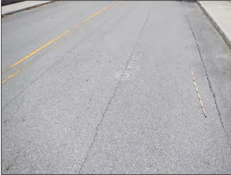
Photo 1 – Longitudinal cracks in the asphalt overlay.
