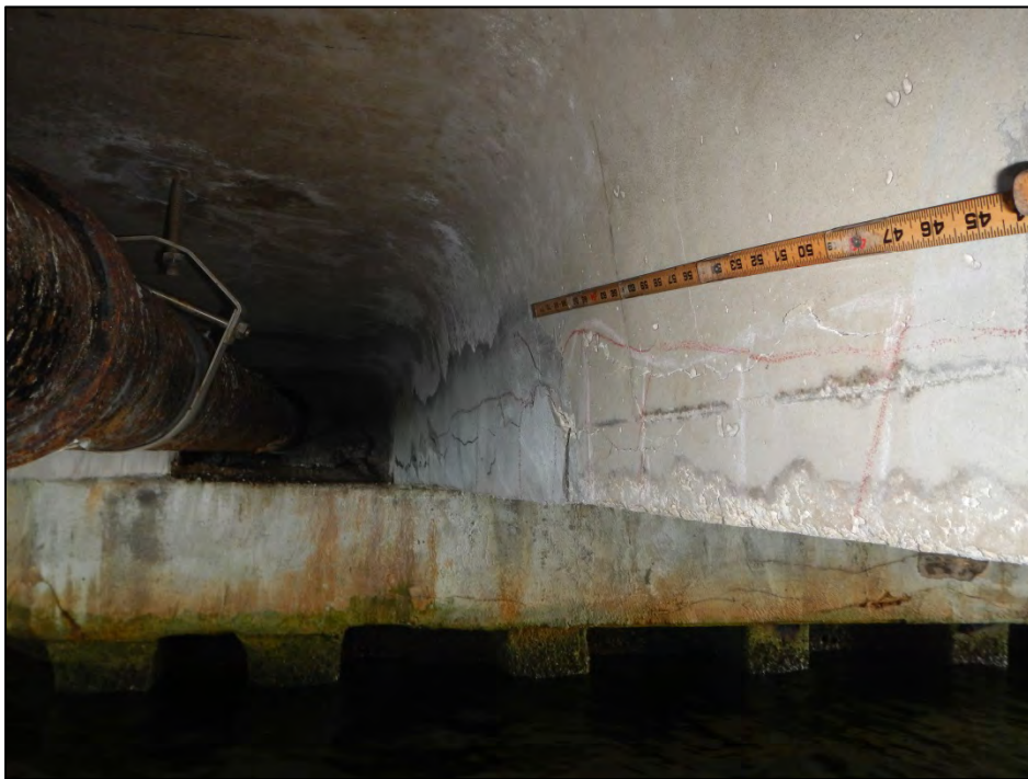
Photo 4 – Delaminated patch on Beam I-4.
