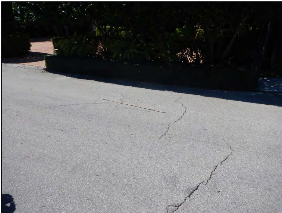
Photo 14 – Cracks in asphalt surfacing over west approach slab.
