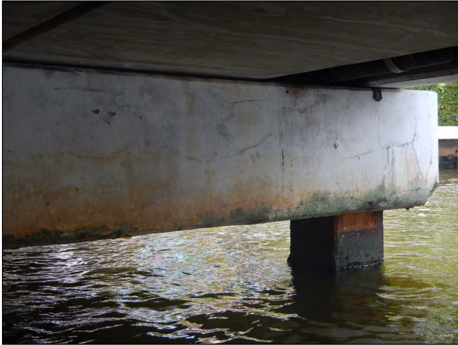
Photo 13 – Spall with corrosion bleedout at the southeast corner of Bent 3 cap.
