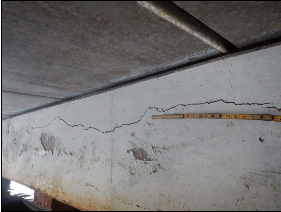
Photo 13 – Delamination in Bent 2 cap.
