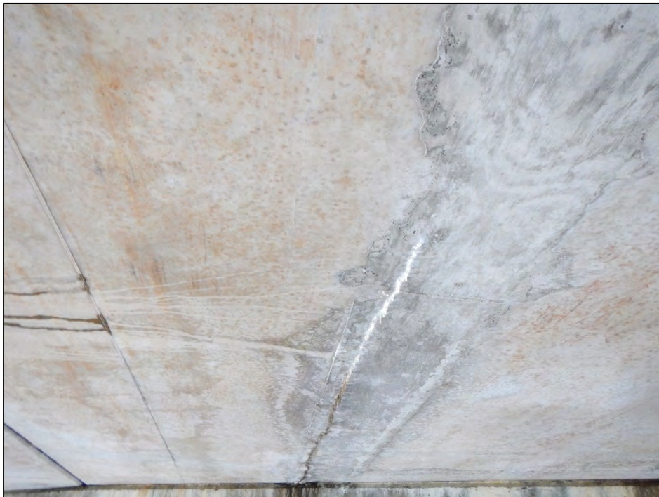
Photo 8 – Slab 3-2 to 3-3 longitudinal crack.
