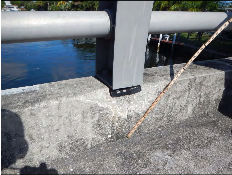
Photo 5 – The concrete parapet below Post I-2 exhibits a spall with exposed steel.
