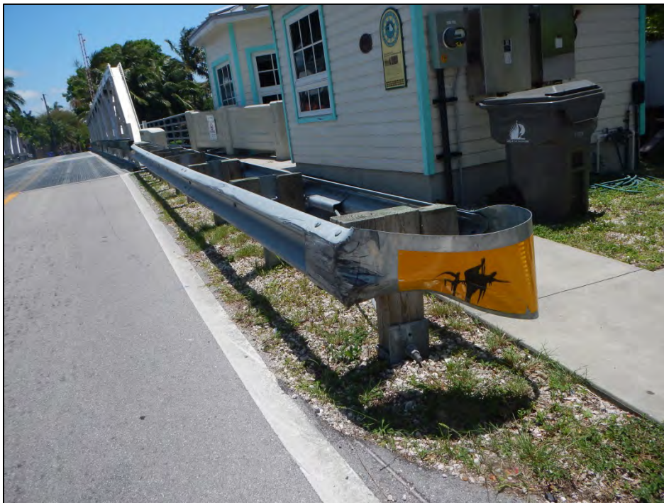
Photo 16 – Impact damage at northwest guardrail end terminal.
