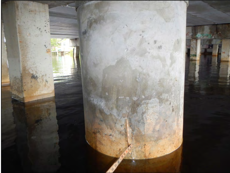
Photo 11 – The southwest quadrant of Pile 3-10 exhibits a delamination.
