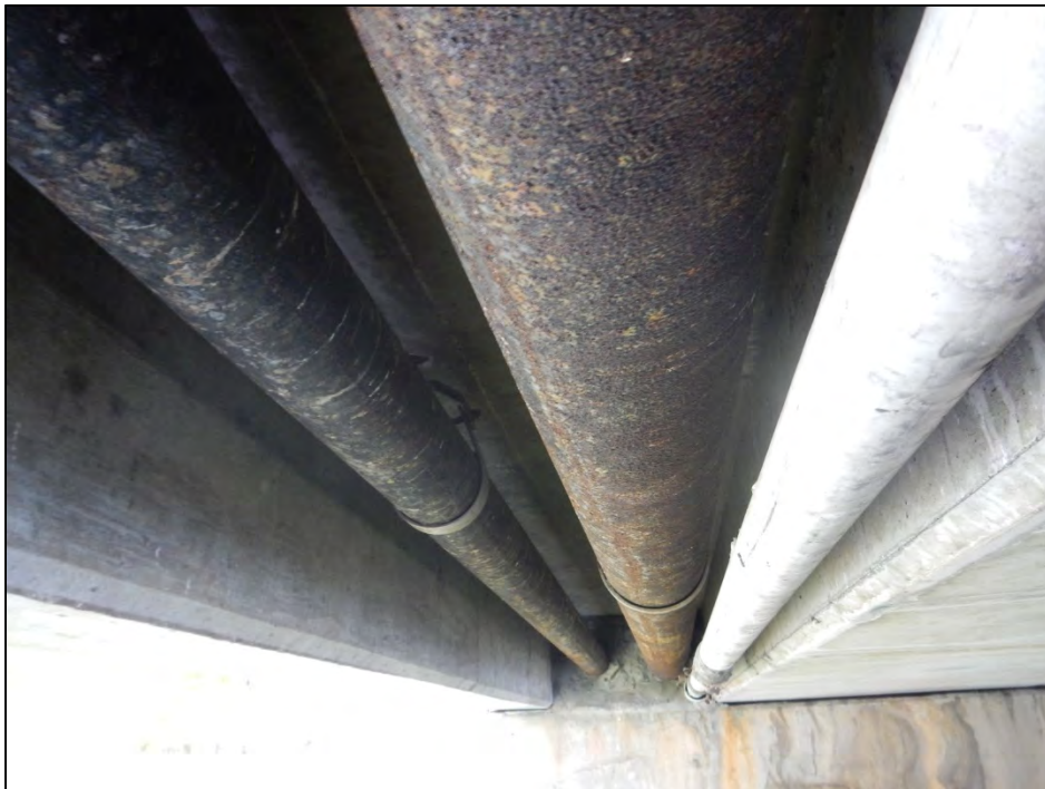
Utilities Mounted Adjacent to Slab Unit
