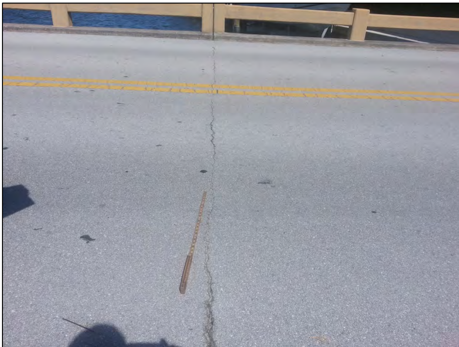
Photo 2 – Typical cracking in the asphalt over intermediate bents.
