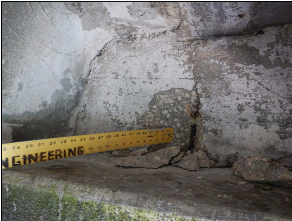
Photo 6 – Spall with exposed reinforcing steel in the backwall at Abutment I.
