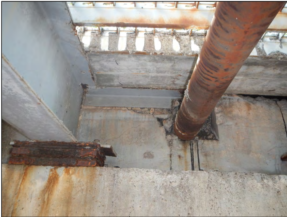
Photo 4 – Typical corrosion on end bent bearings.
