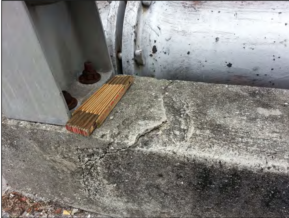
Photo 11 – East railing has a delamination at the north end.
