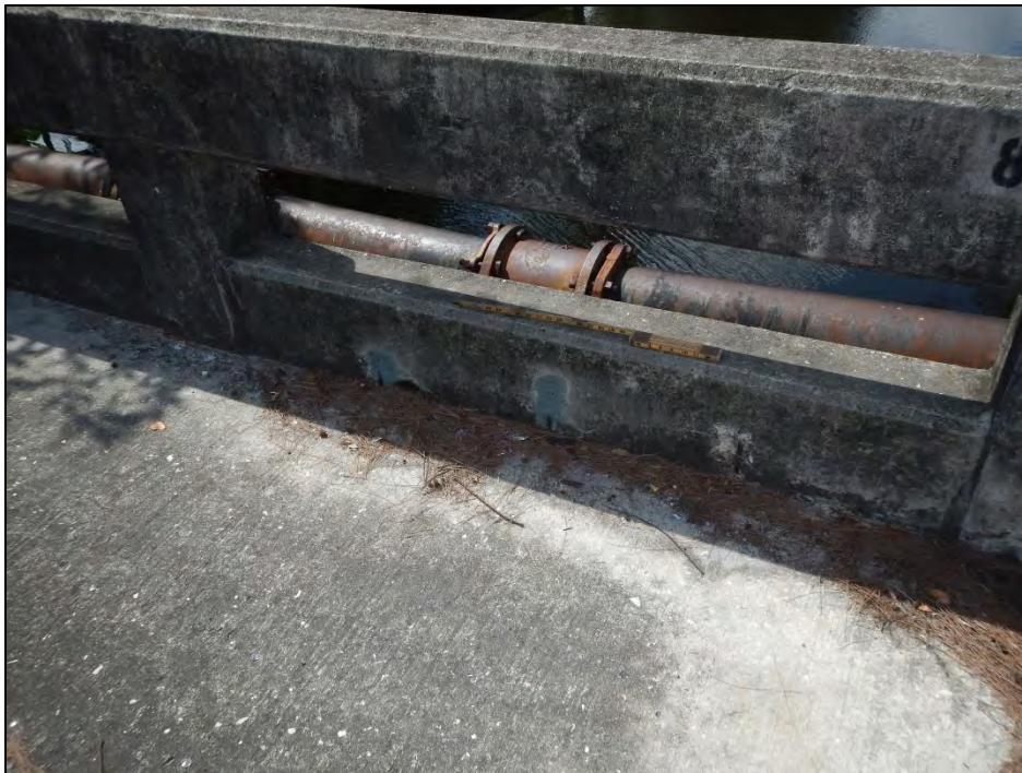
Photo 2 – The north side of the south railing exhibits spalls with exposed steel.
