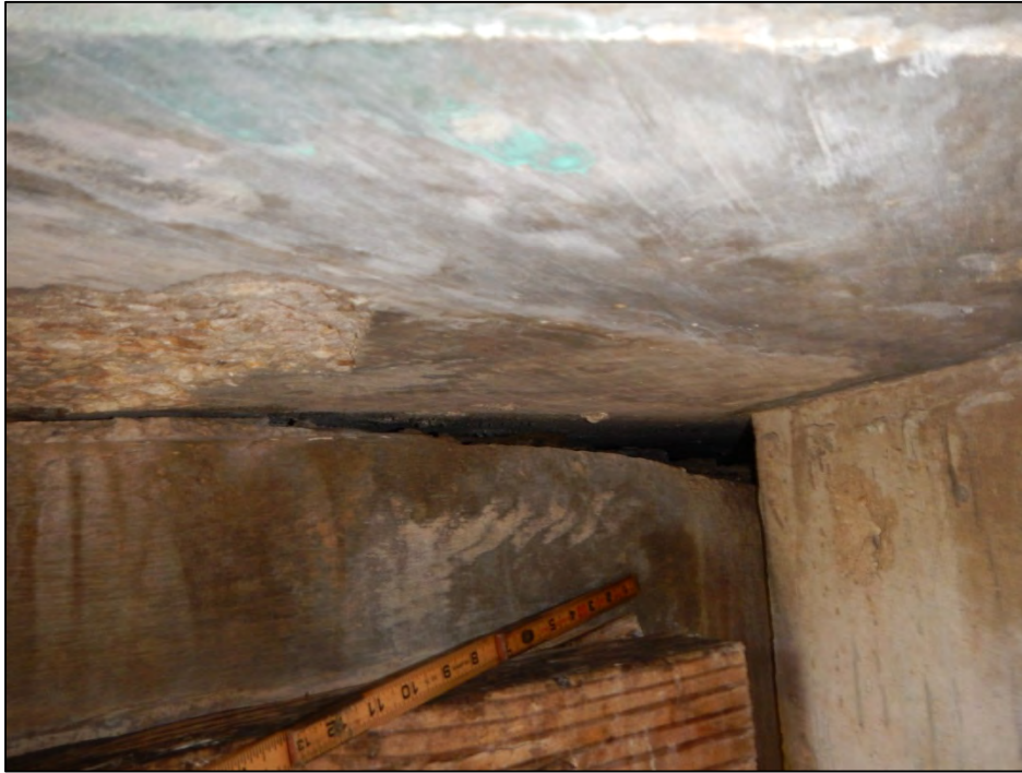
Photo 11 – The End Bent 1 retaining wall exhibits a void behind Pile 1-7.
