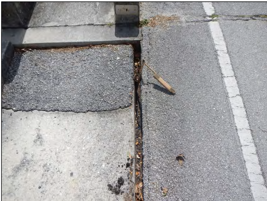
Photo 22 – Northwest approach slab between the sidewalk is not sealed.
