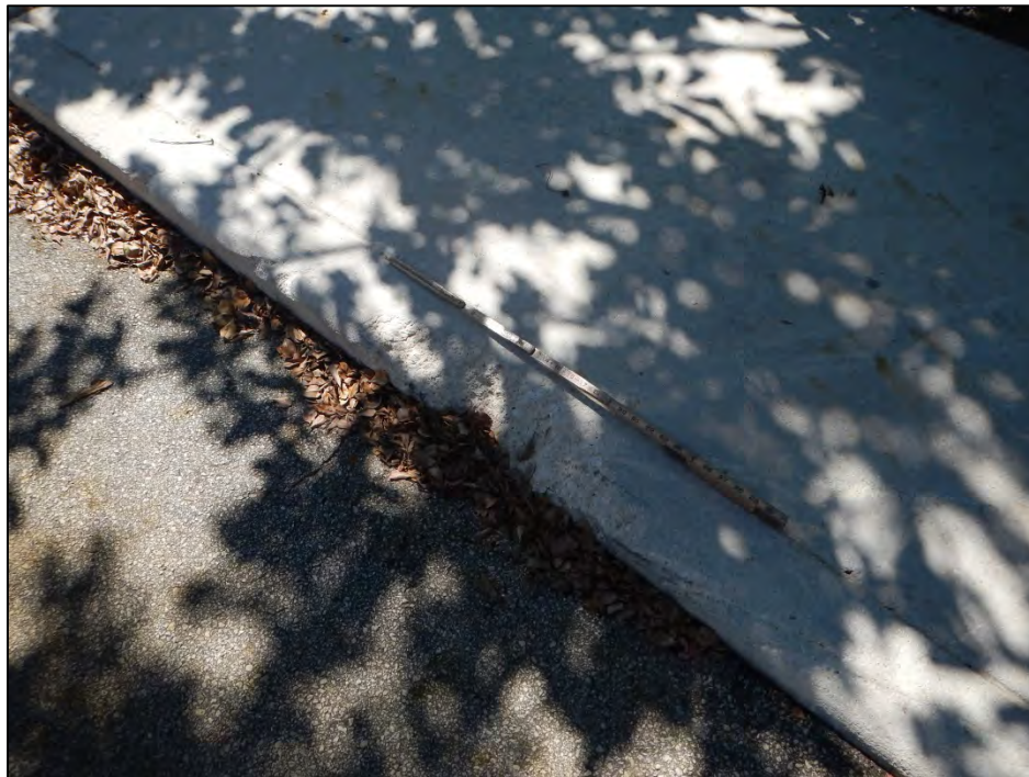
Photo 16 – Spall in northeast approach curb.
