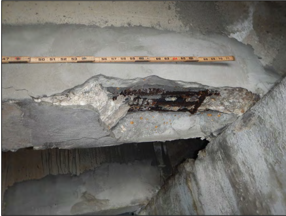
Photo 3 – Spall in the Double T-beam I-2 Right Leg.
