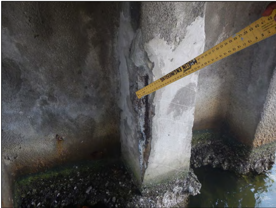
Photo 8 – Spall with exposed reinforcing steel in Pile I-2 at Abutment I.
