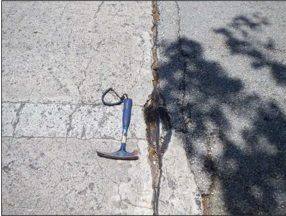
Photo 3 – The center lane over End Bent I exhibits a spall.
