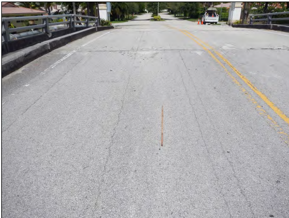
Photo 2 – Deck top longitudinal cracks.
