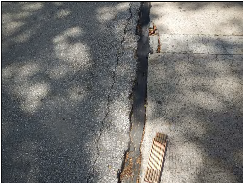
Photo 2 – The End Bent I joint seal is deteriorated.
