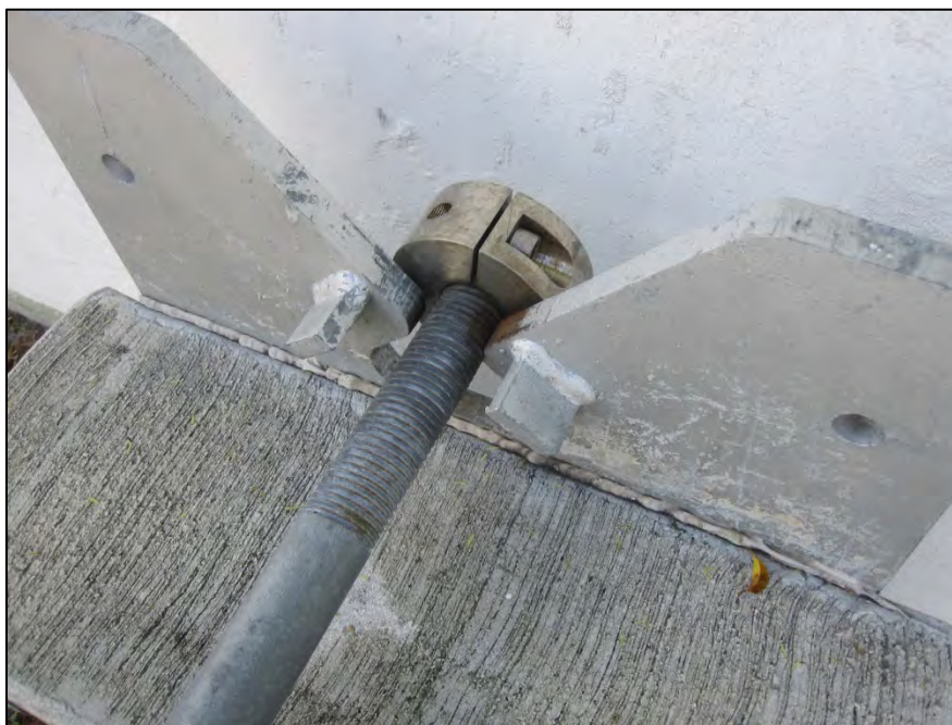
Photo 28 – Barrier gates typically do not fully engage their receivers.
