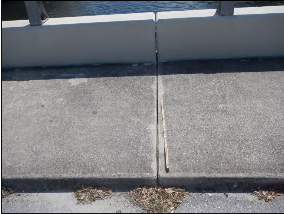
Photo 5 – Deteriorated sidewalk joint.
