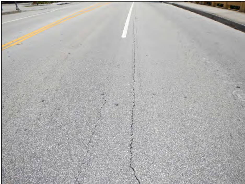
Photo 2 – The deck top exhibits longitudinal cracks.
