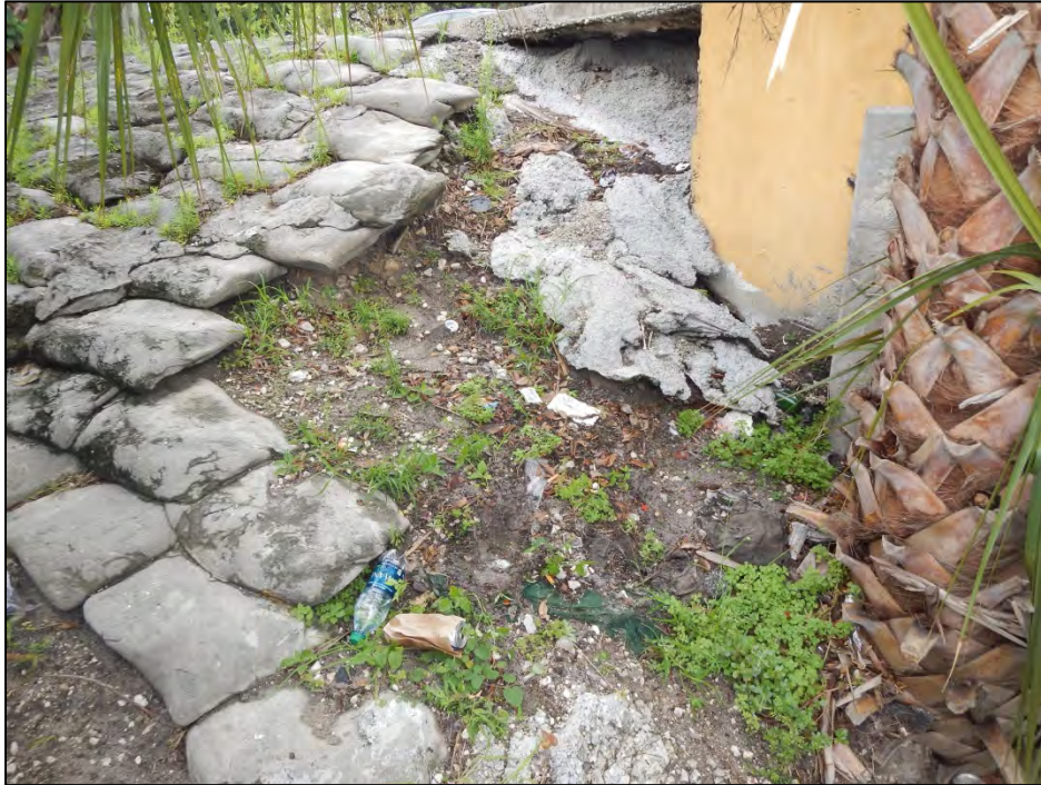
Photo 9 – Southeast abutment corner exhibits missing riprap and an erosion.
