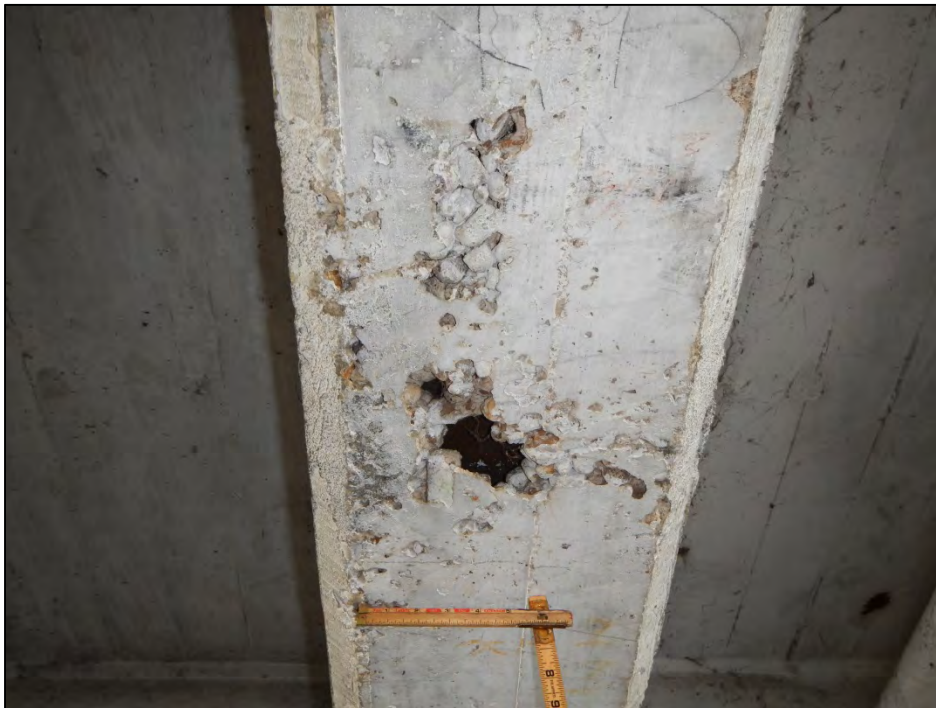
Photo 14 – Beam I-7 mid span exhibits a void.
