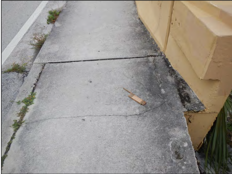
Photo 17 – Southeast approach sidewalk exhibits multi-directional cracks.
