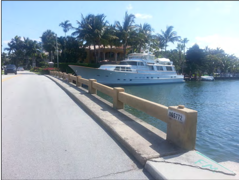
Typical Bridge Railing
