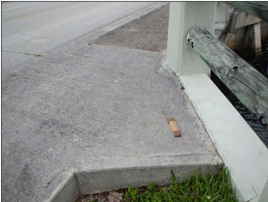
Photo 8 – The northeast approach sidewalk exhibits a spall.
