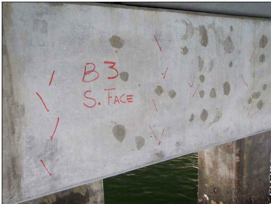
Photo 2 – Cracks in the south face of the Bent 3 cap.
