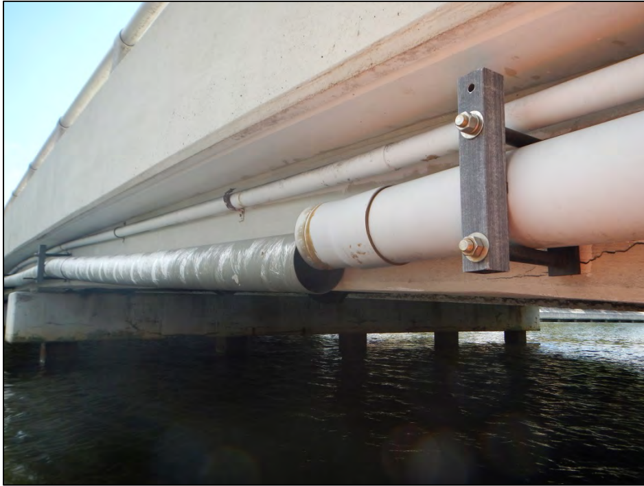
Photo 5 – Disconnected utility pipe attached to Beam 2 in Span 3.
