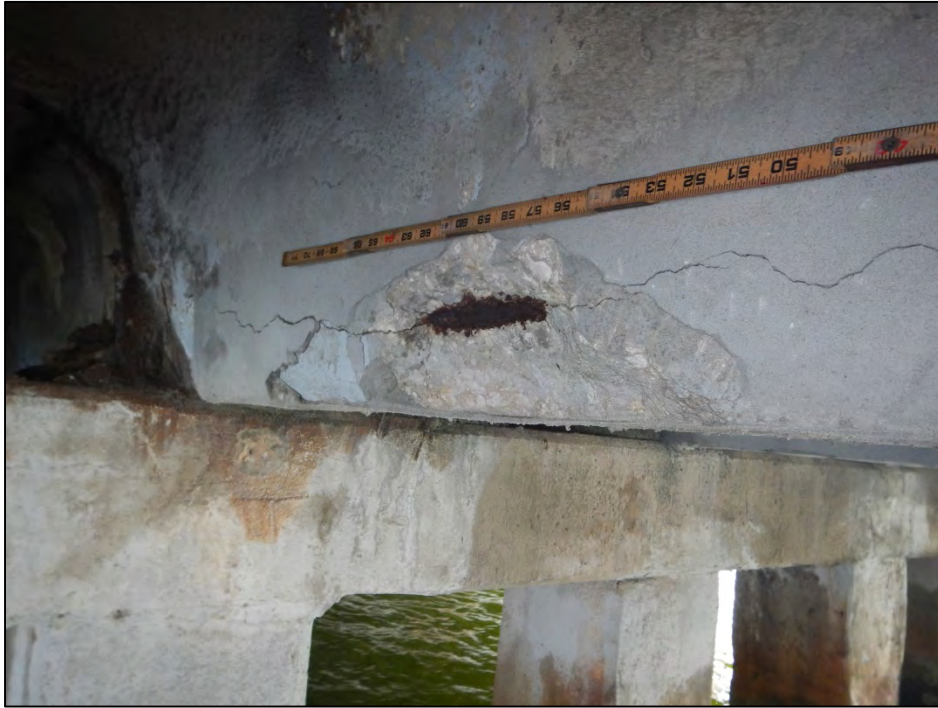
Photo 5 – Spall and delamination on Beam 2-3 right leg.
