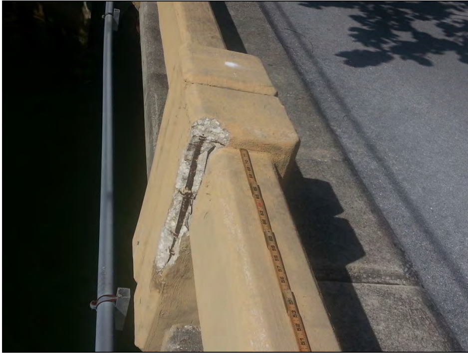
Photo 1 – Spall in Post 4-3, left.
