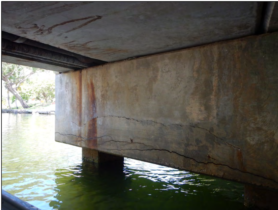
Photo 4 – Delamination in Bent 2 cap.
