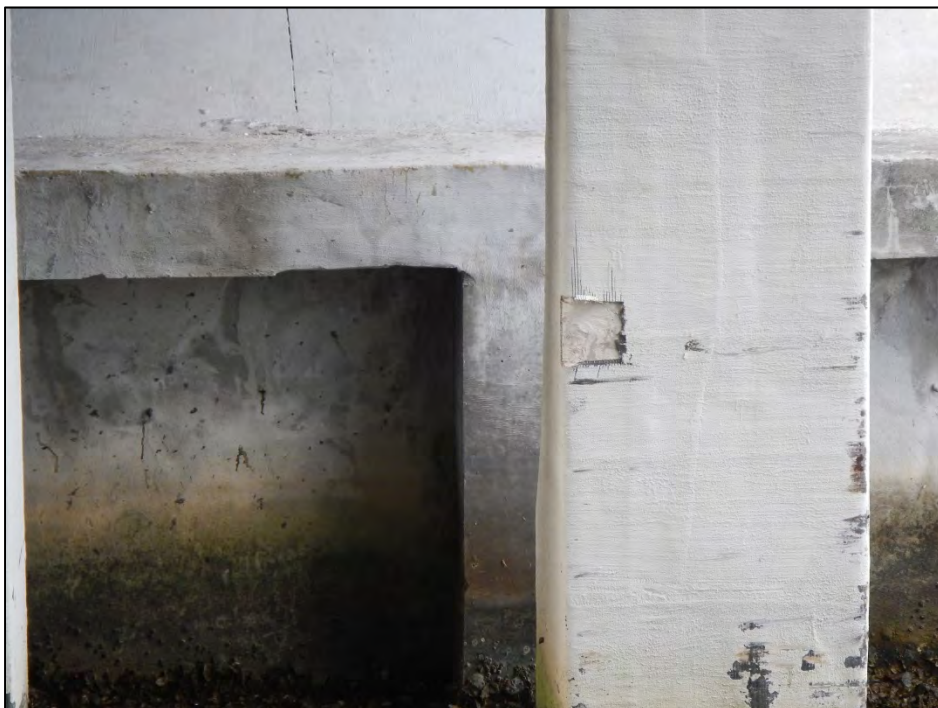
Photo 10 – The northeast corner of Pile Jacket I-I exhibits a spall.
