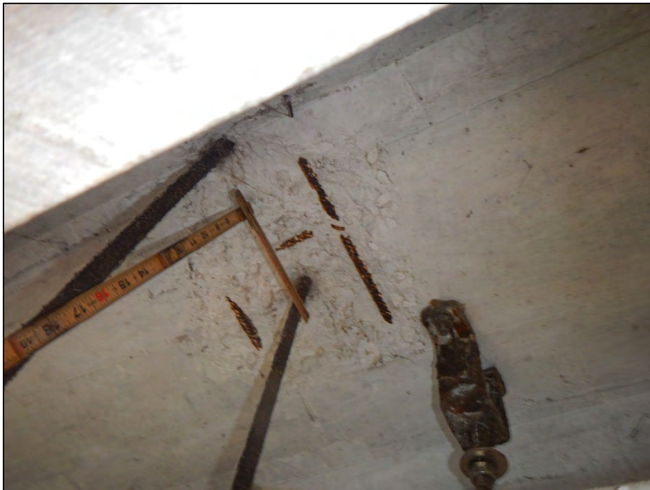
Photo 4 – Bay I mid span exhibits a spall with exposed steel.
