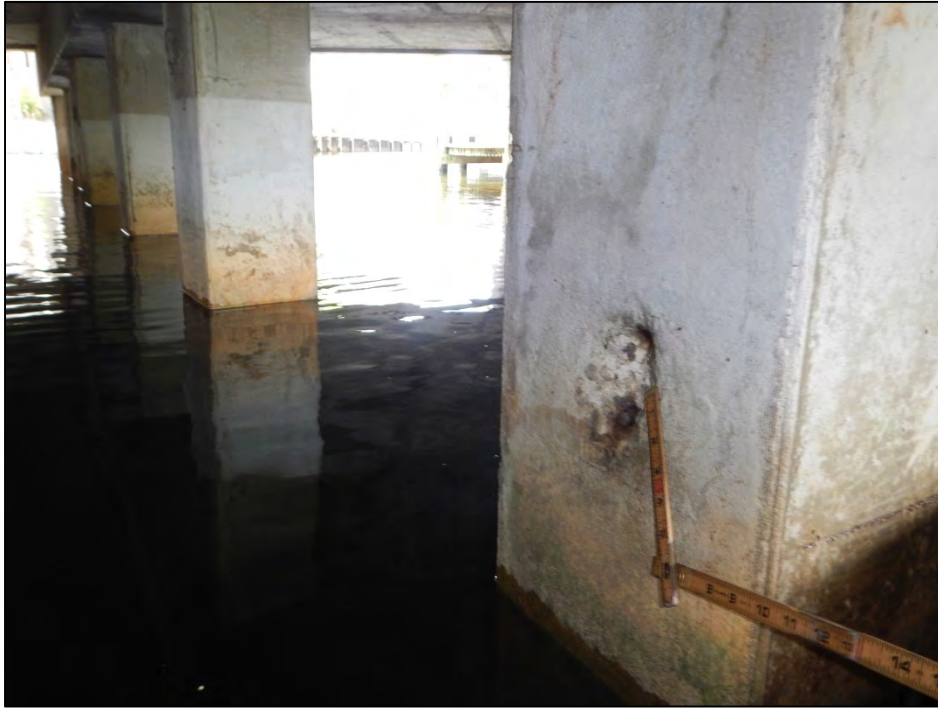
Photo 5 – The east face of Pile 3-2 exhibits an unpatched pickup point.
