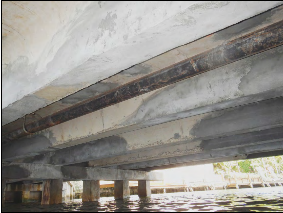
Utilities Mounted under Span I.
