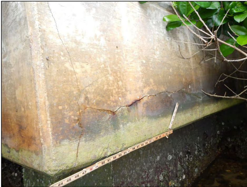
Photo 10 – Delamination in the northwest retaining wall cap.
