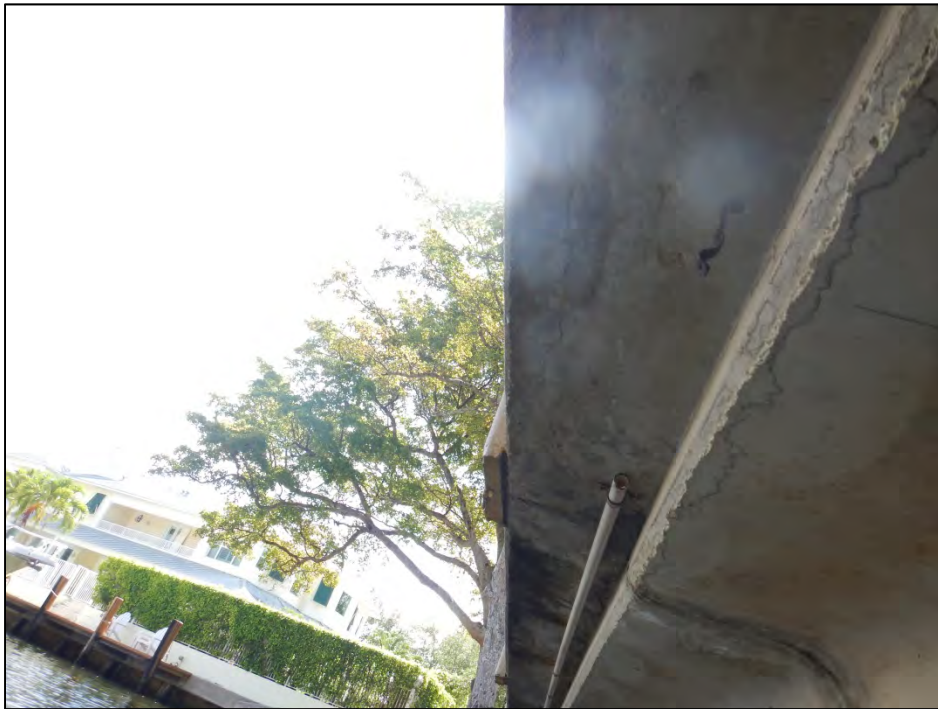
Photo 4 – The right overhang exhibits cracking with delaminations.
