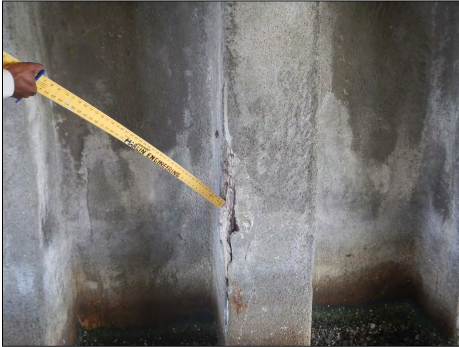
Photo 9 – Spall with exposed reinforcing steel and crack in Pile I-5 at Abutment I.
