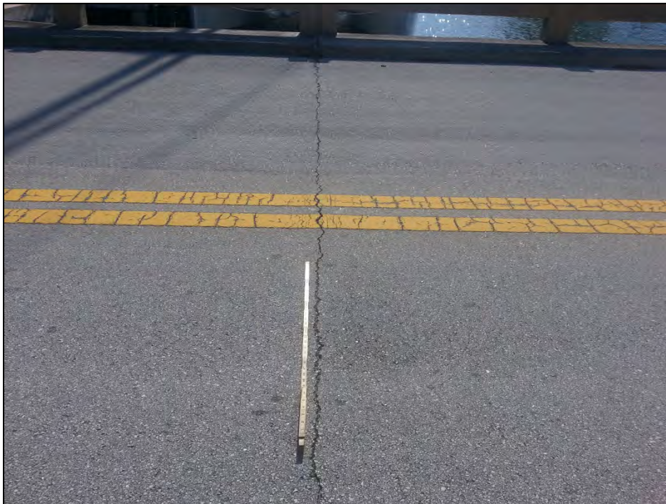
Photo 2 – Cracks in the asphalt over the expansion joints.
