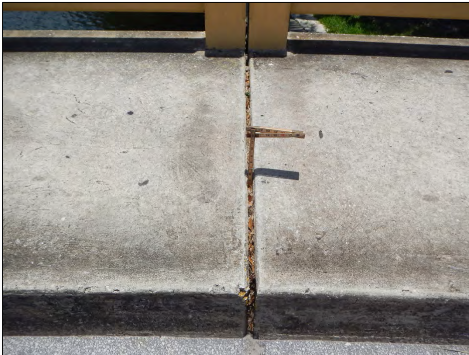
Photo 4 – The right sidewalk joints exhibit deteriorated sealants.
