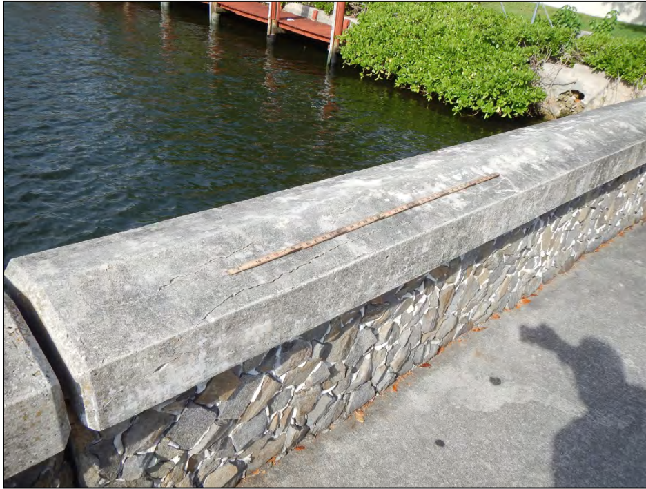
Photo 1 – Delamination in the top face of the railing in Span I.
