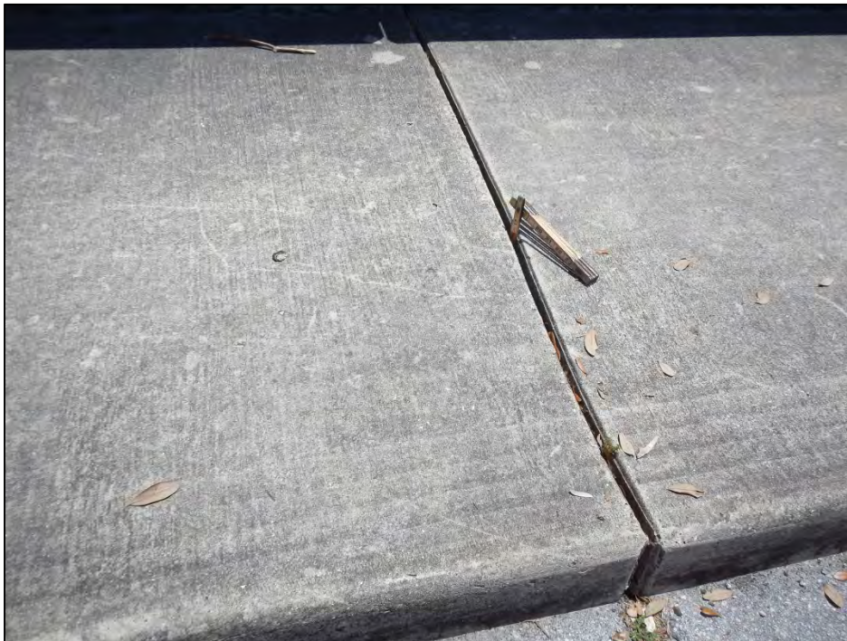
Photo 2 – Deteriorated sidewalk joint sealant.
