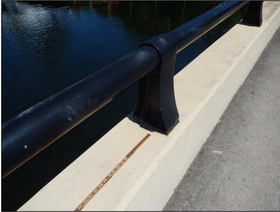
Photo 3 – Missing anchor bolt nuts at left handrail Post 1-3.
