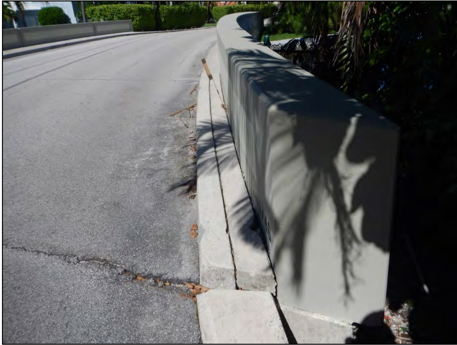
Photo 11 – Gap between wingwall and approach curb.
