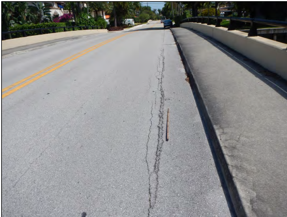
Photo 2 – Longitudinal cracks in asphalt overlay adjacent to right sidewalk.
