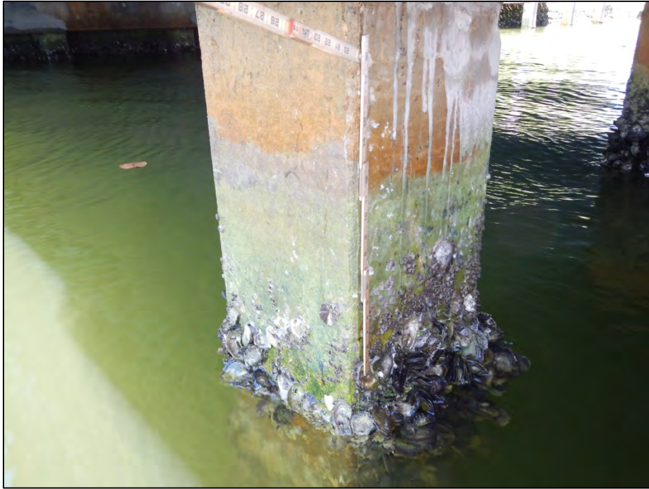
Photo 3 – Vertical cracks on Pile 2-6.
