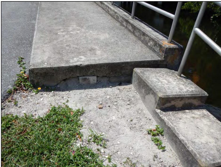
Photo 14 – The northeast sidewalk exhibits a drop-off.
