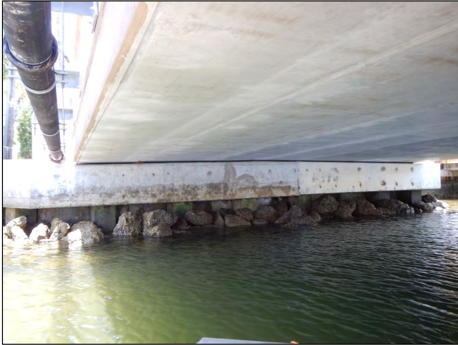
Slab Underside and Abutment. Note Utility Pipe.
