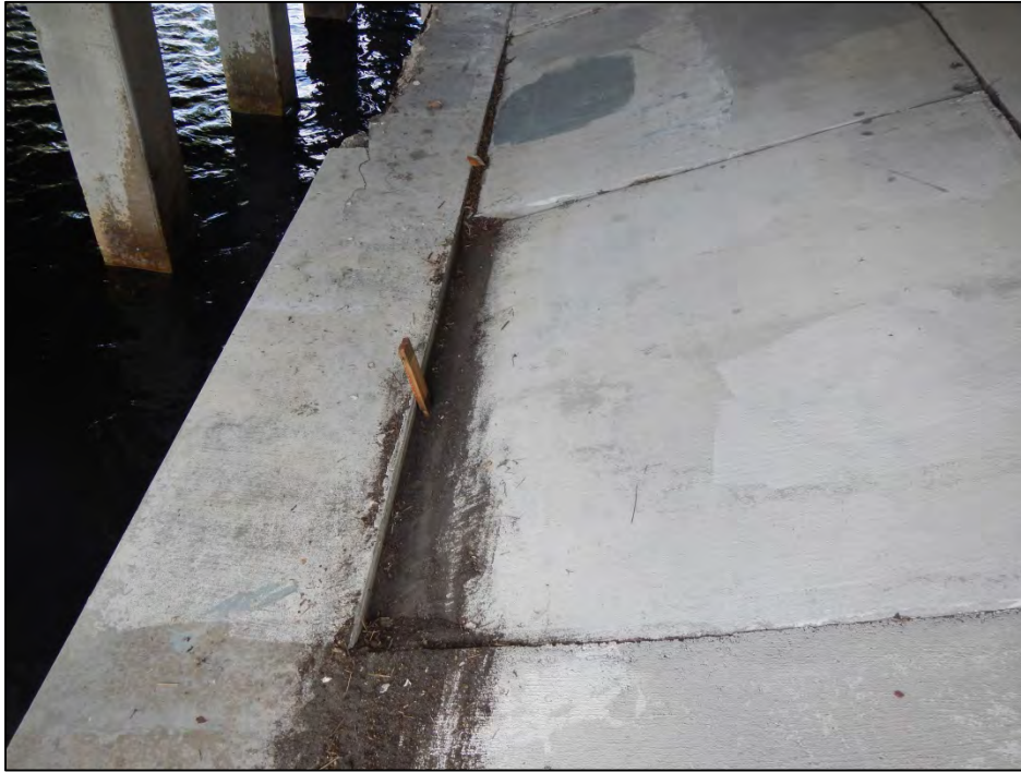
Photo 25 – Slope protection under Span 3 settlement.
