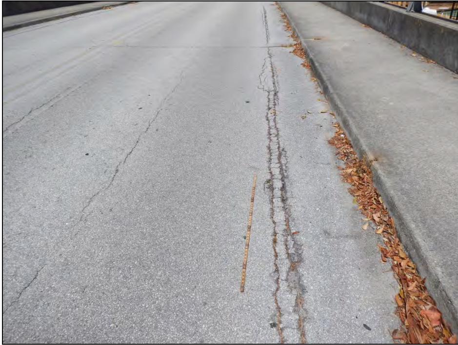
Photo 1 – Rutting in the asphalt overlay.
