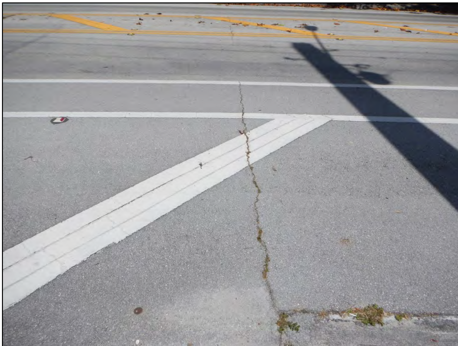
Photo 16 – The south approach roadway exhibits a transverse crack.
