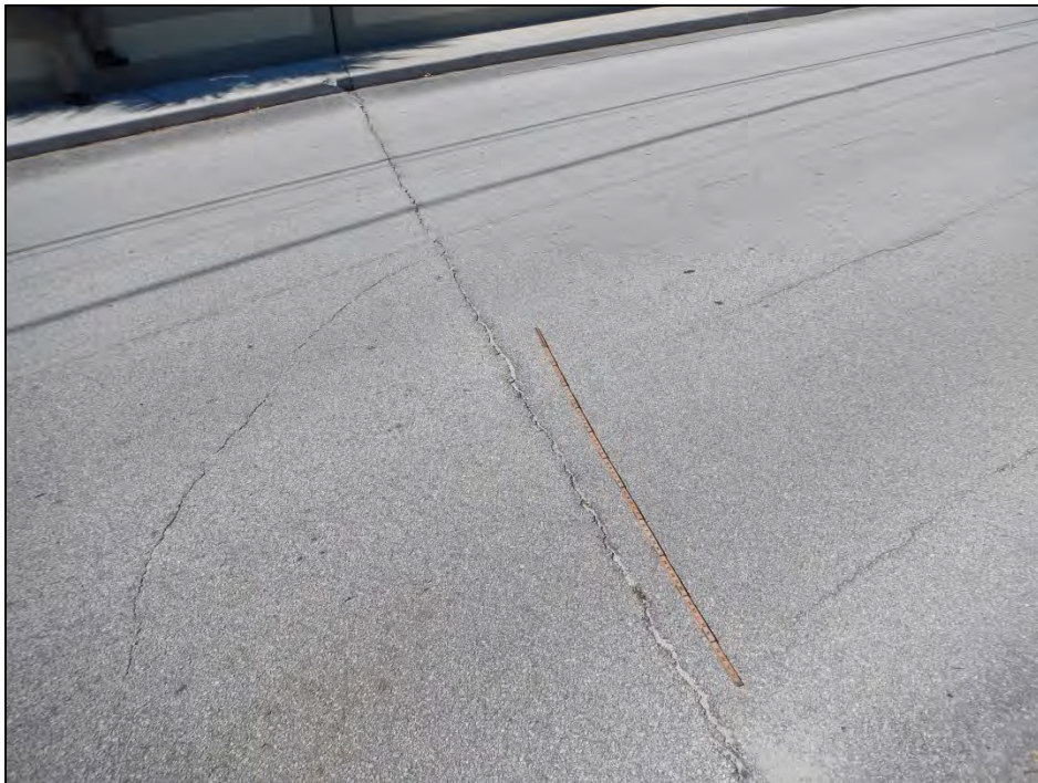
Photo 6 – Diagonal crack in asphalt over west approach slab.
