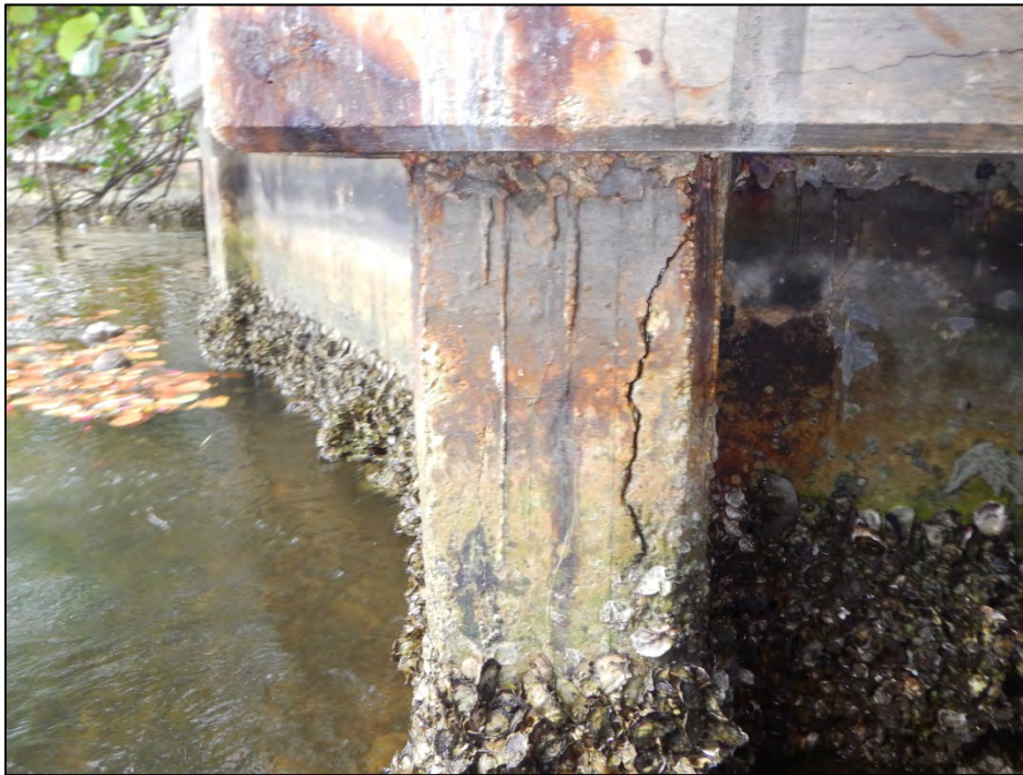
Photo 14 – Pile I-8 exhibits a vertical crack.
