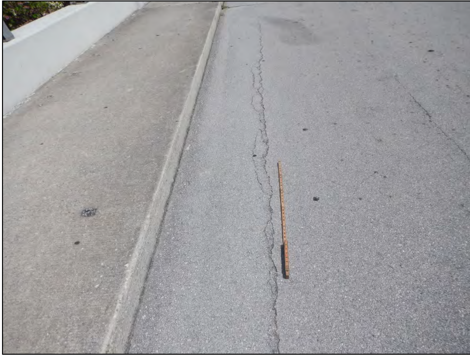
Photo 1 – Longitudinal cracks in asphalt overlay above the slab unit joints.
