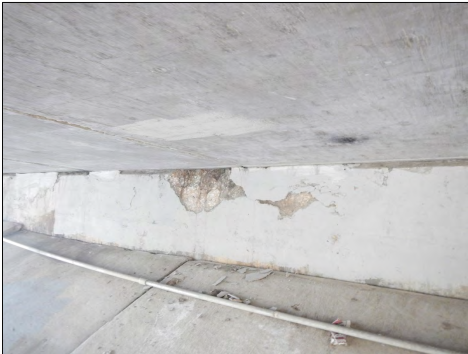
Photo 8 – Abutment 4 cap exhibits a spall under Slab Units 3-3 and 3-4.
