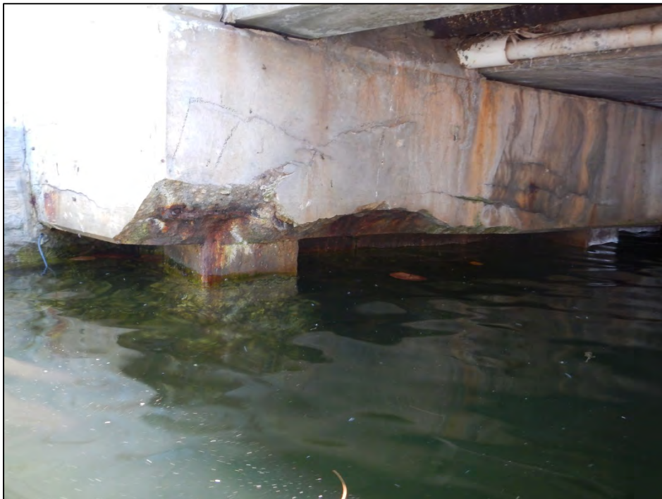
Photo 8 – Spalled area in Abutment 3 cap.
