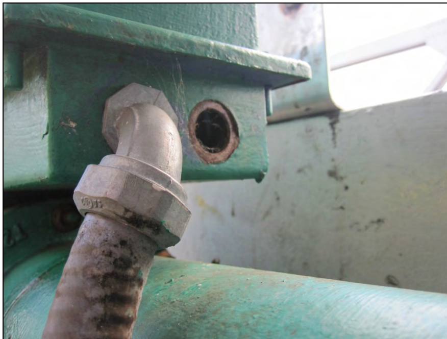
Photo 20 – Unplugged hole in Lock A limit switch enclosure.
