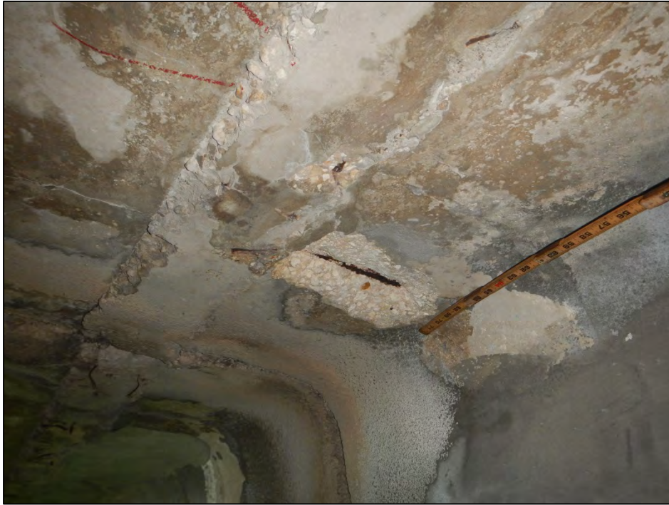
Photo 3 – Spall in the Double T-beam.
