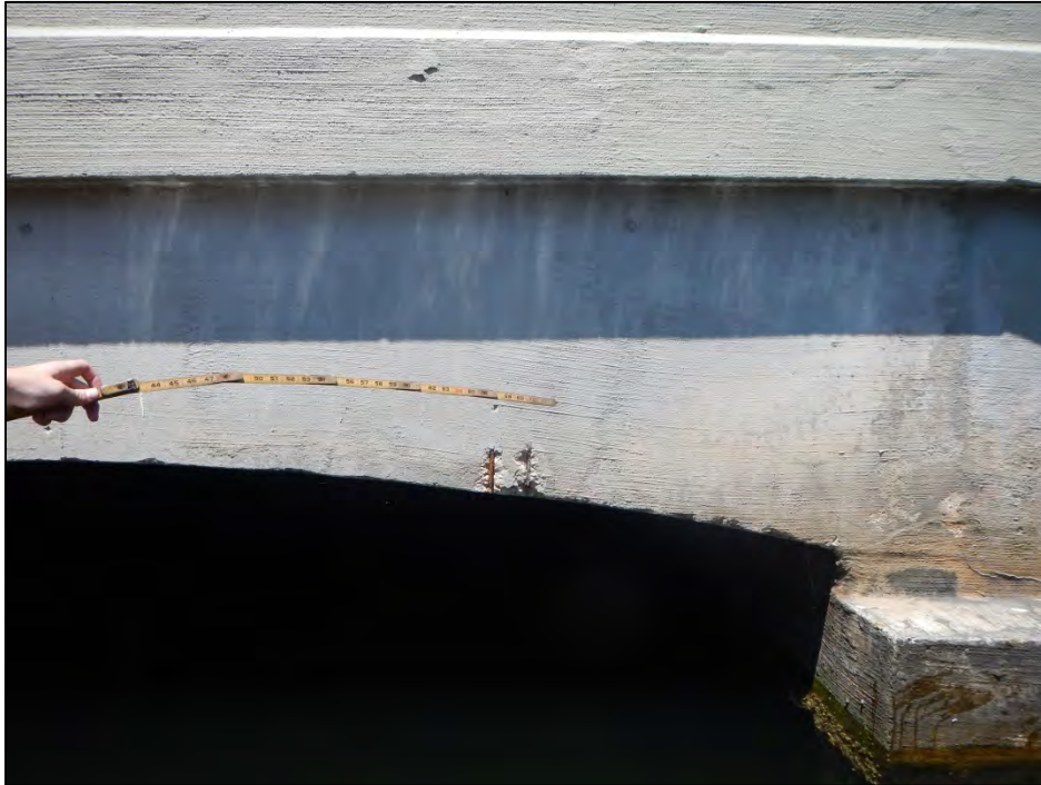
Photo 3 – Spall with exposed steel at east face of Span 1.
