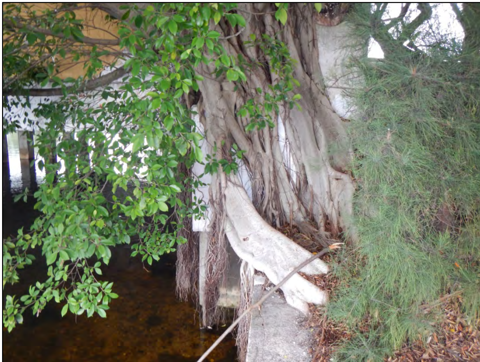
Photo 8 – Tree growth at End Bent 6 cap.
