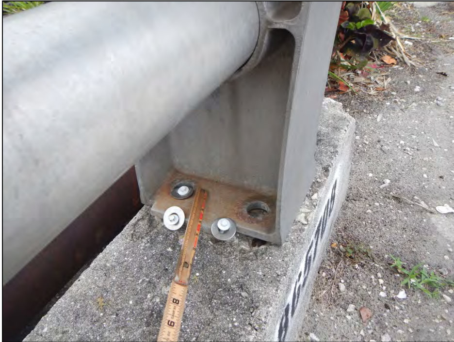
Photo 7 – West railing Post 3 not secured to rail. Note attempt to secure post.
