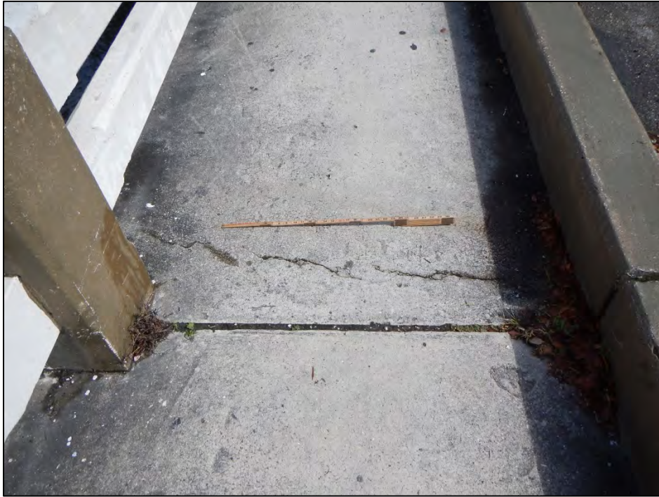
Photo 3 – West sidewalk transverse crack.
