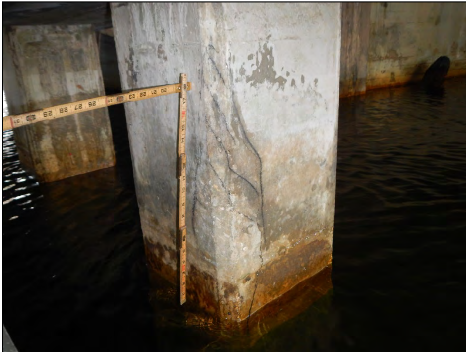
Photo 6 – The southwest corner of Pile 3-6 exhibits a delamination.
