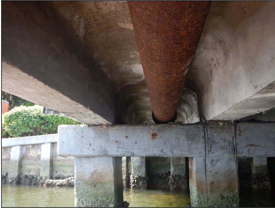
Typical Double T-Beam. Note Utility Pipe in the Bay.
