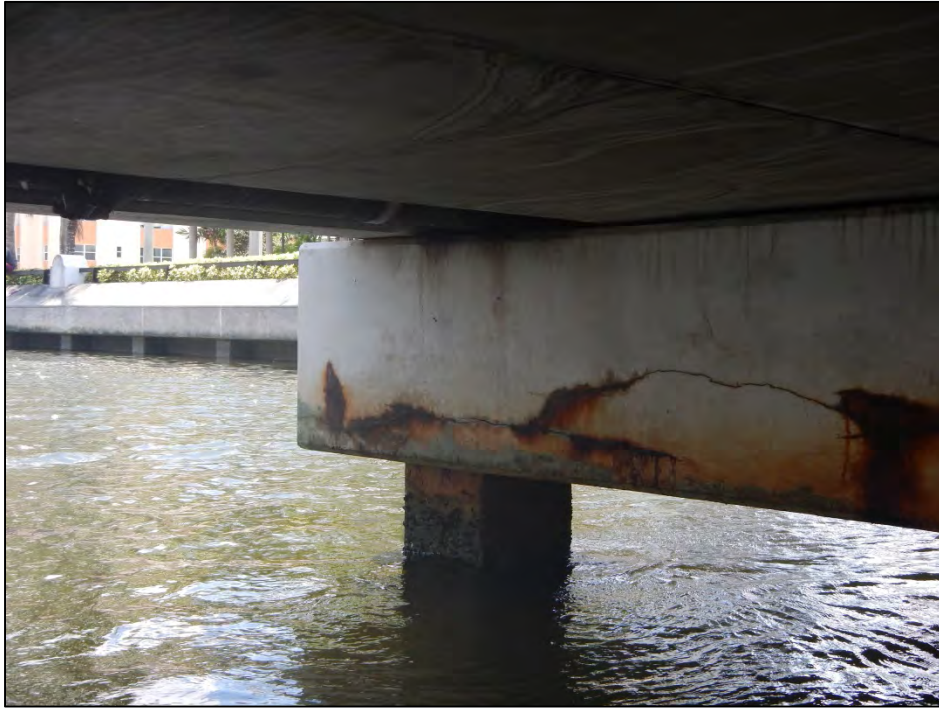
Photo 11 – Delamination in north face of Bent 2 cap.
