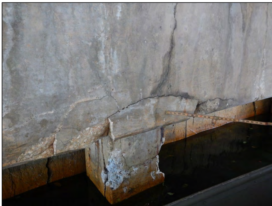
Photo 6 – Delamination/spall at Abutment I cap above Pile I-3. Note delaminated/spalled pile.
