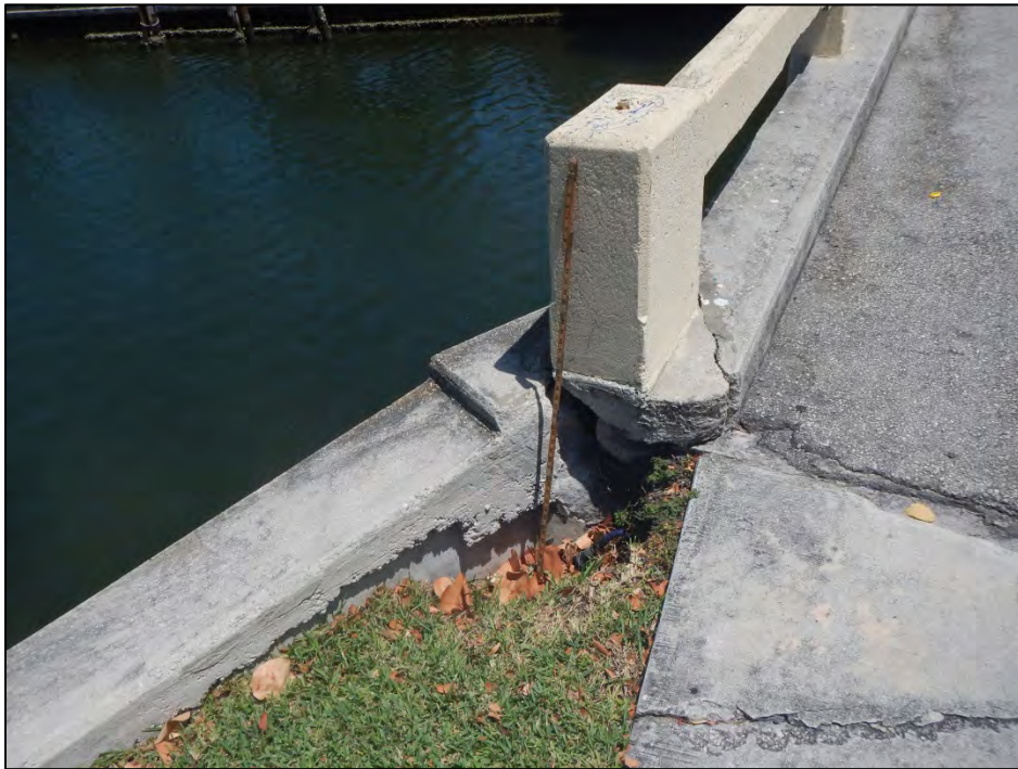
Photo 10 – Void behind the southwest retaining wall at railing post I-I.
