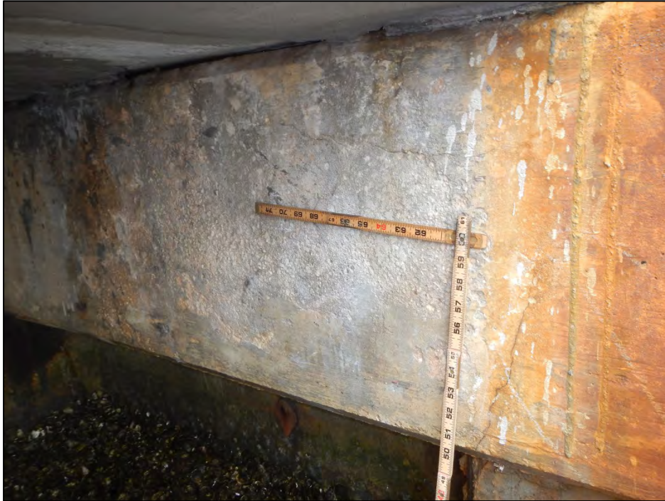
Photo 13 – Abutment I cap has a horizontal crack at the east end.
