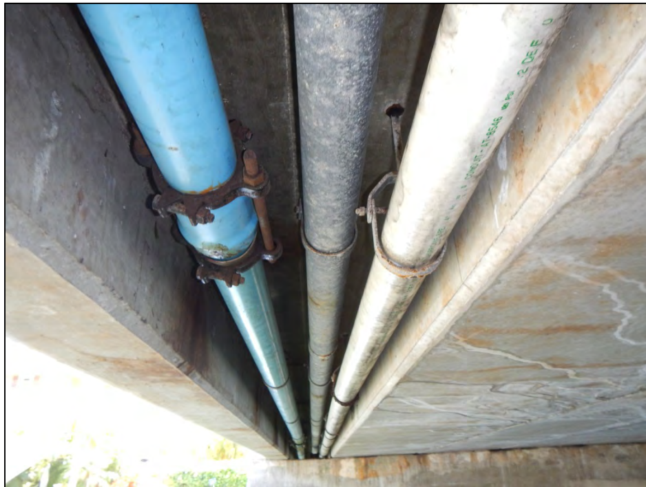
Concrete Slab Underside and Concrete T-beam. Note Utility Pipe.
