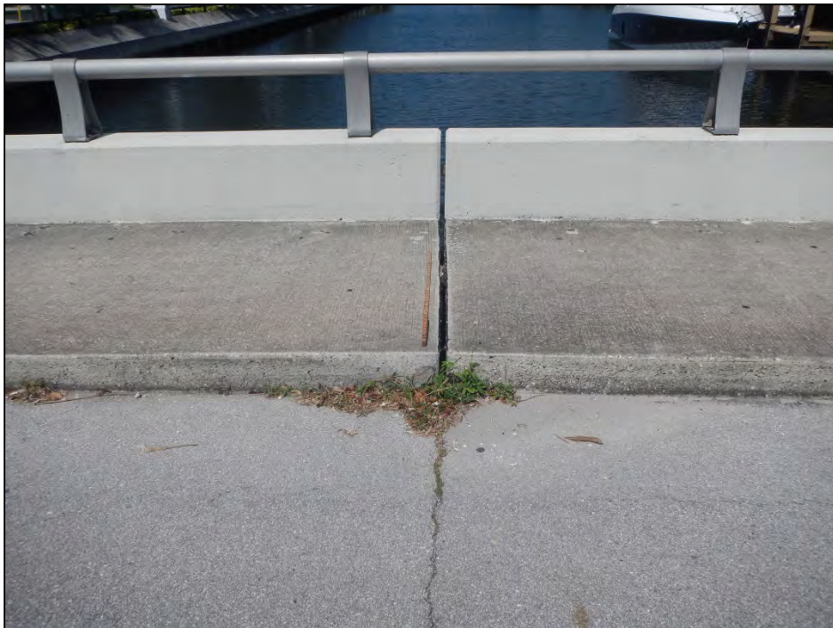
Photo 4 – Deteriorated sidewalk joint.
