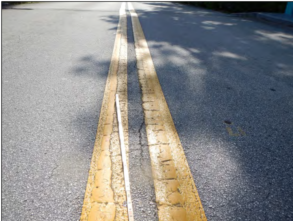
Photo 2 – The deck top exhibits intermittent longitudinal cracks.
