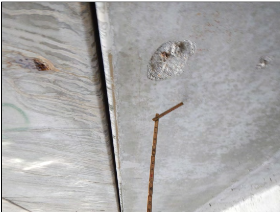
Photo 6 – Slab 1-4 exhibits a spall adjacent to slab 1-3.
