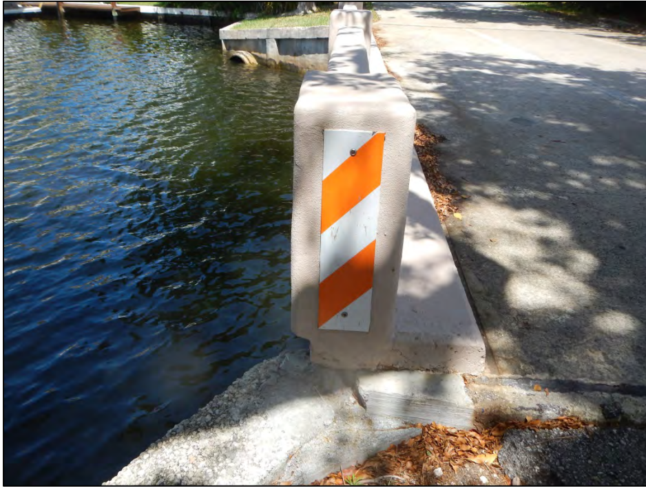
Photo 7 – The northwest corner object marker diagonal striping is oriented incorrectly.
