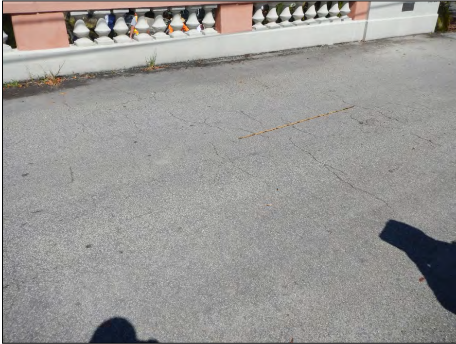
Photo 1 – Delaminated and cracked asphalt overlay.
