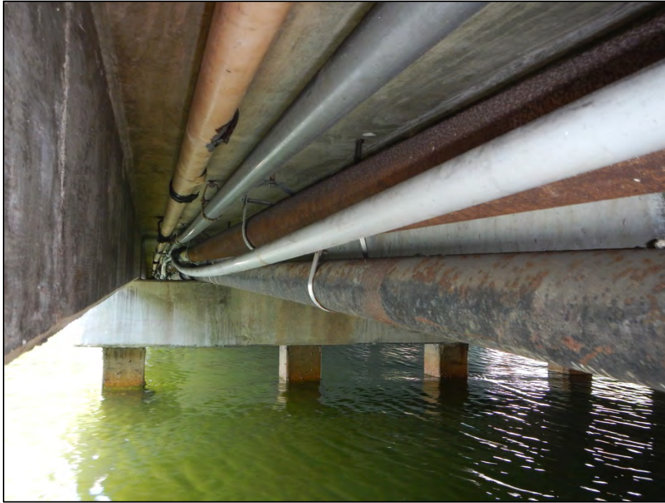
Utilities mounted to deck underside
