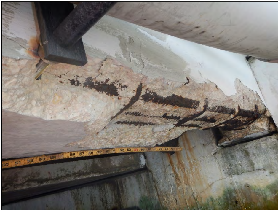
Photo 8 – Spall with exposed corroded rebar in Beam 3-2.
