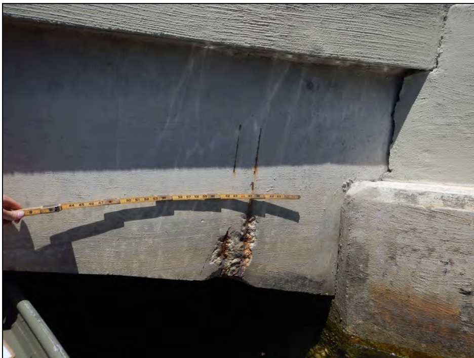
Photo 4 – Spall with exposed steel at east face of Span 2.
