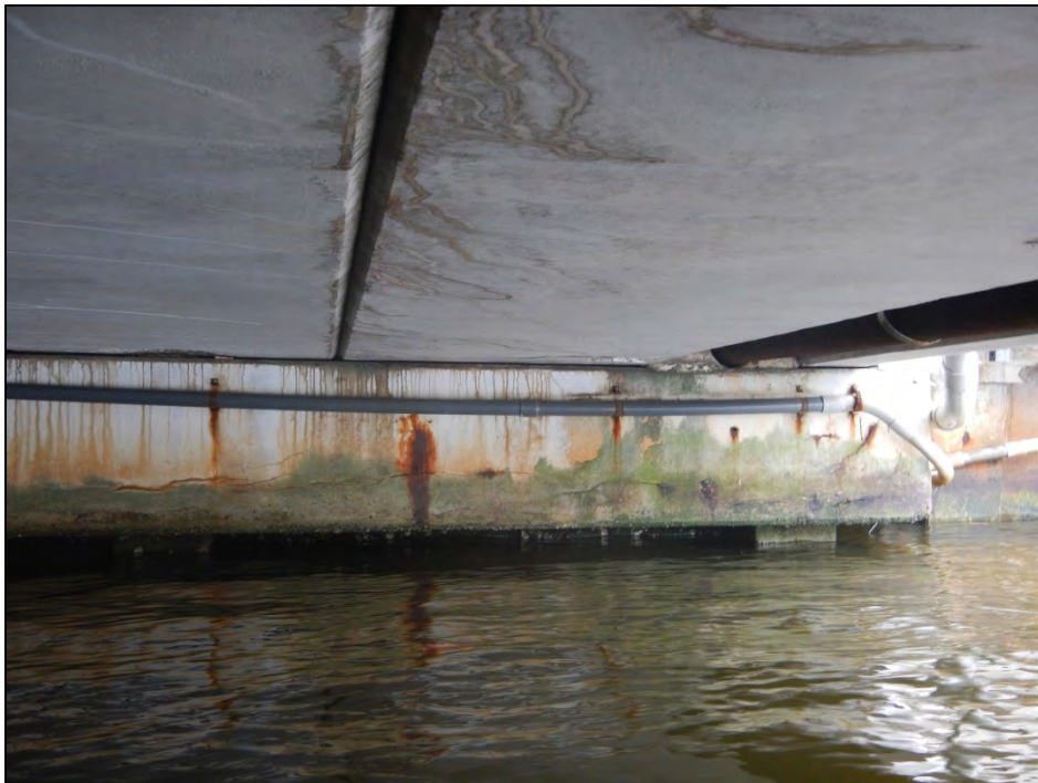
Photo 10 – Delamination at Abutment 4 cap.
