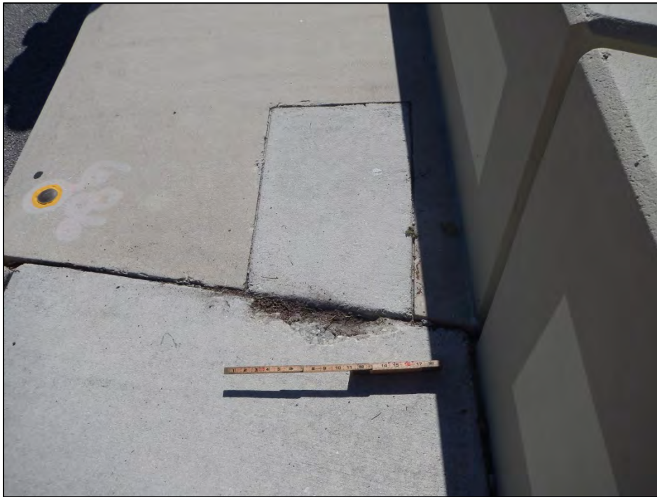
Photo 10 – Spall in northeast approach sidewalk.
