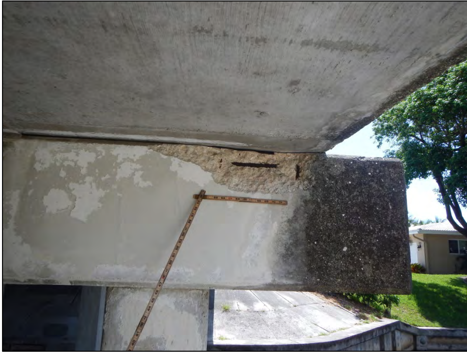
Photo 13 – The south end of Bent 2 cap exhibits a spall with exposed steel.
