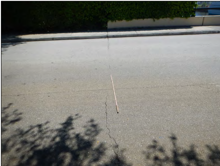
Photo 4 – Typical transverse cracks in asphalt surfacing at end of approach slab.
