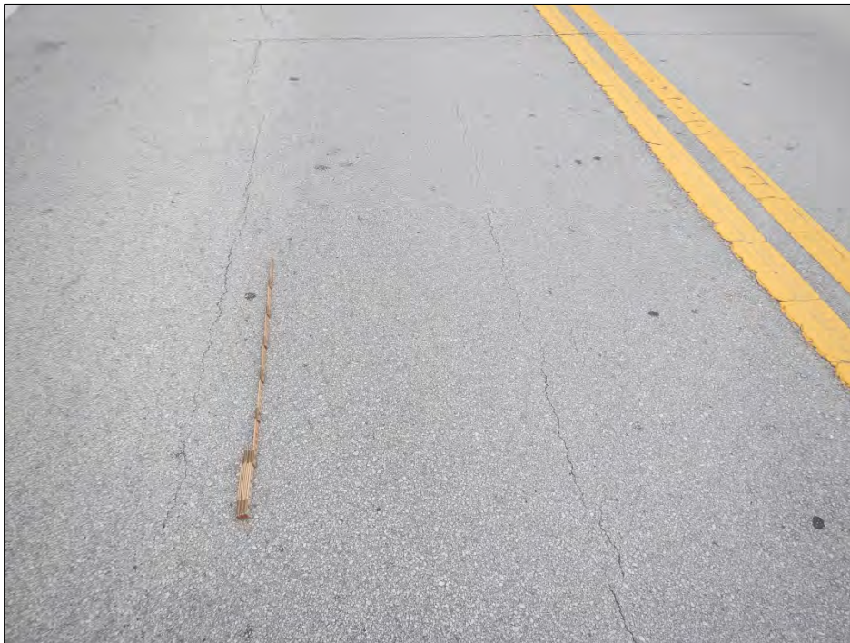
Photo 2 – Span 1 deck top longitudinal cracks.
