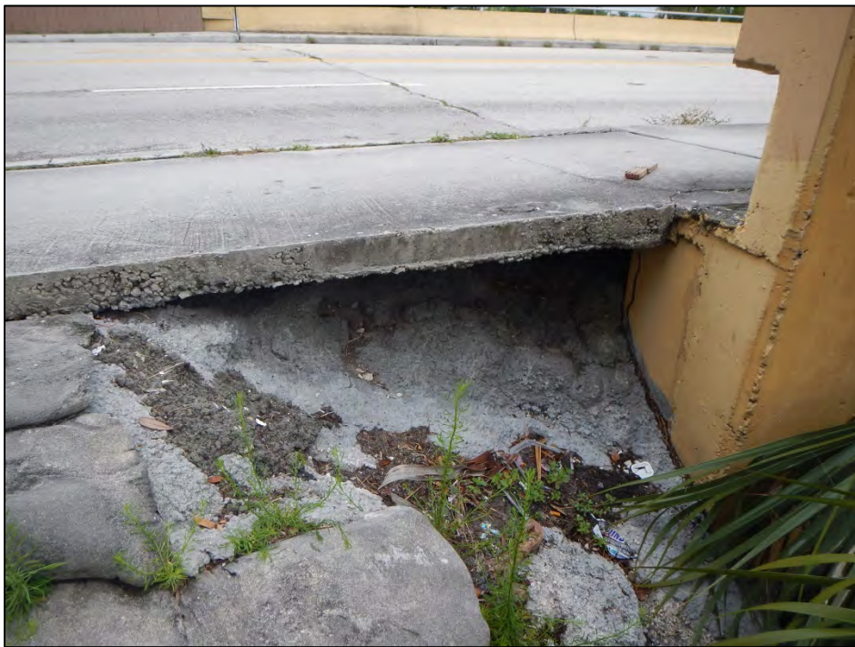
Photo 18 – Southeast approach sidewalk undermining.
