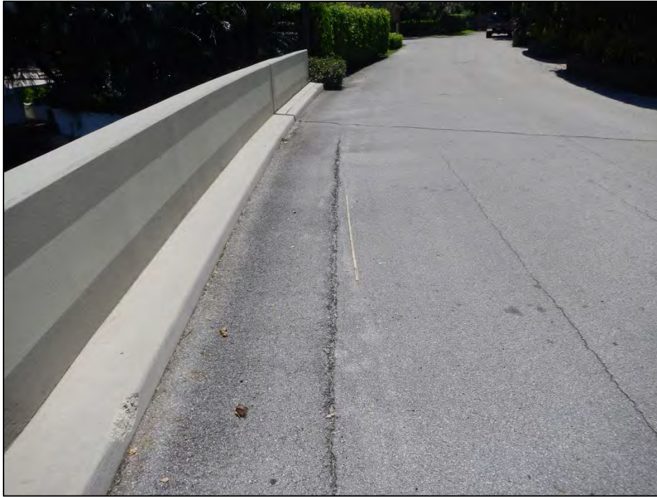
Photo 1 – Cracks in asphalt overlay.
