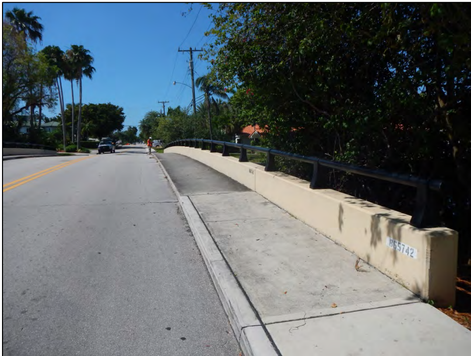
Typical Bridge Railing
