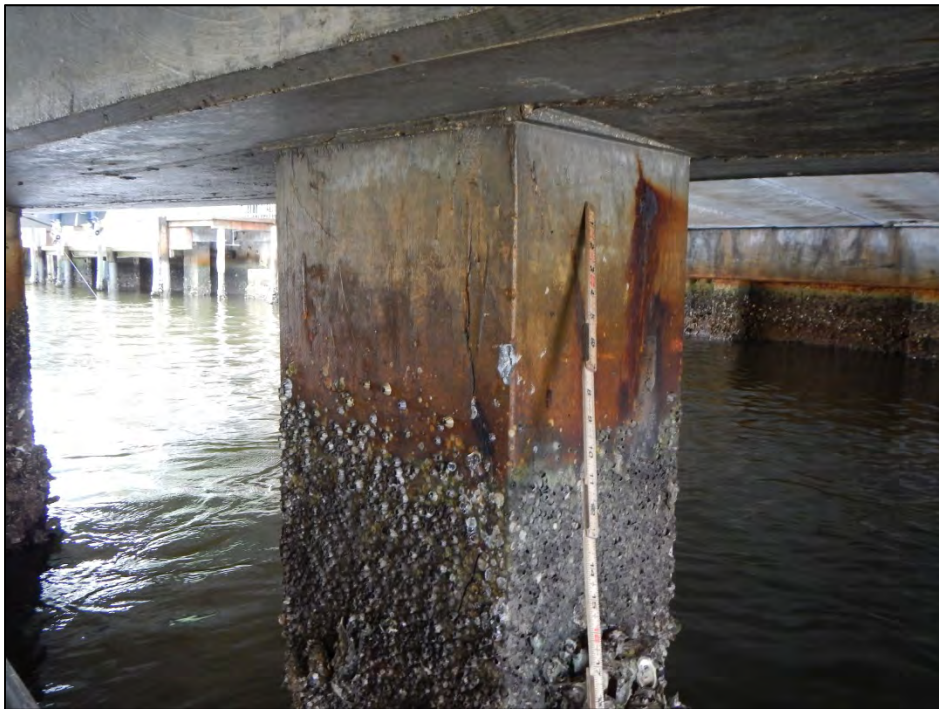
Photo 8 – Typical delamination and corrosion staining on Pile 3-4.
