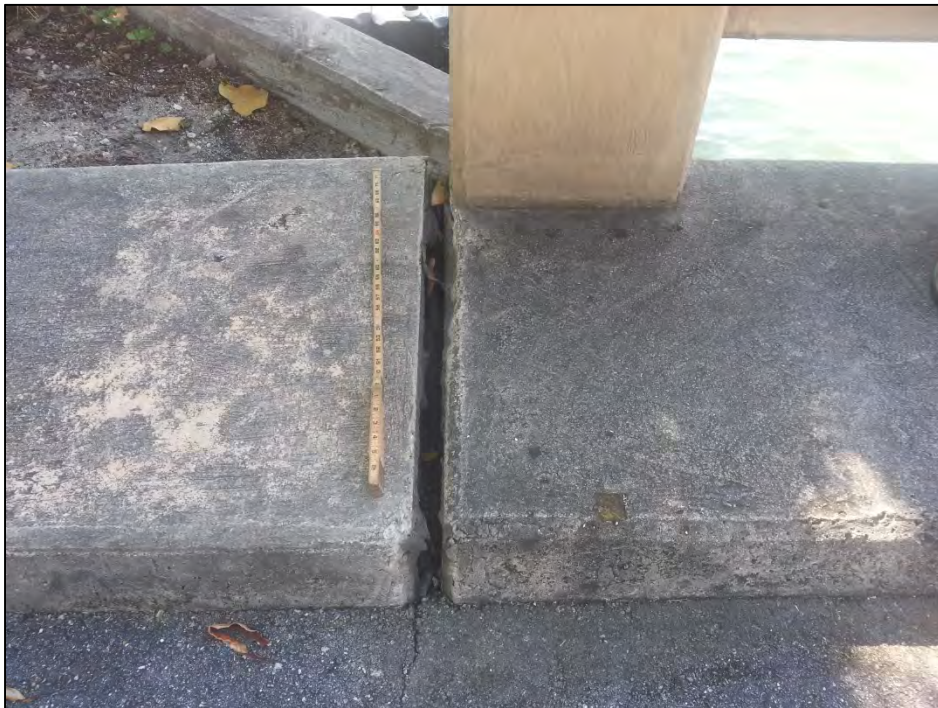
Photo 2 – Complete adhesion failure of the joints in the left sidewalk.
