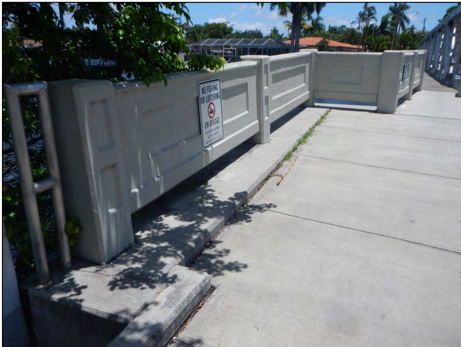
Photo 4 – Typical deteriorated approach sidewalk seal.
