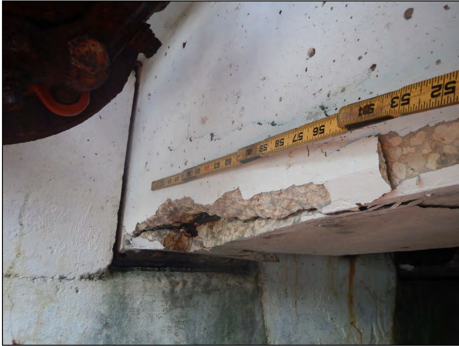
Photo 7 – Spalls with exposed corroded rebar in Beam 3-1.
