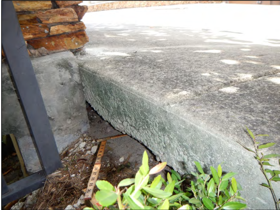
Photo 13 – The northwest sidewalk exhibits undermining.
