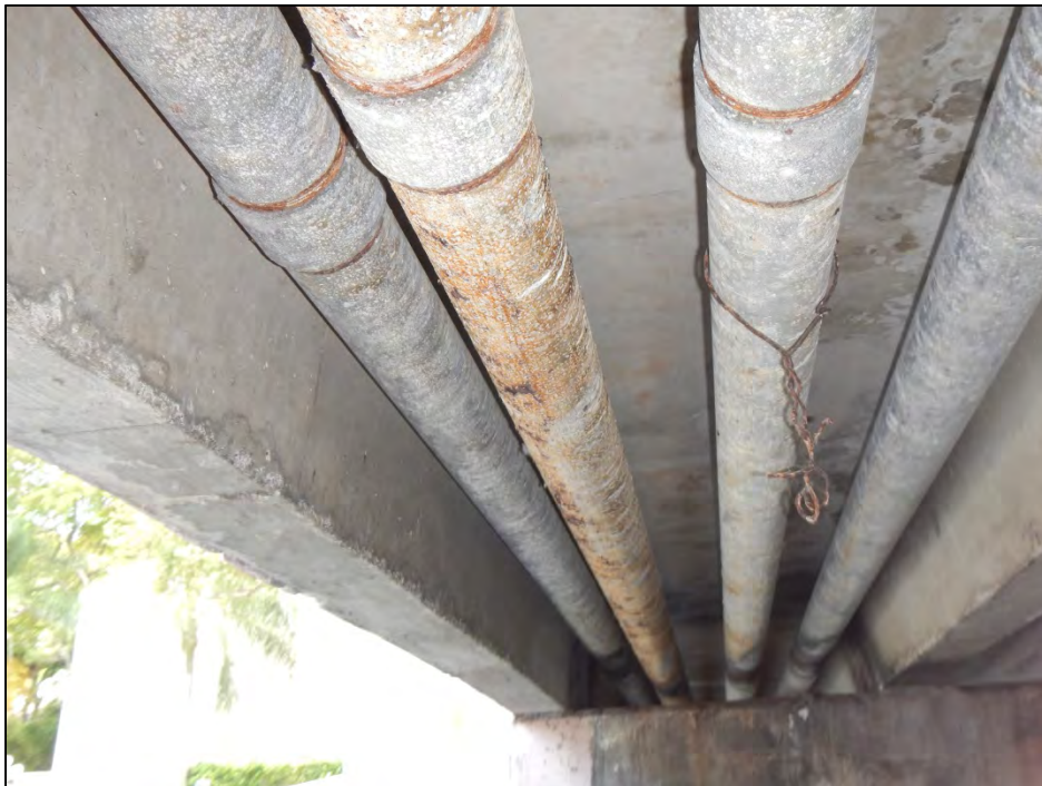
Utilities Mounted under East Side of Bridge
