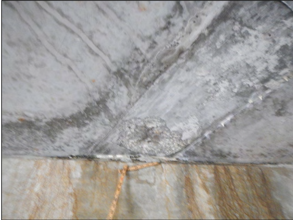
Photo 9 – Spall at the joint between Slab Units 2-2 and 2-3.
