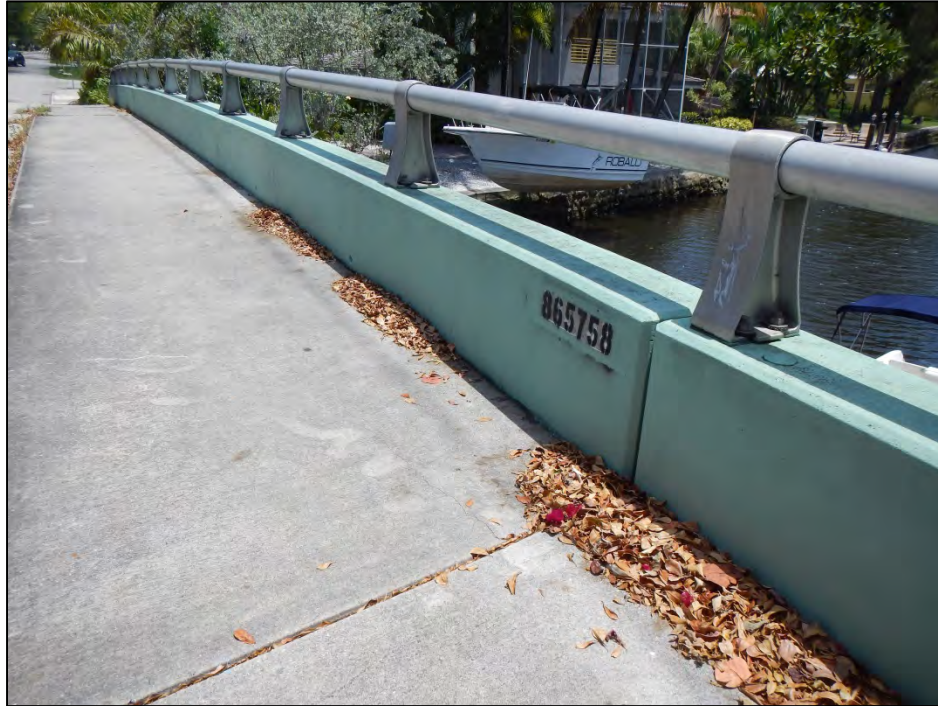
Typical Bridge Railing
