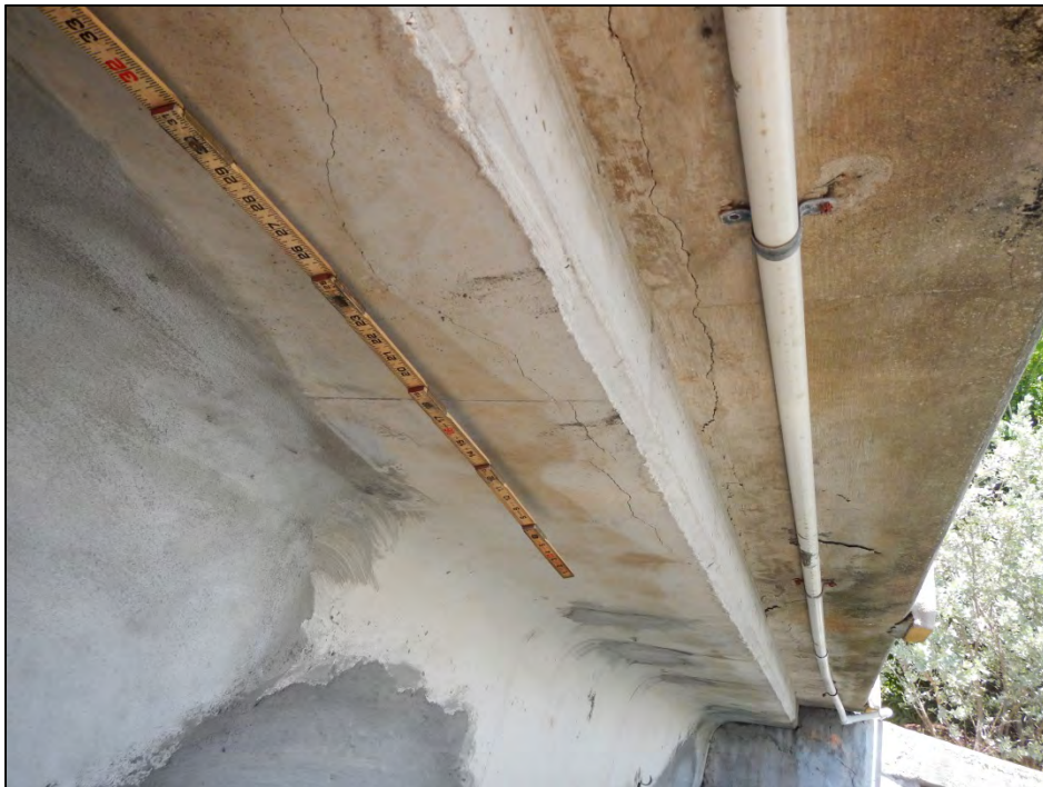
Photo 4 – The south fascia over Span 2 exhibits a long crack and delamination.
