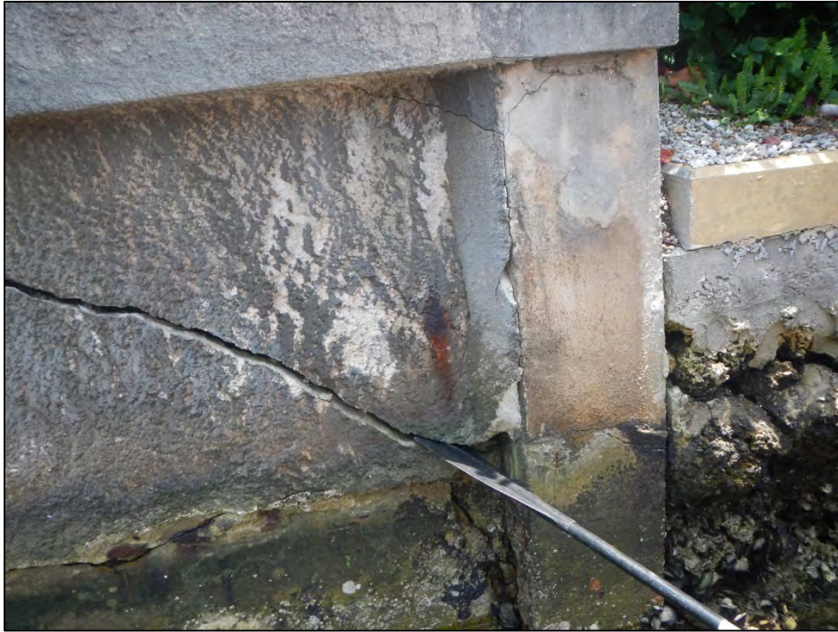
Photo 7 – Southwest wingwall crack/fracture.
