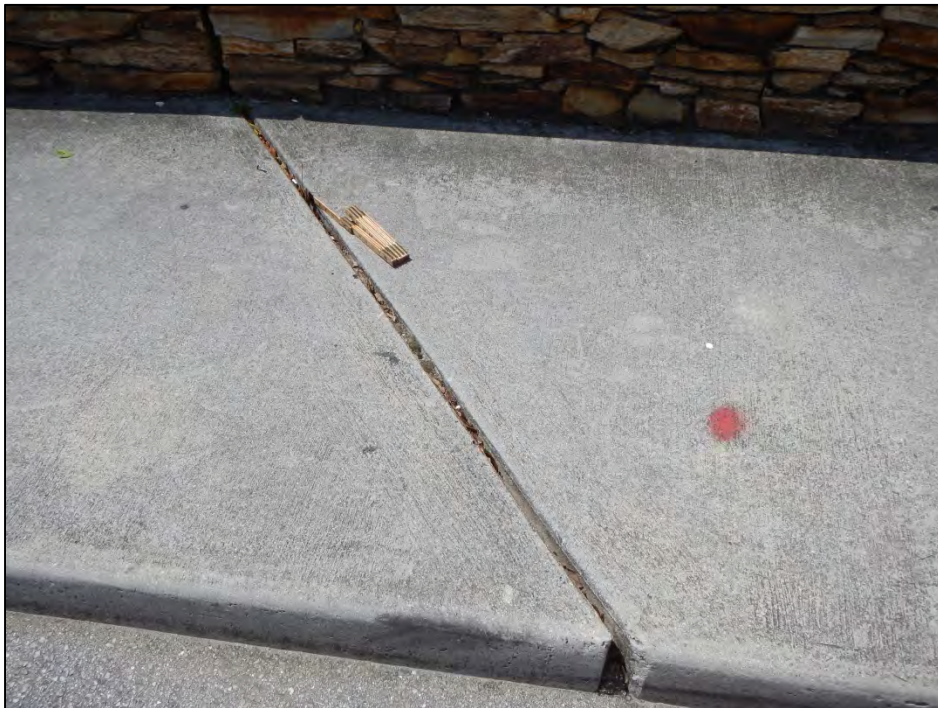
Photo 2 – The right sidewalk joint seal over Bent 3 is deteriorated.
