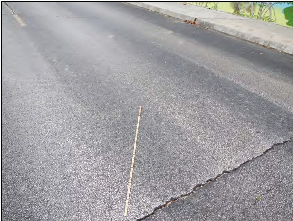
Photo 16 – West approach slab diagonal crack.
