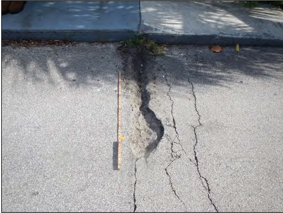
Photo 3 – The westbound deck top exhibits a pothole over Abutment I.
