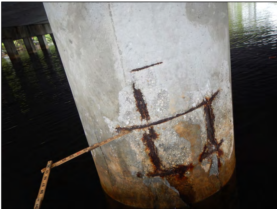
Photo 12 – Pile 3-11 exhibits a spall with exposed steel.
