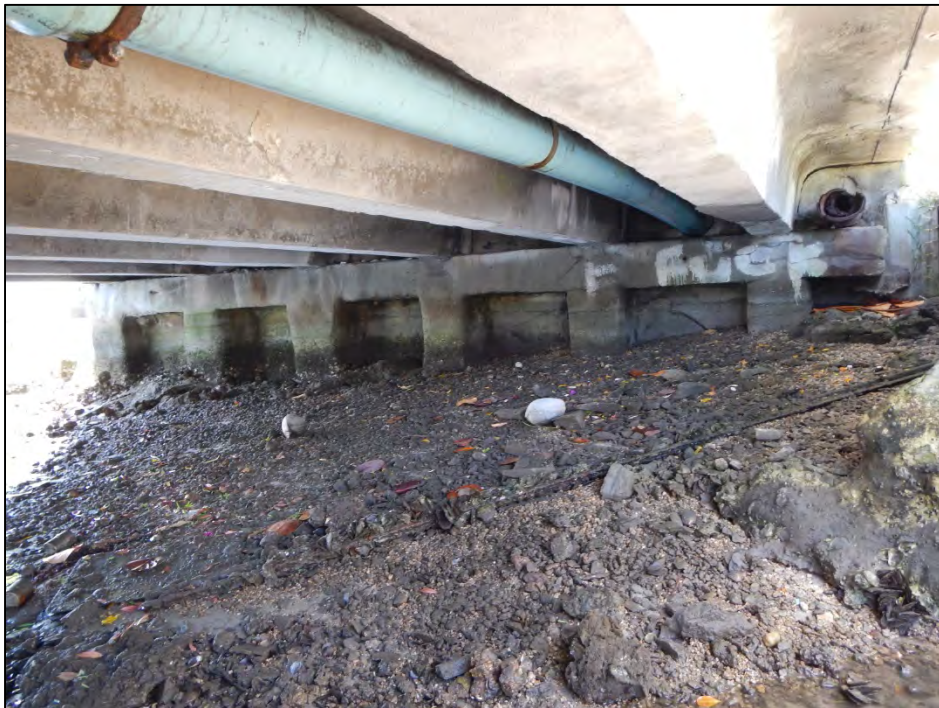
Photo 4 – Abutment 4 face with typical repair patches.
