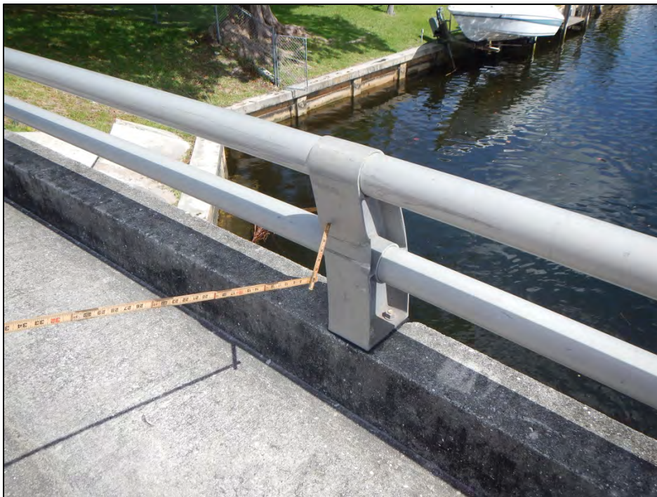
Photo 8 – Post 2-2 Left exhibits impact damage.
