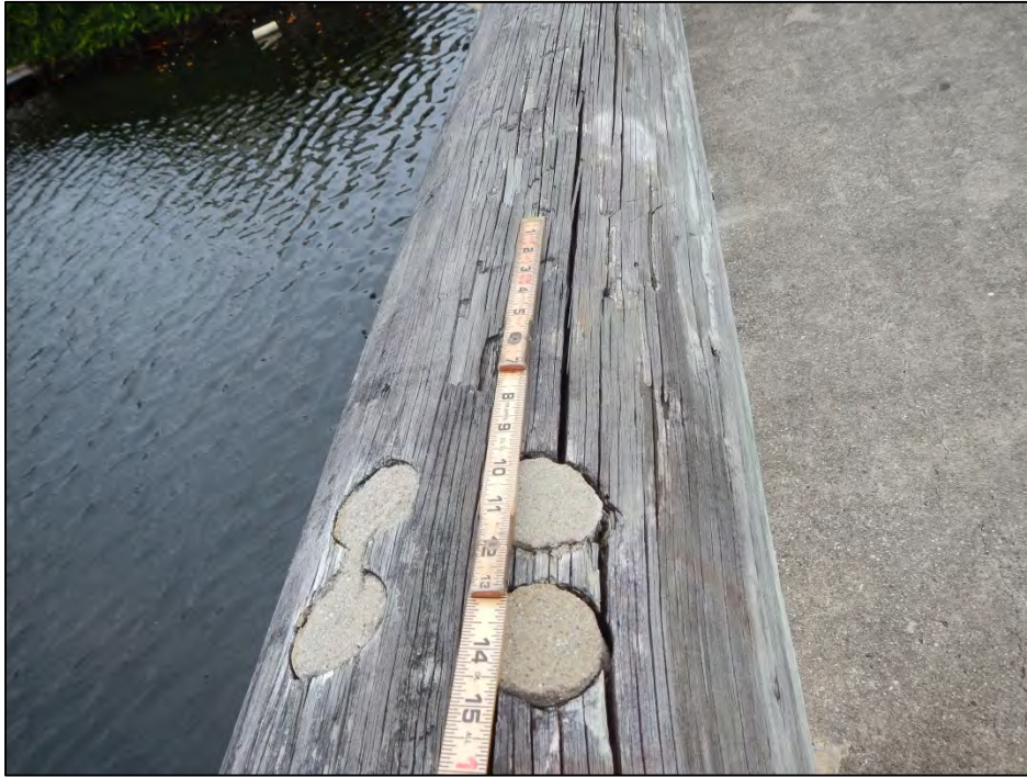
Photo 3 – Timber rail splitting.
