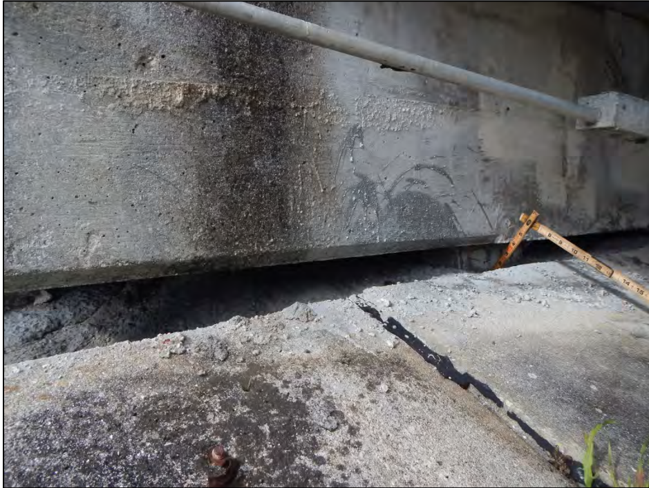
Photo 15 – The End Bent I cap has separated from the slope protection.
