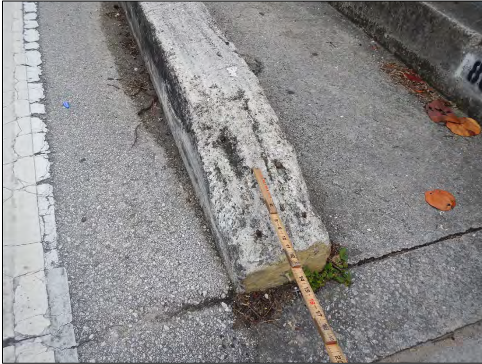
Photo 3 – East curb south end spall with exposed steel.
