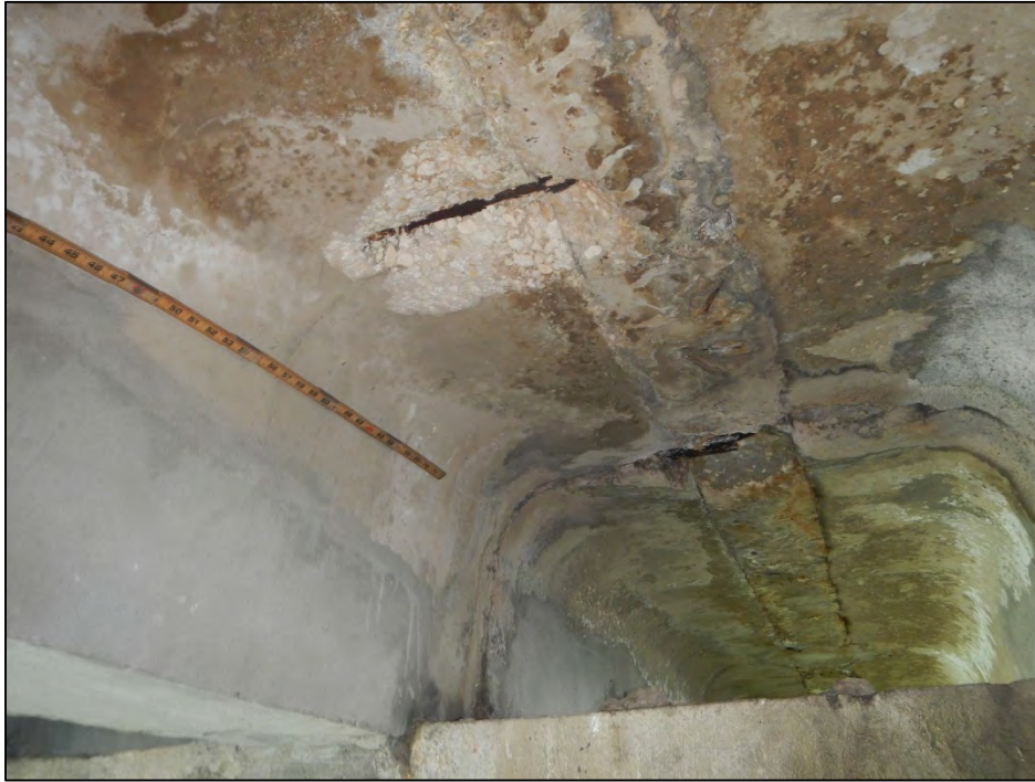
Photo 3 – Spall with exposed reinforcing in the top flange of the left leg of Beam 1-2.
