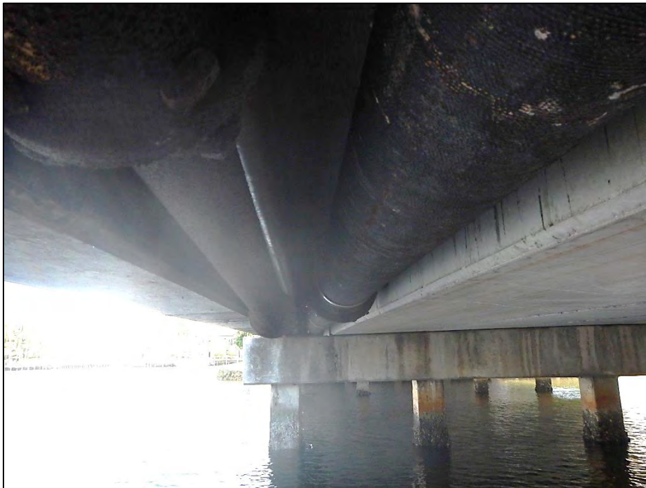
Utilities mounted to deck underside
