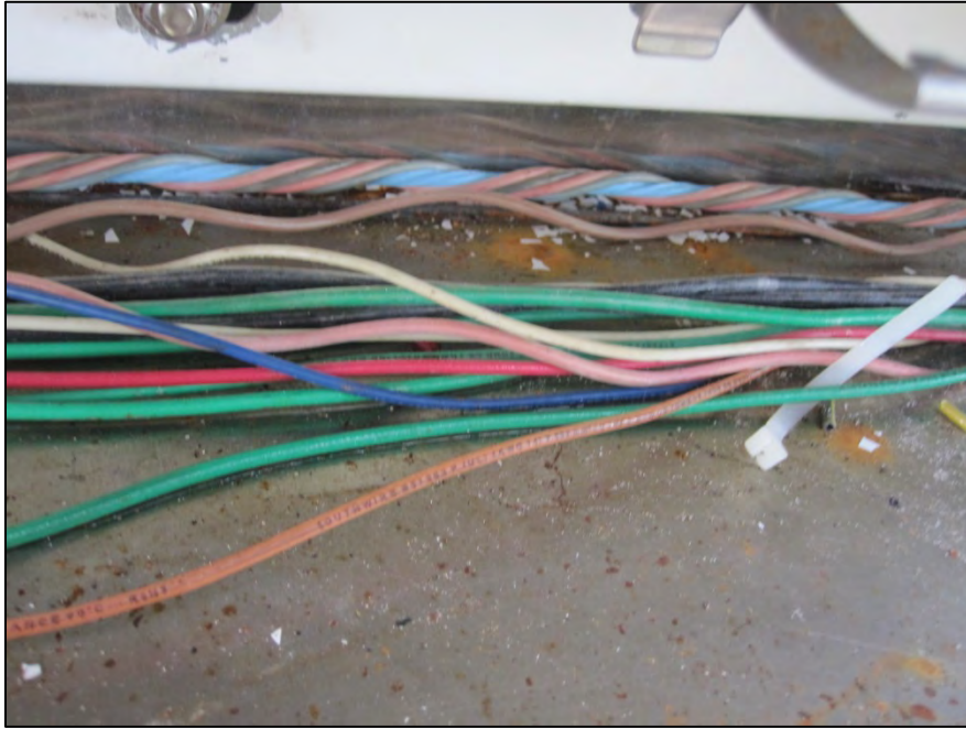
Photo 25 – Evidence of water intrusion at the terminal box in the machinery area.
