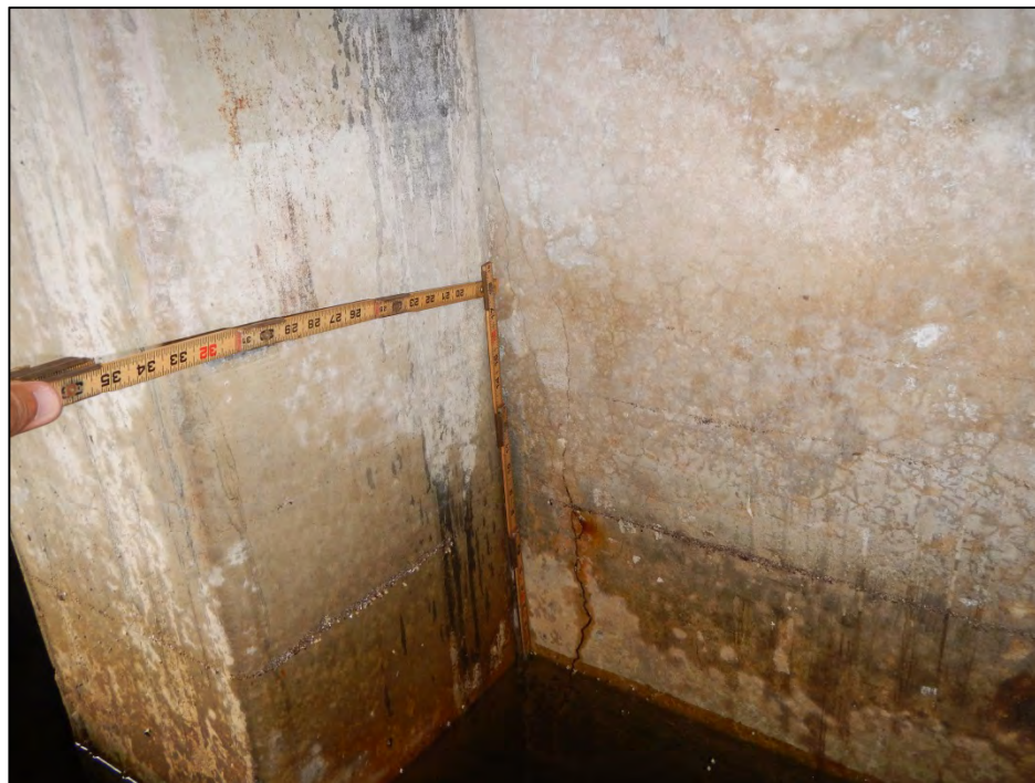
Photo 10 – The End Bent I retaining wall north of Pile I-7 exhibits a vertical crack.
