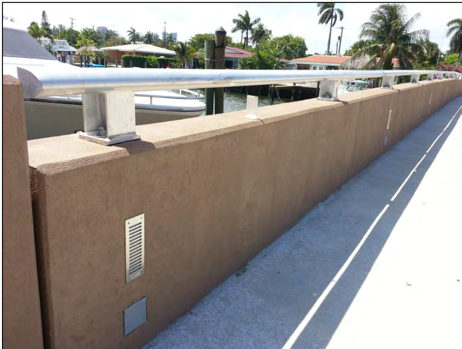
Typical Bridge Railing
