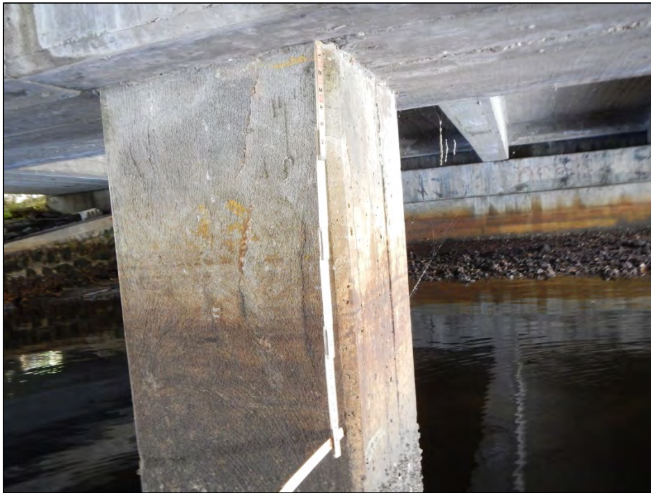
Photo 8 – Delamination at the northwest corner of Pile 2-5.
