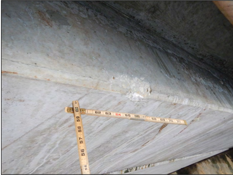
Photo 1 – Spall in the deck underside, Slab Unit I-I.
