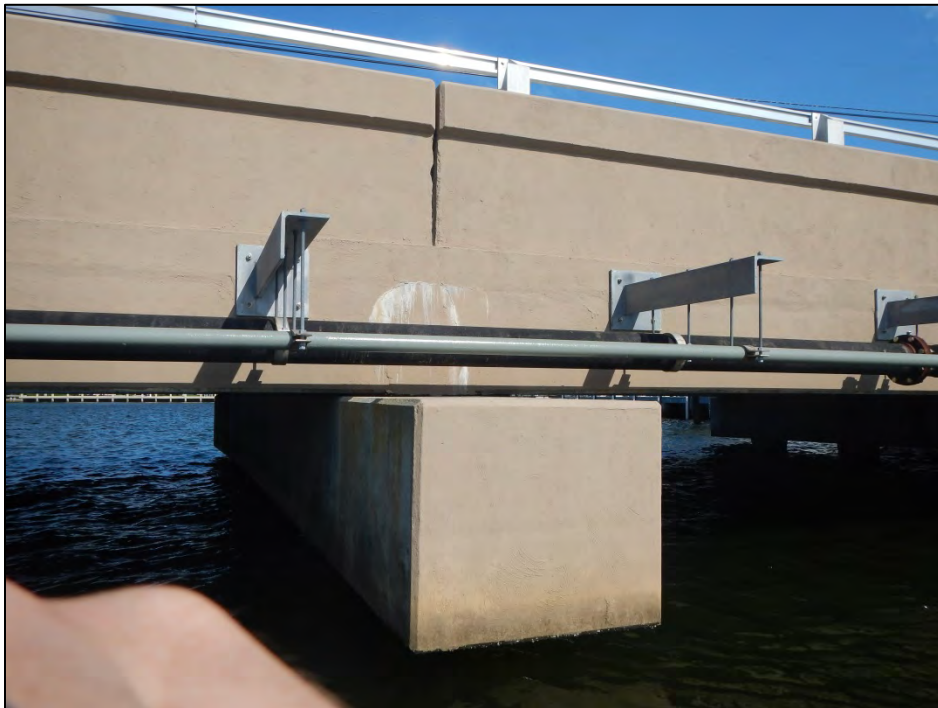
Photo 2 – Cracks in the slab unit over each bent.
