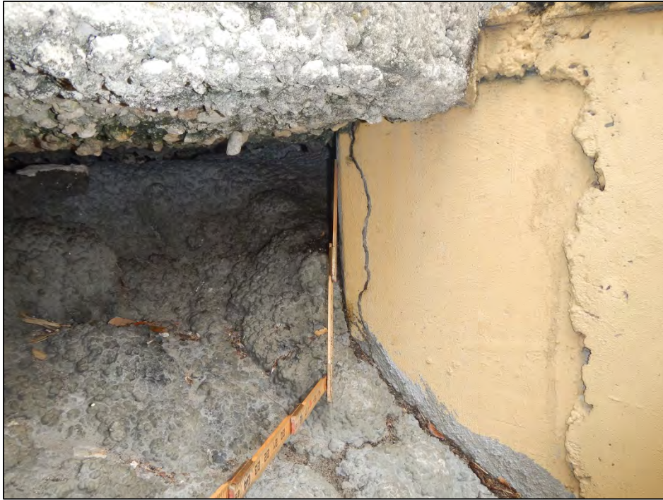
Photo 19 – Southeast wingwall exhibits a delamination.
