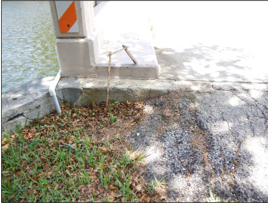
Photo 7 – The northwest corner is missing the sidewalk transition.
