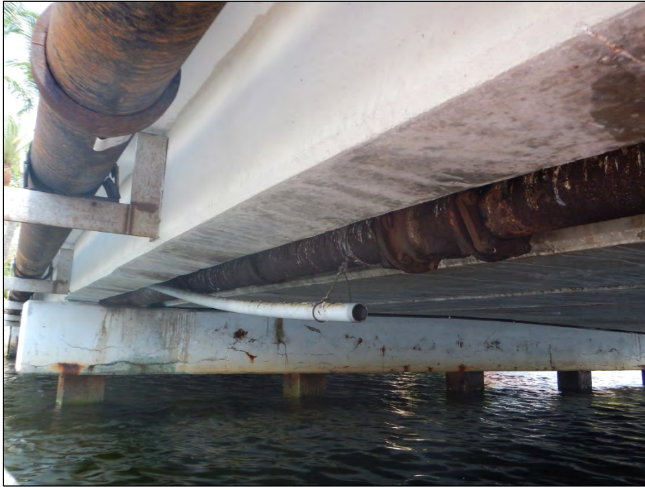
Utilities mounted to deck underside
