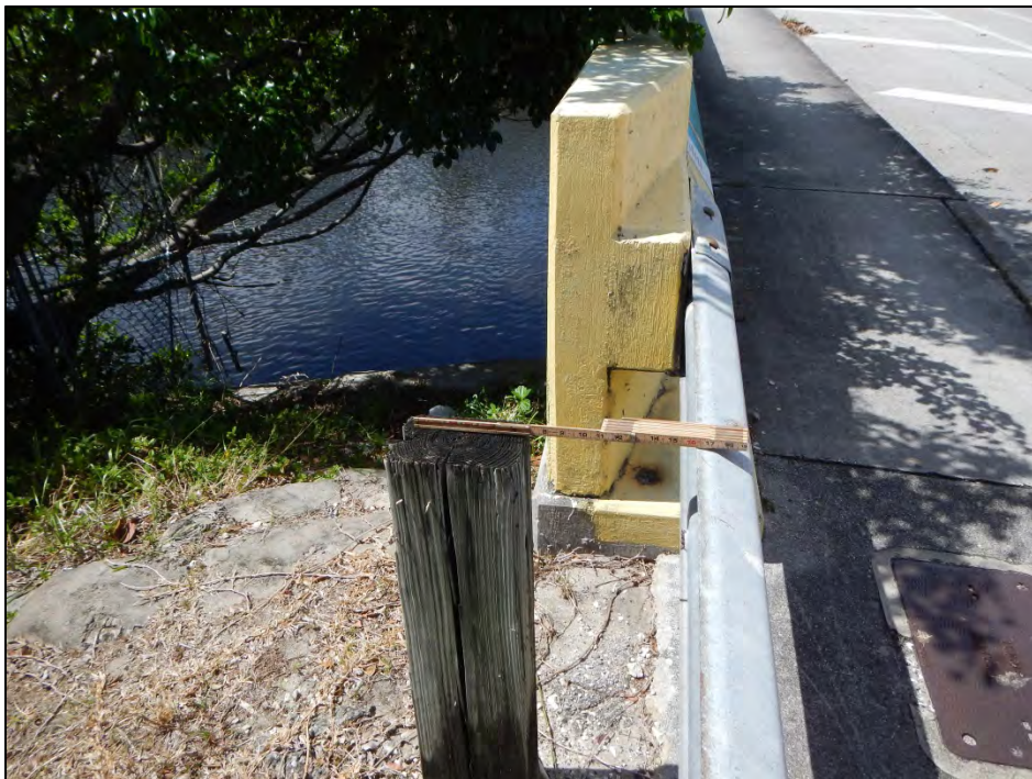
Photo 20 – Southwest guardrail cushion block missing.
