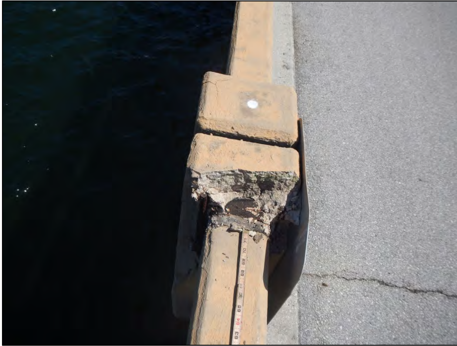
Photo 1 – Spall in Post 5-1, right.
