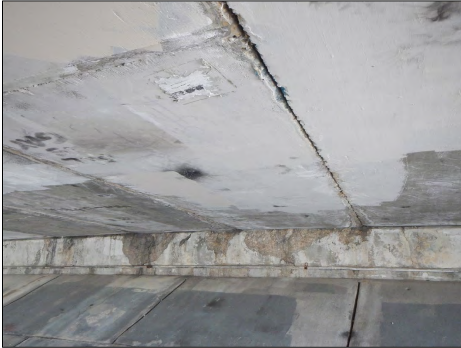
Photo 9 – End Bent 1 cap exhibits spalls between Slab Units 1-5 and 1-7.
