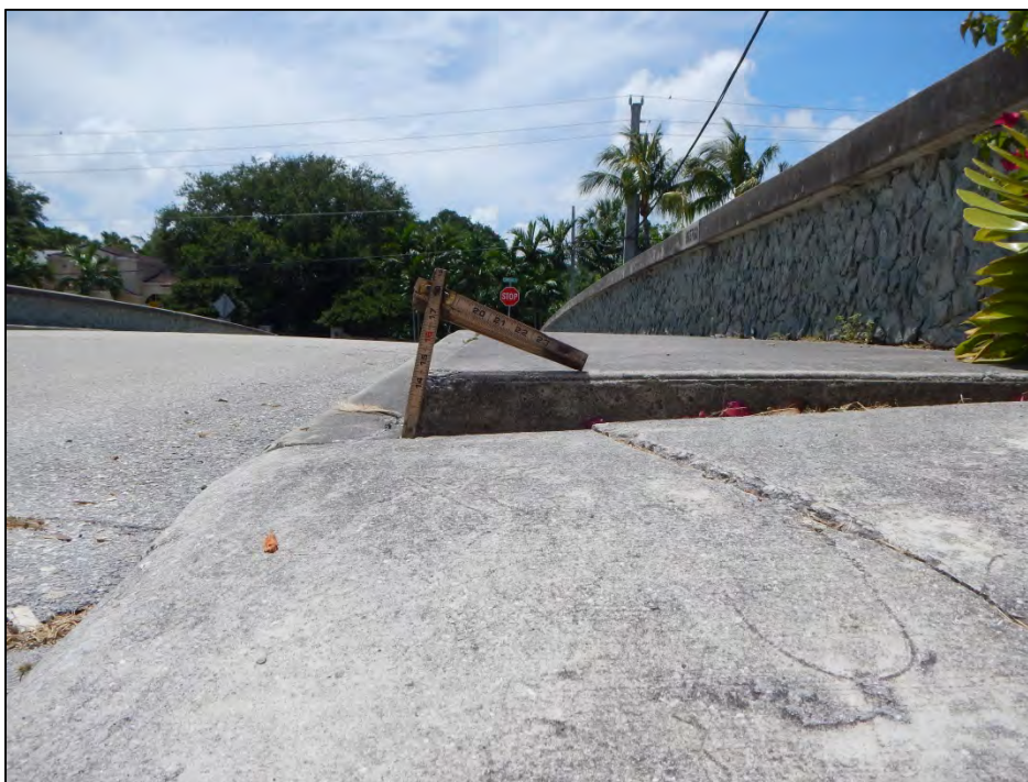
Photo 5 – Elevation differential in the northeast approach sidewalk.
