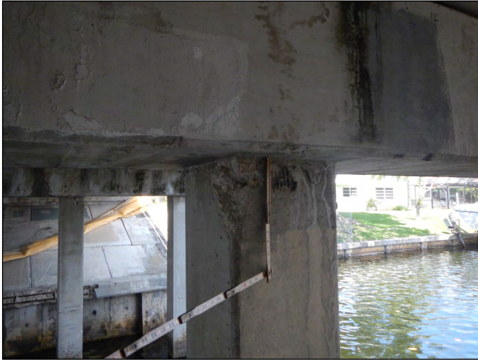
Photo 19 – The southeast corner of Pile 3-2 exhibits a spall.
