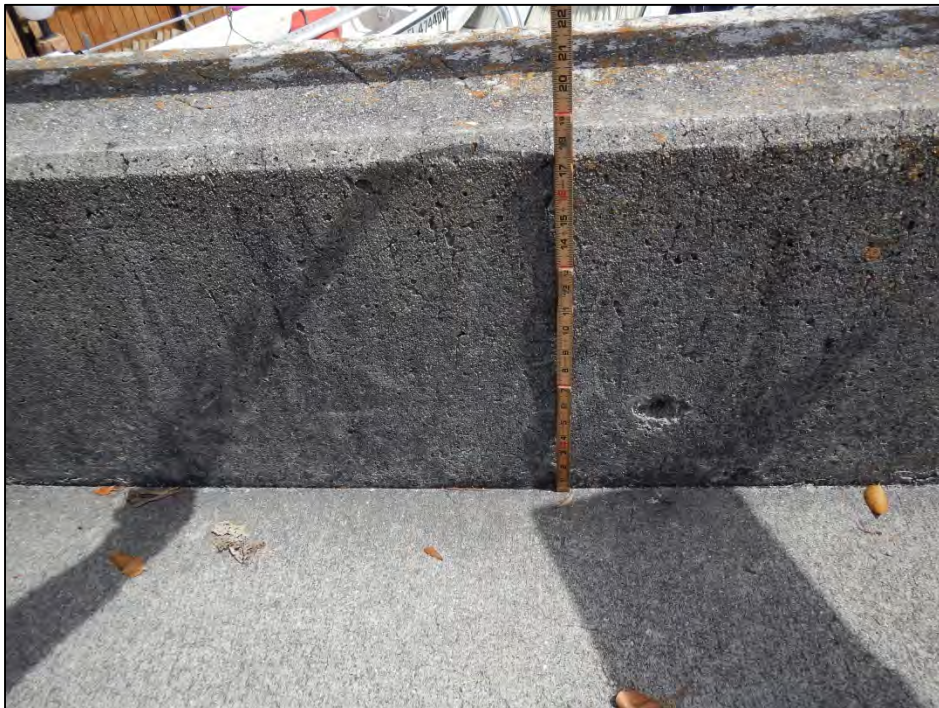
Photo 2 – Spall in the south face of the left parapet.
