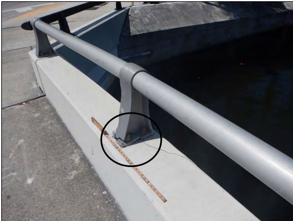
Photo 4 – Fractured handrail support in Span 1 at the left parapet.
