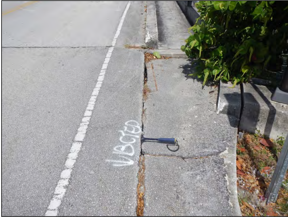
Photo 23 – Northeast approach slab between the sidewalk is not sealed.
