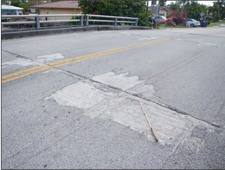
Photo 3 – Disintegrated asphalt over Bent 2.
