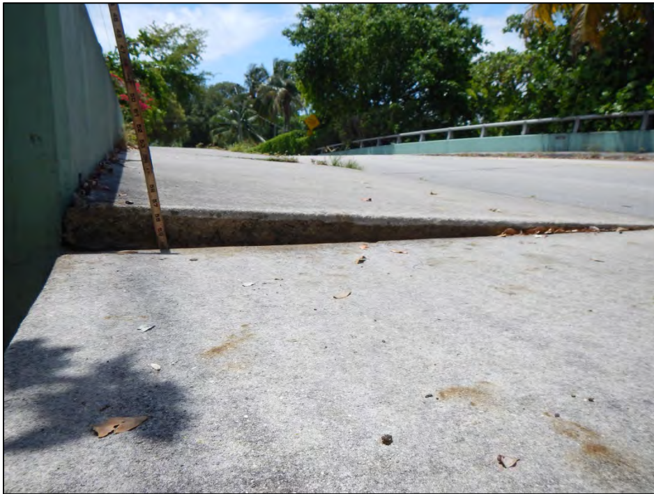
Photo 4 – Settlement of the northeast approach sidewalk.
