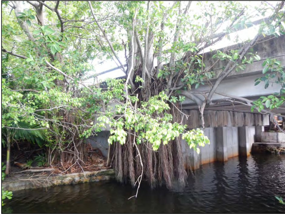
Photo 3 – Tree growing at the south end of the Abutment I cap.
