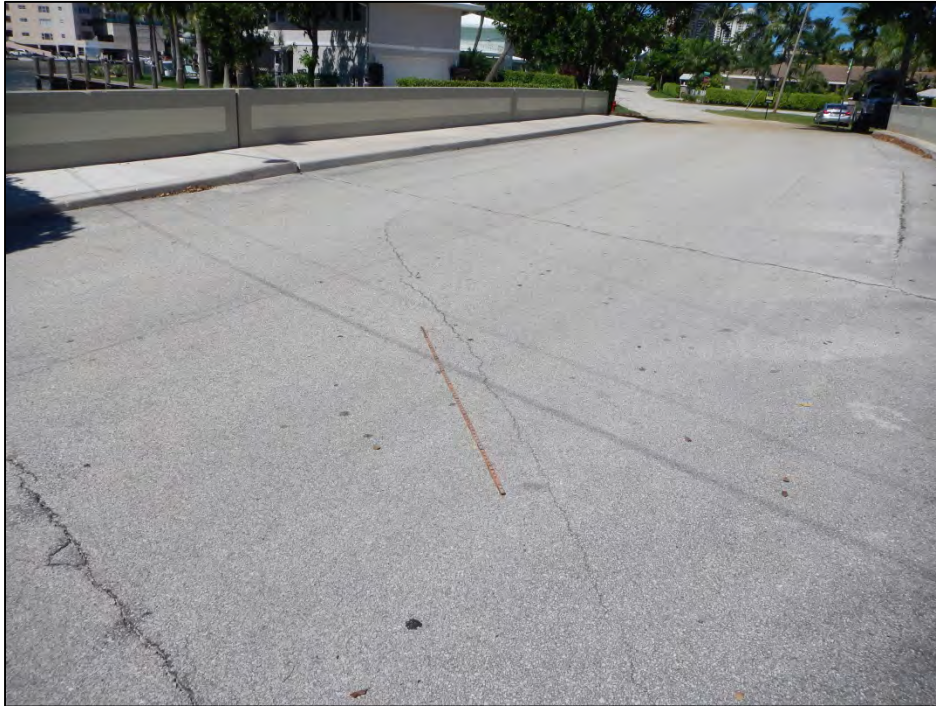
Photo 13 – Diagonal crack in asphalt surfacing over west approach slab.
