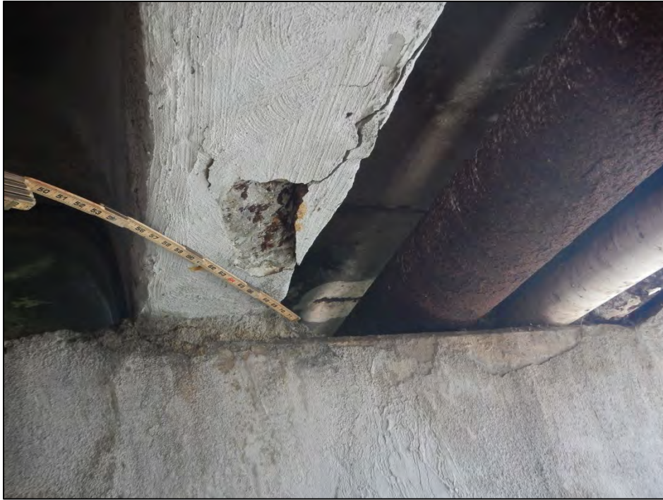
Photo 3 – Spall in Beam 4-I north of Bent 5.
