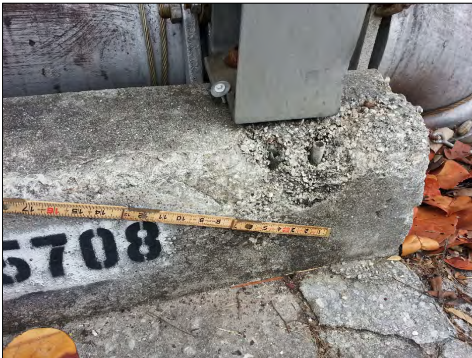
Photo 10 – East railing has a spall with exposed steel at the south end.
