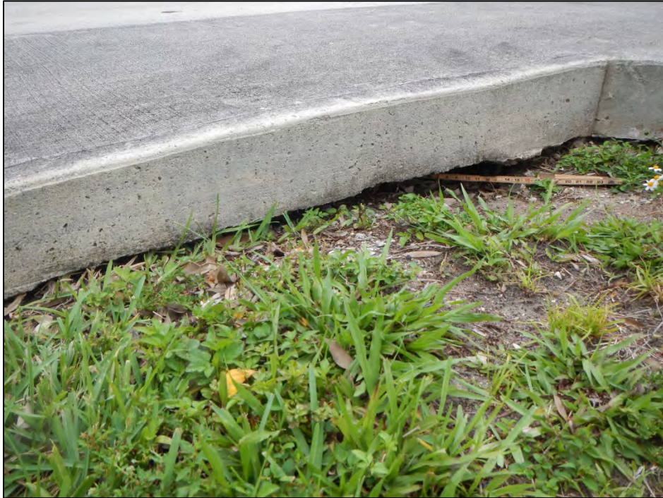
Photo 9 – The northeast approach sidewalk has an area of undermining.
