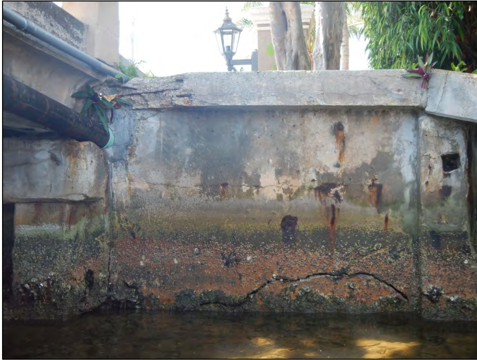
Photo 9 – Spall with exposed reinforcing steel in the southwest retaining wall.
