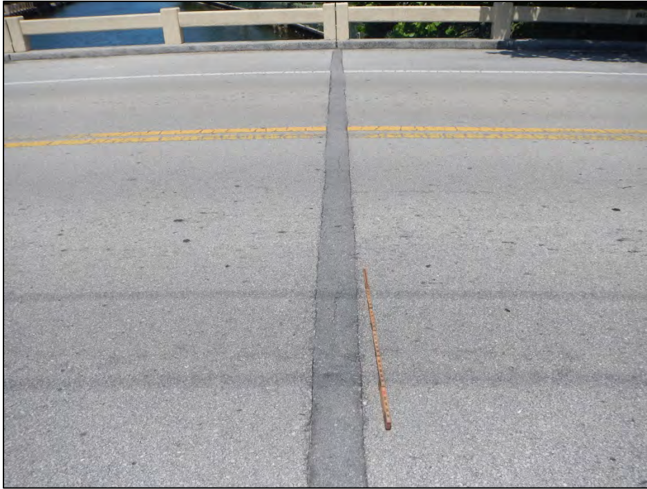
Photo 1 – Repaired asphalt over expansion joint.
