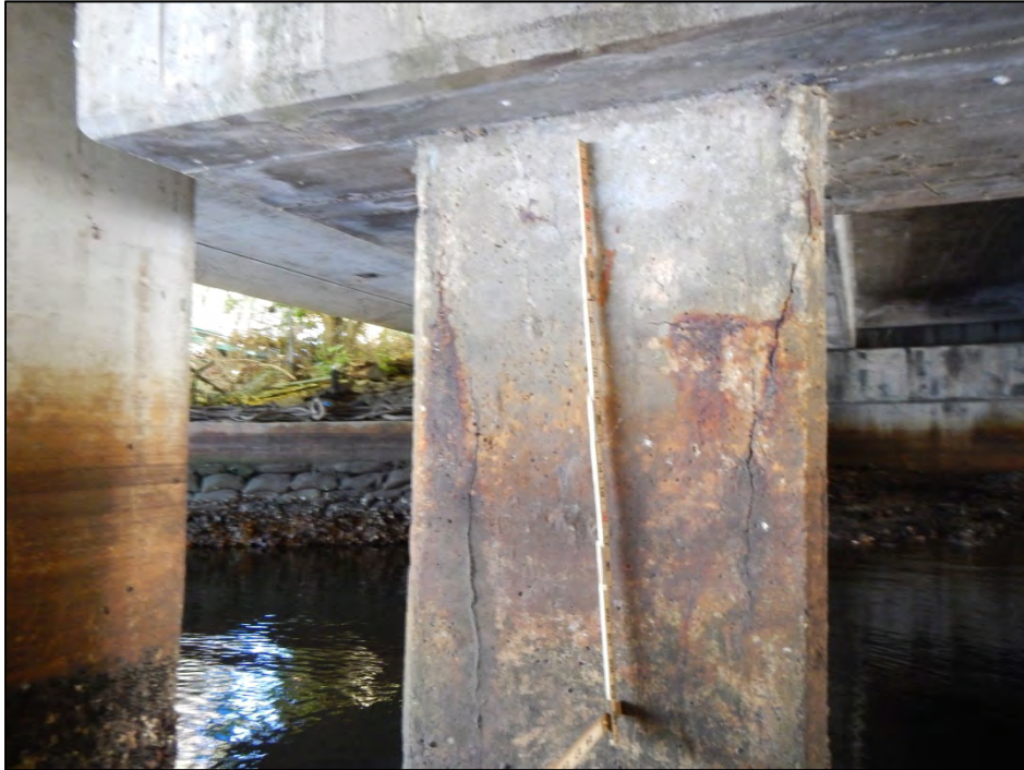
Photo 9 – The north face of Pile 2-7 exhibits vertical cracks.
