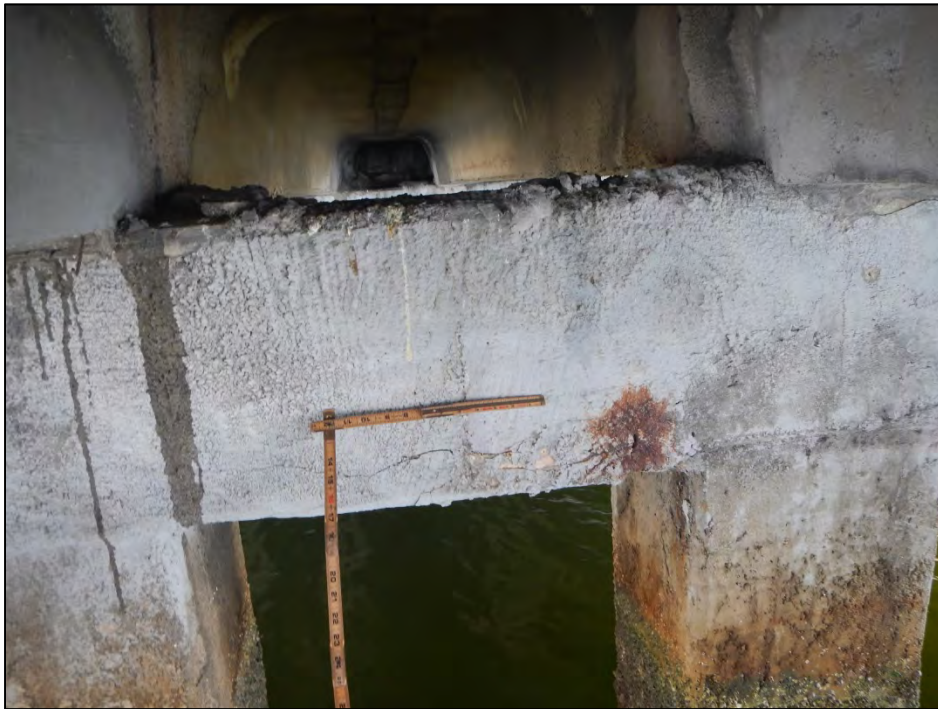
Photo 6 – Delamination in the cap at Bent 8.
