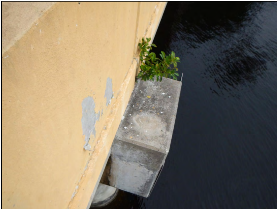
Photo 10 – The east end of Bent 4 exhibits vegetative growth.
