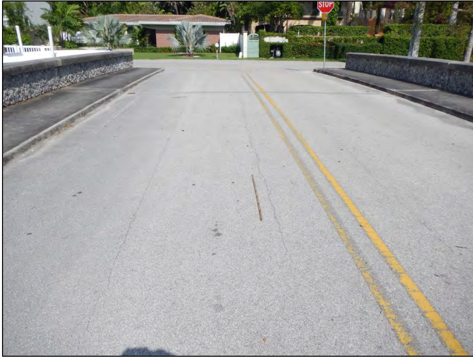
Photo 1 – Longitudinal crack in the asphalt.
