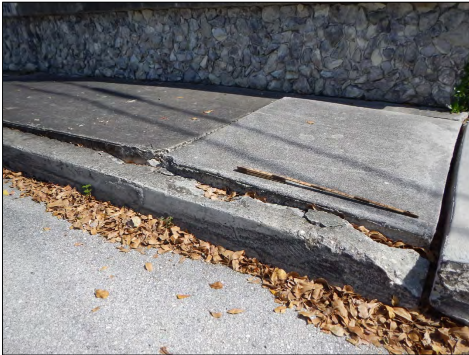
Photo 4 – Spalls and delaminations along the approach slab curb and sidewalk.
