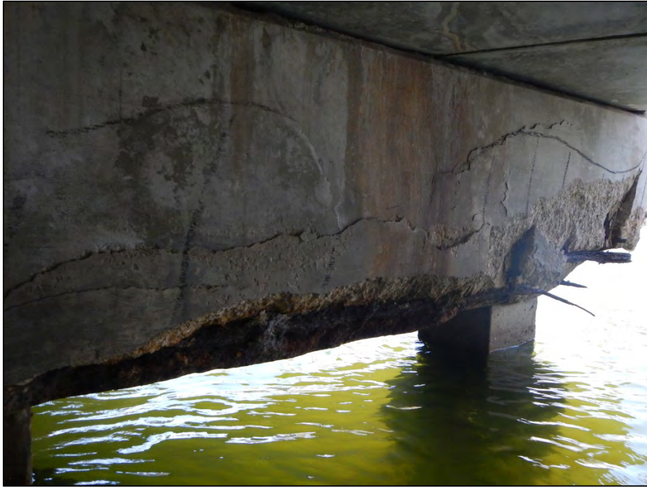
Photo 9 – Spall with exposed rebar at Bent 2 cap.
