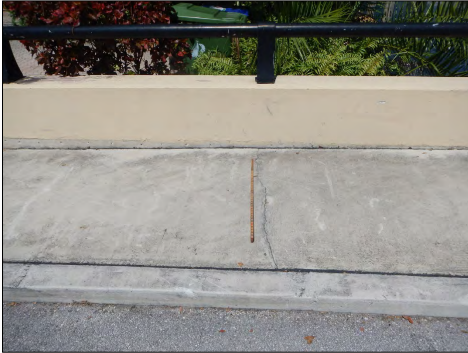
Photo 7 – Transverse crack in southwest approach sidewalk.
