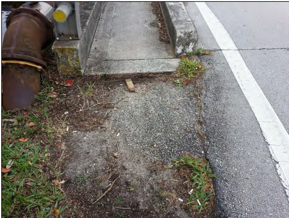
Photo 4 – Southwest corner bridge sidewalk has a drop-off at the end, creating a trip hazard.
