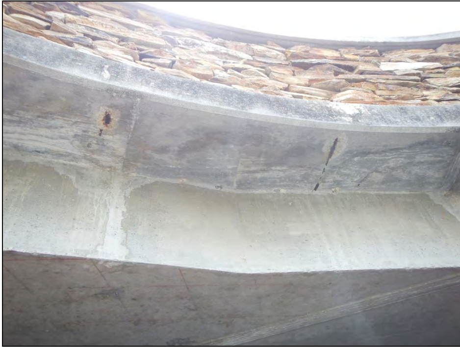
Photo 3 – The left side of Span 3, mid span, exhibits a spall.
