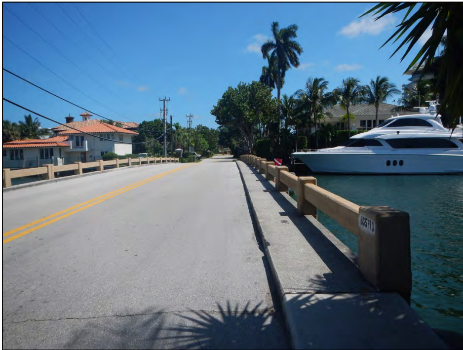
Typical Bridge Railing
