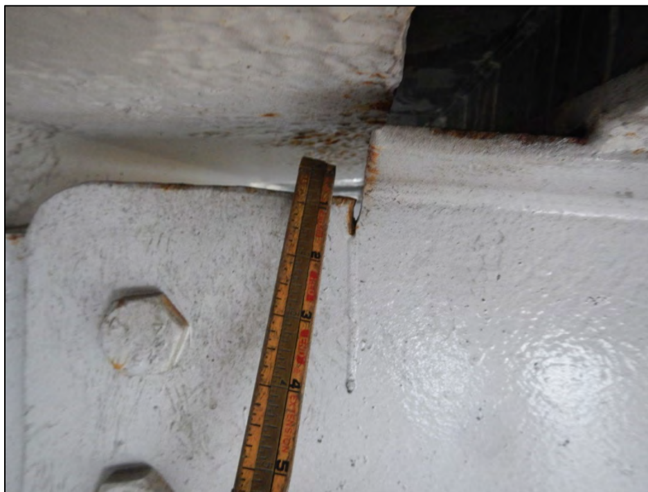
Photo 6 – Gouge within coping of Stringer 5-6.
