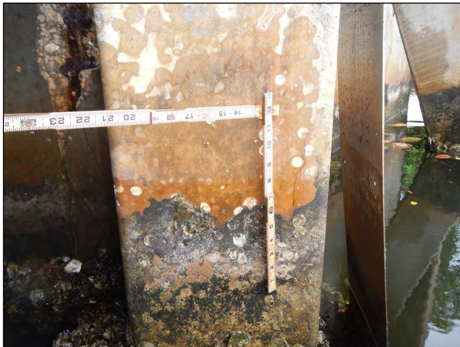
Photo 6 – The southwest corner of Pile 2-8 exhibits a vertical crack.
