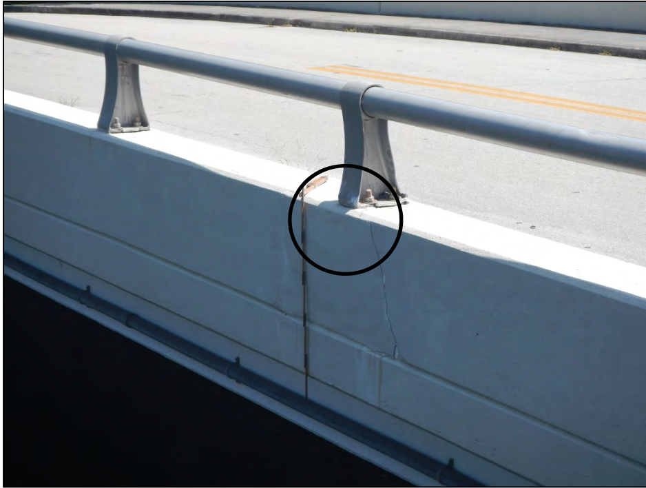
Photo 3 – Delaminated patch in left parapet beneath handrail support.
