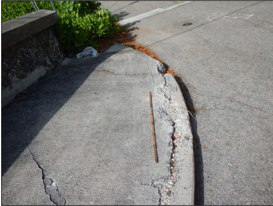
Photo 9 –Spall in the southwest approach curb.
