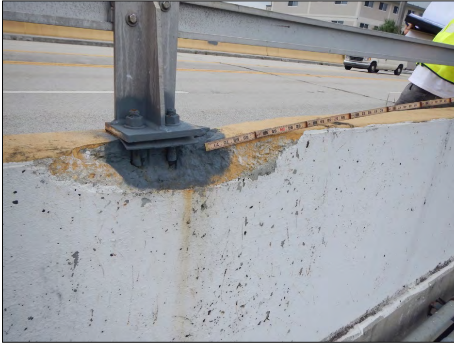
Photo 5 – Spall with exposed steel below Post 3-4L.
