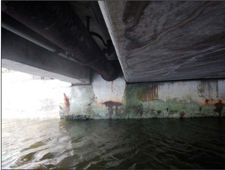
Photo 11 – Spall with exposed corroded rebar at Abutment 4 cap over Pile 4-1.
