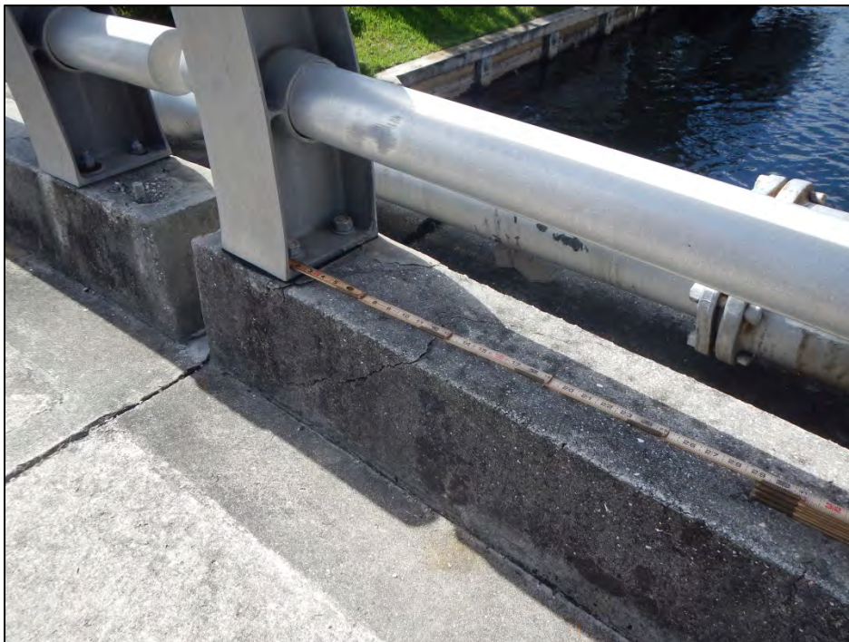
Photo 6 – Delamination at Post 2-3 Right.
