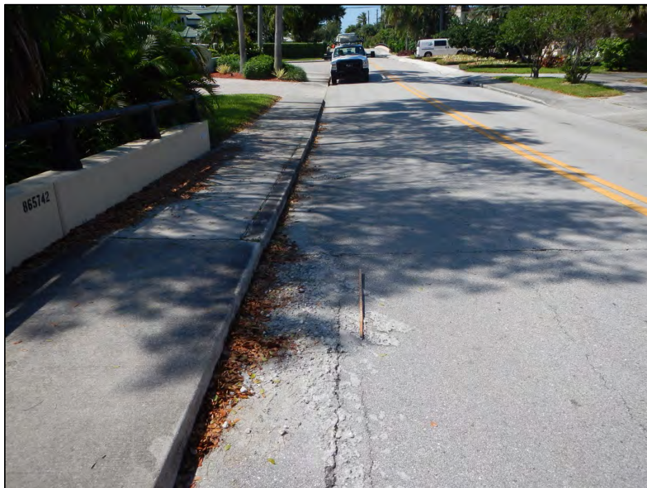
Photo 2 – Spilled concrete adjacent to the right sidewalk at Abutment 1.
