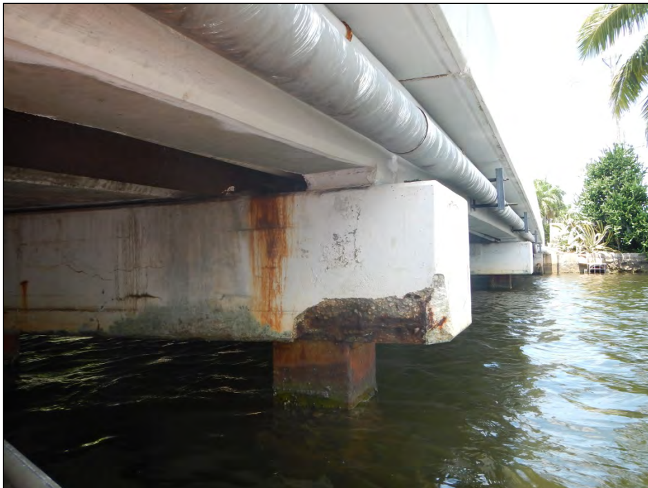
Photo 16 – Spall with exposed corroded rebar at southeast corner of Bent 2 cap.
