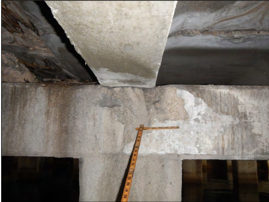
Photo 9 – The north face of Bent 3 cap below Beam 3-3 exhibits a spall.
