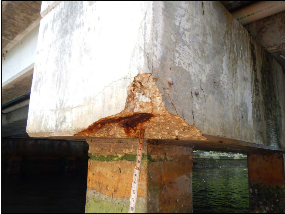
Photo 7 – Spall in the underside of the Bent 3 cap.
