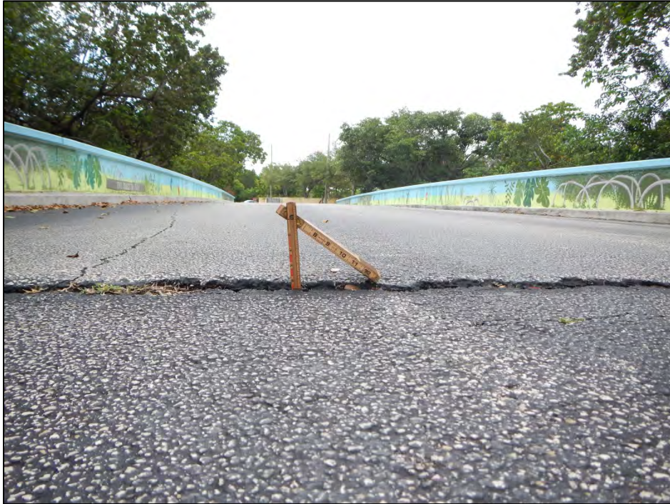
Photo 17 – West approach slab difference in elevation.
