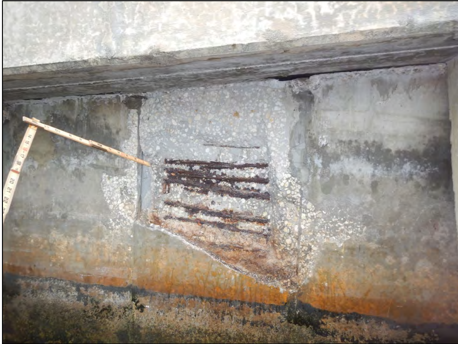
Photo 11 – The south face of the southwest retaining wall exhibits a spall/delamination.
