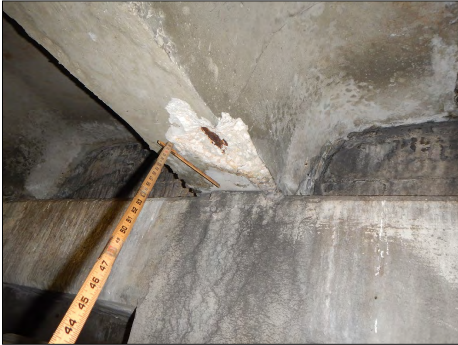
Photo 5 – Beam I-5 right exhibits a spall/delamination with exposed steel.
