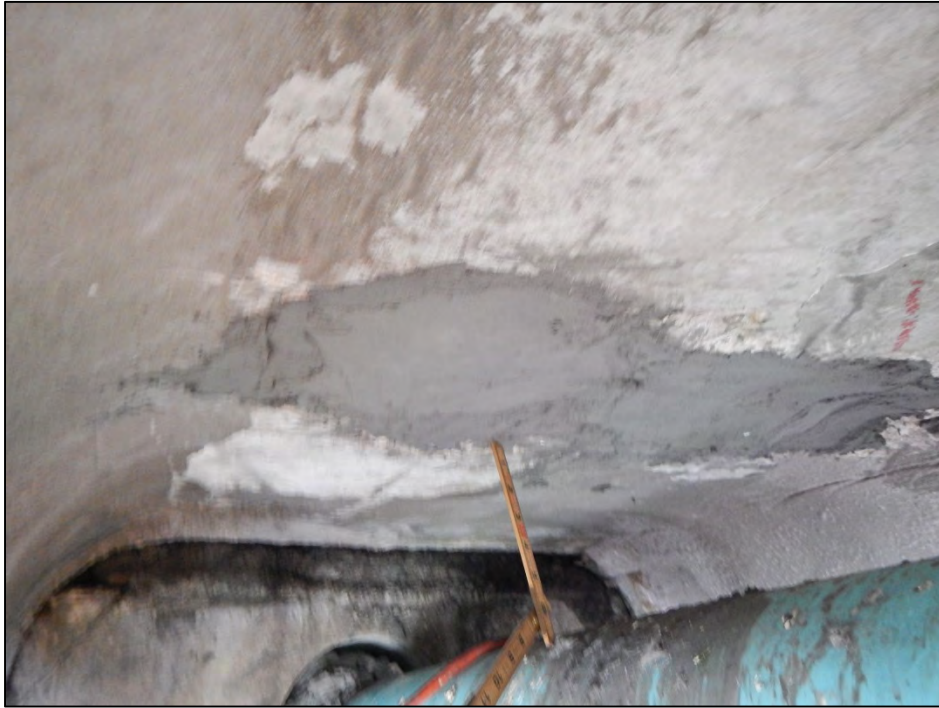
Photo 3 – Typical repair patch on bottom flange of T-beams.
