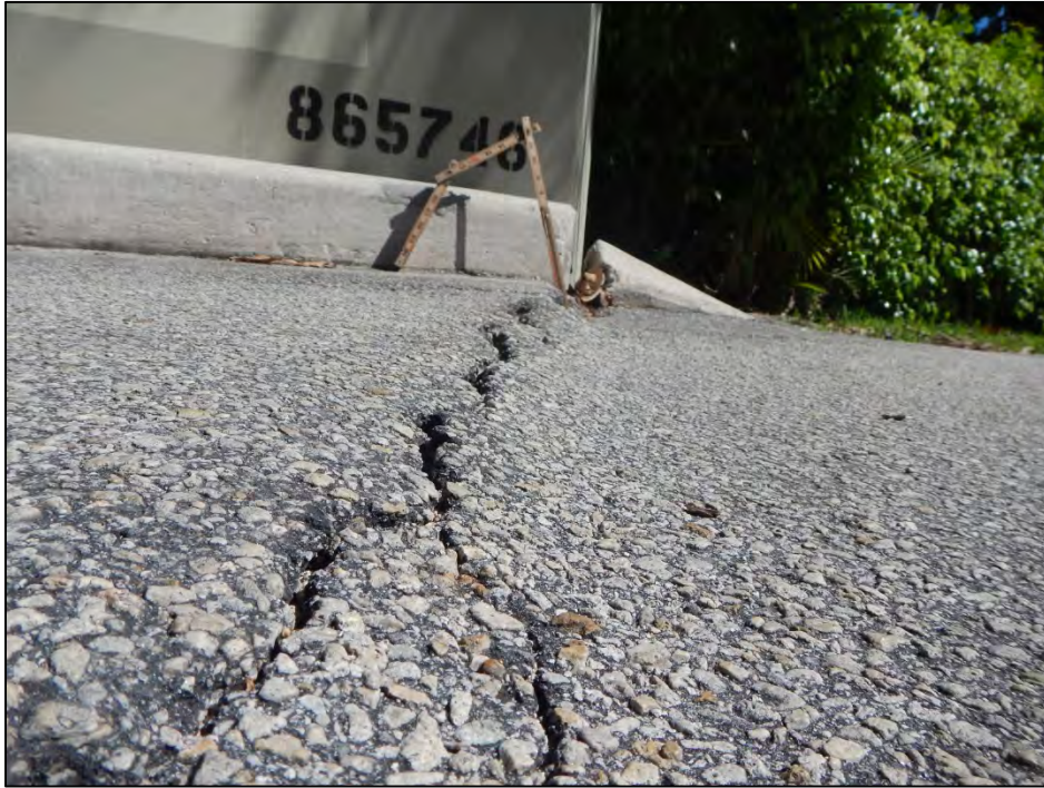
Photo 9 – Typical elevation differential between approach roadway and approach slab.
