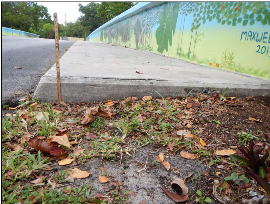
Photo 18 – Southwest approach sidewalk exhibits a difference in elevation.
