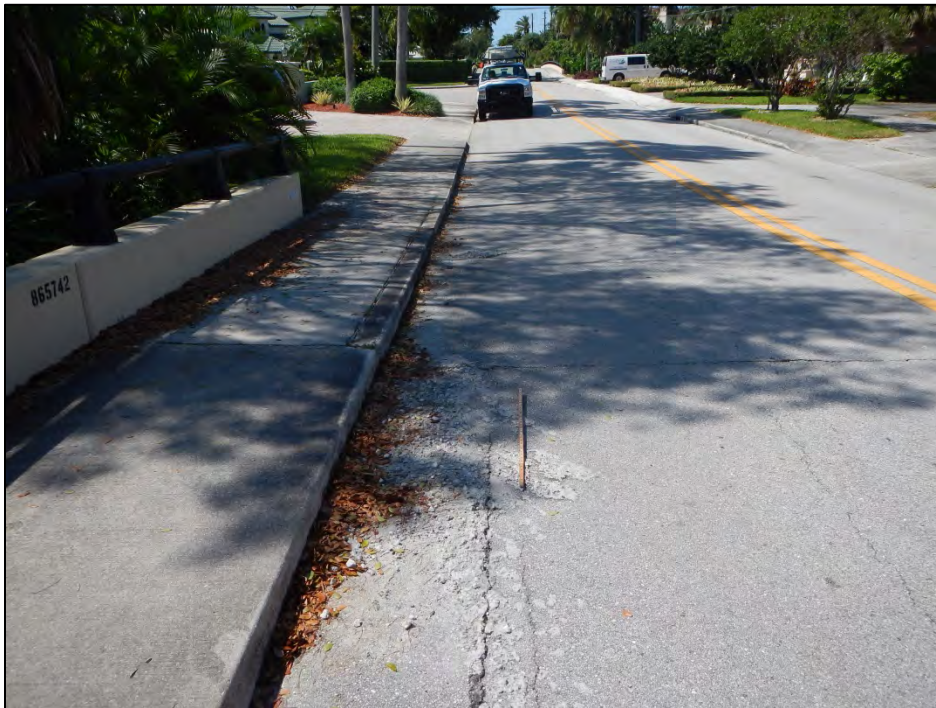
Photo 12 – Spilled concrete on the south approach at the east sidewalk.
