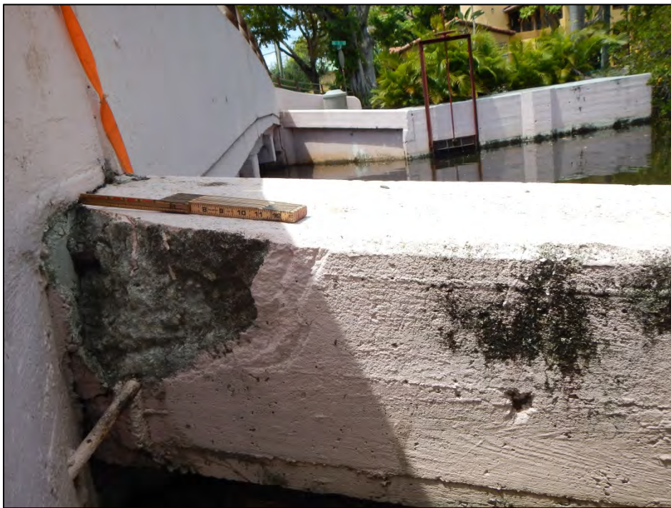
Photo 10 – The southeast retaining wall cap exhibits a spall at Abutment I.
