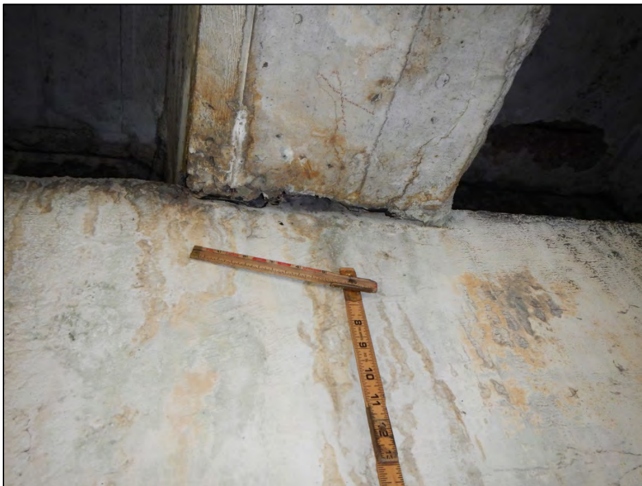
Photo 12 – Beam 1-5 over Abutment 2 exhibits a void.
