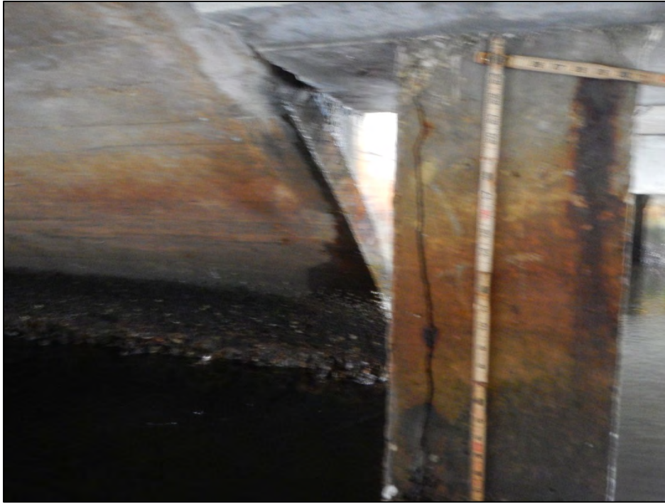
Photo 15 – The north face of the northeast corner of Pile 2-3 exhibits a vertical crack with corrosion bleed-out.
