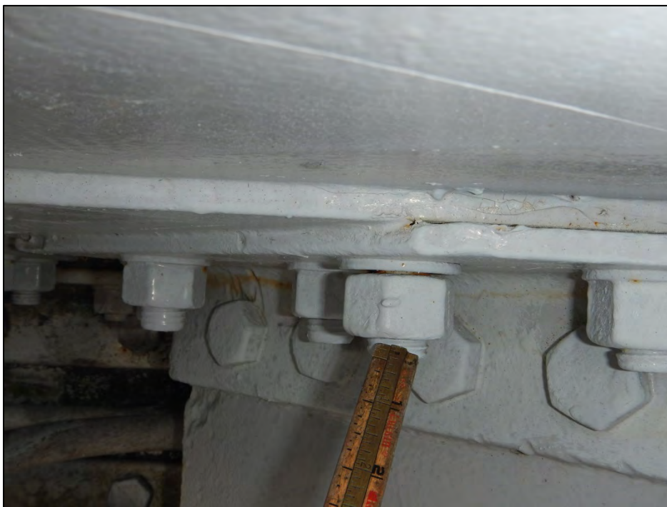
Photo 12 – Loose connection bolt at the east vertical connection to L6.
