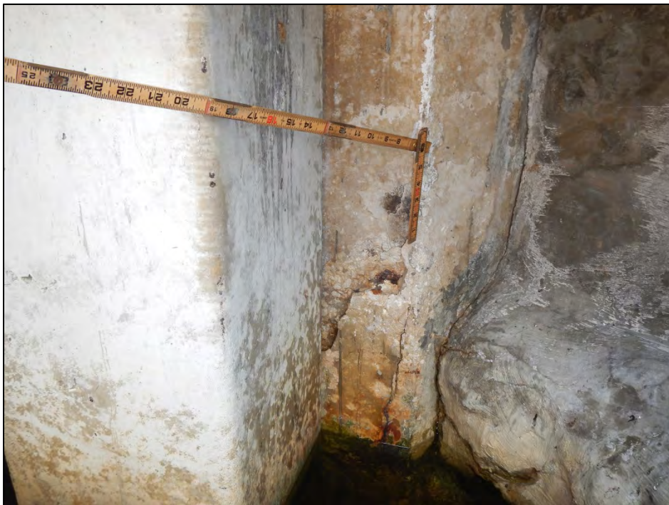
Photo 8 – The south end of the End Bent 4 retaining wall exhibits a spall.
