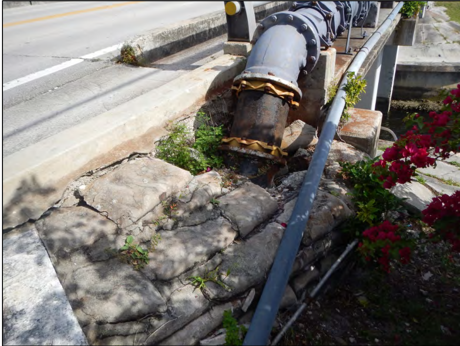
Photo 17 – The southeast corner exhibits a washout area.
