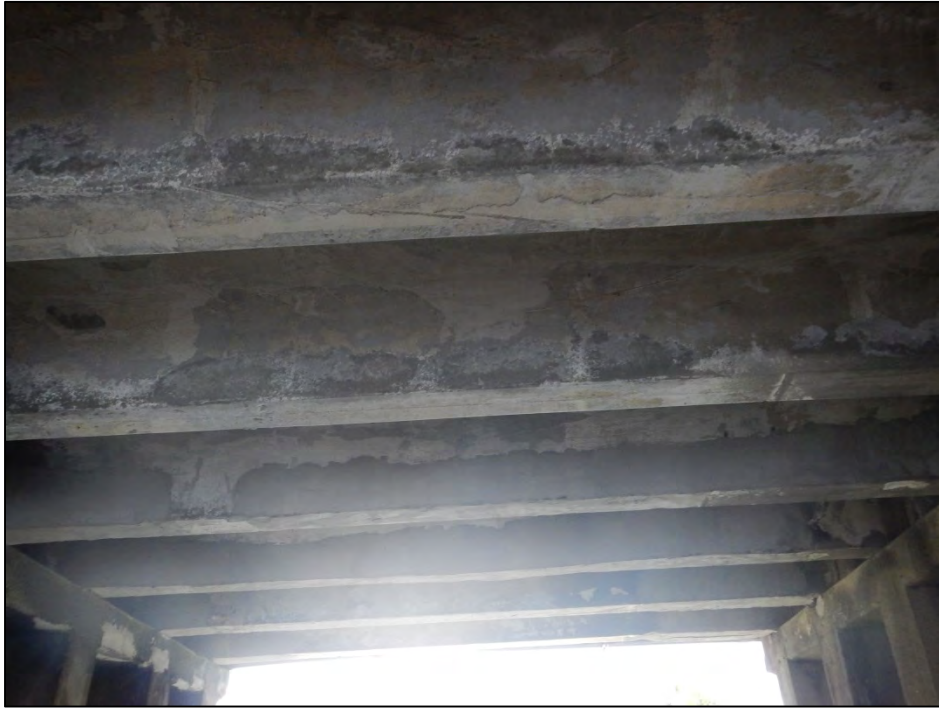
Photo 5 – Typical cracks in previously repaired areas on the double T-Beams
