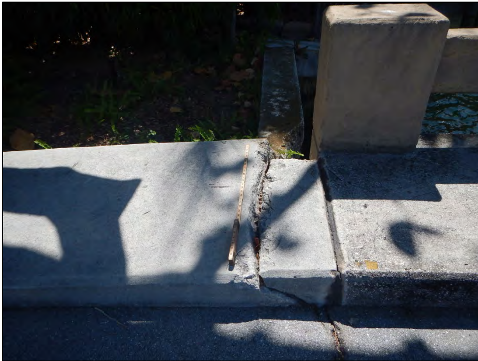
Photo 8 – Spall with exposed reinforcing steel in the Approach Slab sidewalk.
