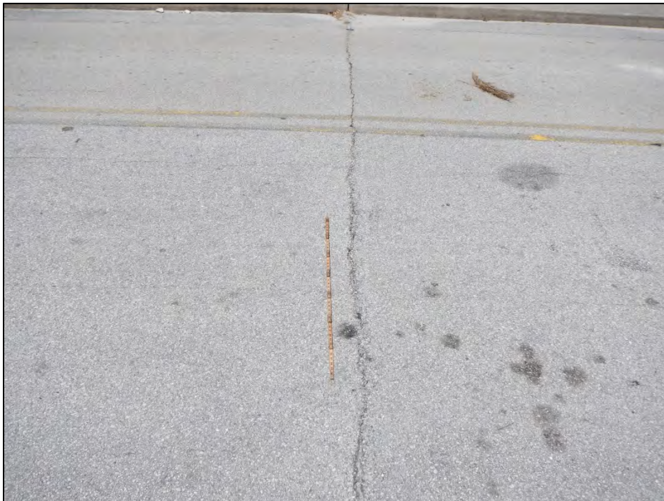
Photo 2 – Crack in the asphalt over the joints.
