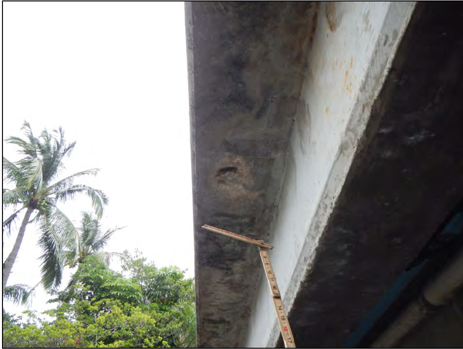
Photo 5 – Spall in the underside of the left sidewalk in Span 2.
