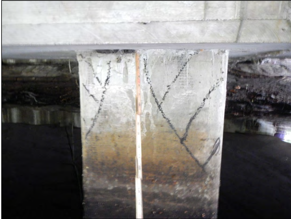
Photo 11 – Pile 5-5 exhibits delaminations in the west face.
