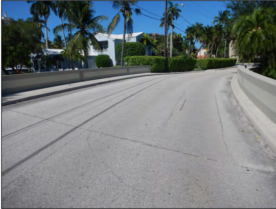
Photo 1 – Cracks in asphalt overlay.
