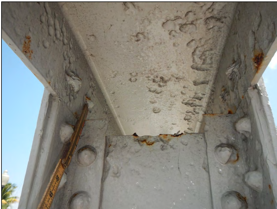
Photo 8 – Typical painted section loss and pitting in upper chords. Note section loss on rivets.
