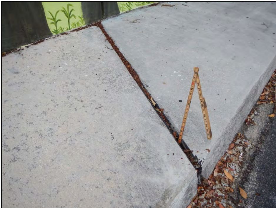
Photo 4 – End Bent 6 sidewalk right side joint deterioration.
