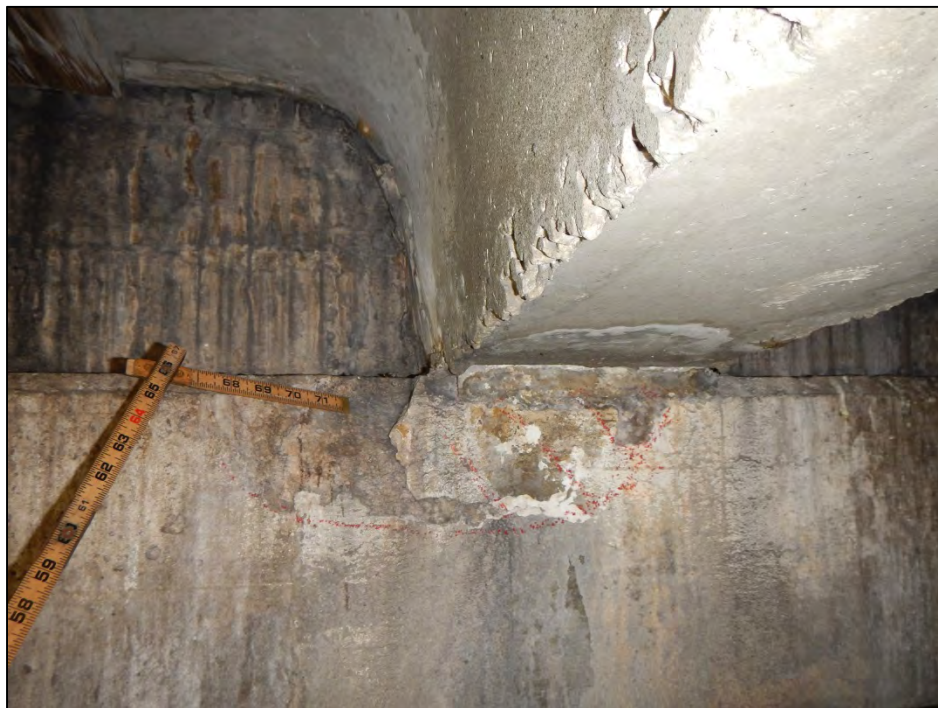
Photo 8 – Abutment 1 cap below Beam 5-I exhibits a spall/delamination.
