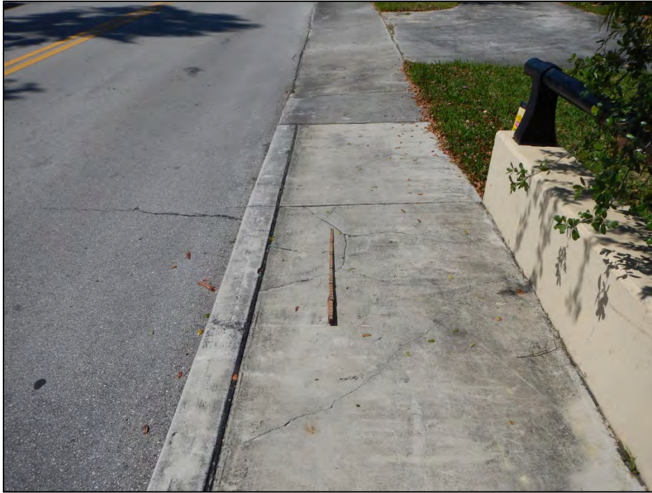
Photo 11 – Cracks in southwest approach sidewalk.
