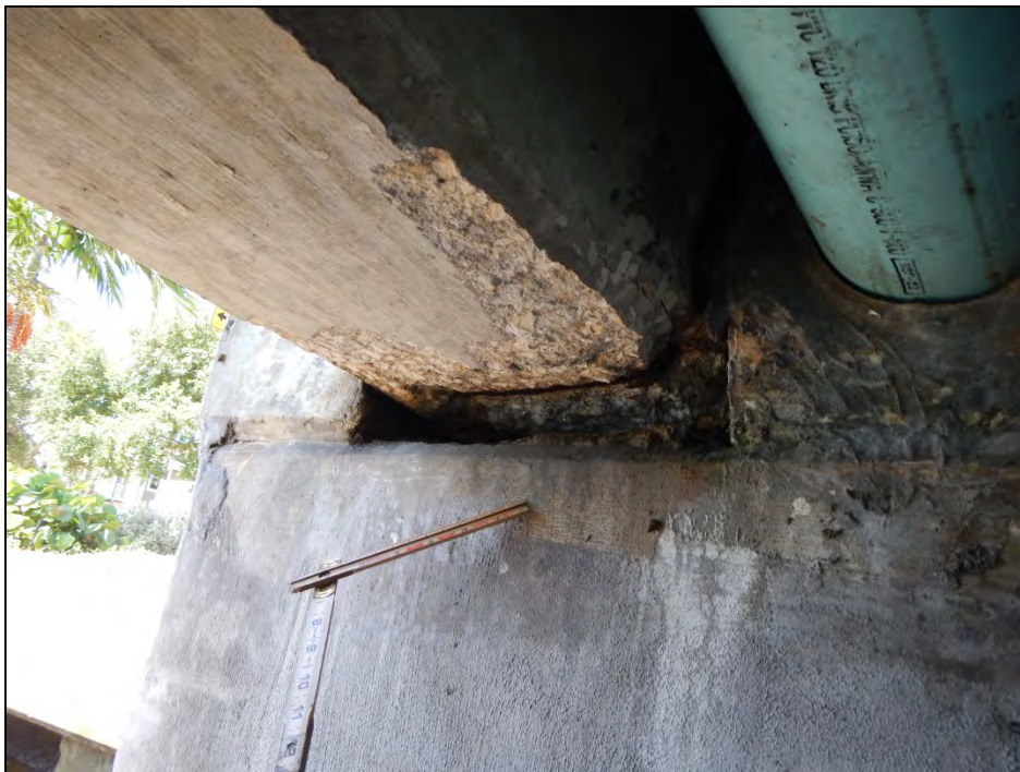
Photo 3 – Spall in Beam I-2 over Abutment I.
