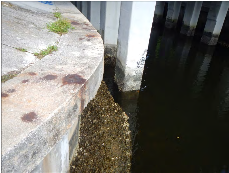
Photo 18 – The End Bent I bulkhead cap exhibits cracking.
