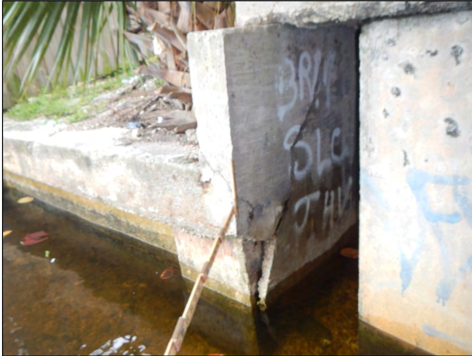
Photo 15 – Crack at the west face of the southeast corner retaining wall.
