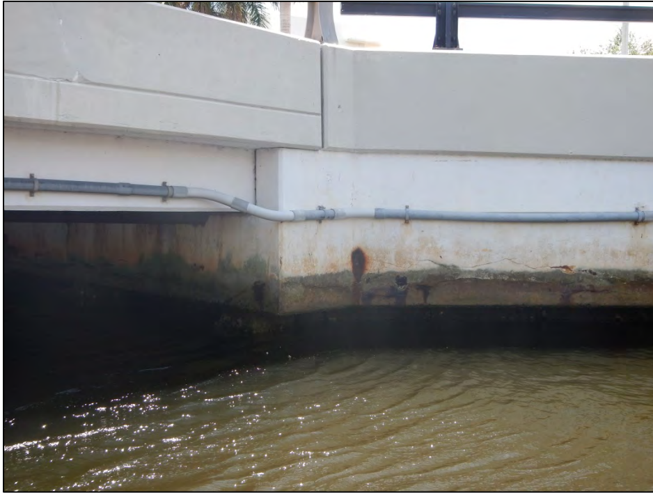
Photo 15 – Delamination at the southwest retaining wall cap.
