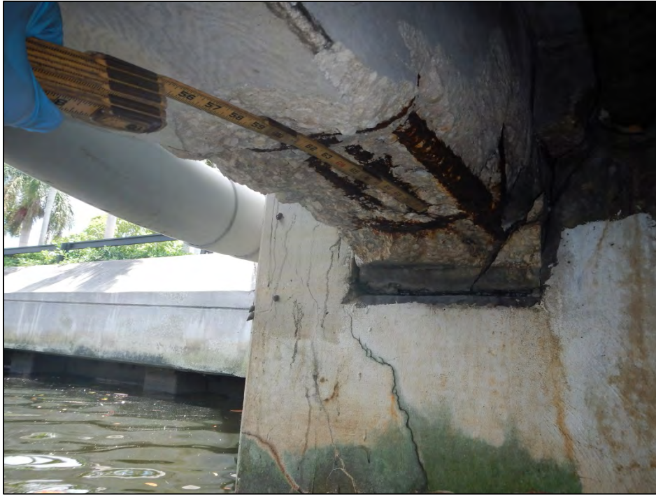
Photo 9 – Spalls with exposed corroded rebar in Beam 1-2.
