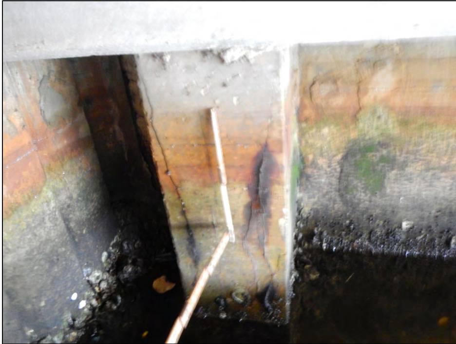
Photo 13 – The north face of Pile 1-3 exhibits vertical cracks with corrosion bleed-out.
