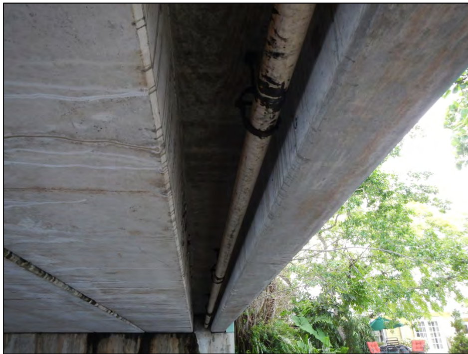
Concrete Slab Underside and Concrete T-beam. Note Utility Pipe in the Bay.
