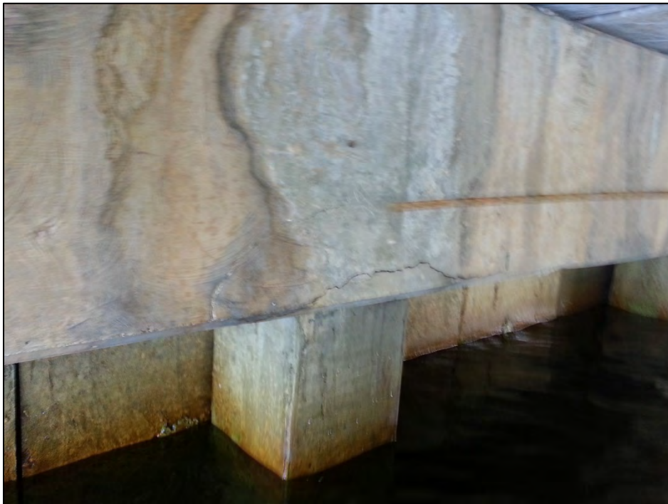
Photo 6 – Delamination in Abutment I cap over Pile I-4.
