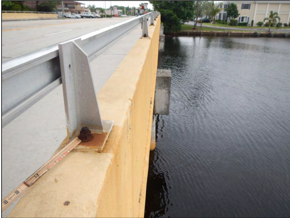
Photo 3 – The aluminum railing Post I-3 right exhibits bolt corrosion.
