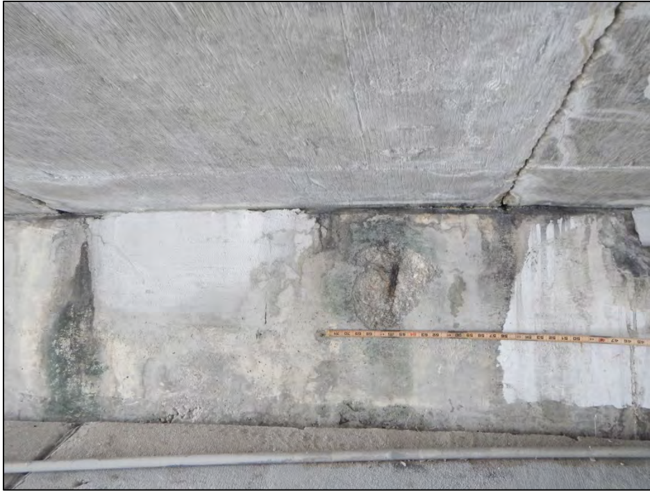
Photo 7 – Abutment 1 cap has a spall under Slab Unit 1-7.
