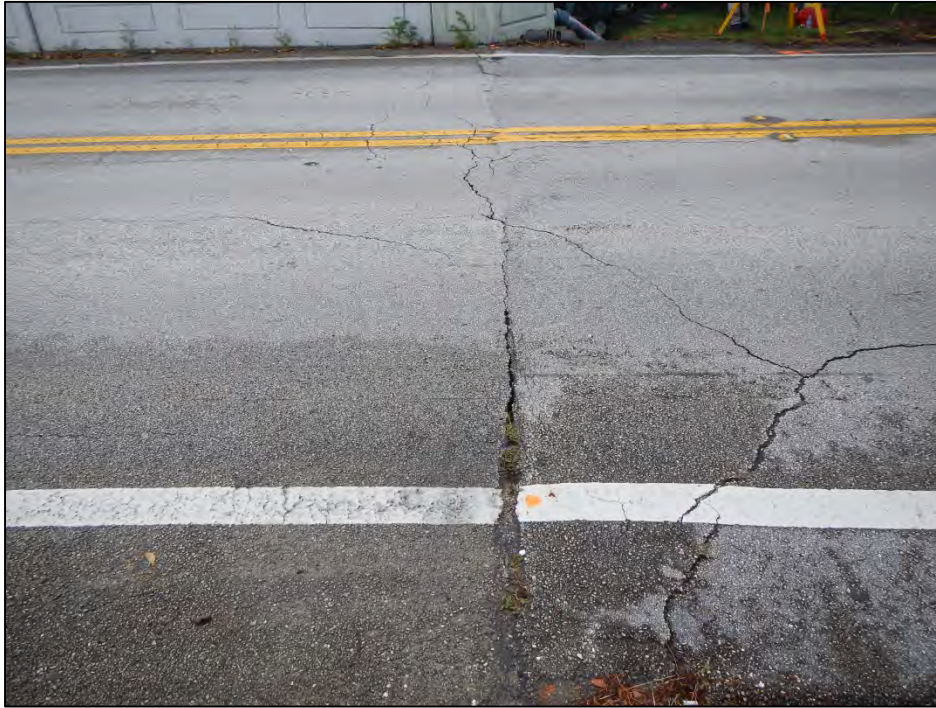
Photo 1 – End Bent 1 joint seal transverse crack.
