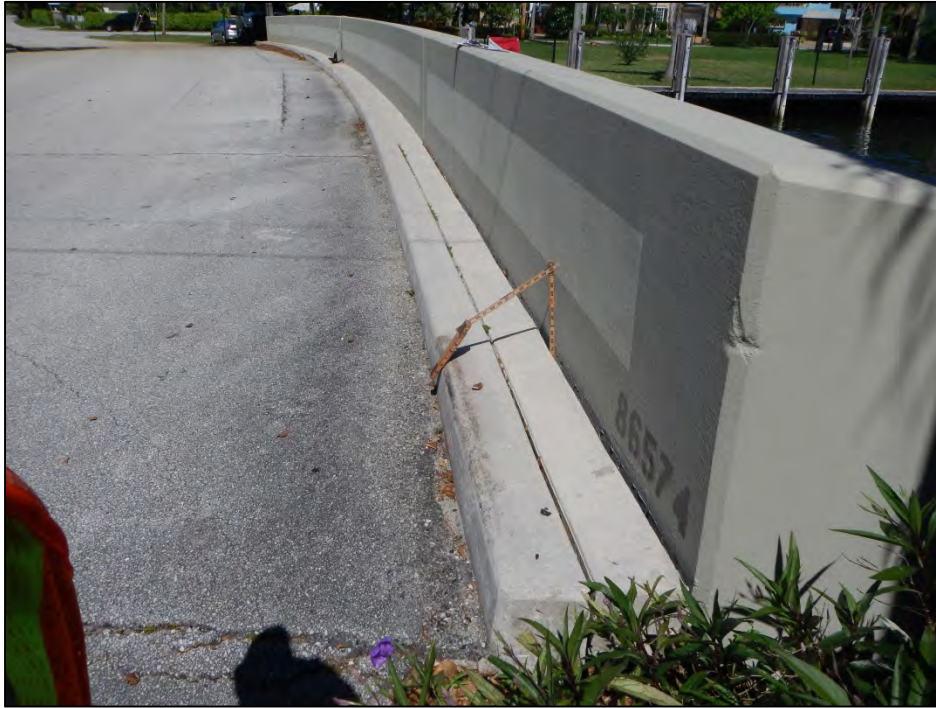
Photo 17 – Gap between wingwall and approach curb.
