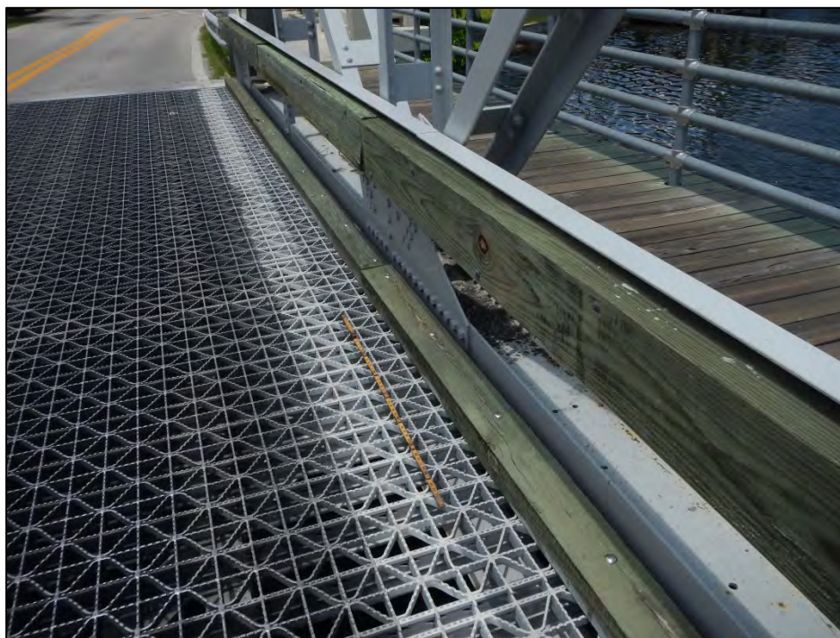
Photo 1 – General location of cracked weld between Stringer 8-8 and grid deck.
