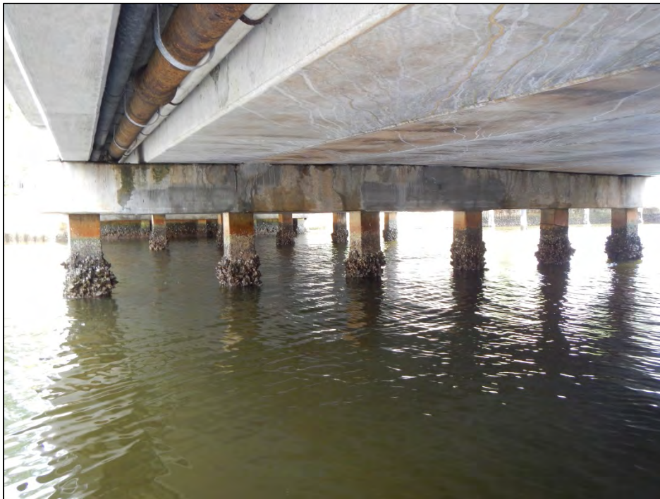
Span Underside and Intermediate Bent. Note Utility Pipe.
