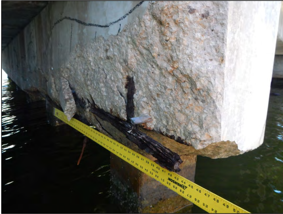
Photo 11 – Spall with exposed rebar at Bent 2 cap.
