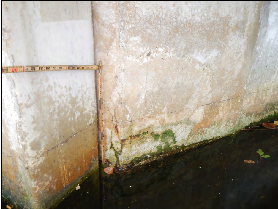
Photo 9 – The northwest retaining wall exhibits a delamination.
