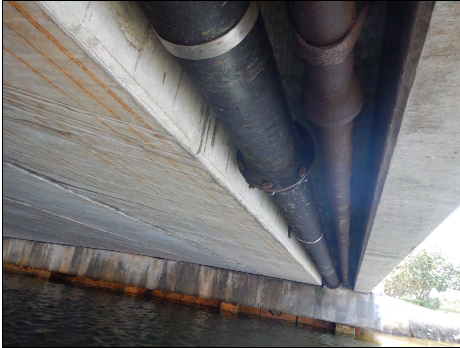
Utilities mounted to deck underside
