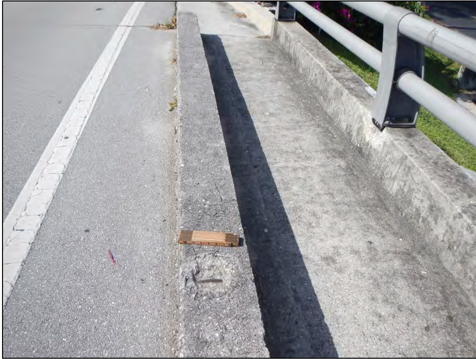
Photo 3 – The left curb over Span I has a spall with exposed steel.
