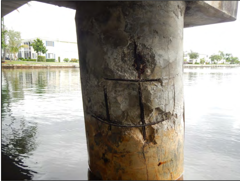
Photo 13 – Pile 3-12 exhibits spalls and delaminations.
