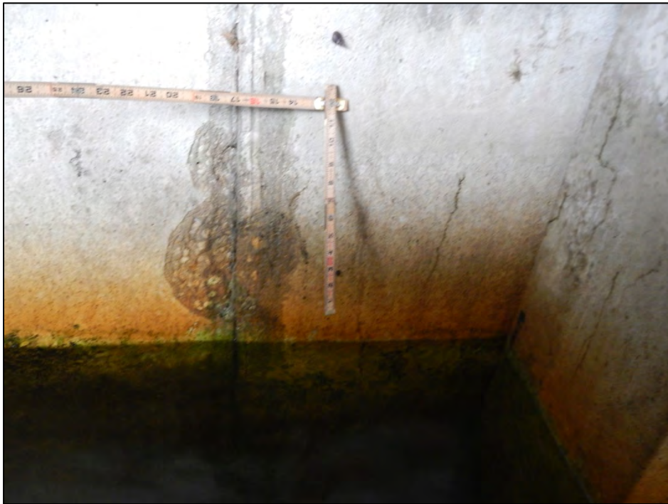
Photo 6 – Spall in the sheet piles at Abutment I retaining wall.
