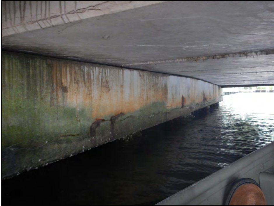
Photo 9 – Delamination at Abutment 1 cap.
