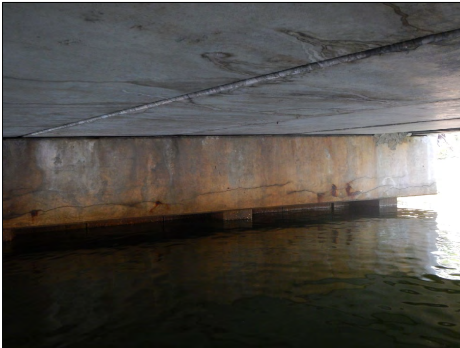
Photo 2 – Delamination in Abutment 1 cap.
