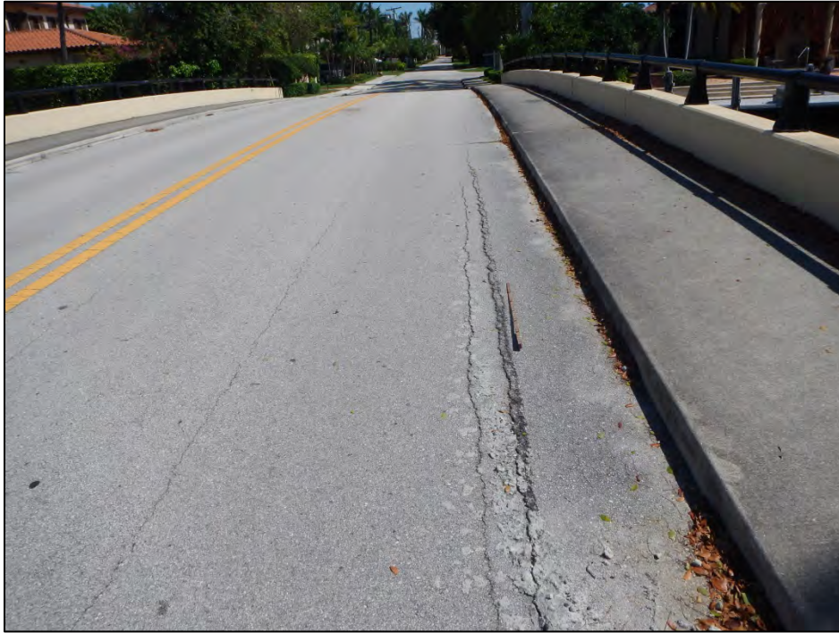
Photo 1 – Longitudinal cracks in asphalt overlay over slab unit joints.
