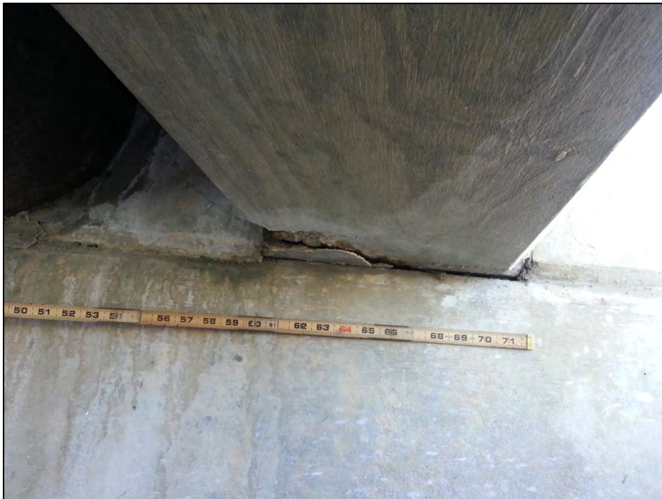
Photo 6 – Spall in Beam 3-2 at Abutment 4.
