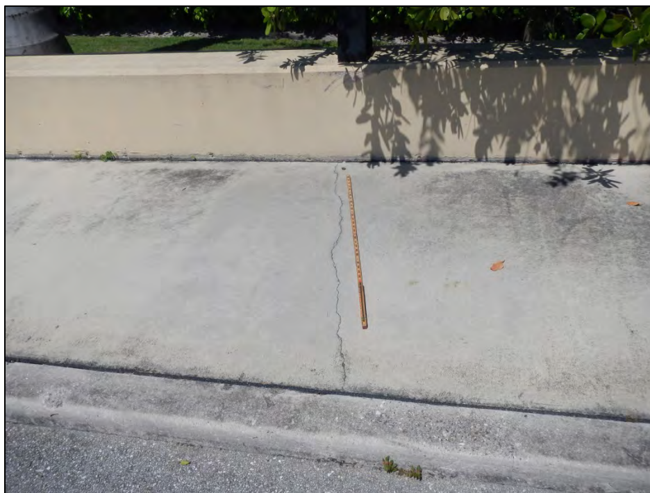
Photo 8 – Crack in southwest approach sidewalk.
