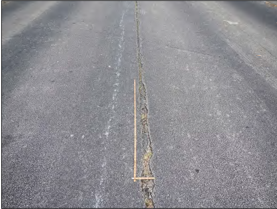
Photo 3 – Centerline longitudinal crack.
