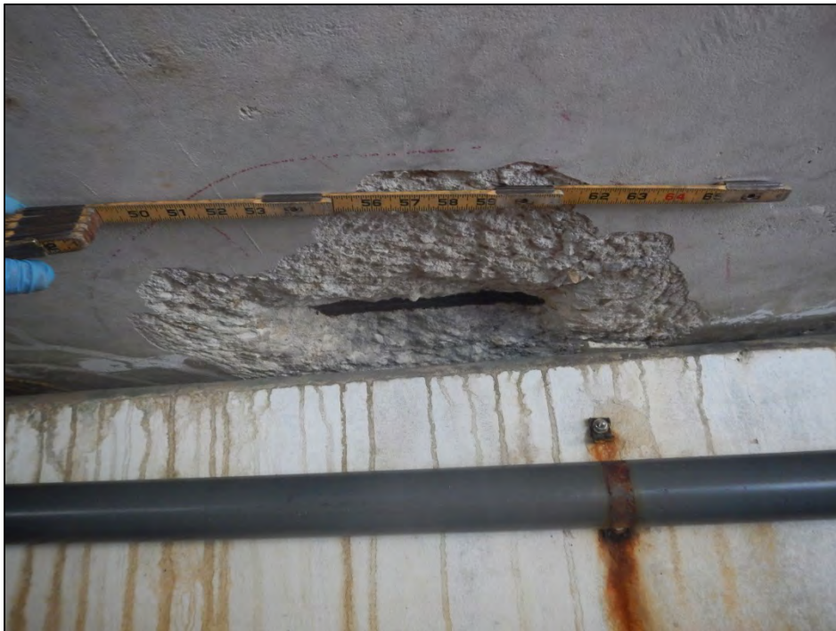
Photo 6 – Spall/Delamination with exposed prestressing strand in Slab Unit 3-6.
