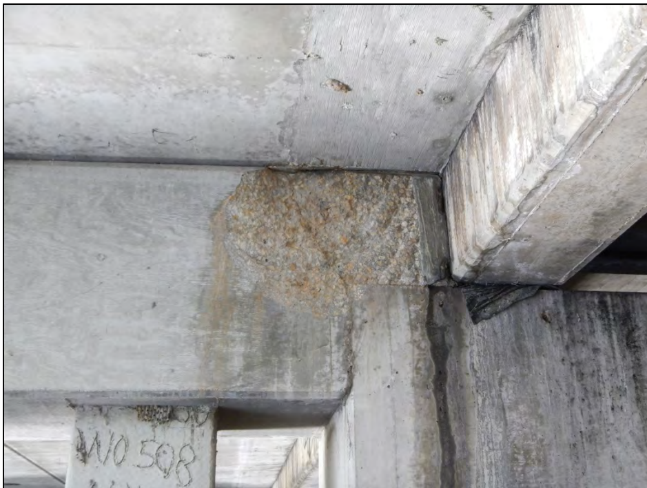
Photo 14 – The south face of Bent 2 cap exhibits a spall.
