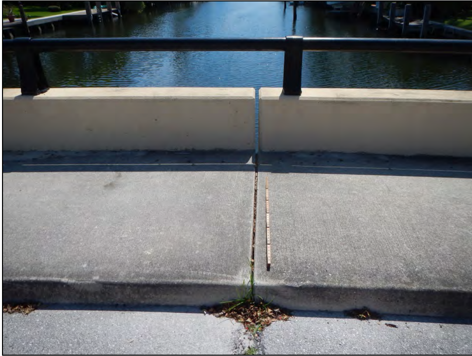
Photo 5 – Deteriorated sidewalk joint sealant; joint filled with dirt and debris.
