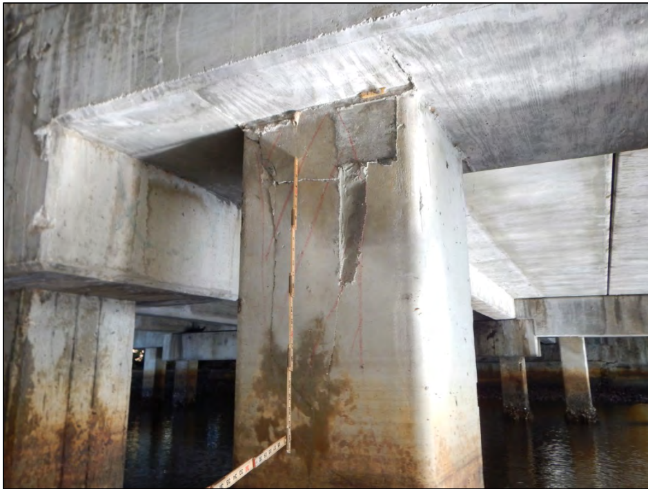
Photo 10 – Cracks and delaminations in the north face of Pile 3-3.
