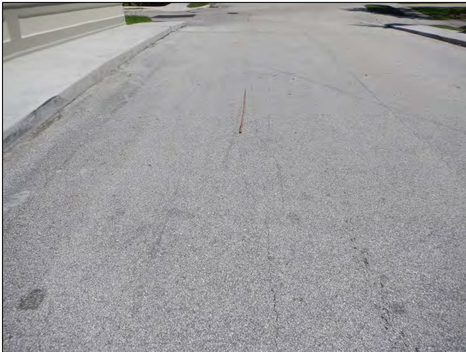
Photo 2 – Longitudinal cracks in asphalt surfacing.
