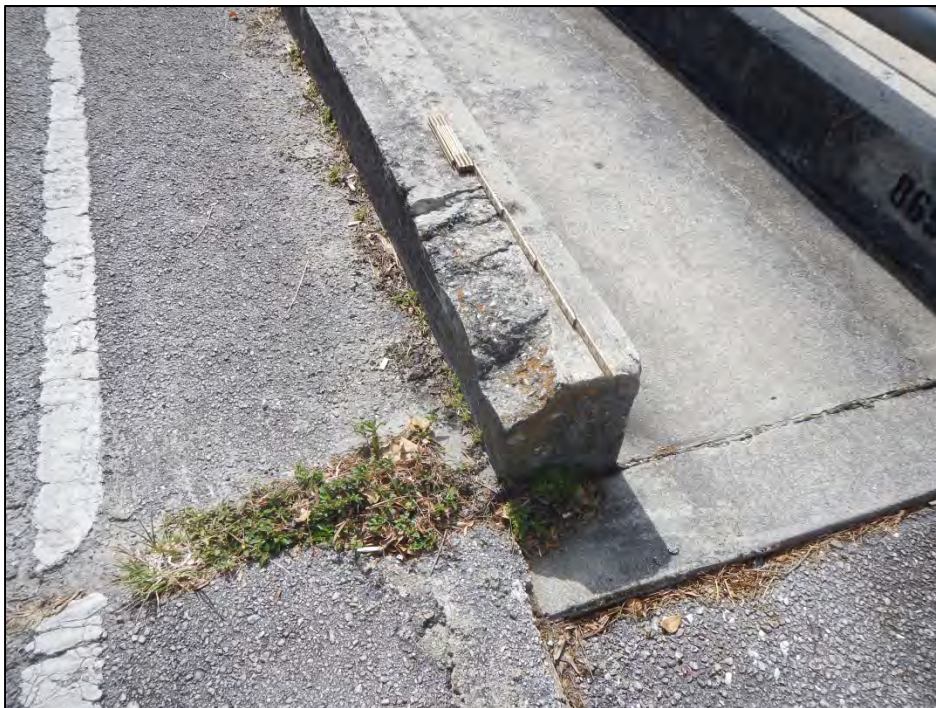
Photo 4 – The south curb over End Bent 1 exhibits a spall.
