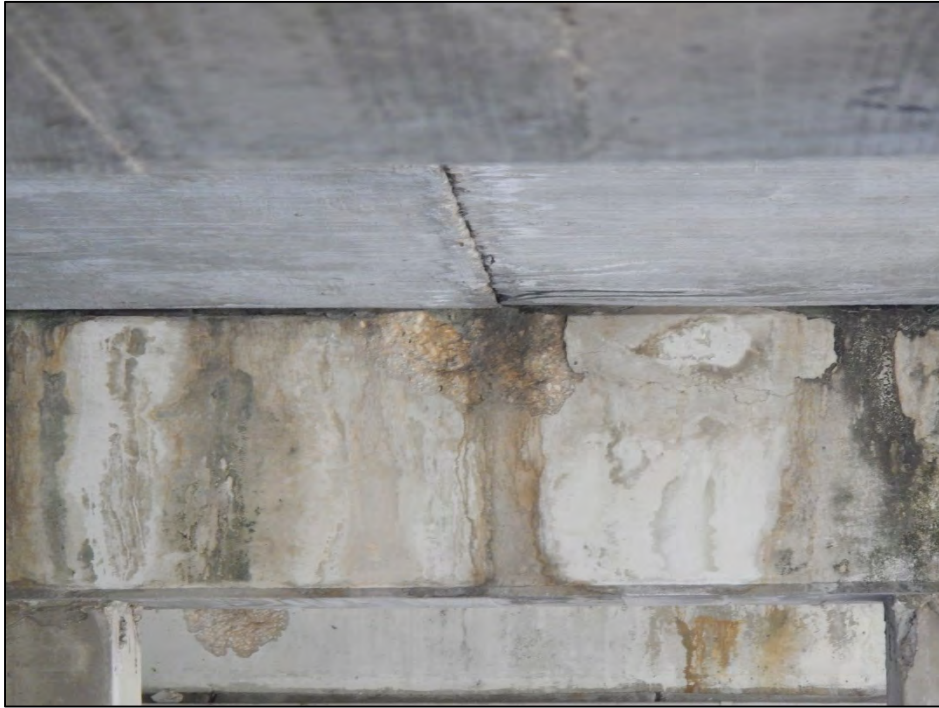
Photo 17 – Bent 3 cap exhibits a spall between Slab Units 2-8 and 2-9.
