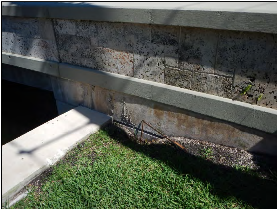
Photo 18 – Fill void at northwest wingwall.
