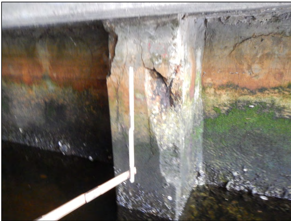
Photo 14 – The northwest corner of Pile 1-2 exhibits spalls and delaminations.
