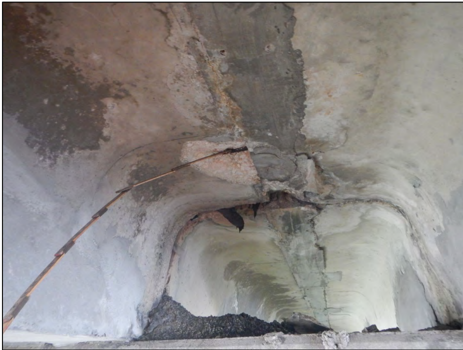
Photo 4 – Typical spall with exposed rebar and delamination in the double T-beams.
