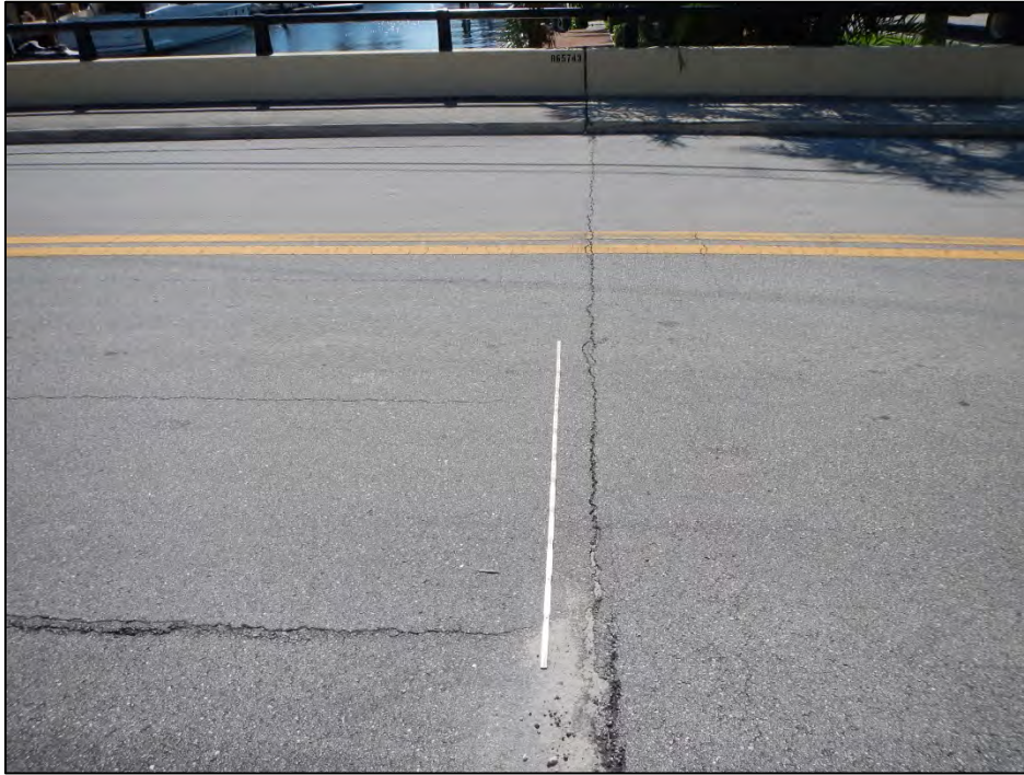
Photo 1 – Cracks in asphalt overlay at slab unit joints and expansion joints.
