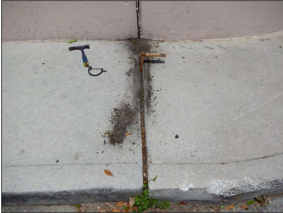
Photo 3 – The right sidewalk joint seal over End Bent 1 is deteriorated.
