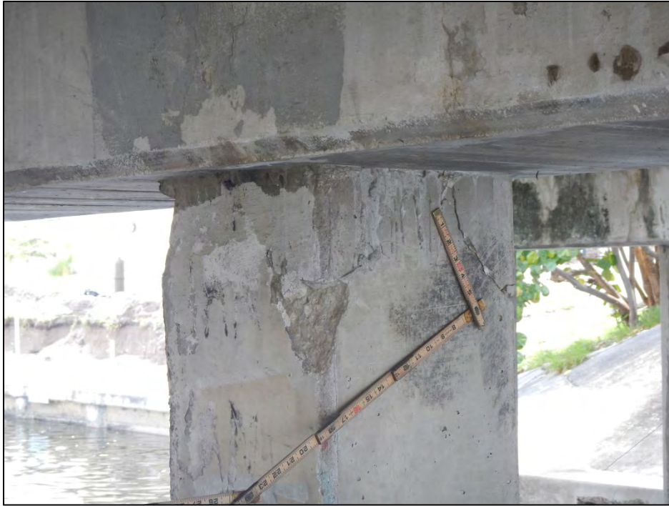
Photo 15 – Pile 2-4 adjacent to the cap exhibits spalls/delaminations.
