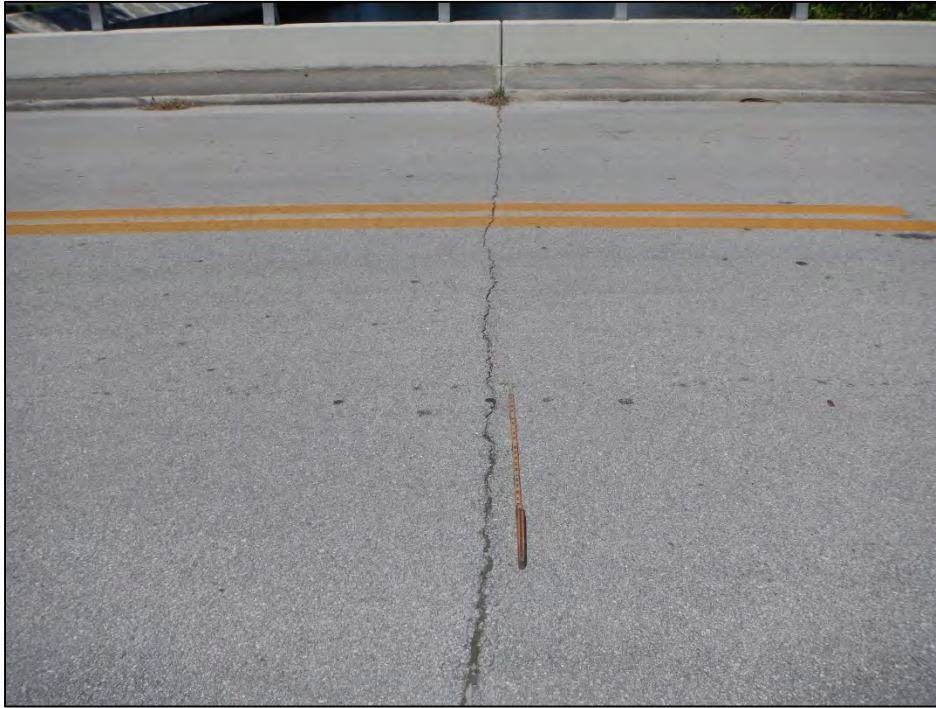
Photo 1 – Transverse cracks in asphalt overlay.
