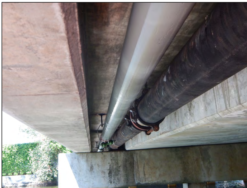
Utilities mounted to deck underside
