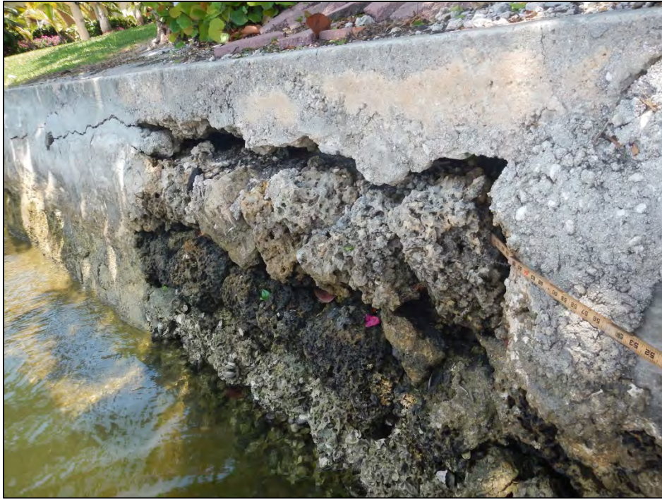
Photo 9 – Northeast wingwall void.
