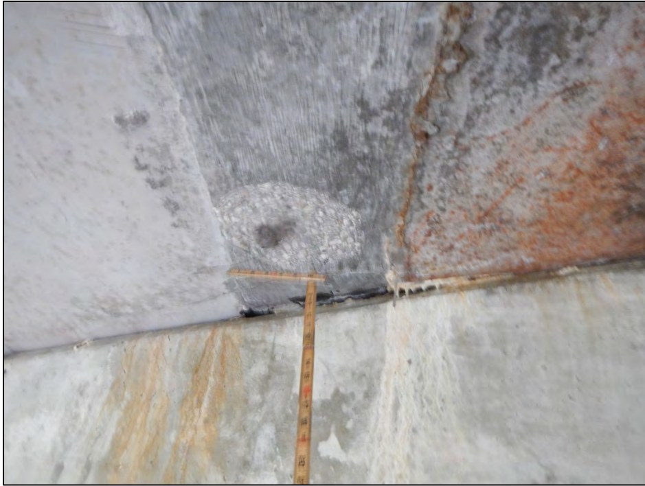
Photo 7 – Slab 4-I joint spall.
