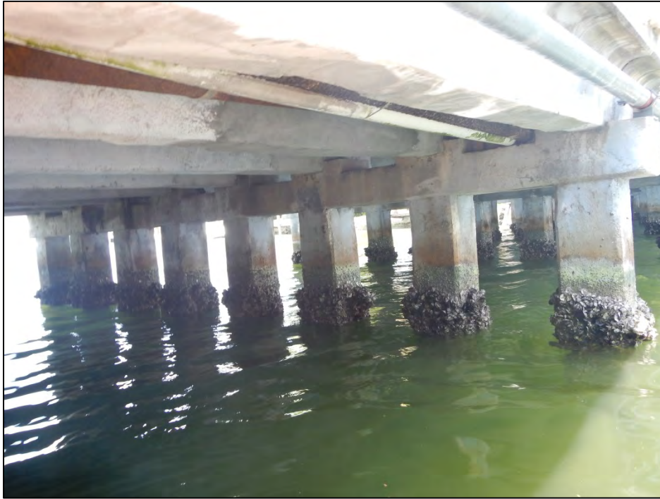
Photo 5 – Delaminations and cracks in the cap at Bent 2.
