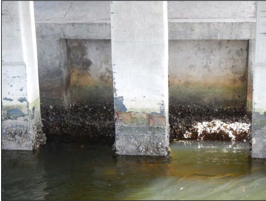
Photo 11 – The south face of Pile 3-4 exhibits a spall with exposed steel.
