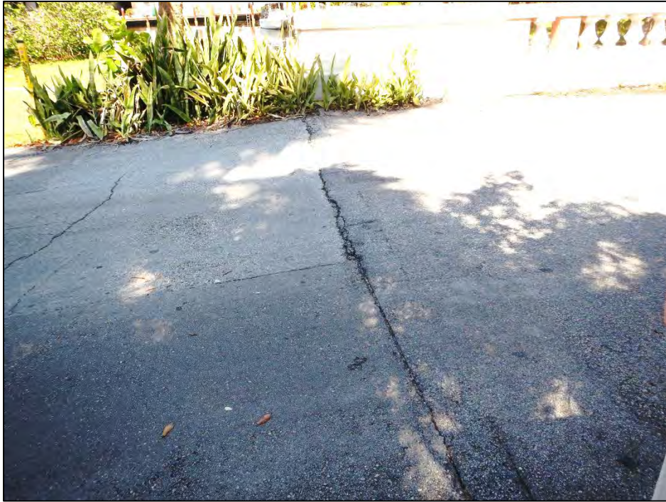
Photo 3 – Condition at south transition from approach to bridge.
