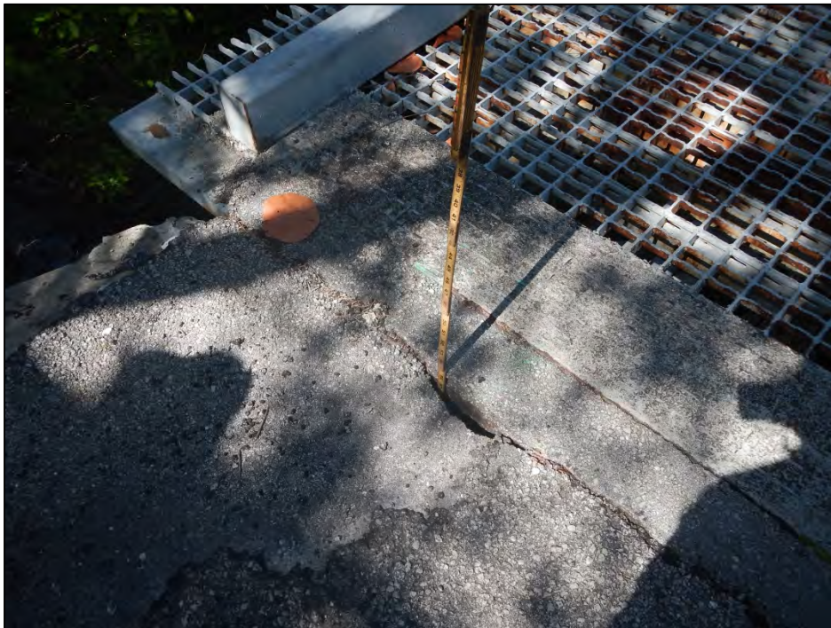
Photo 8 – Full depth void in the west approach roadway/bridge deck transition.
