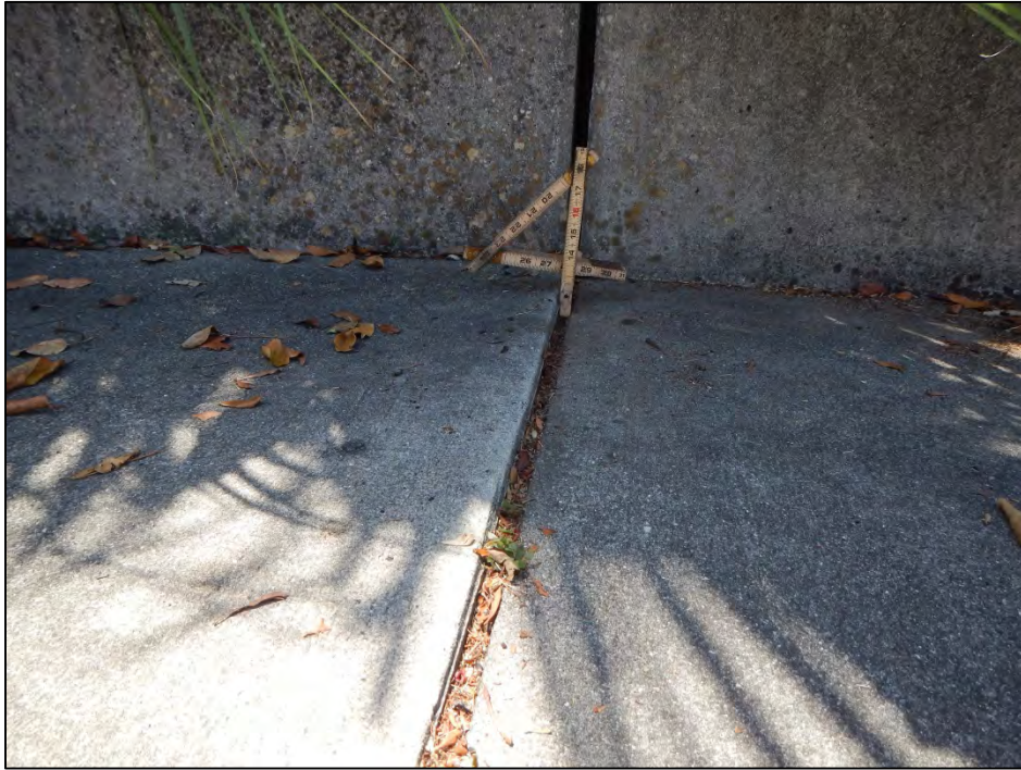
Photo 5 – Settlement in the southeast approach sidewalk.
