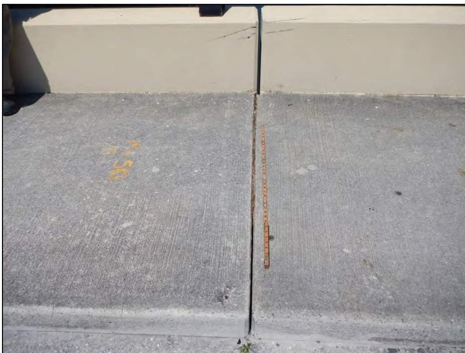
Photo 4 – Sidewalk joints filled with dirt and debris.
