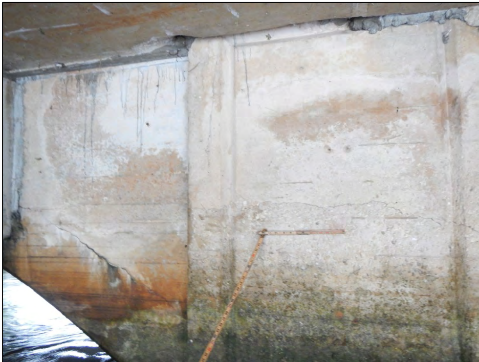
Photo 10 – West side of Pier 2 of the arch – diagonal and horizontal cracks.
