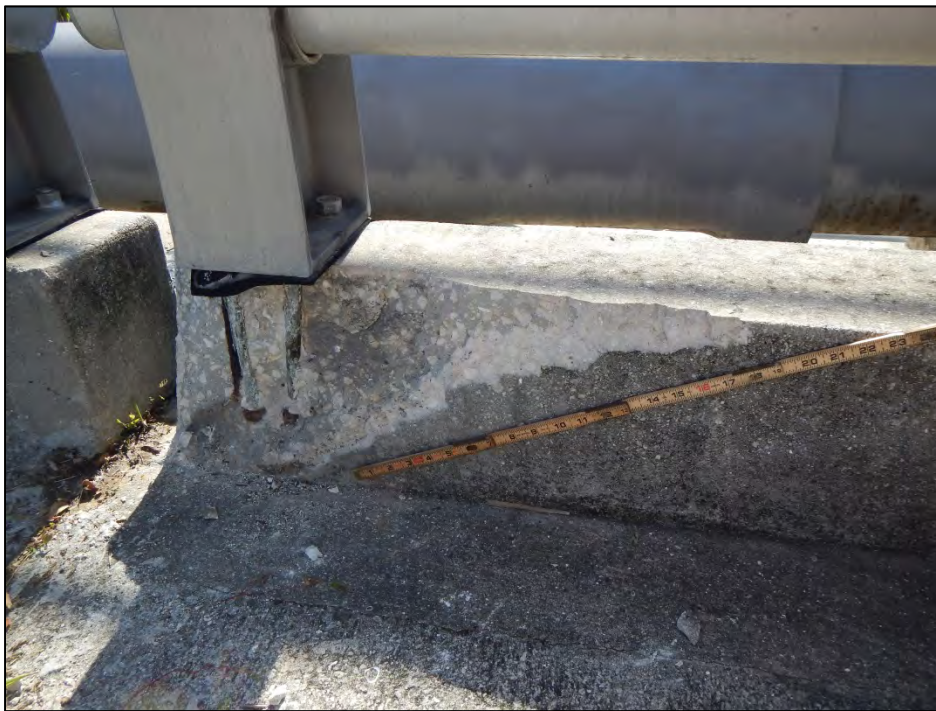
Photo 6 – The concrete parapet below Post I-3 right exhibits a spall with exposed anchors.
