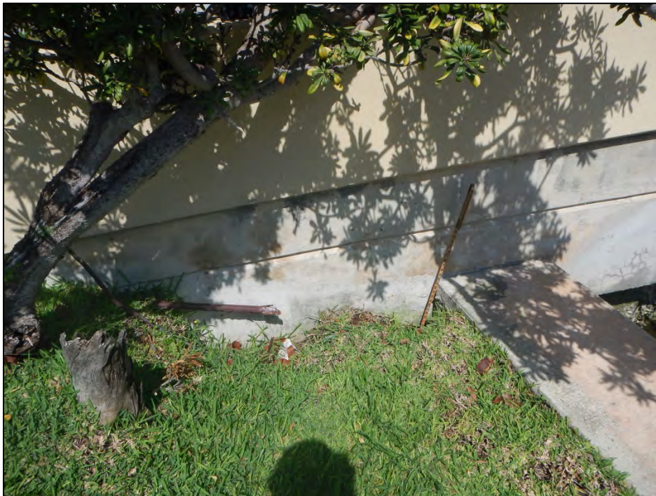
Photo 4 – Backfill void at southeast corner.
