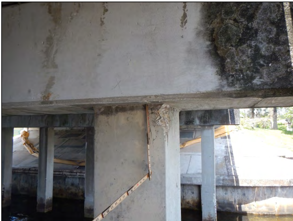
Photo 18 – The northeast corner of Pile 3-1 exhibits a spall.
