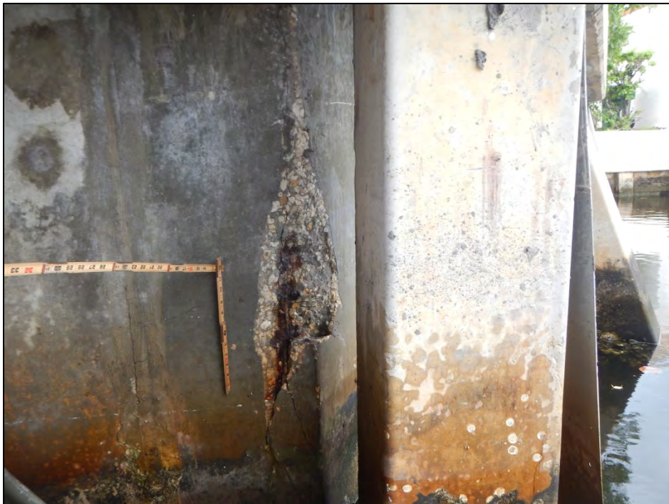
Photo 10 – The south end of the Abutment 2 backwall exhibits a spall/delamination.
