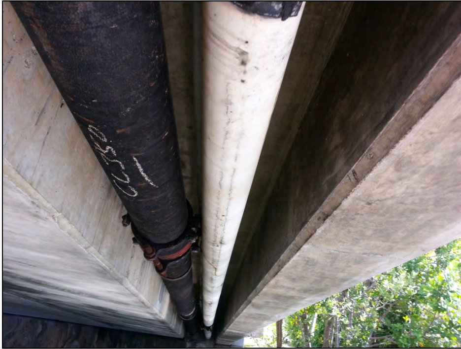
Utilities mounted to deck underside
