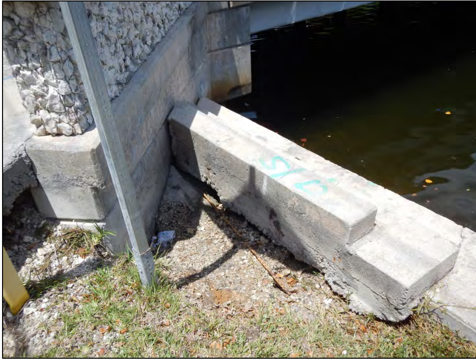
Photo 5 – Washout area behind the retaining wall adjacent to the southwest concrete barrier.
