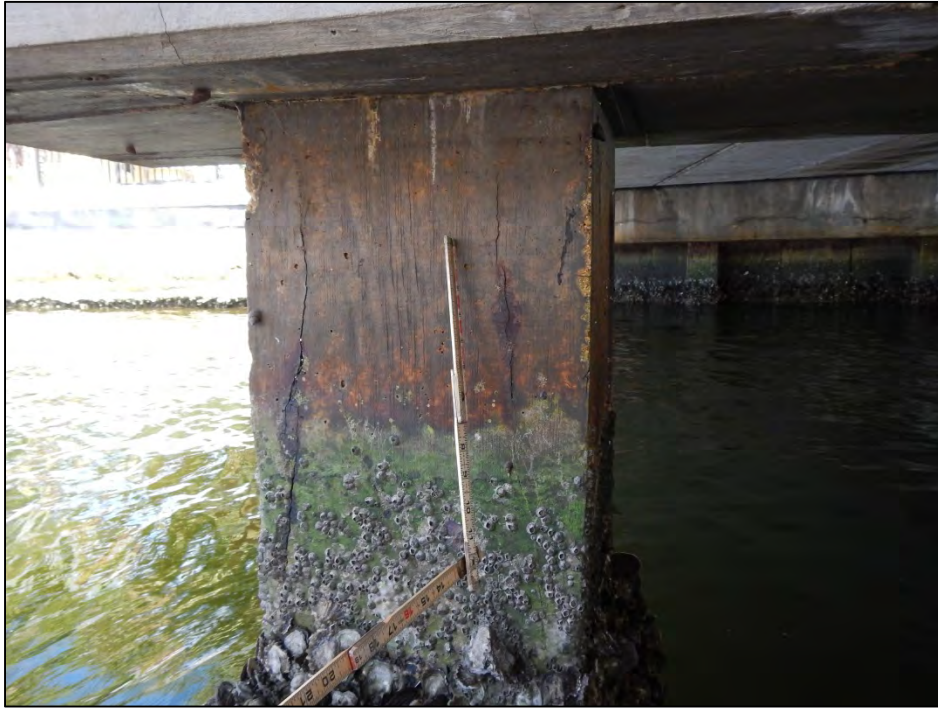
Photo 5 – Corrosion staining and cracks on Pile 3-I.
