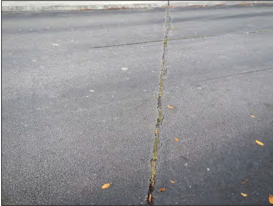
Photo 1 – End Bent 1 joint seal transverse crack.
