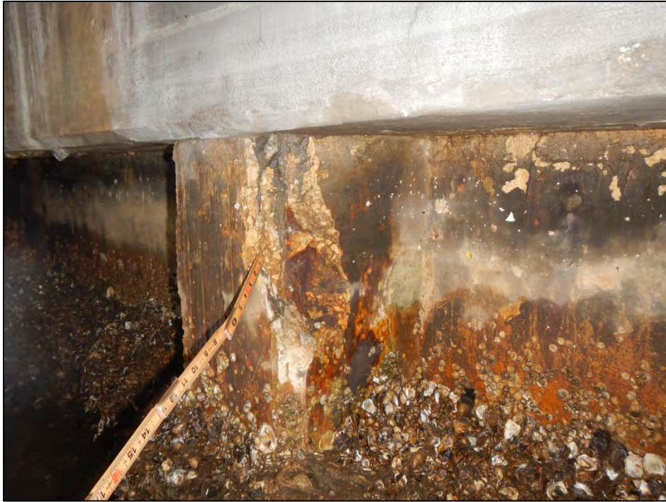
Photo 15 – Pile 2-4 exhibits a spall with corroded exposed steel.
