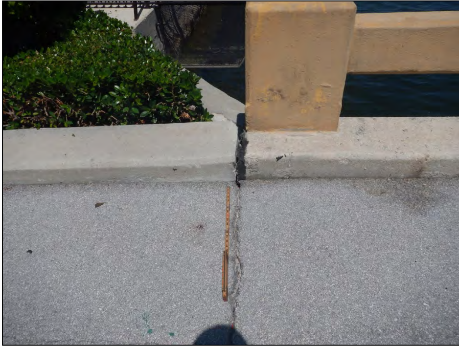
Photo 1 – Deteriorated joint sealant in the left sidewalk over Abutment 1.
