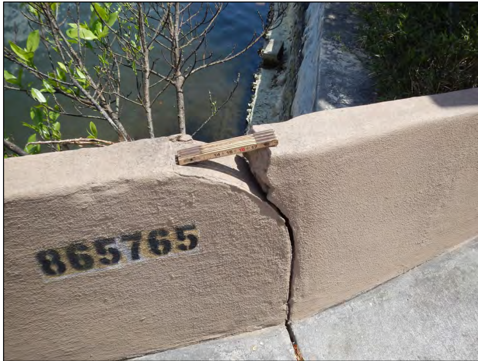
Photo 1 – Spall in the barrier.
