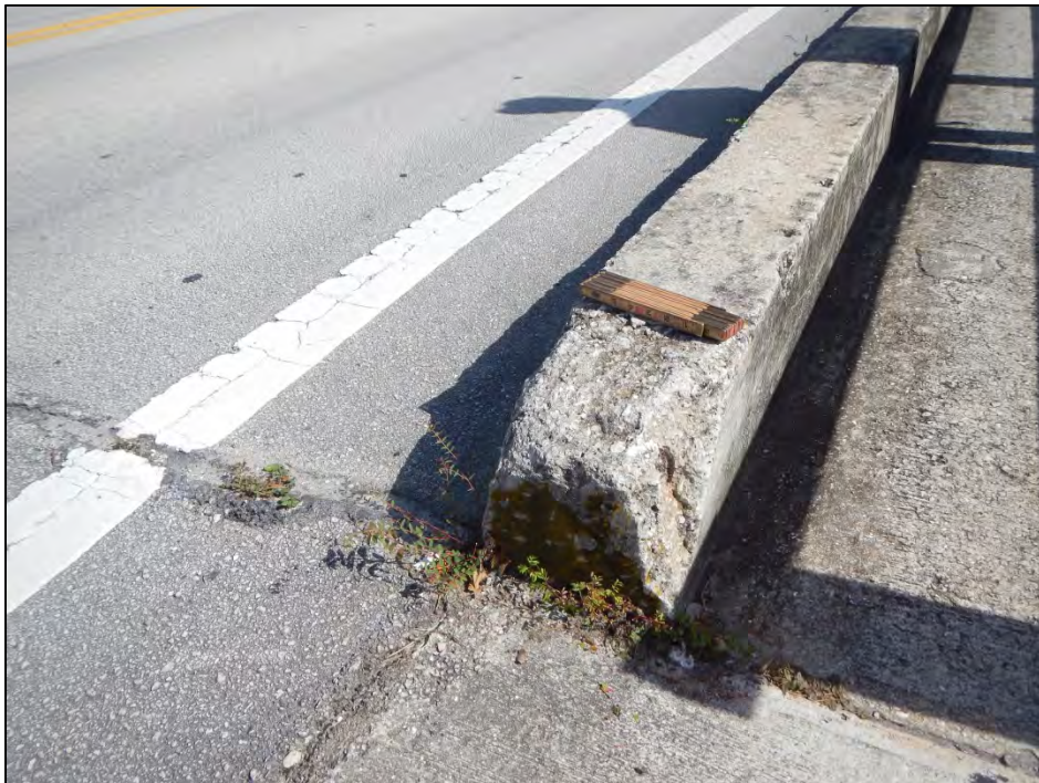
Photo 4 – The right curb over Span I has a spall with exposed steel.
