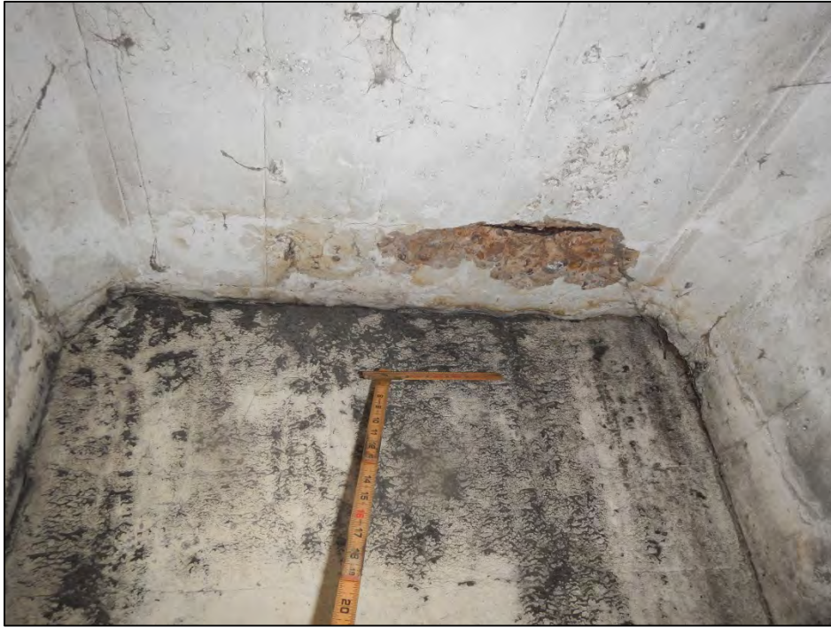
Photo 5 – Bay 5 over Abutment 2 exhibits a spall with exposed steel.
