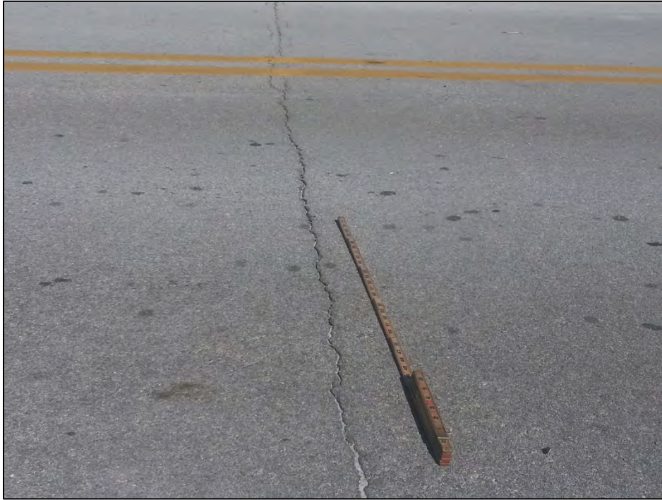
Photo 1 – Cracks in the asphalt overlay.
