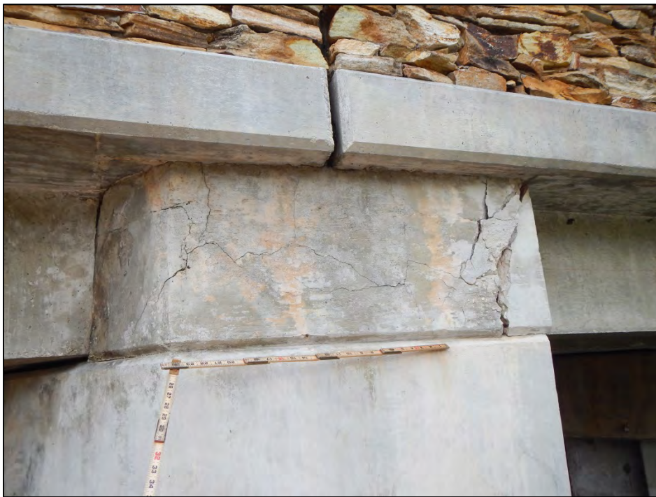
Photo 6 – The Bent 2 cap has a delamination in the north end.
