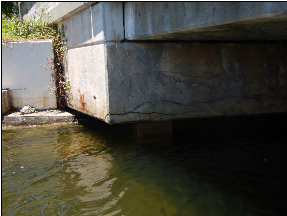
Photo 6 – Delaminated area in Abutment I cap.
