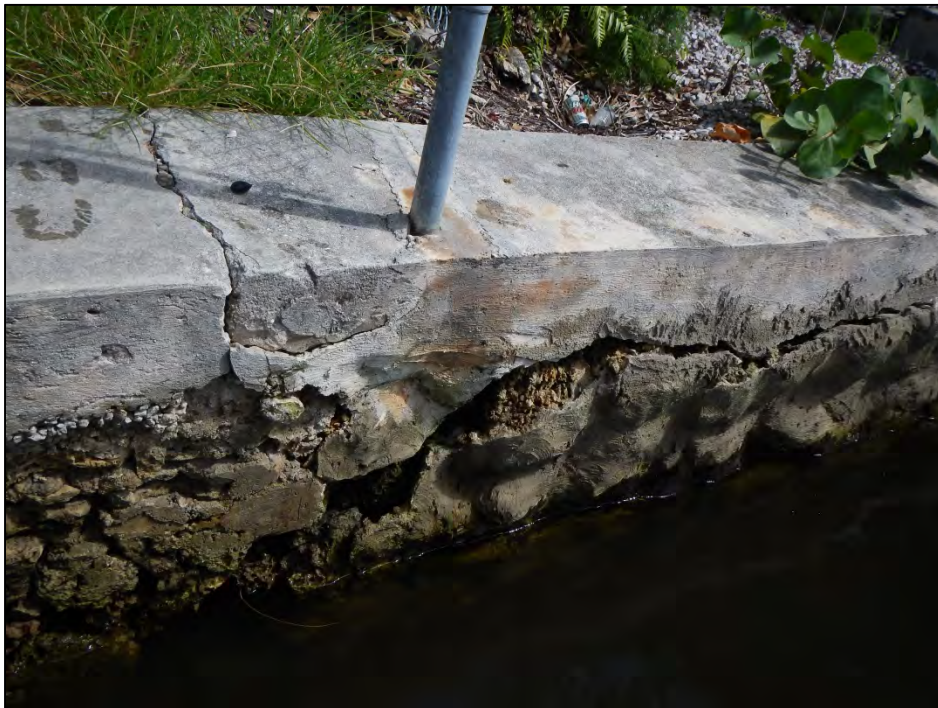
Photo 6 – Crack and rotation in the northeast retaining wall.
