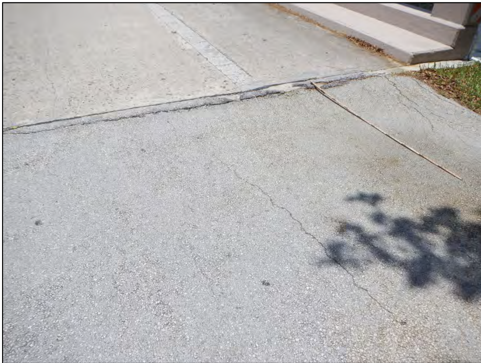
Photo 6 – The east approach roadway exhibits longitudinal cracks.
