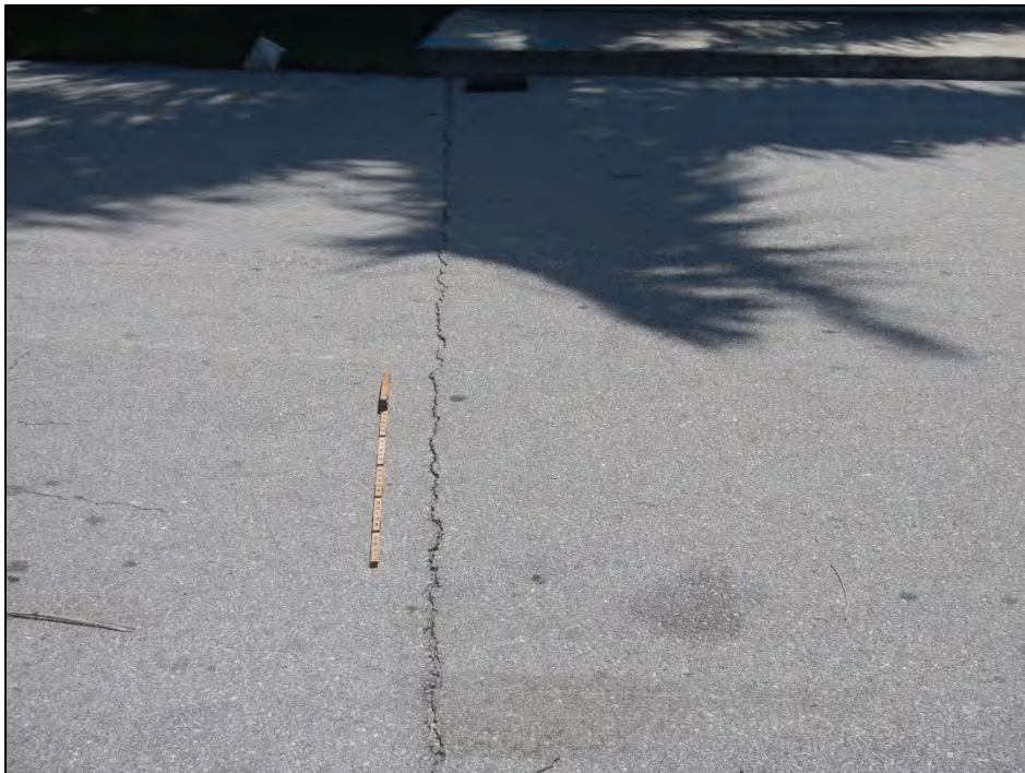
Photo 14 – Crack in asphalt at the roadway transition.
