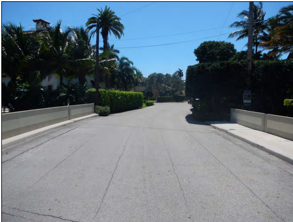
Photo 2 – General view of cracks in asphalt overlay.
