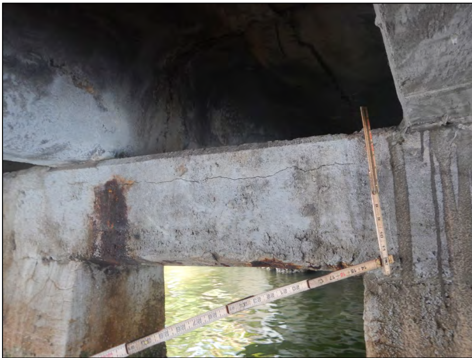
Photo 4 – Cracks and corrosion staining on the intermediate Bent caps.
