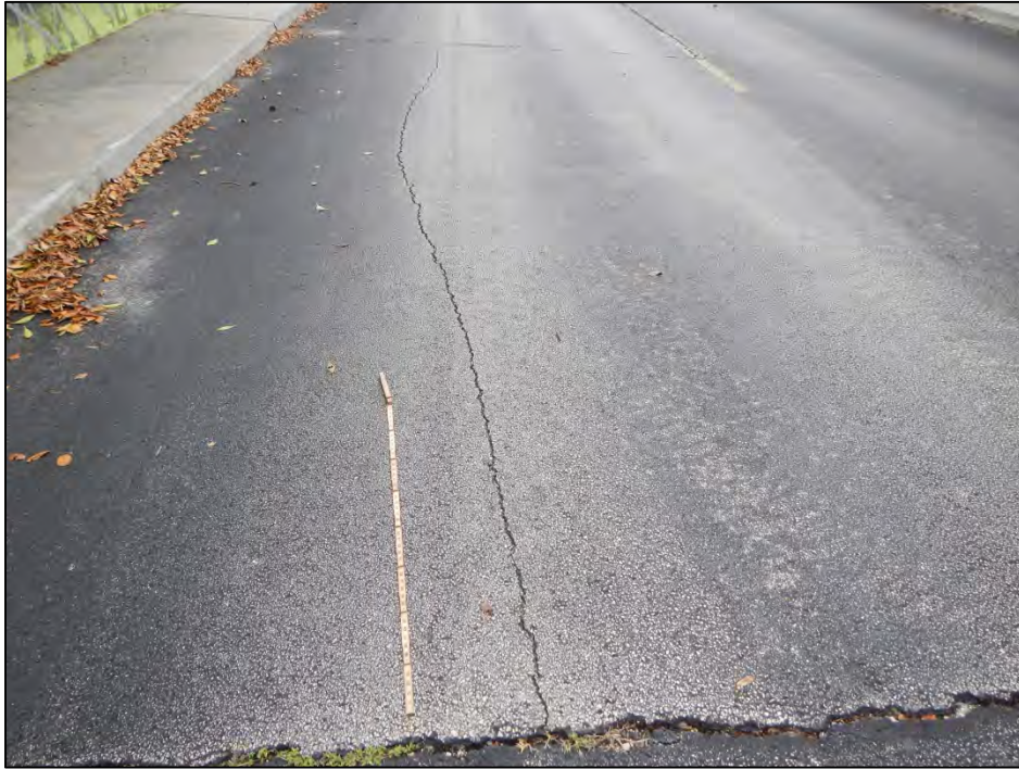
Photo 15 – West approach slab longitudinal crack.
