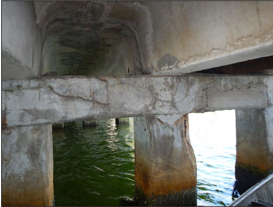
Photo 7 – Spall and delamination on the southeast corner of Pile Jacket 4-7.
