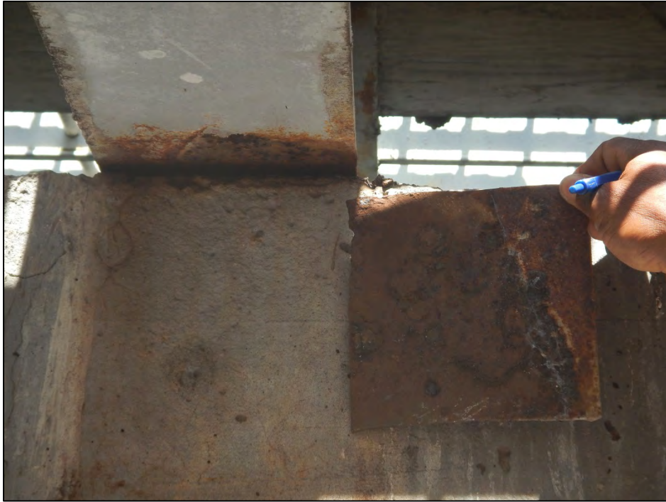
Photo 5 – Loose shim plate at Beam 1-3.
