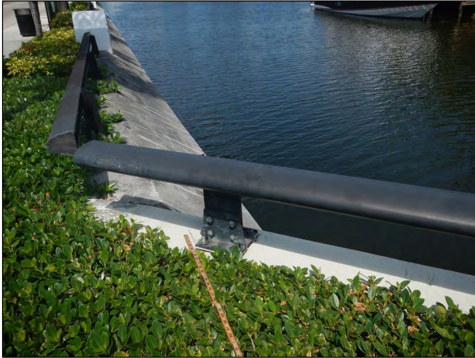
Photo 3 – Loose nuts at the southwest corner of the pedestrian railing.
