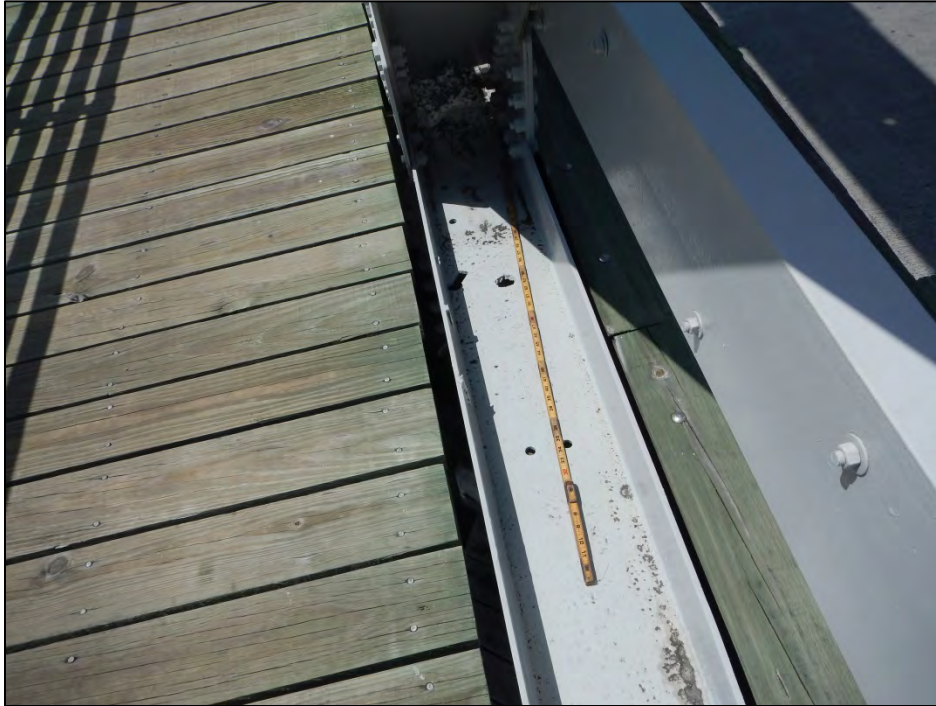
Photo 7 – Typical holes in bottom chord.
