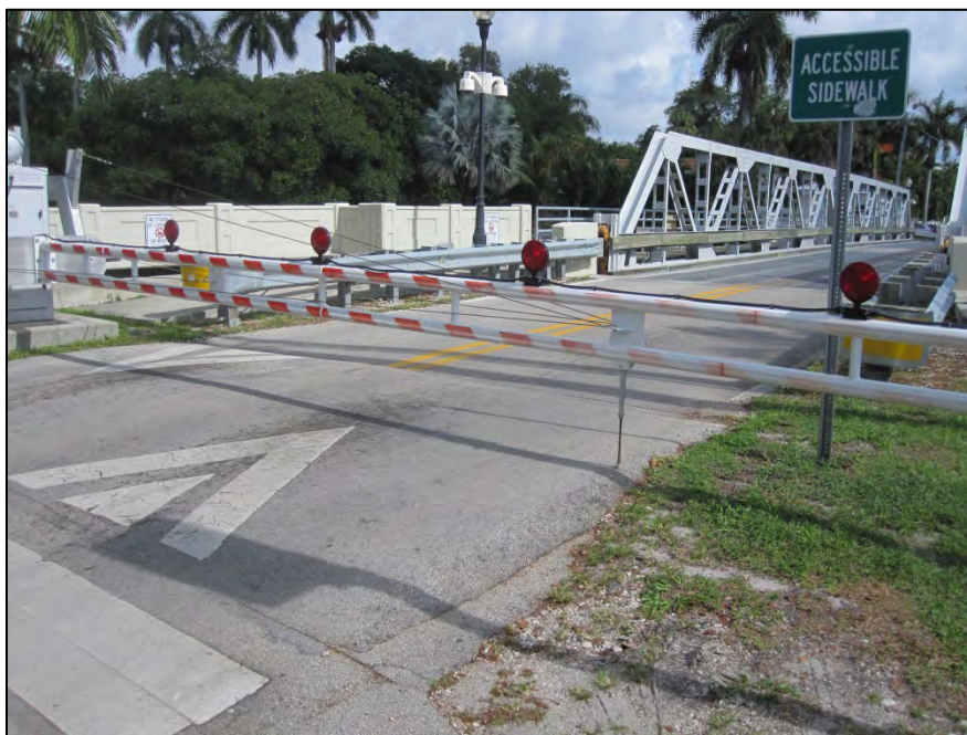
Photo 29 – Faded striping on the far gate arm.
