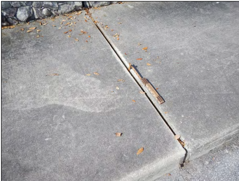
Photo 2 – Deteriorated sidewalk joint sealant.
