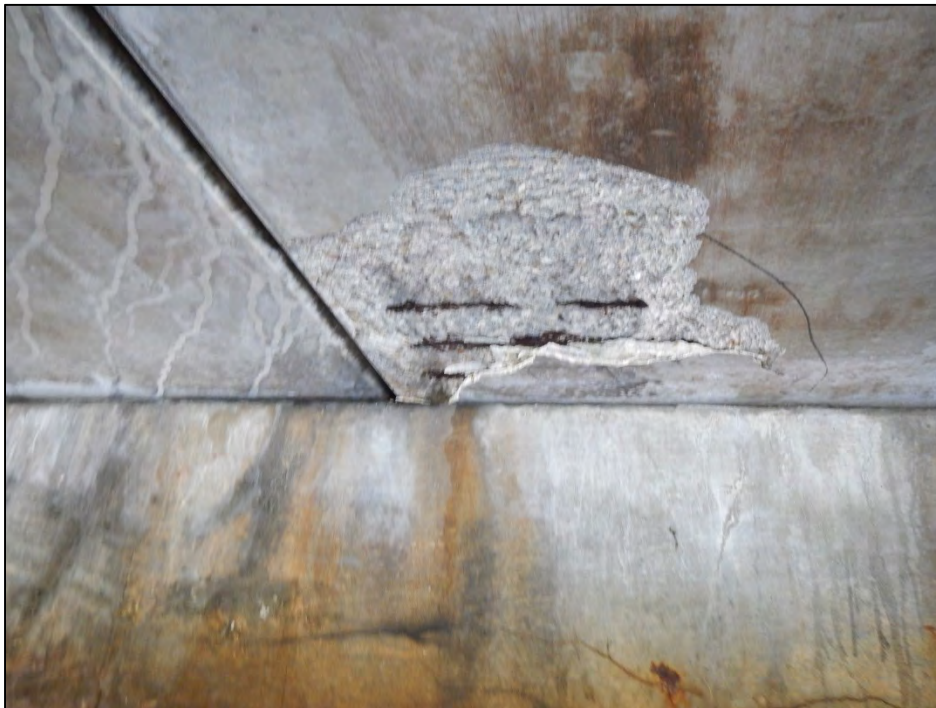
Photo 4 – Spall with exposed rebar in the underside of Slab Unit 3-4.
