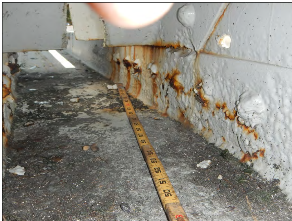
Photo 9 – Corrosion with section loss on rivets.
