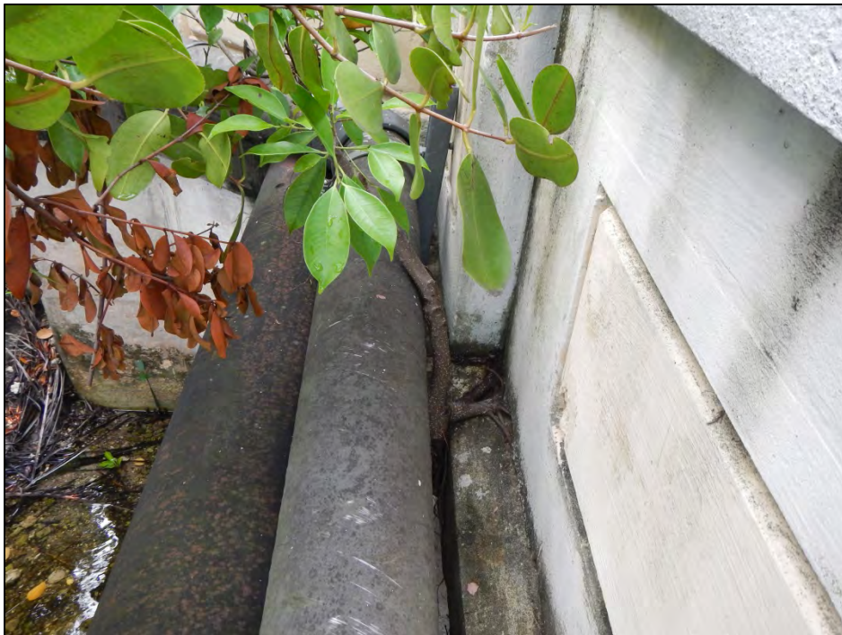
Photo 12 – End Bent 1 at the east side exhibits vegetative growth.
