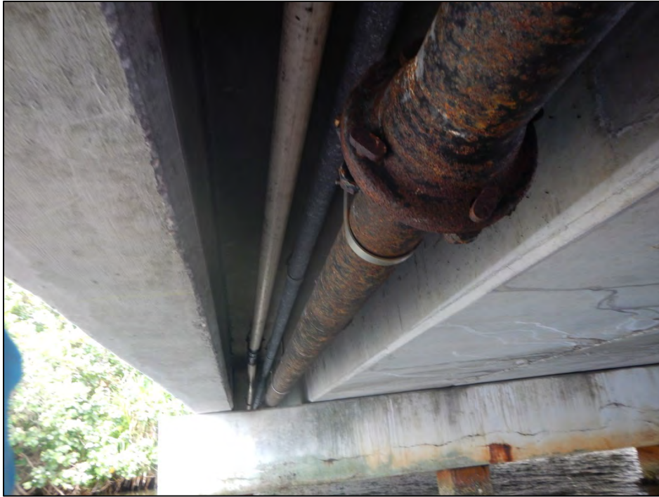
Utilities mounted to deck underside
