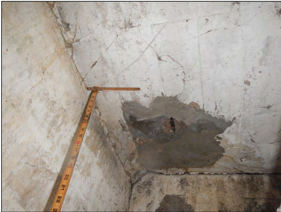
Photo 6 – Bay 7 over Abutment 1 exhibits a spall/delamination with exposed steel.
