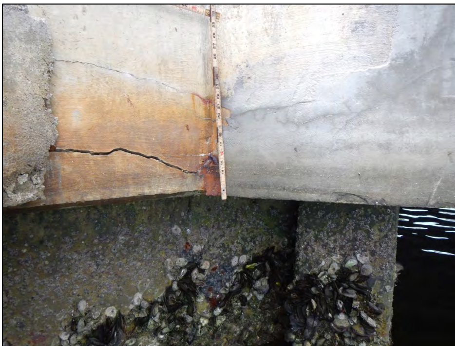
Photo 6 – Delamination with corrosion staining in the southwest wingwall cap.
