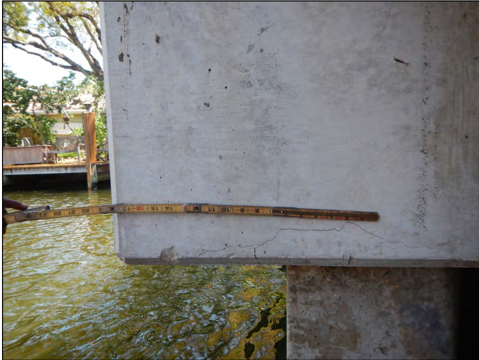
Photo 9 – Delamination in the north face of Bent 3 cap.
