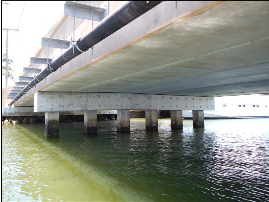
Slab Underside and Intermediate Bent. Note Utility Pipe.
