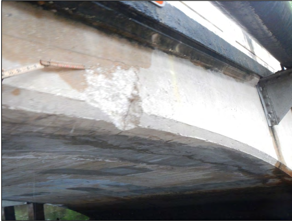
Photo 9 – Span 2 east side spall and delamination at mid span.
