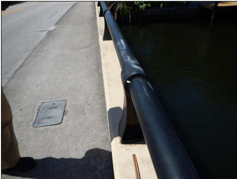
Photo 4 – Handrail pipe does not extend into post.
