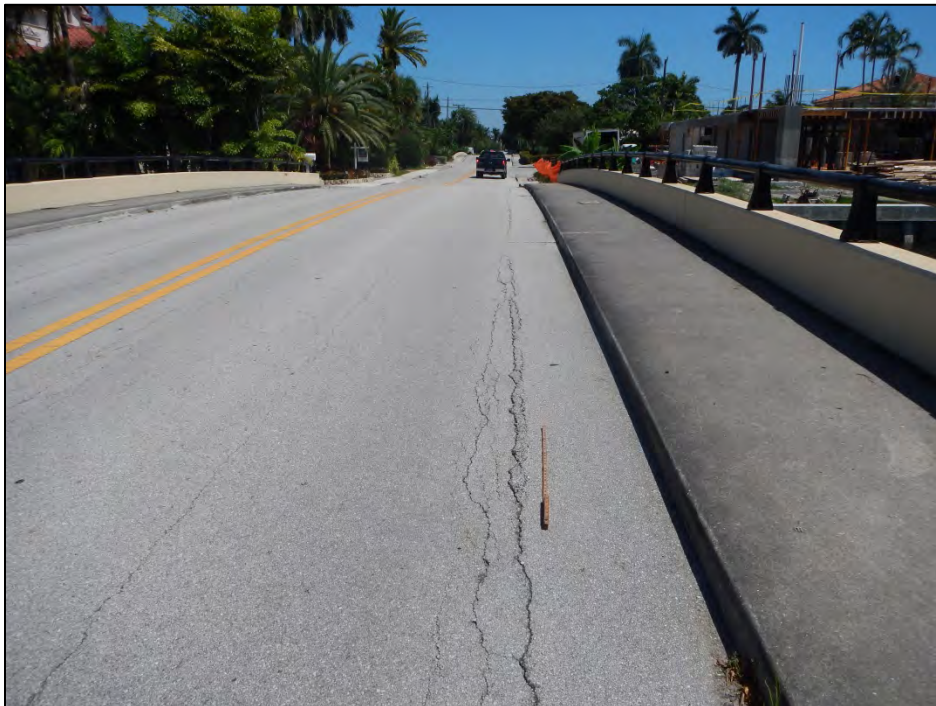
Photo 2 – Longitudinal cracks in asphalt overlay in Span 1.
