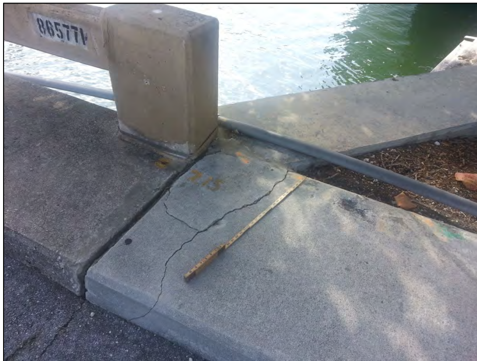
Photo 8 – Delamination on the northwest approach sidewalk.
