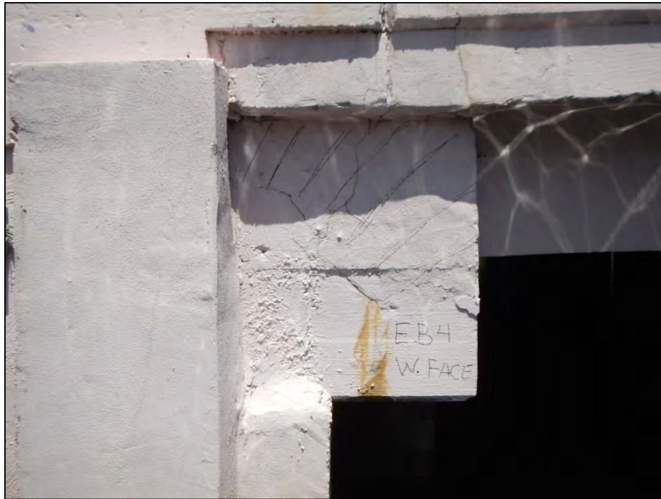
Photo 7 – The west face of Abutment 4 exhibits a delamination.
