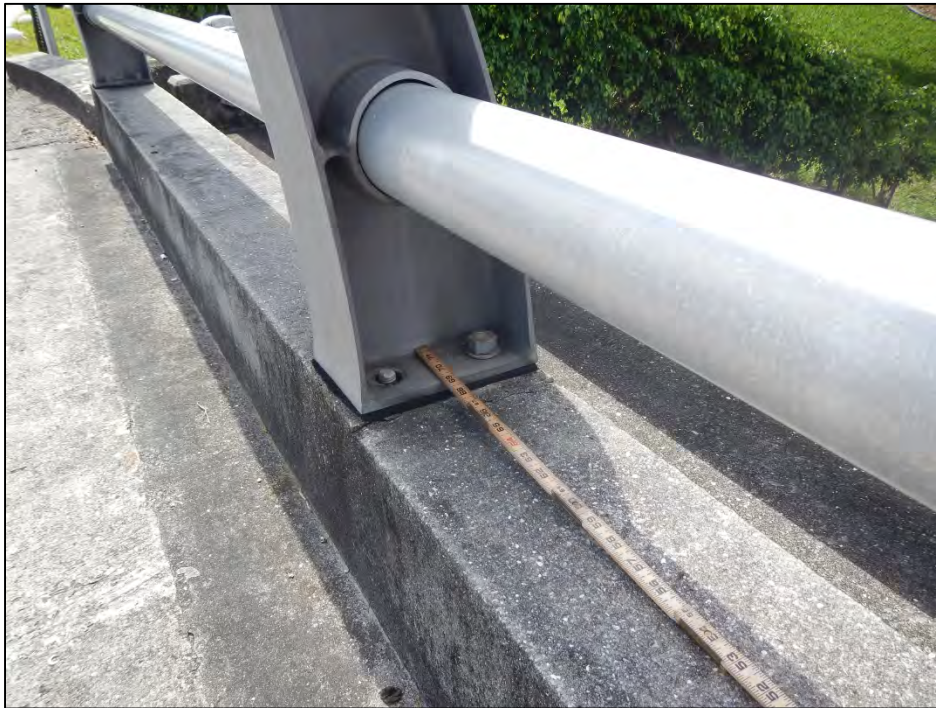
Photo 5 – Post 3-2 Right is missing an anchor bolt nut.
