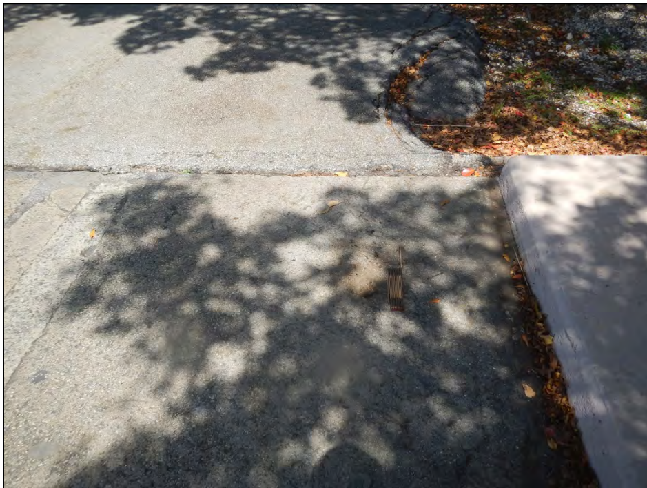
Photo 6 – The deck top exhibits an unpatched pick up point.
