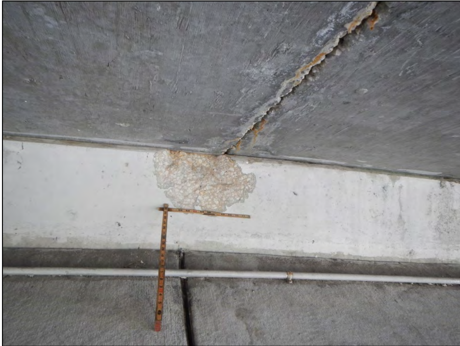
Photo 11 – End Bent 4 cap exhibits a spall between Slab Units 3-7 and 3-8.
