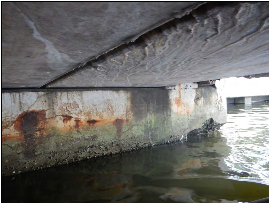
Photo 10 – Spall with exposed corroded rebar at Abutment 1 cap.
