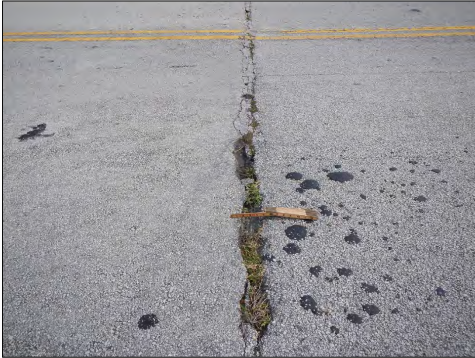
Photo 1 – End Bent 1 joint seal transverse crack.
