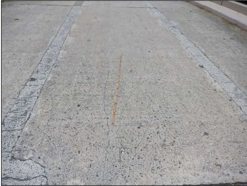
Photo 5 – The deck top exhibits multi-directional cracks.
