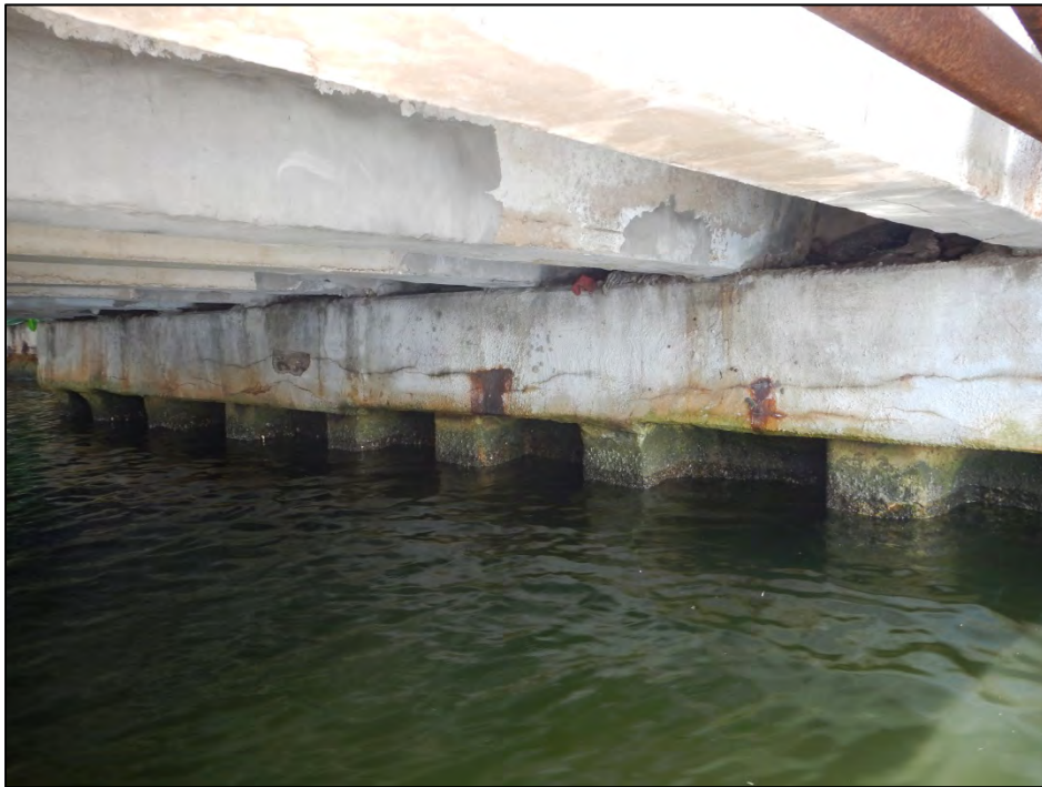
Photo 6 – Delamination on the Bent 5 cap.
