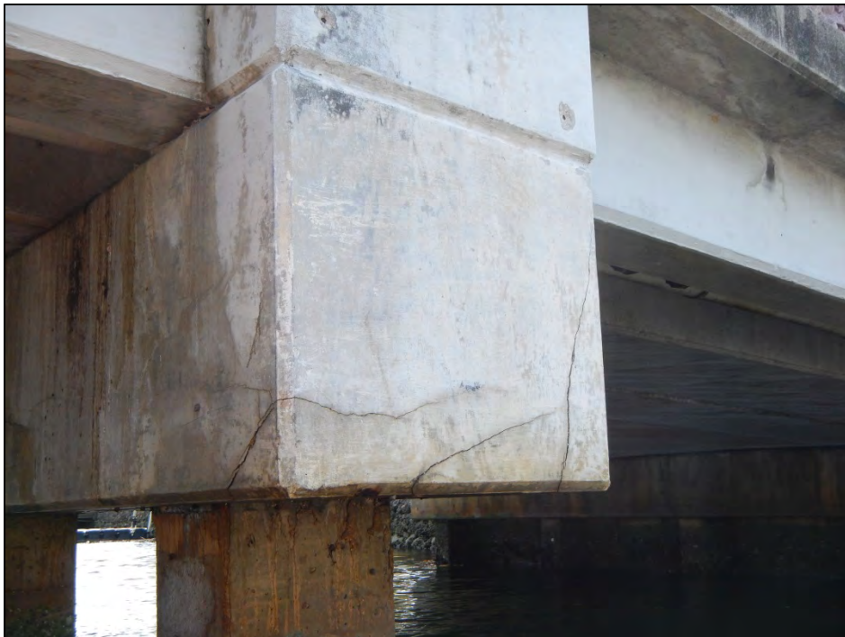
Photo 4 – Spalls and delaminations in the cap at Bent 2.
