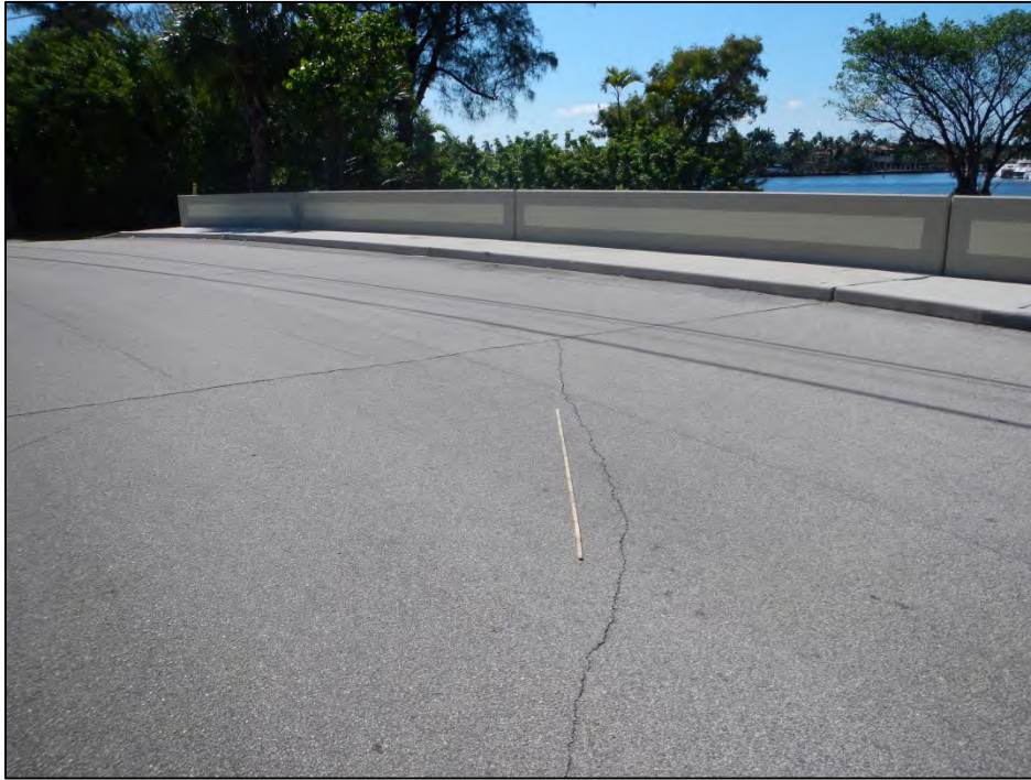
Photo 7 – Diagonal crack in asphalt over east approach slab.
