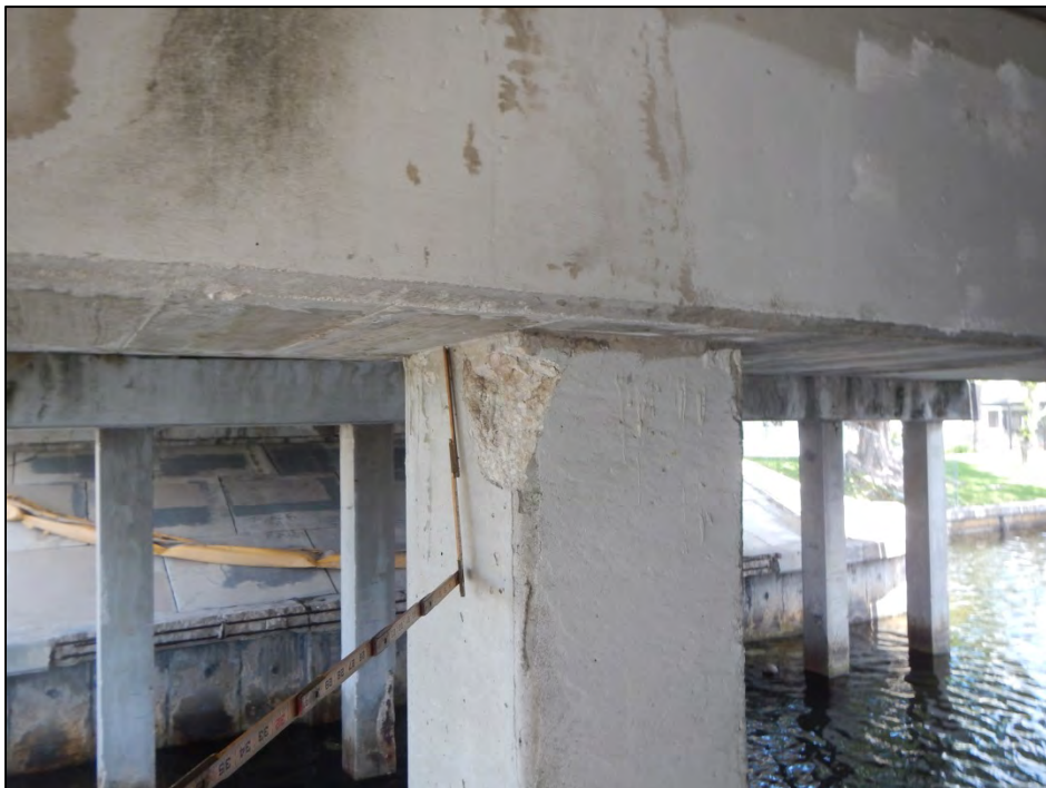
Photo 20 – The southeast corner of Pile 3-6 exhibits a spall.
