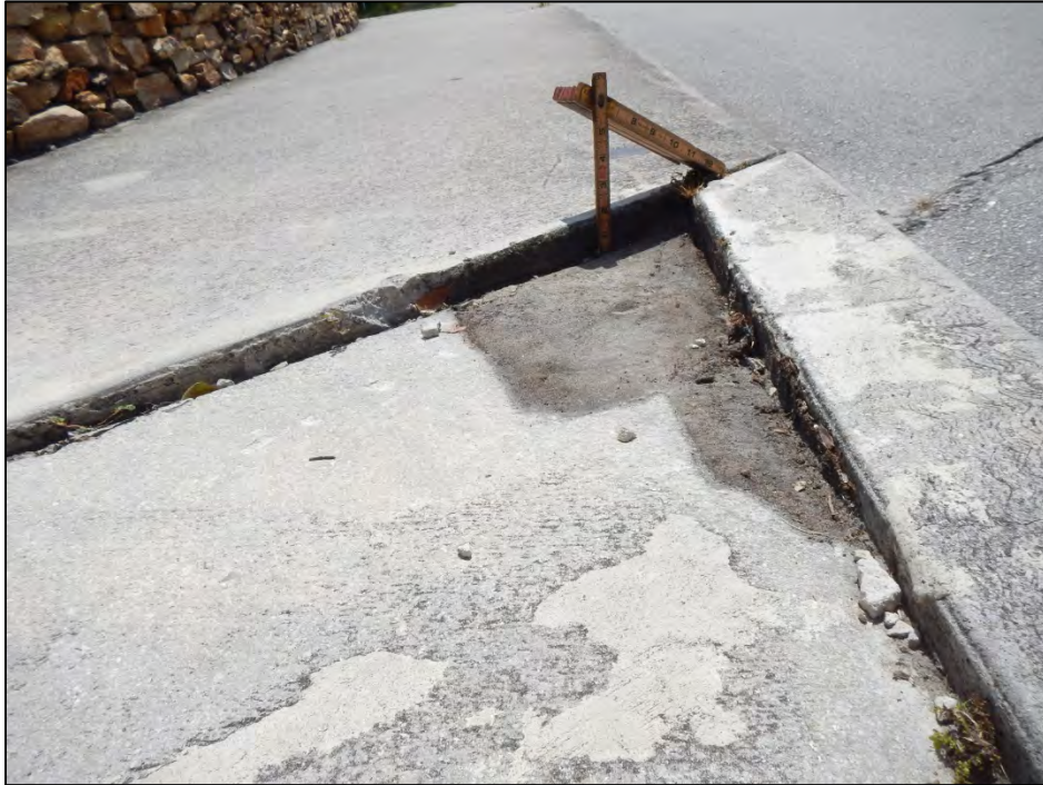
Photo 15 – The northwest sidewalk exhibits a drop-off.
