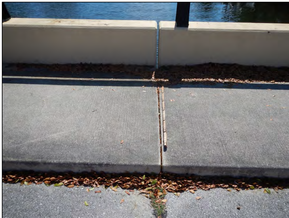
Photo 4 – Deteriorated sidewalk joint filled with dirt and debris.
