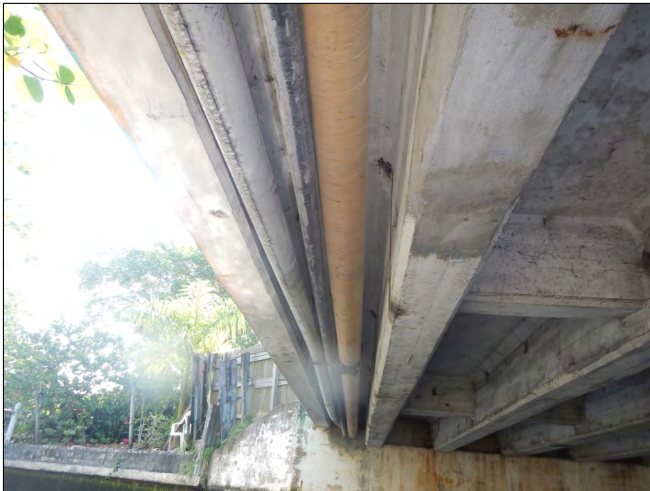
Utilities Mounted under North Fascia
