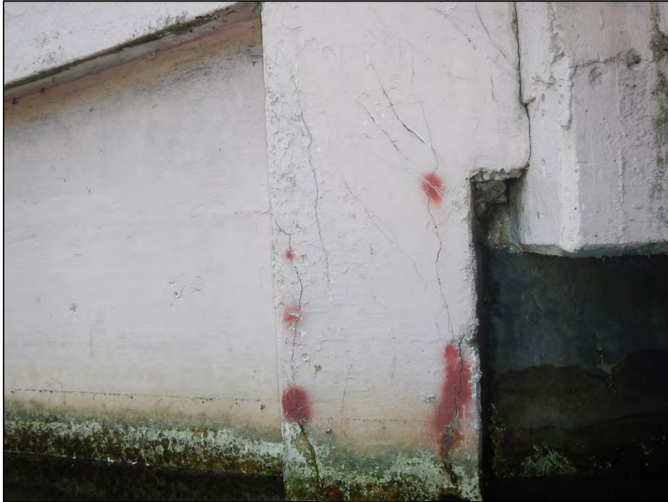
Photo 11 – The first pile of the southeast retaining wall exhibits a delamination with corrosion staining.
