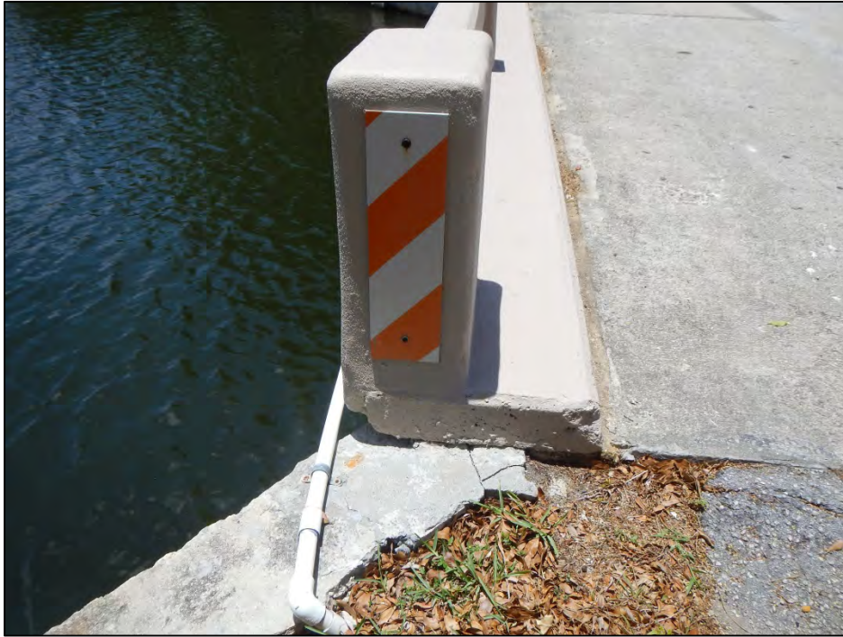
Photo 1 – The diagonal warning sign stripes are oriented incorrectly.
