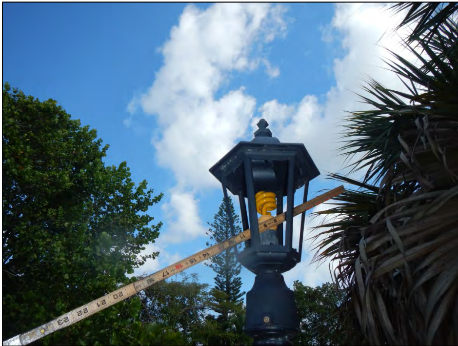
Photo 10 – The first light pole on the south barrier is missing glass panels at the lamp fixture.
