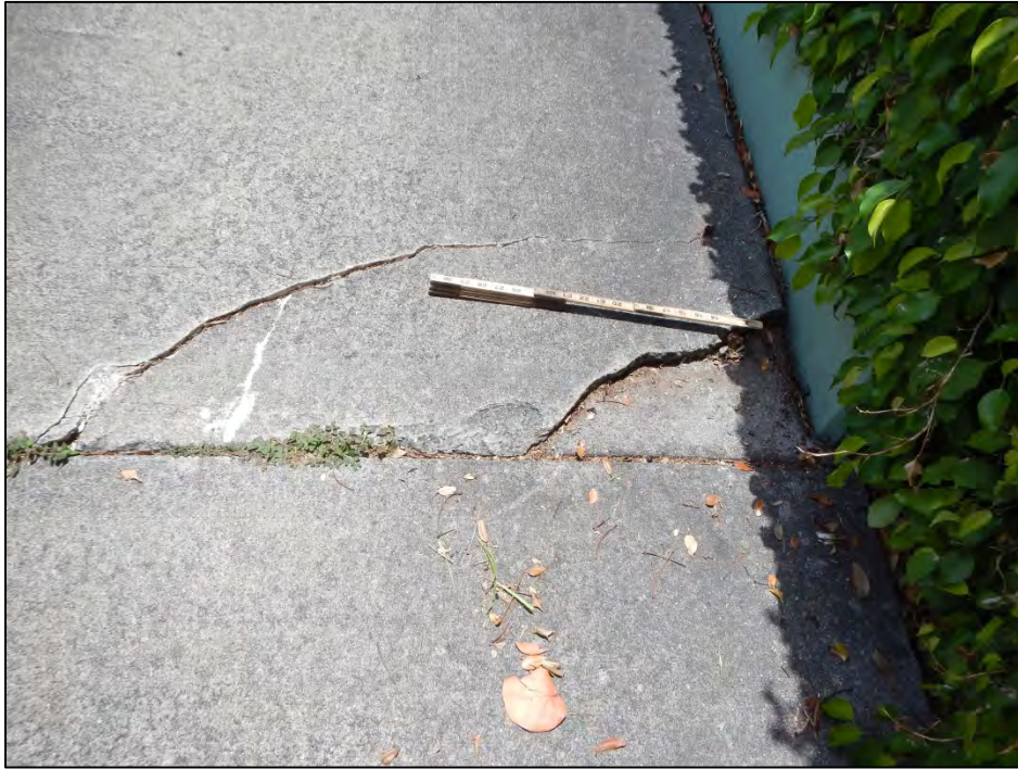
Photo 5 – Cracks in the northwest approach sidewalk.
