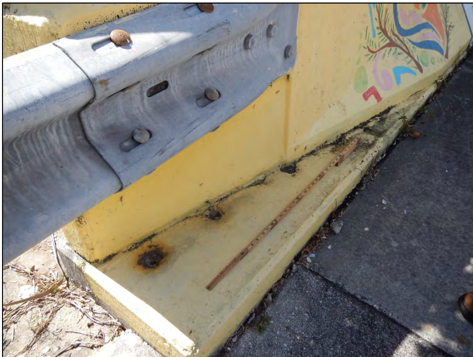
Photo 18 – Southwest approach concrete barrier spalls.
