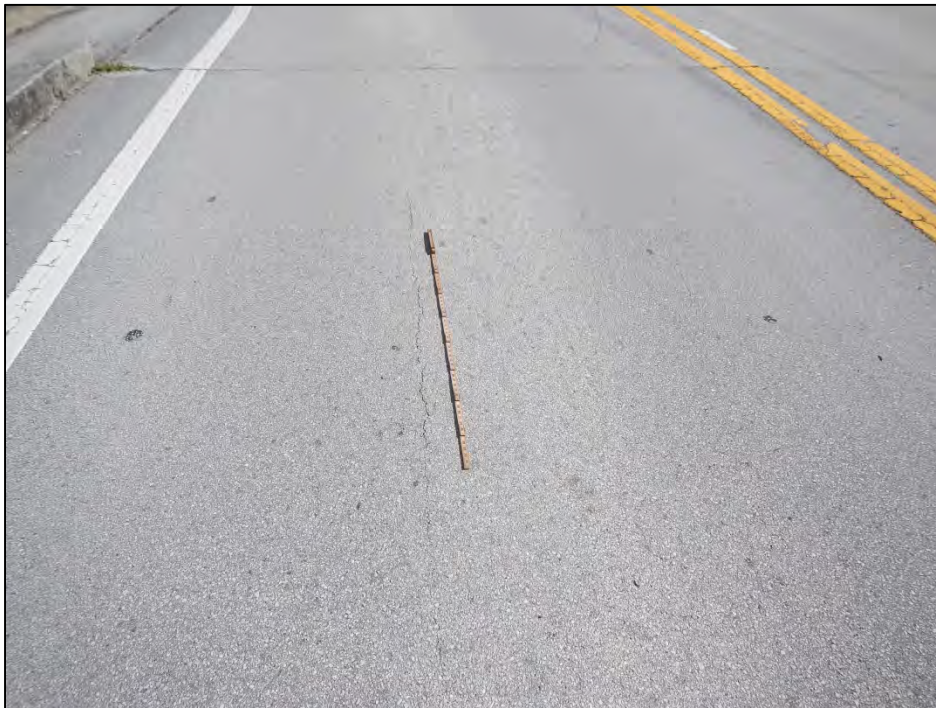
Photo 2 – Deck top longitudinal crack over Span 3.
