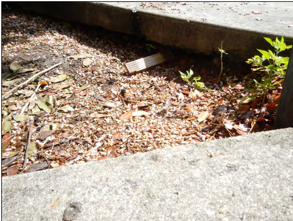
Photo 18 – Northwest approach sidewalk exhibits undermining.
