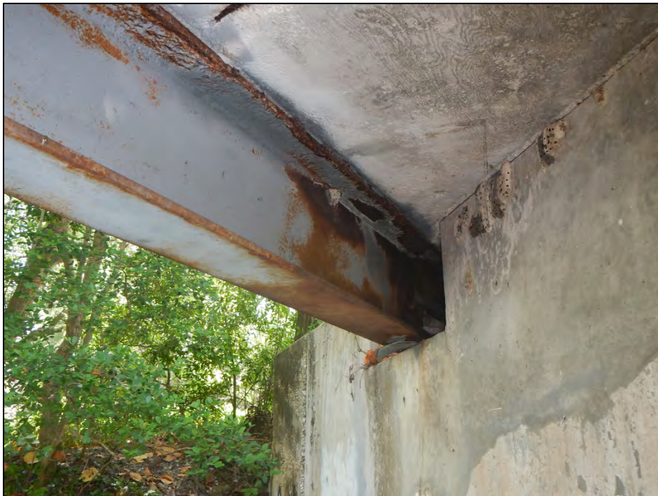
Photo 2 – Corrosion with section loss in Beam 1-8 at Abutment 1.
