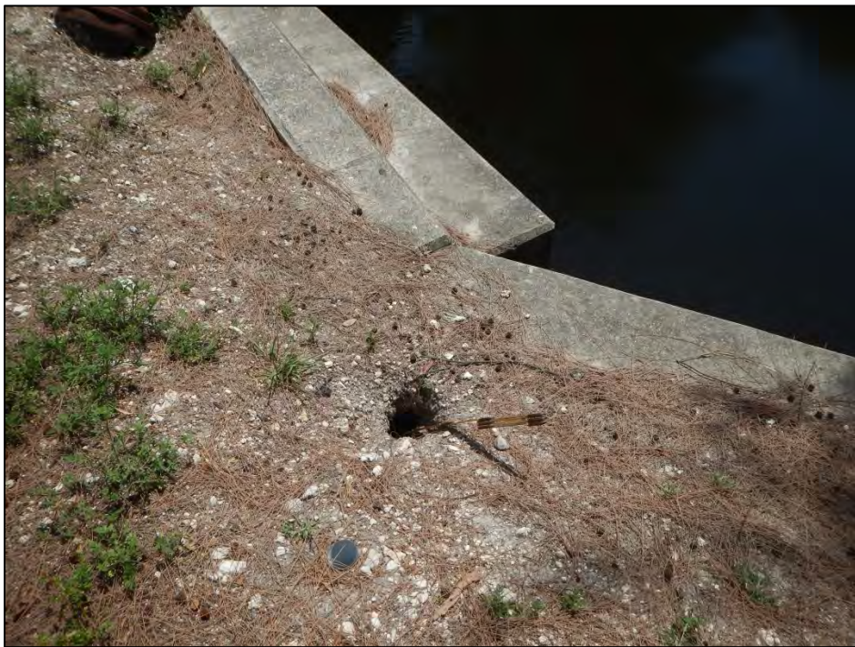
Photo 6 – The southwest retaining wall exhibits a washout behind the bulkhead cap.
