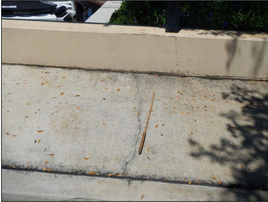
Photo 5 – Cracks in northwest approach sidewalk.
