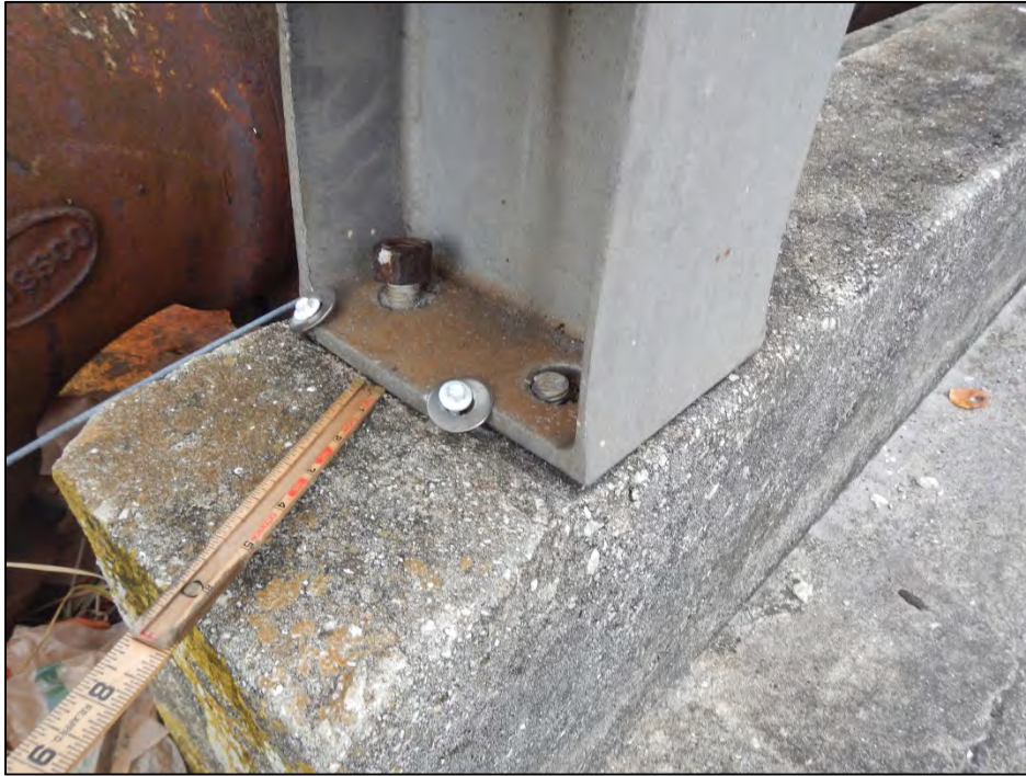
Photo 5 – West railing Post I-2L exhibits 2 of 4 anchor bolt nuts missing.
