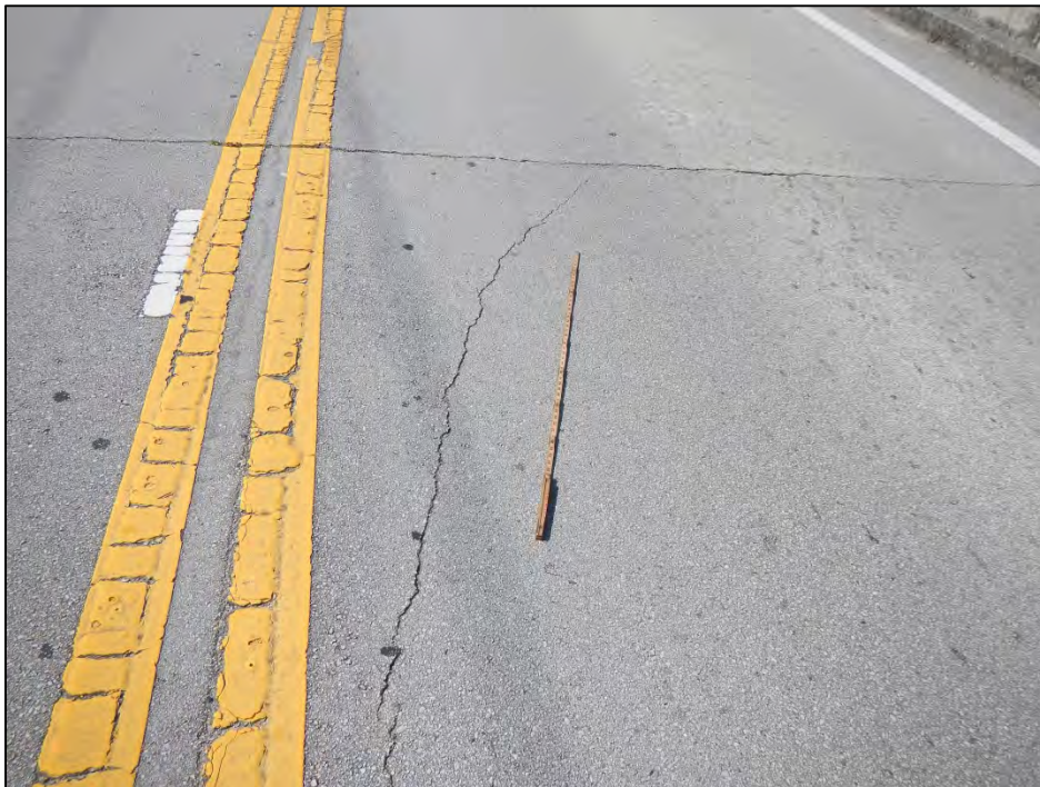
Photo 12 – The north approach slab exhibits a longitudinal crack.
