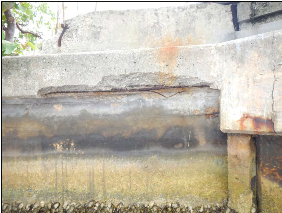
Photo 16 – Southeast wingwall cap exhibits a spall with exposed steel.
