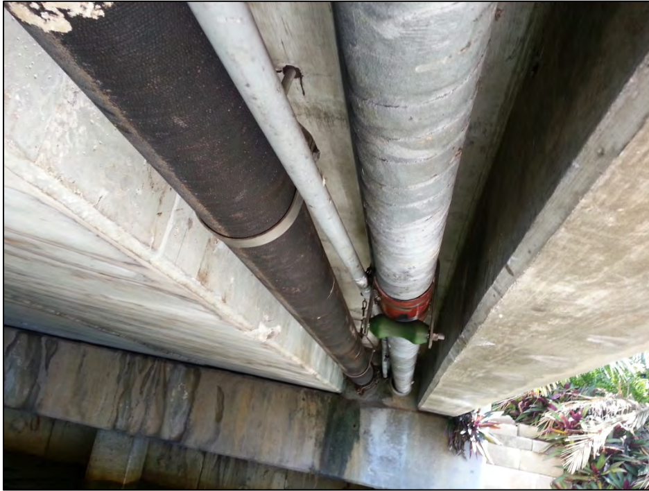
Utilities mounted to deck underside
