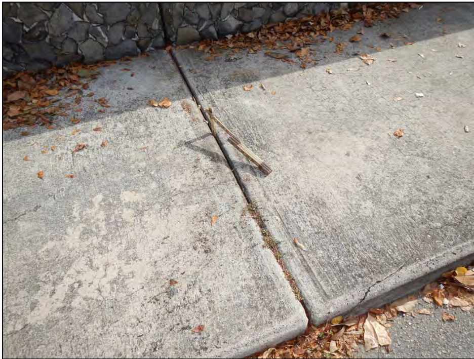
Photo 2 –Deteriorated sidewalk joint sealant.
