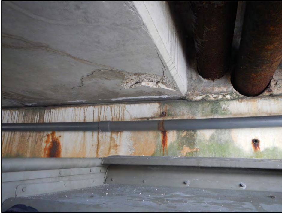
Photo 7 – Spall/Delamination in Slab Unit 3-7 at Abutment 4.
