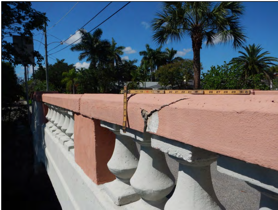
Photo 6 – Delaminated/spalled area near midspan of east railing.
