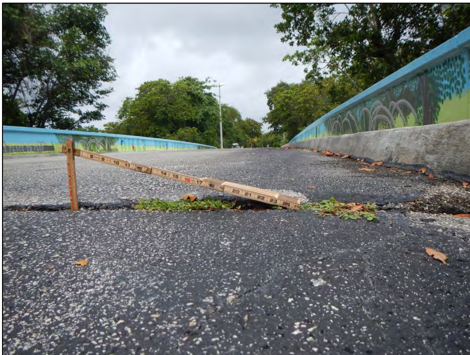
Photo 14 – East approach slab difference in elevation.
