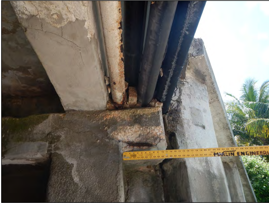
Photo 7 – Spall in the cap at Abutment I with exposed reinforcing steel.
