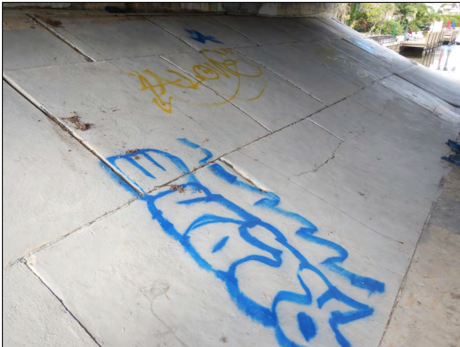
Photo 16 – The End Bent I slope protection exhibits graffiti.
