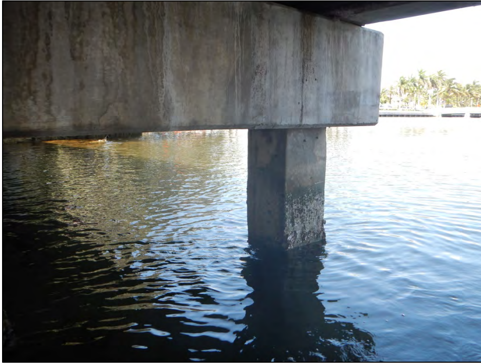
Photo 3 – Crack with corrosion bleedout in Pile 2-I.
