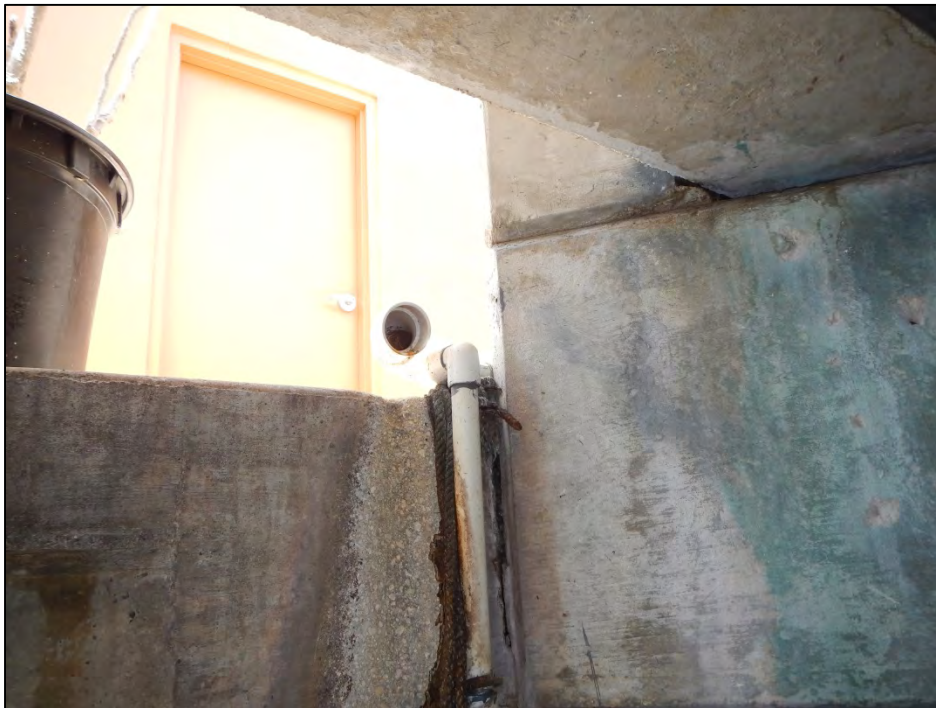
Photo 12 – The southwest wingwall has a utility pipe disconnection.
