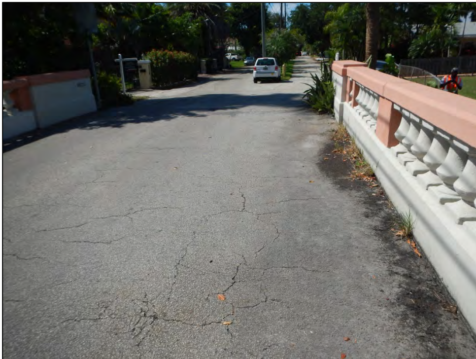
Photo 2 – Depressed area in west half of asphalt overlay near railing.
