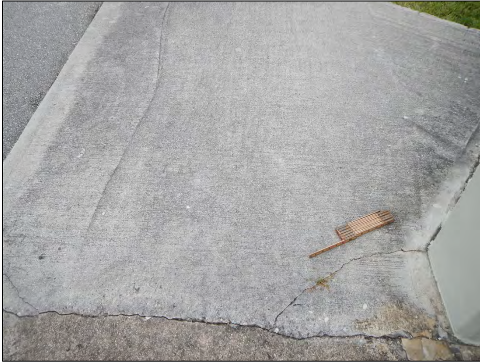
Photo 7 – The southeast approach sidewalk exhibits diagonal cracks.
