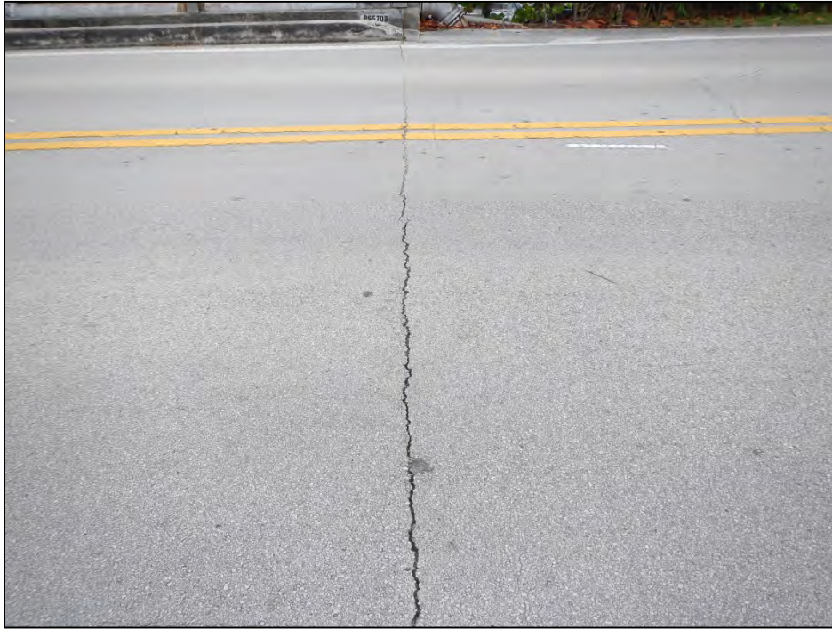
Photo 1 – End Bent 1 joint seal transverse crack.
