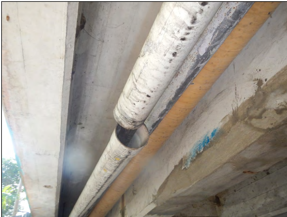
Photo 8 – The utility conduit under Bay I is disconnected.
