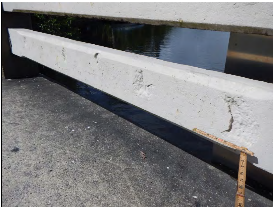
Photo 6 – Left rail between Posts 1-3 and 1-4 exhibits 6 spalls.
