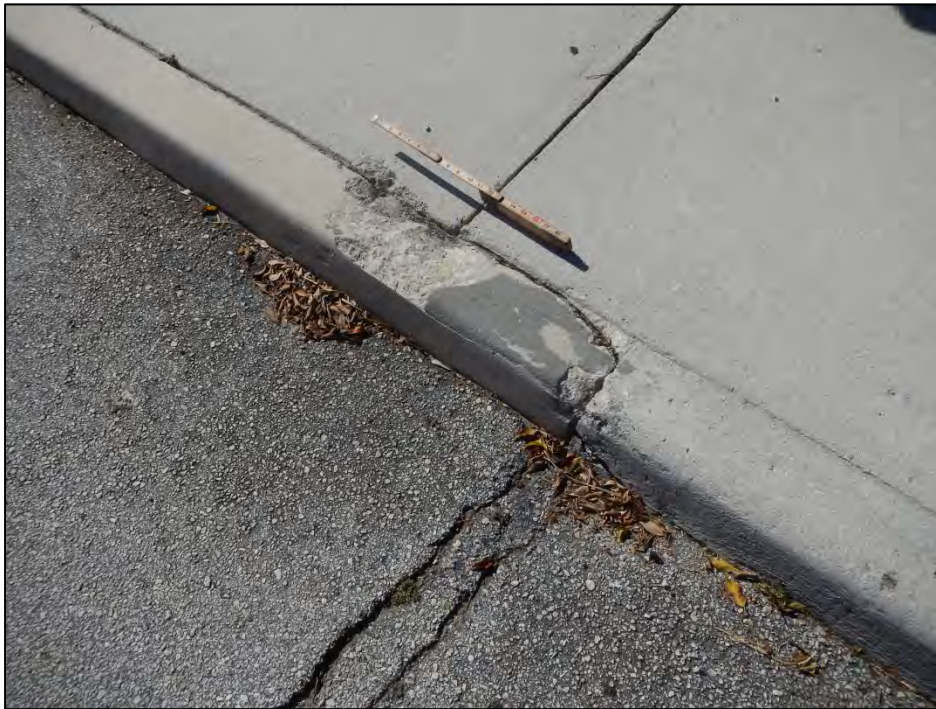
Photo 8 – Spall in northeast approach curb.
