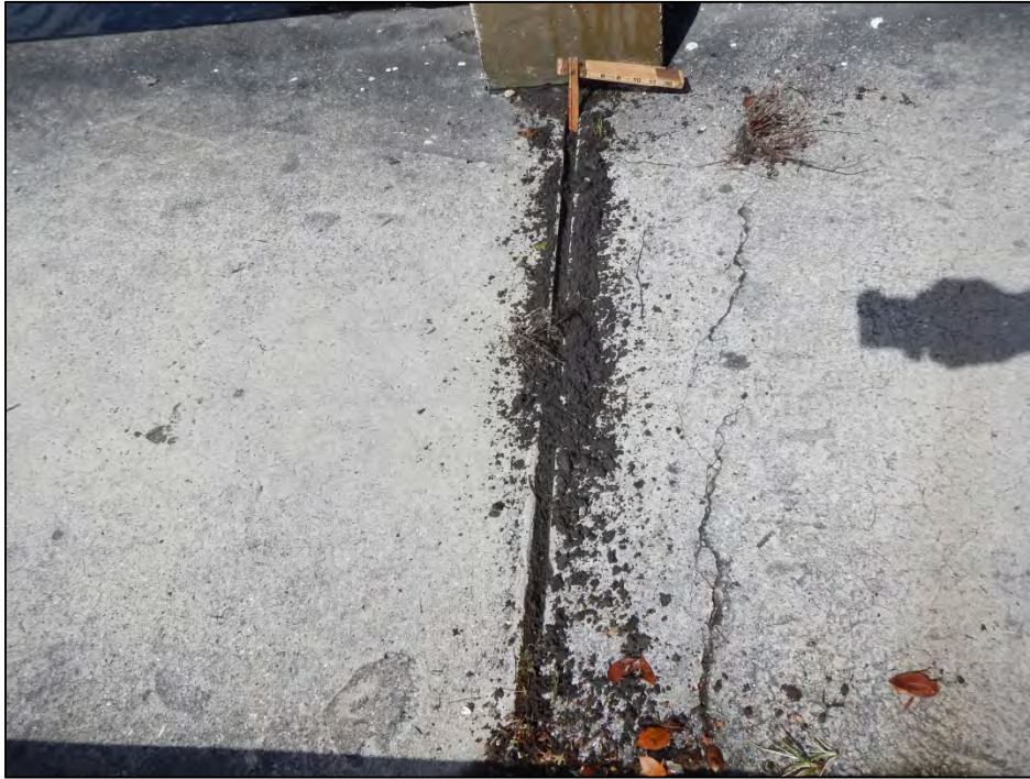
Photo 7 – Joint seal at the west sidewalk is deteriorated and filled with debris.
