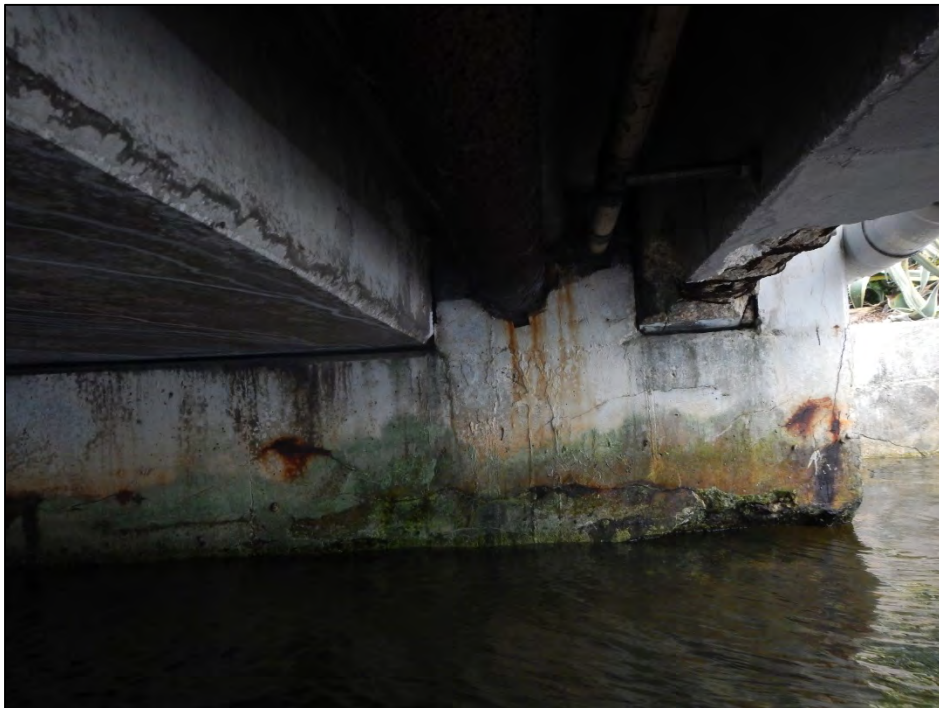
Photo 12 – Spall with exposed corroded rebar at Abutment 4 cap over Pile 4-5.
