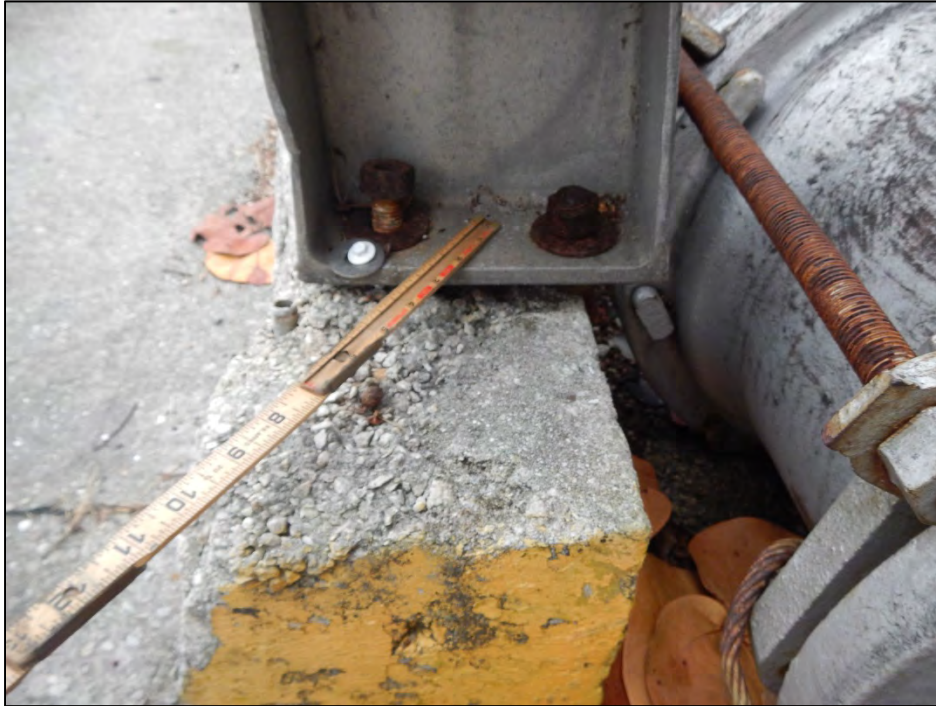
Photo 9 – East railing Post 1 has an improper repair.
