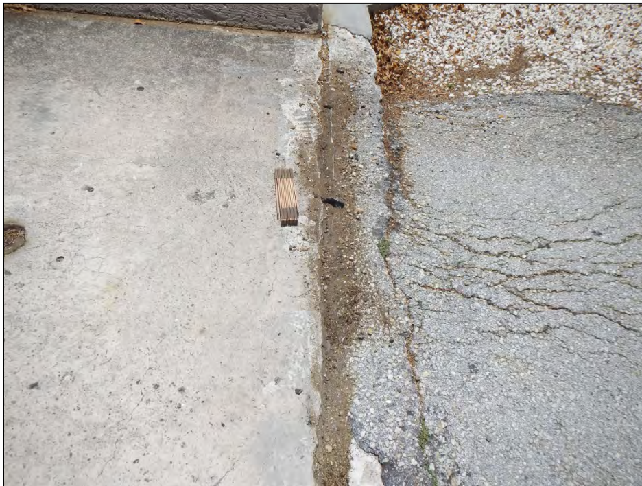
Photo 2 – Abutment I joint seal is deteriorated.
