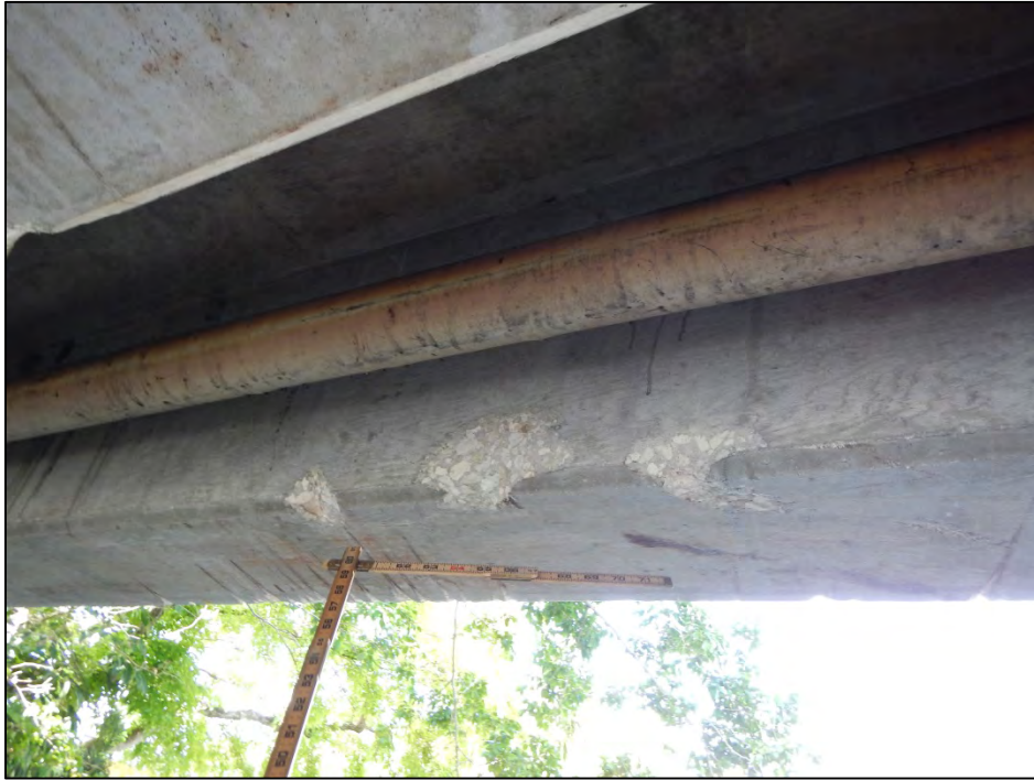
Photo 3 – Beam I-I spalls with no exposed steel.
