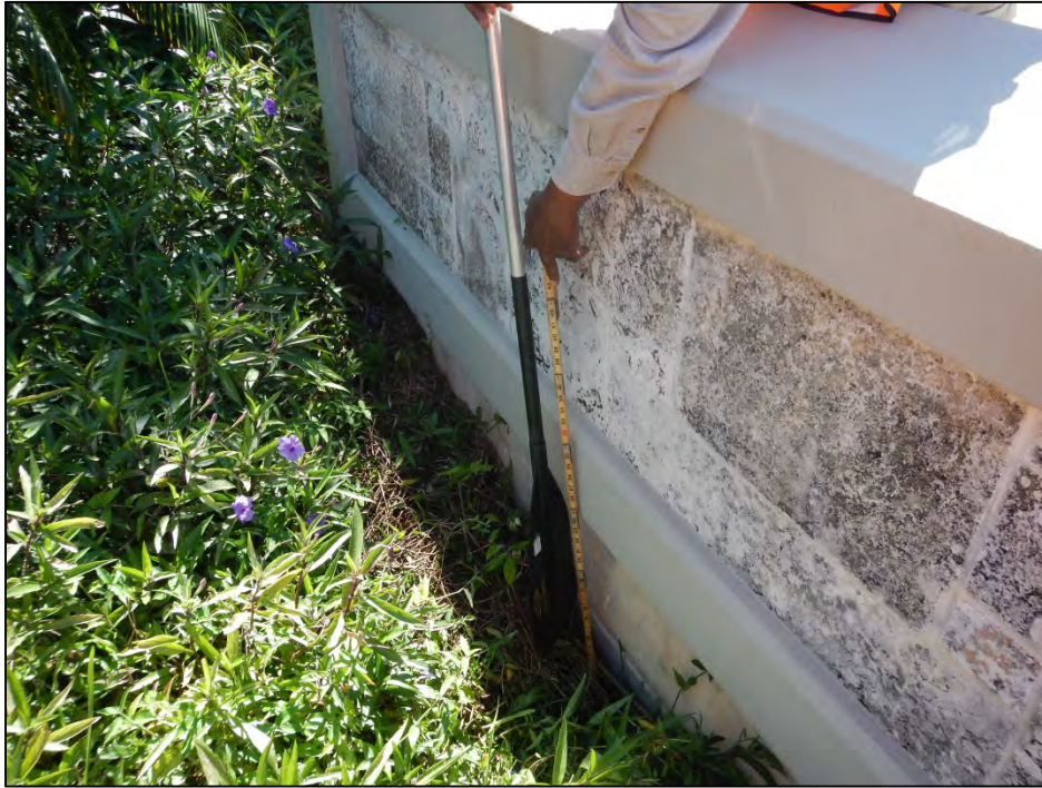
Photo 19 – Fill void at southwest wingwall.
