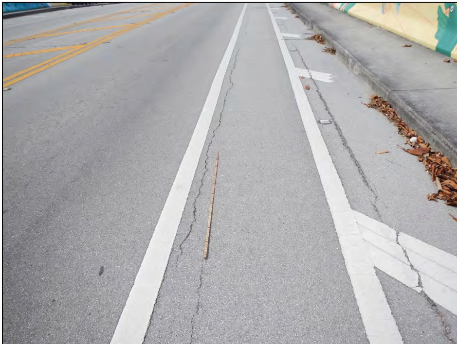
Photo 2 – Longitudinal cracks in asphalt over joints between slab units.
