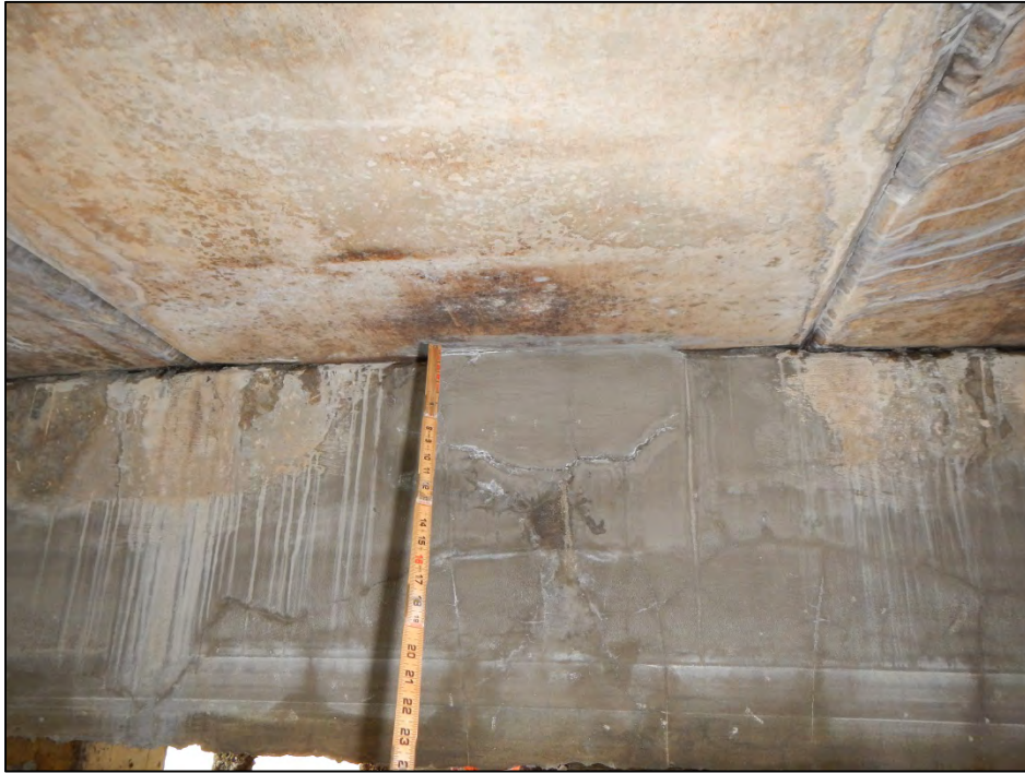
Photo 3 – Bent 2 cap delamination.
