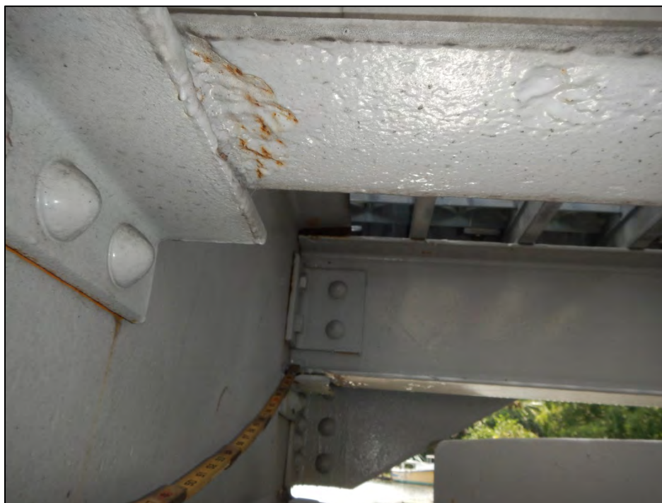
Photo 5 – Typical pitting and section loss at stringers.
