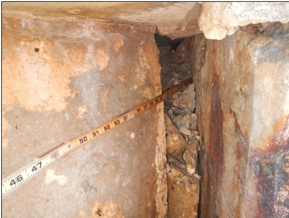
Photo 8 – Southeast corner open transition joint in the wingwall.
