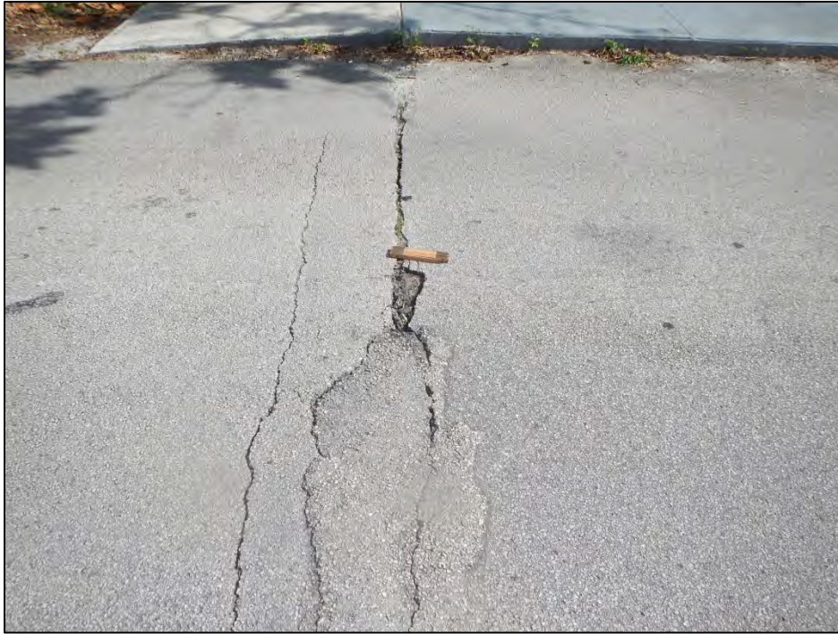
Photo 1 – Overlay exhibits transverse cracks at Abutment 2.
