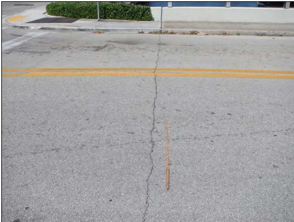
Photo 2 – Transverse crack in the asphalt overlay at Abutment 1.
