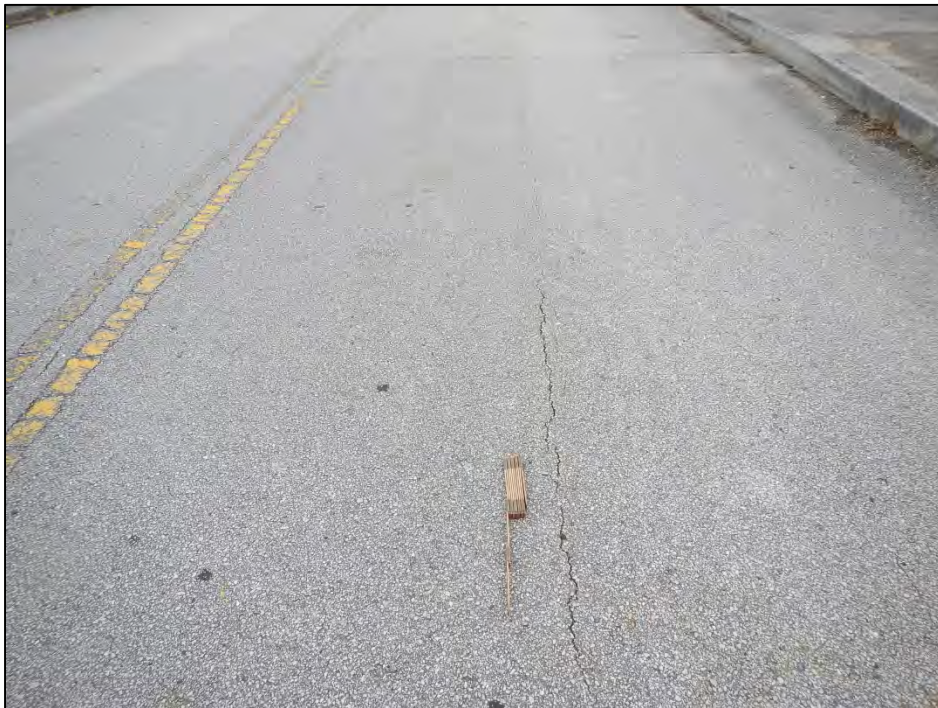
Photo 2 – Westbound deck top longitudinal cracks.
