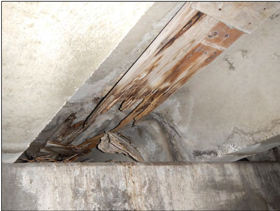
Photo 6 – Pieces of wood form-boards were left in-place along the beams.
