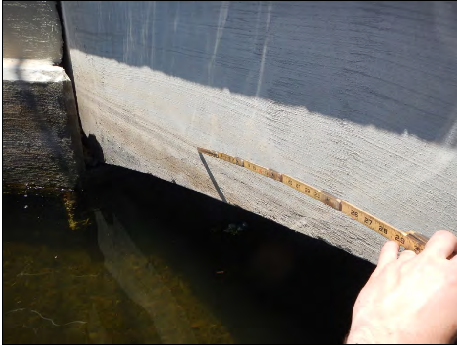
Photo 5 – Crack in east face of Span I near Abutment I.
