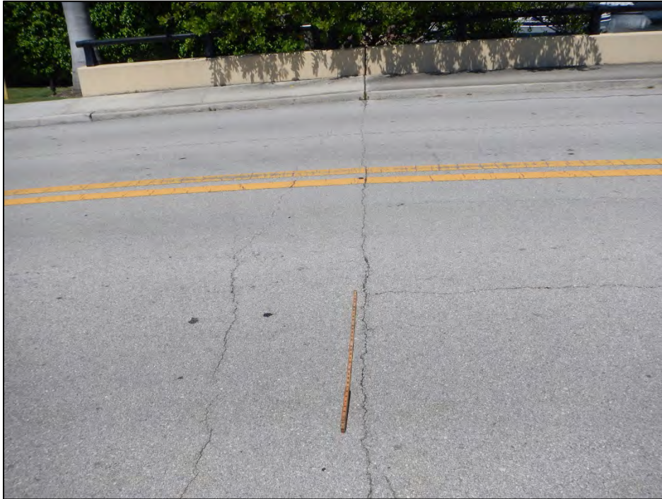
Photo 1 – Transverse cracks in asphalt overlay at Abutment 1.
