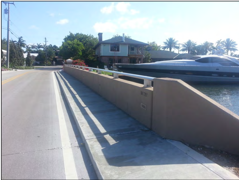
Typical Bridge Railing
