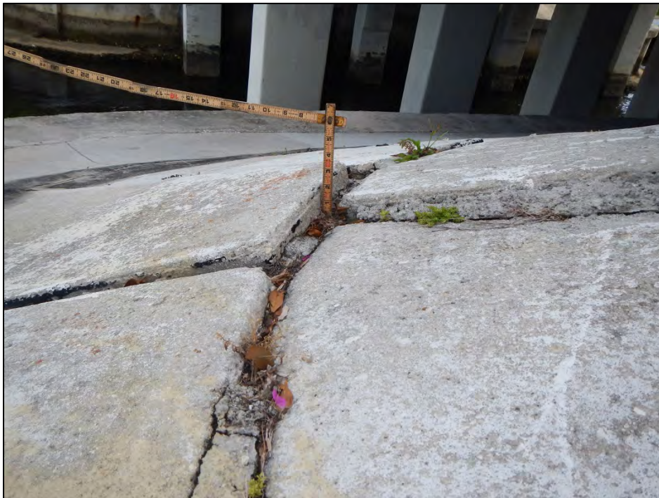
Photo 14 – The southwest slope protection exhibits settlement.
