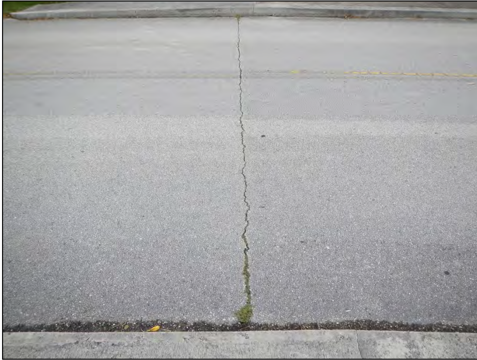
Photo 1 – Abutment 1 joint seal transverse crack.
