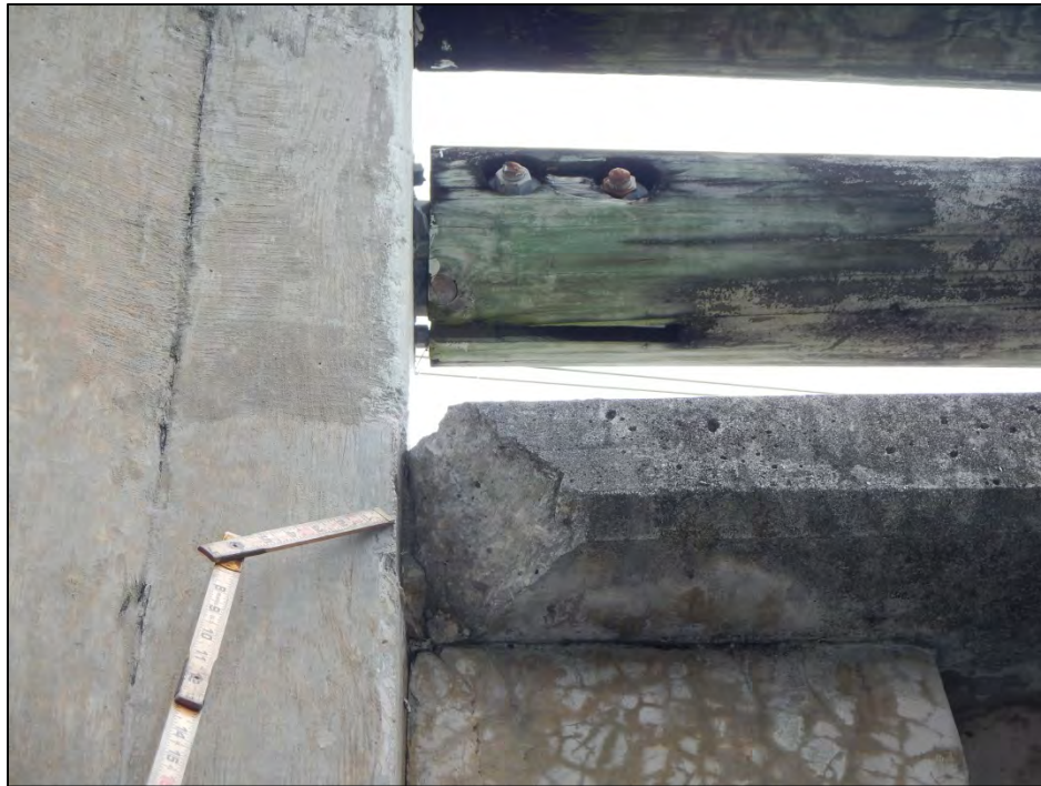
Photo 5 – The east end of the north fascia exhibits a spall over Abutment 2.
