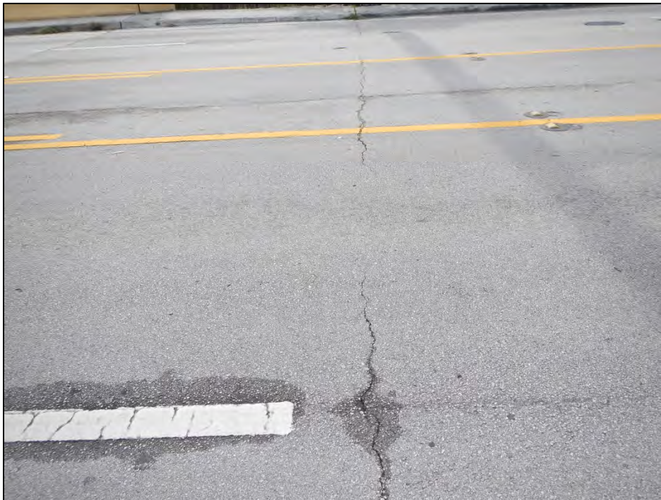
Photo 16 – Approach slab roadway transverse crack.
