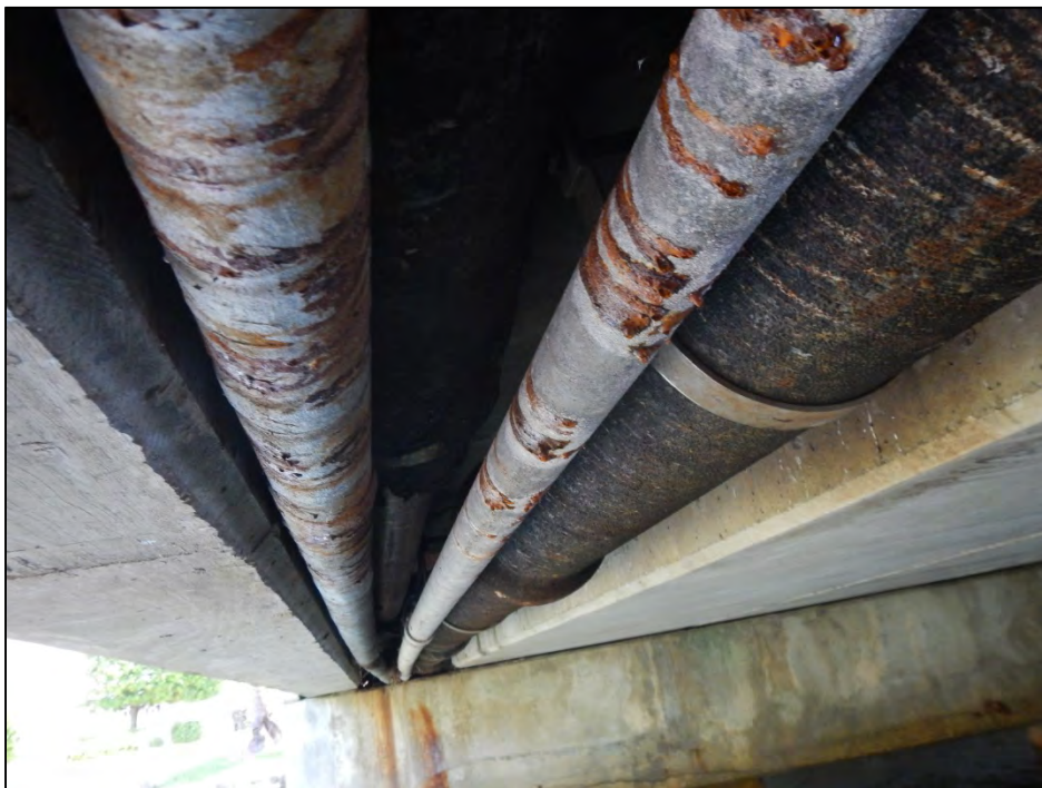
Utilities Mounted Adjacent to Slab Unit
