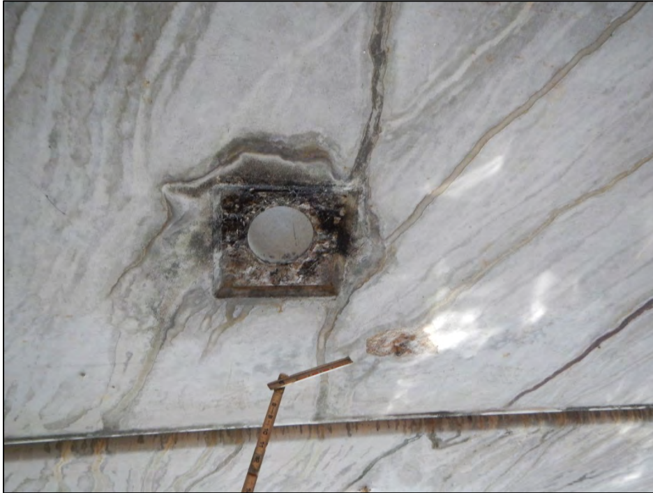
Photo 5 – Spalls near vent holes in Slab 1-2.
