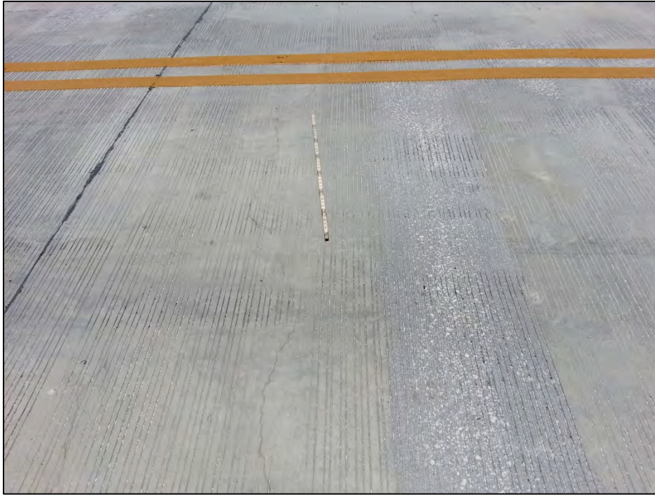
Photo I – Cracks in the Deck Top.
