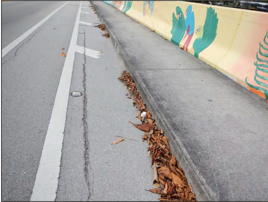
Photo 3 – Dirt and Debris in shoulder area.
