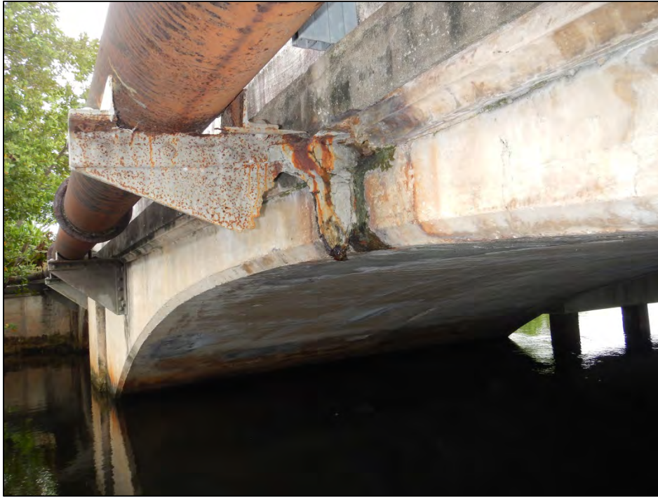
Photo 11 – Utility pipe support at the east side with 100% section loss.
