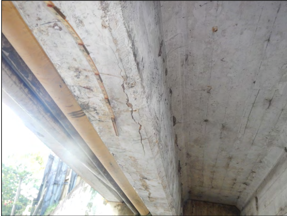
Photo 11 – The bottom face of Beam 1-2, 8 ft. from Abutment 2, exhibits a delamination.
