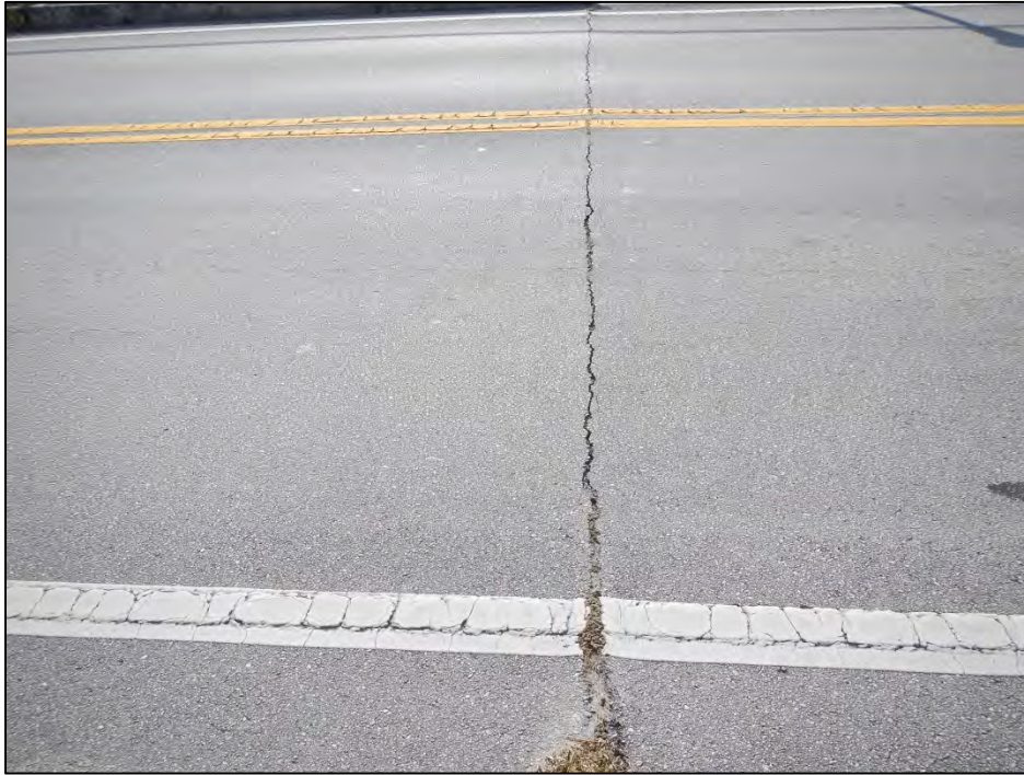
Photo 1 – End Bent 1 joint seal transverse crack.
