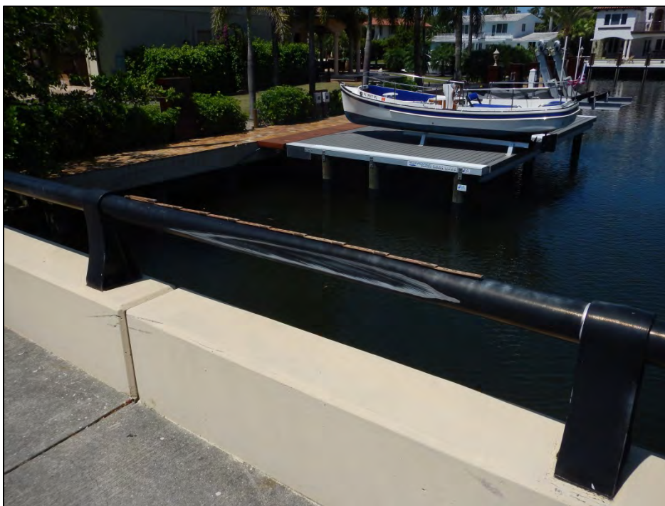
Photo 3 – Impact damage to aluminum rail in Span 2.
