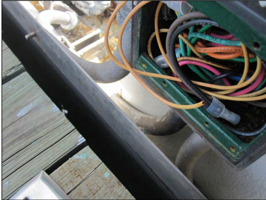
Photo 19 – Uncapped conductor within junction box feeding Lock A.
