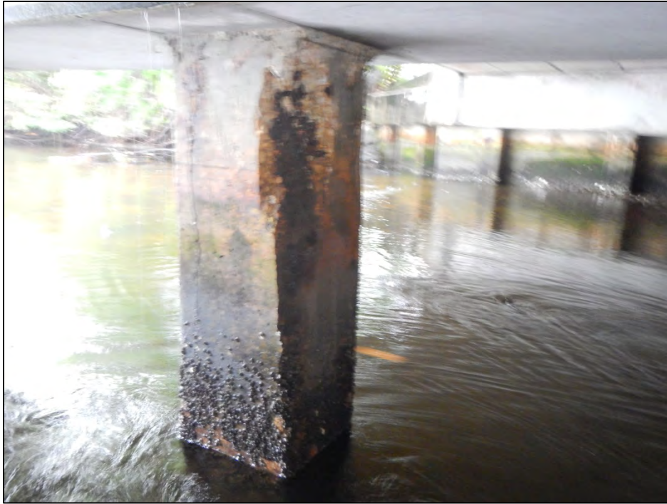
Photo 17 – All faces of Pile 3-2 exhibit spalls with associated cracks with corrosion bleed-out.
