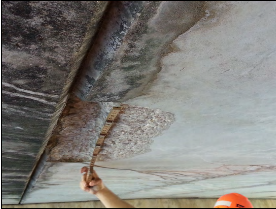
Photo 5 – Spall in Slab Unit 3-6.
