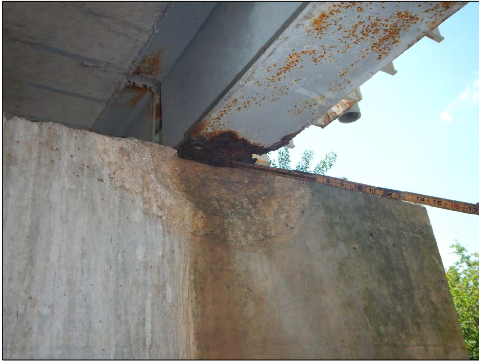
Photo 3 – Section loss on Beam 2-I. Note spall in Bent 2 cap.
