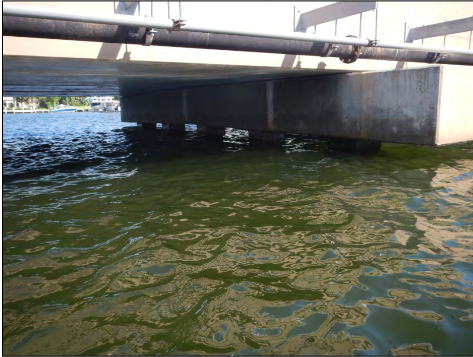
Typical Deck Underside and Intermediate Bent. Note Utility Pipe.
