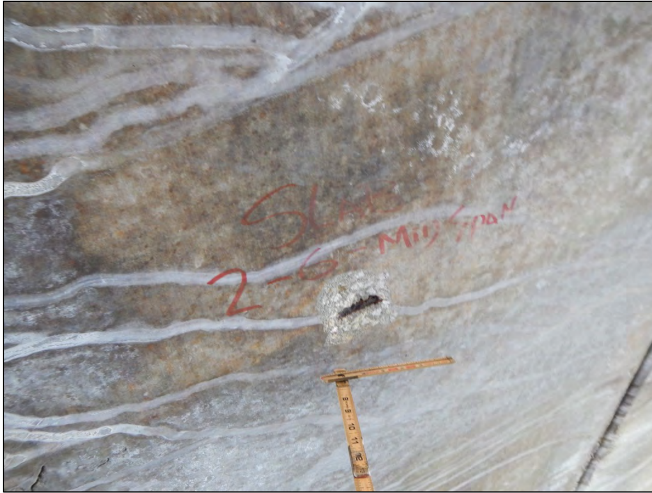
Photo 1 – Spall in the underside of Slab Unit 2-6.
