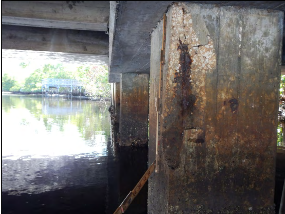
Photo 13 – The southeast corner of Pile 4-6 exhibits a spall with exposed steel.
