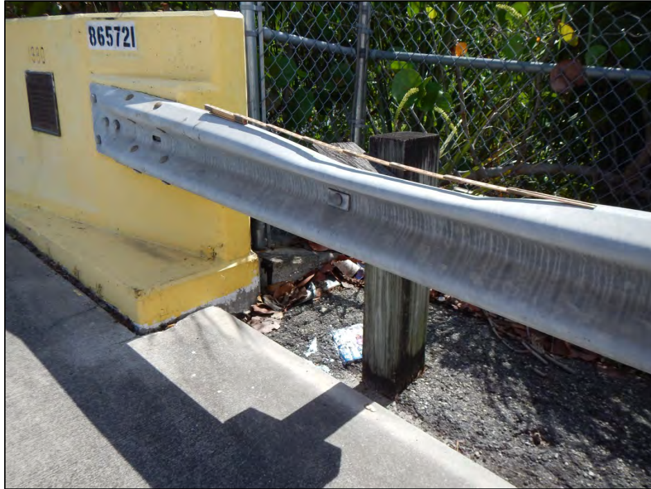
Photo 21 – Northwest guardrail impact damage.
