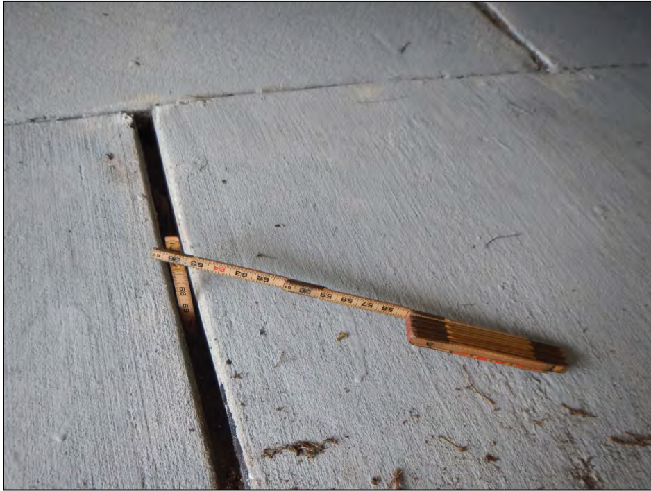
Photo 13 – Concrete panels are not sealed below Slab Unit I-10.
