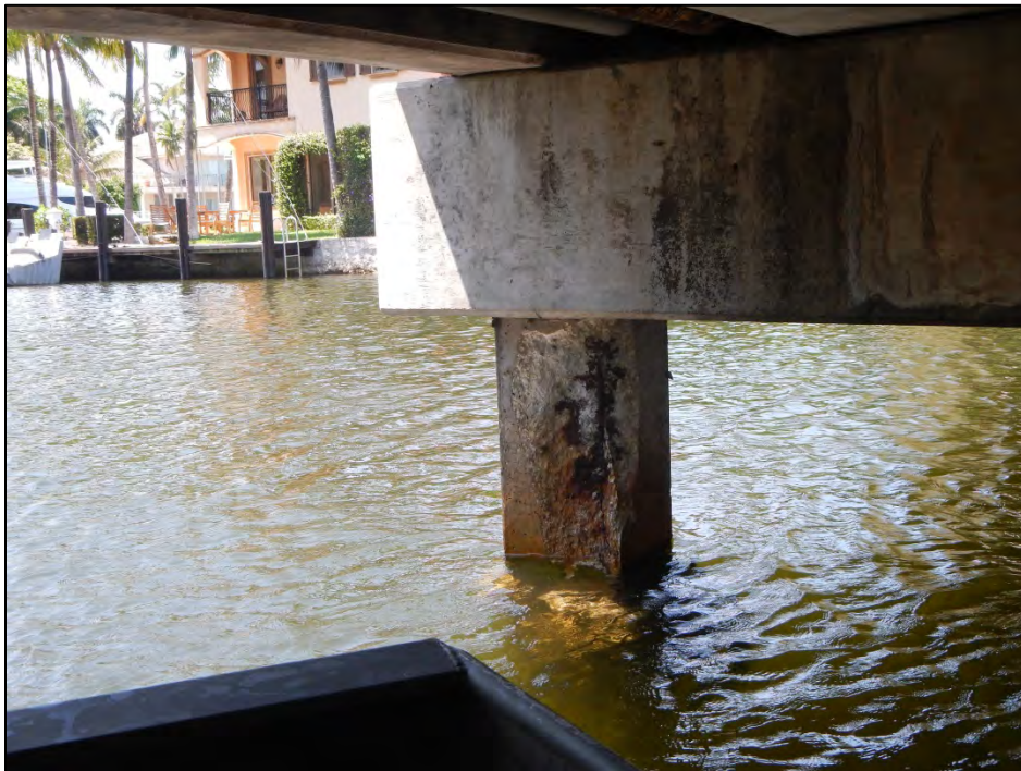
Photo 10 – Spall with exposed corroded steel at the southeast corner of Pile 2-1.
