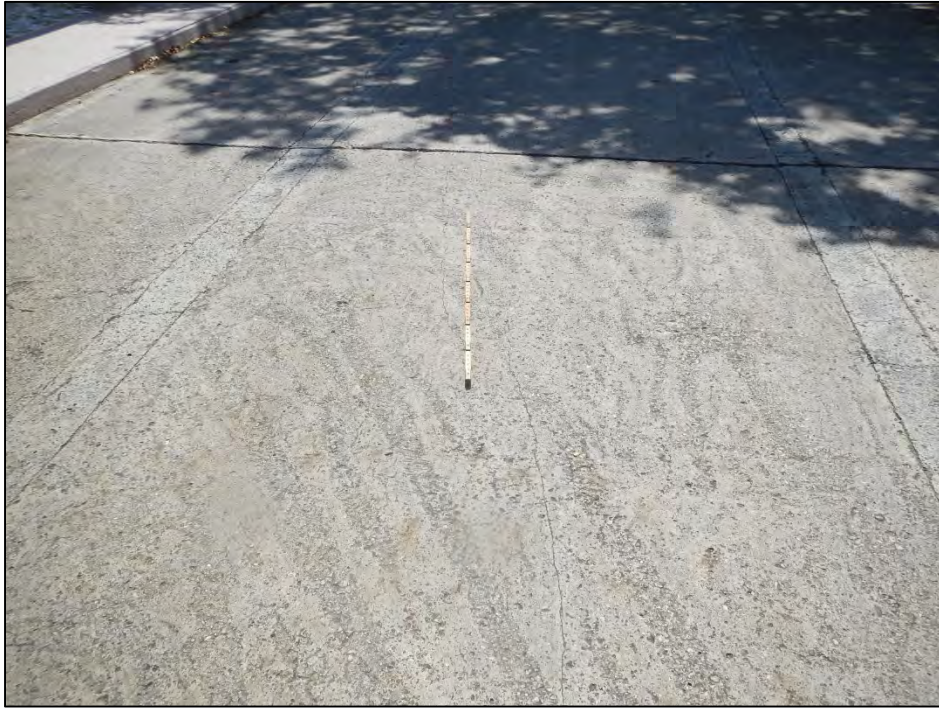
Photo 5 – The deck top over Span 2 exhibits longitudinal cracks.
