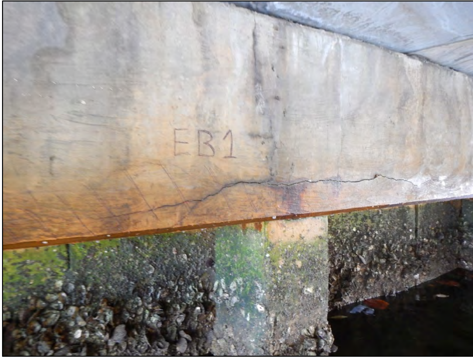
Photo 3 –Delaminations and cracks in the End Bent 1 cap.
