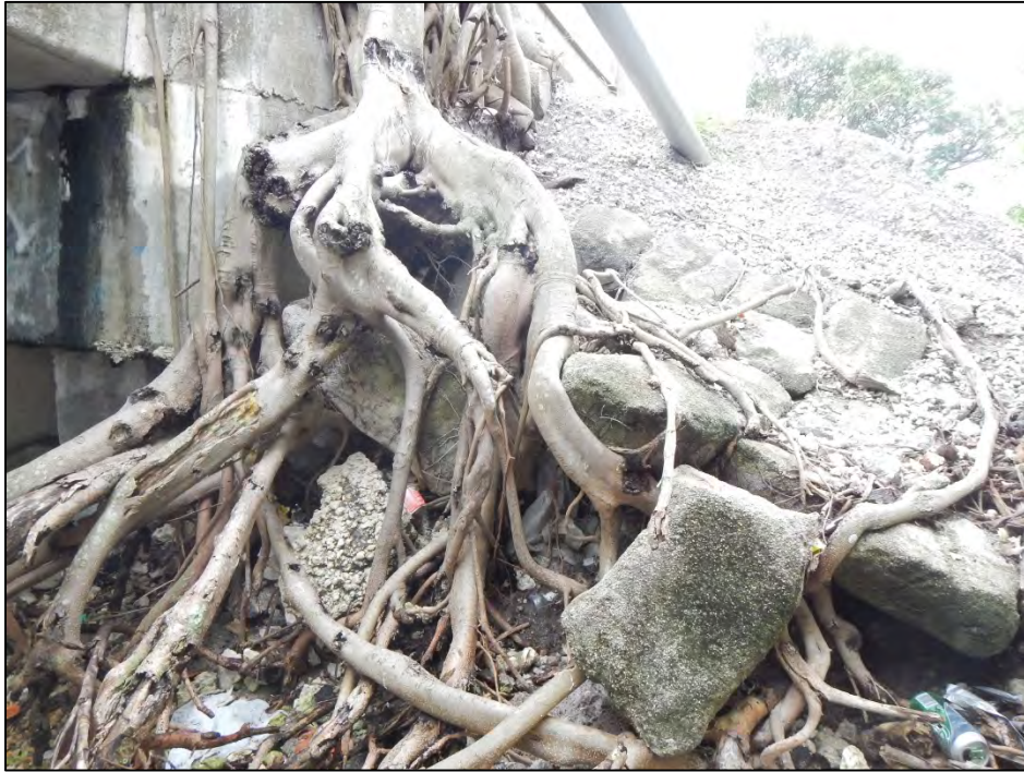
Photo 7 – Tree root is undermining the west end of End Bent 1.
