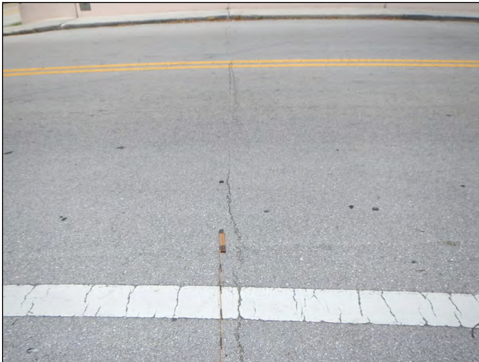
Photo 4 – The deck top exhibits a transverse crack over Bent 3.
