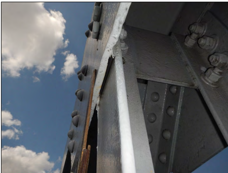
Photo 14 – Bent gusset plate at west top chord U11 connection to vertical member.
