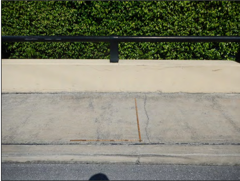
Photo 3 – Cracks in southwest approach sidewalk.
