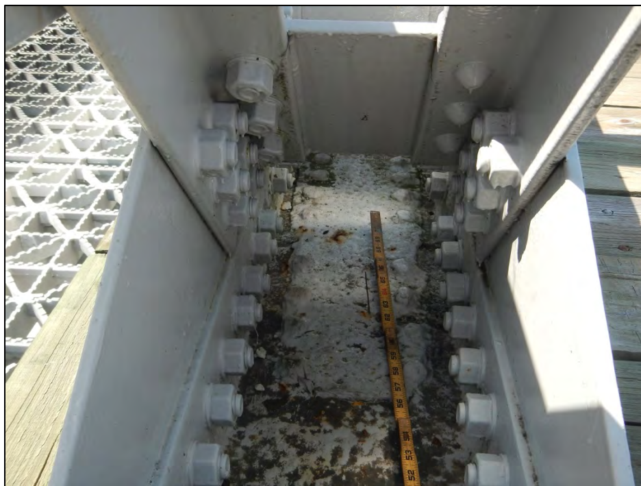
Photo 10 – Typical corrosion with section loss on splice plates and connection bolts.
