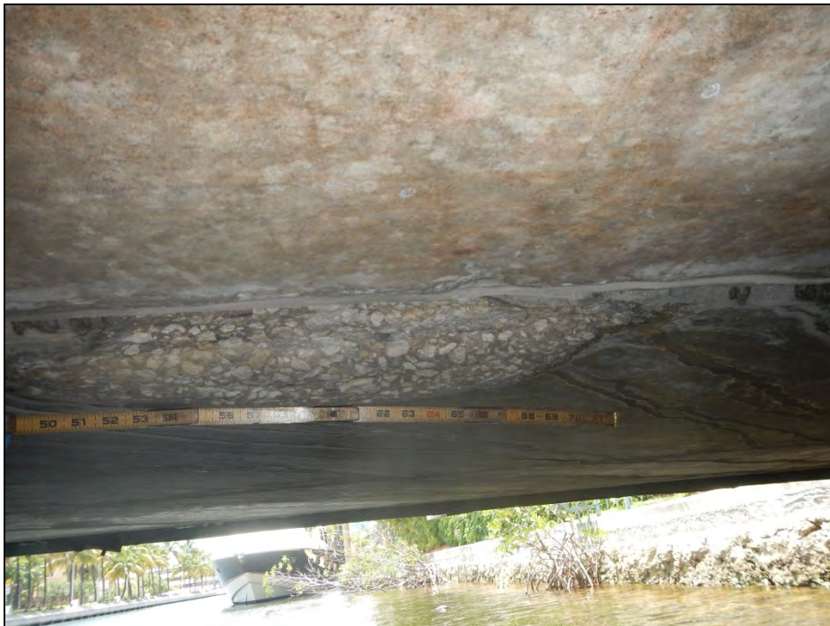
Photo 6 – Spall in Slab Unit 3-1.
