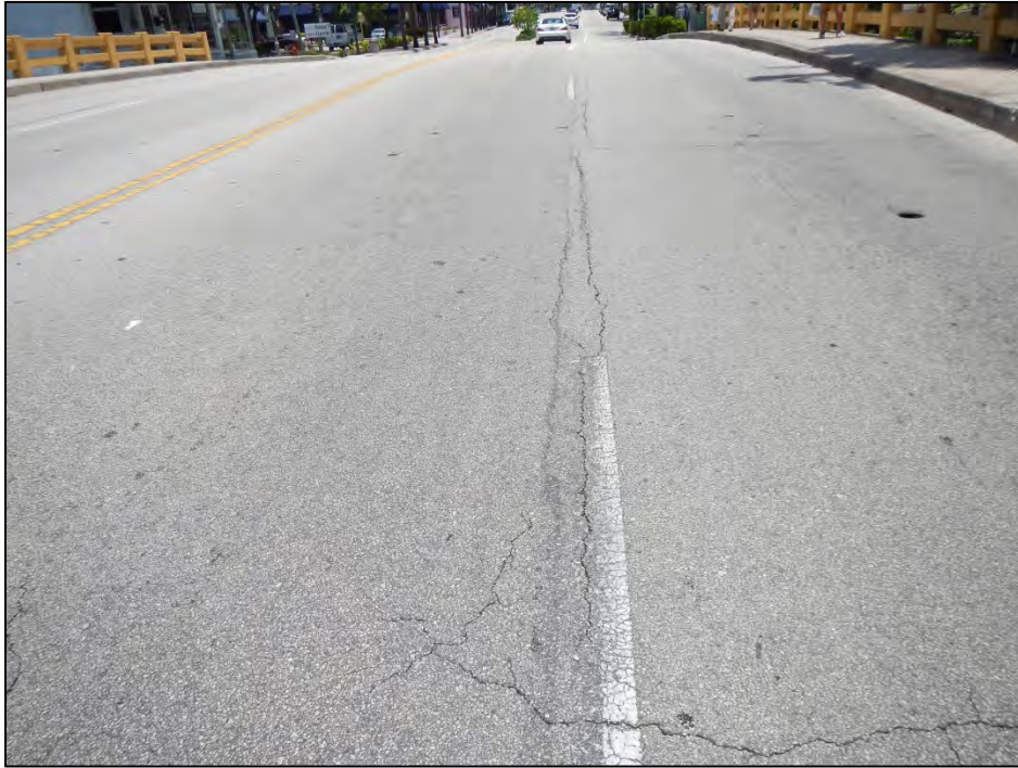
Photo 7 – The south approach slab exhibits longitudinal cracks.
