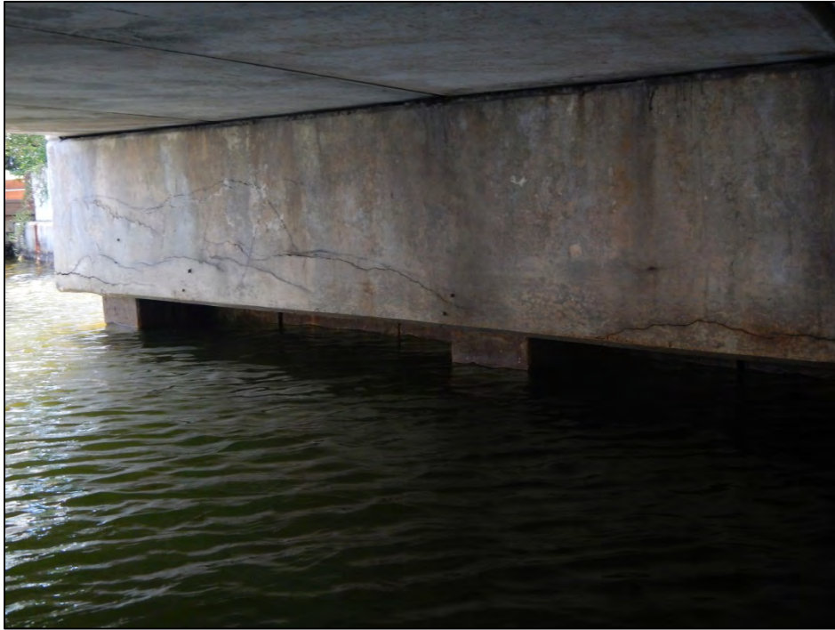
Photo 7 – Delaminated area in Abutment 1 cap.
