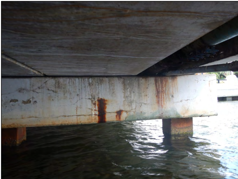
Photo 14 – Corrosion staining on Bent 2 cap.
