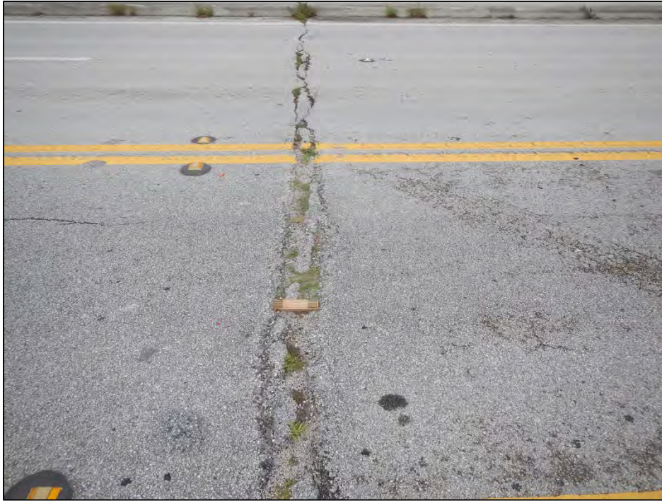
Photo 1 – Bent 2 joint seal transverse crack.
