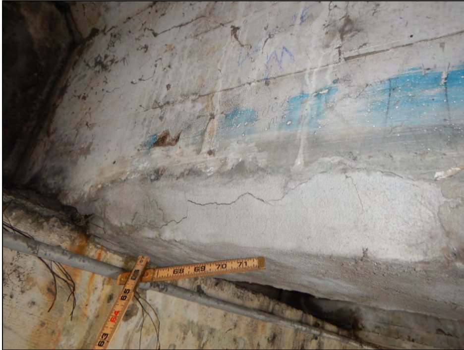
Photo 13 – Beam I-7 over Abutment I exhibits a delamination.
