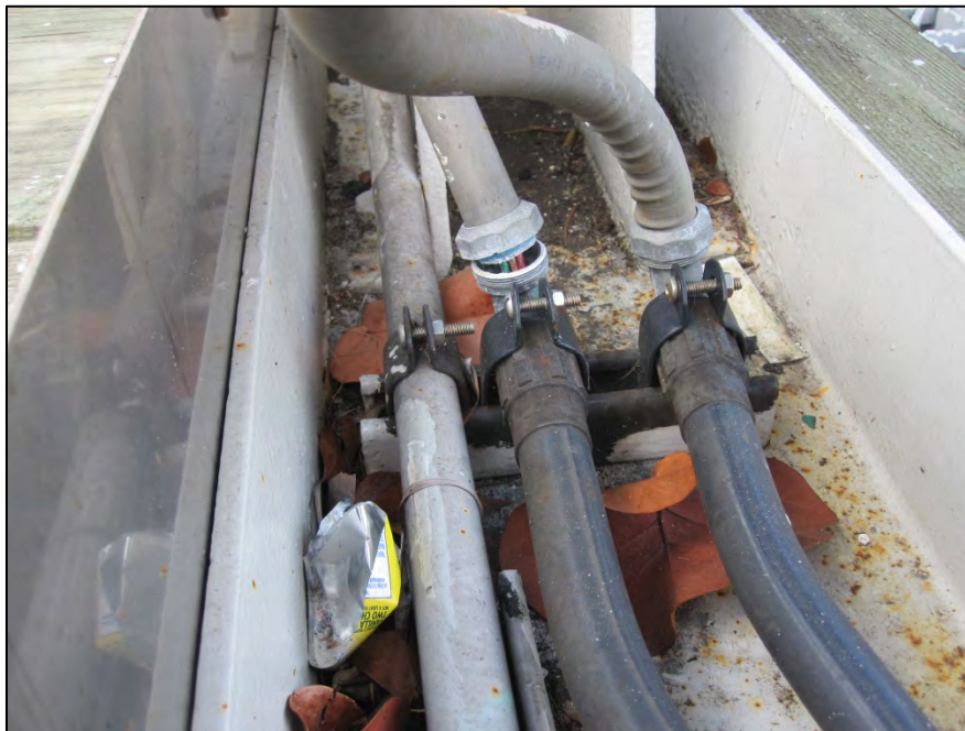
Photo 22 – Insecure flexible conduit fitting at Lock B.
