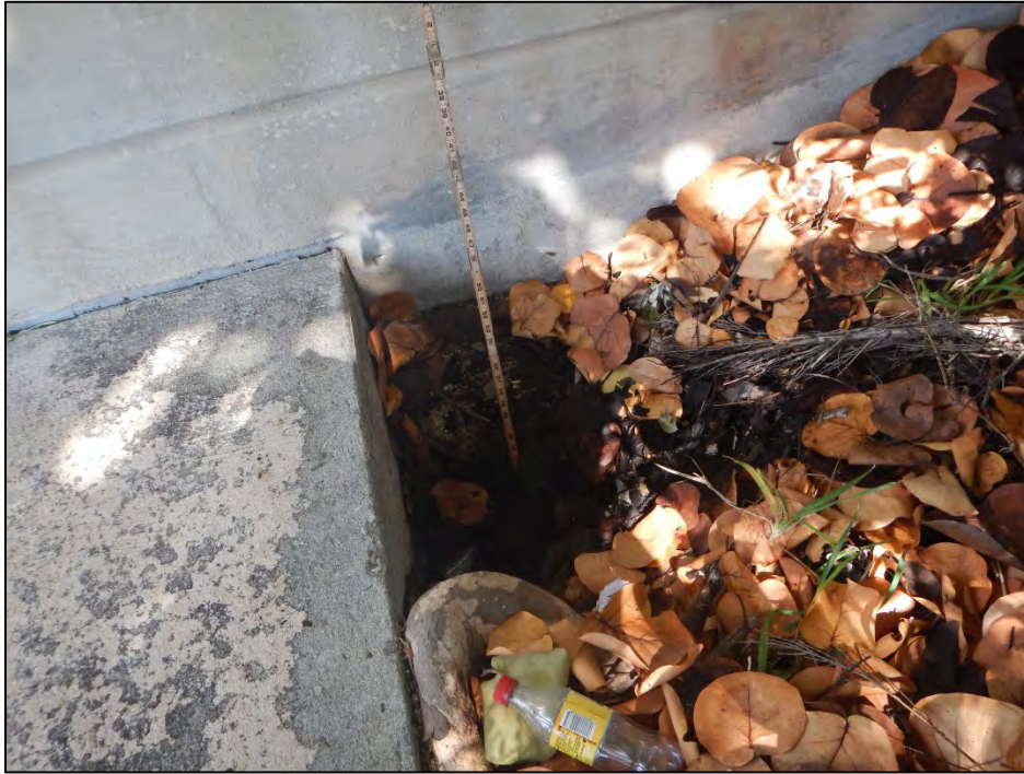
Photo 5 – Open retaining wall joint and backfill void at the northeast corner.
