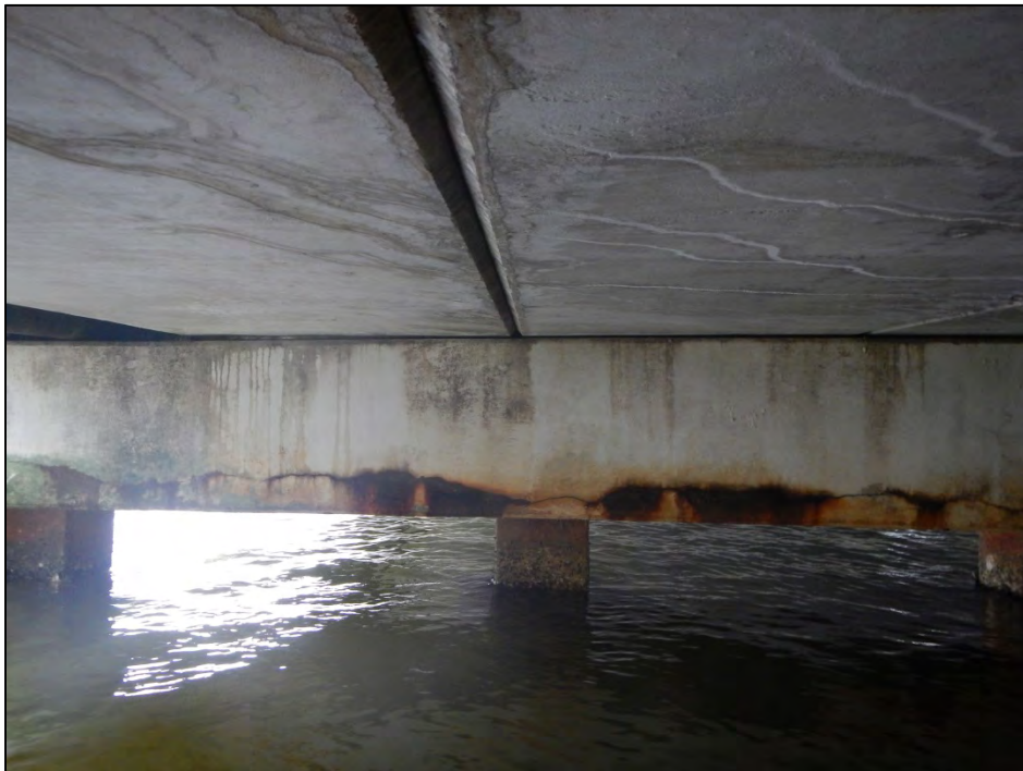
Photo 12 – Delamination in north face of Bent 3 cap.
