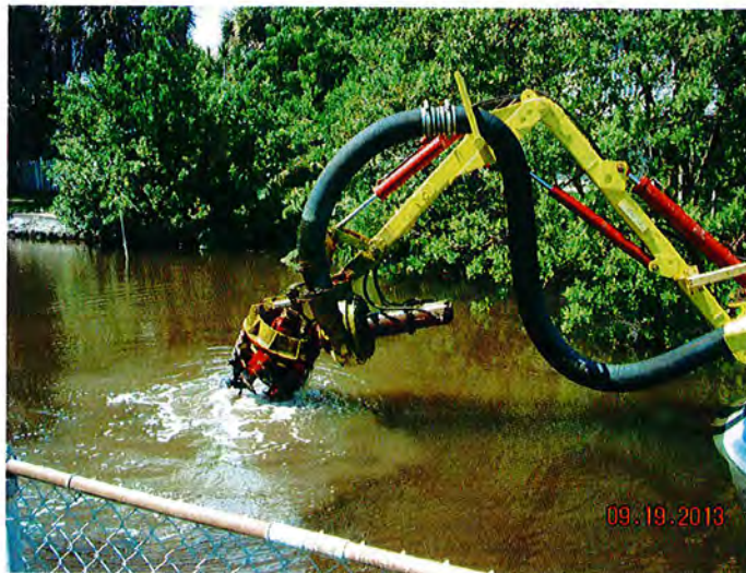
Canal Dredging by Hydraulic Method (Picture 5)
