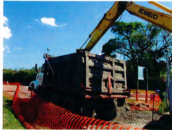
Loading to Water-tight Trucks (Picture 7)
