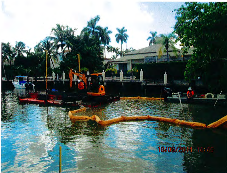
Canal Dredging by Mechanical Excavation Method (Picture 3)
