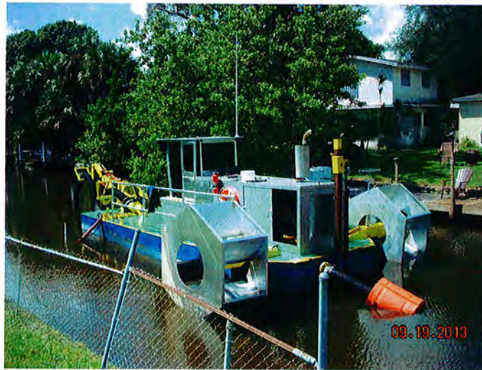
Canal Dredging by Hydraulic Method (Picture 4)
