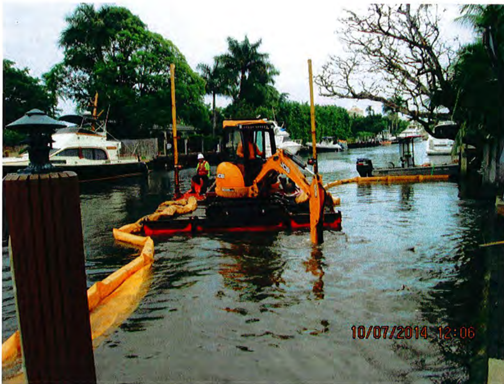
Canal Dredging by Mechanical Excavation Method (Picture 1)
