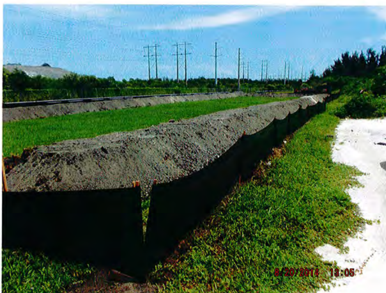
Drying Basin Located at Compost Facility Site, City of Dania Beach (Picture 8)
