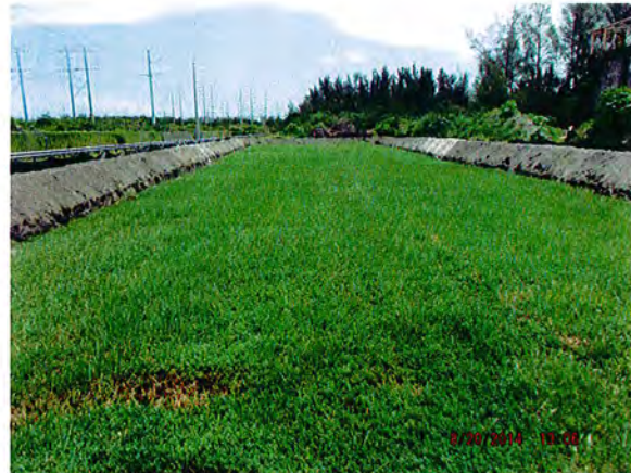
Drying basin bottom (Picture 10)
