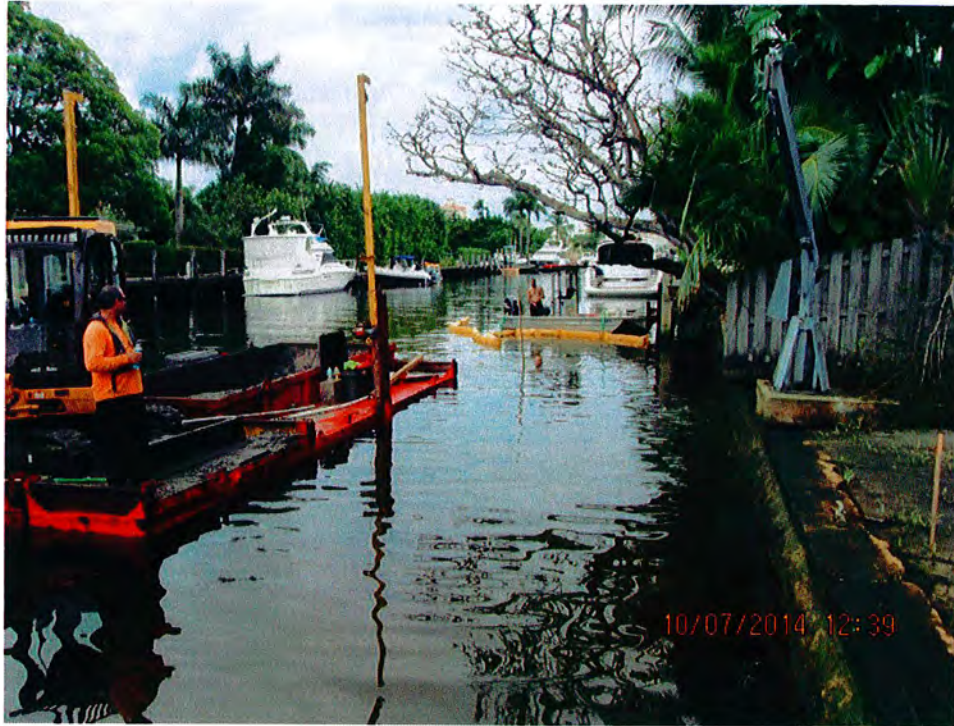
Canal Dredging by Mechanical Excavation Method (Picture 2)
