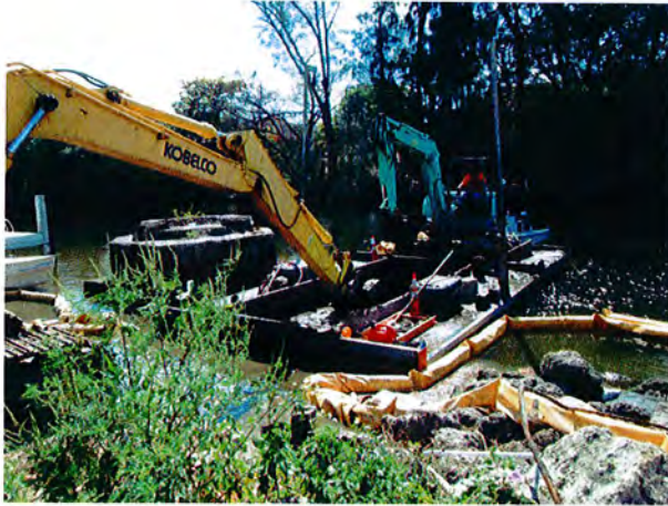
Hauling from Barge (Picture 6)
