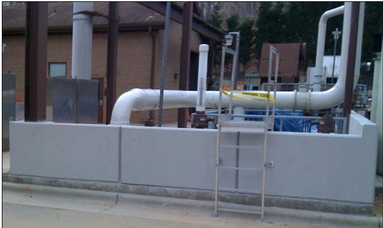
Figure WW13-6. Flood Wall
