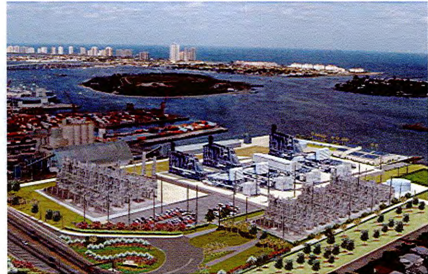
FPL's Riviera Beach Next Generation Clean Energy Center, 2014
