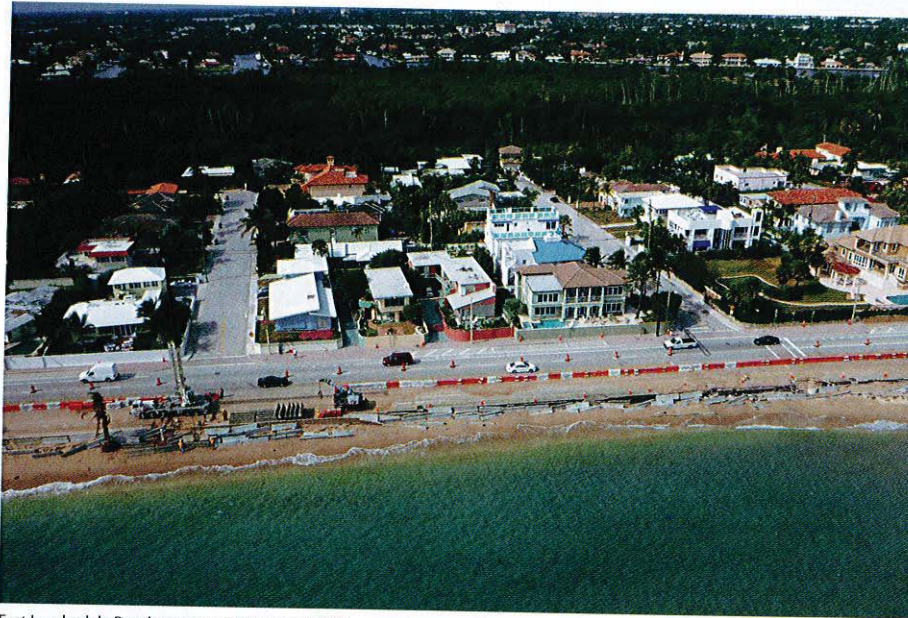
Fort Lauderdale Beach erosion in November 2012.
